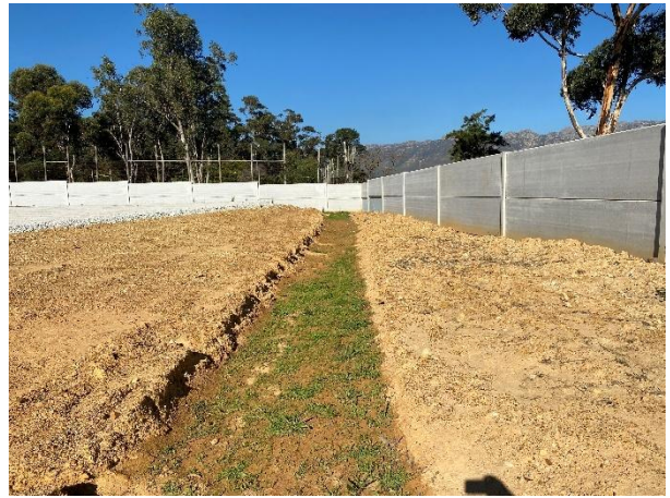
Trenches are currently being excavated for the installation of the bulk stormwater pipeline.
