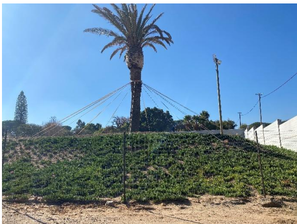
Anchoring of the palm tree using cables and ropes to stabilise the tree for landscaping.
