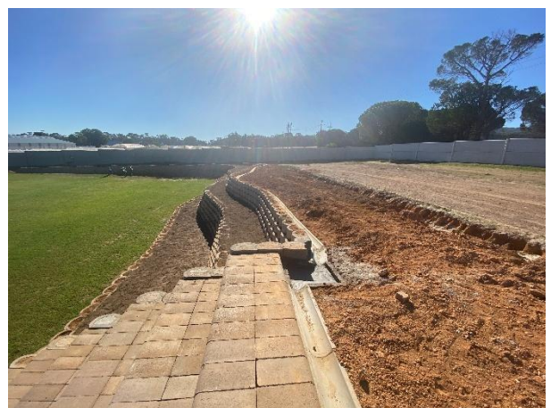
The northeastern Field B embankment, pavilion, and concrete retention wall have been constructed.
