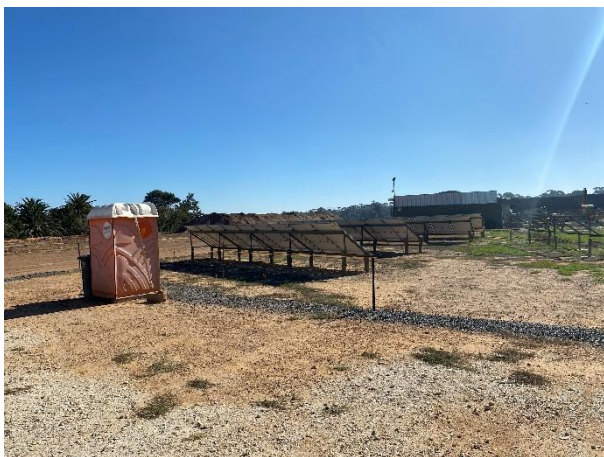
Solar panels temporarily installed and utilised until the completion of the parking area.
