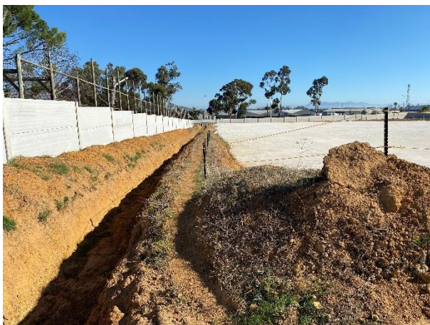
Preparation for the installation of the bulk stormwater pipeline along the eastern boundary of Field C.
