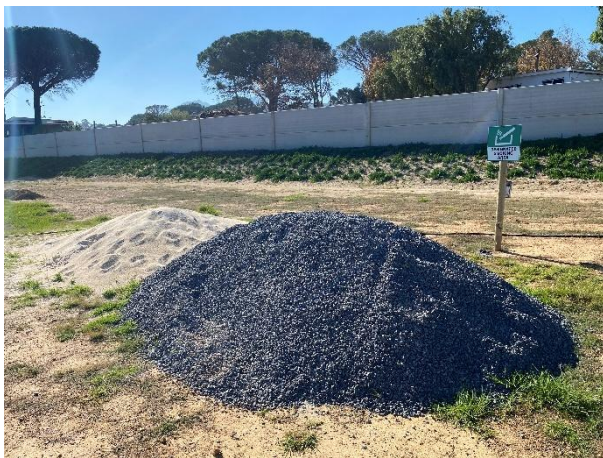
Temporary building material stockpiles.
