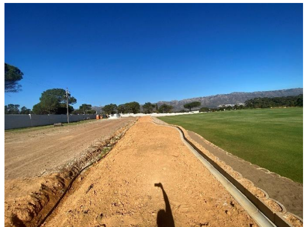
The northeastern embankment of Field B, to be landscaped along with accommodation pods placed.
