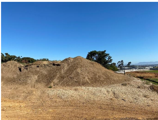
Temporary G5 material stockpiles for layered road works and levelling of the sports fields.
