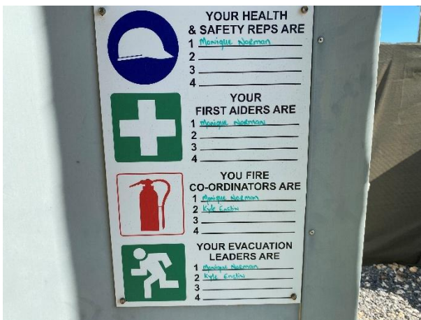
Site safety information board.
