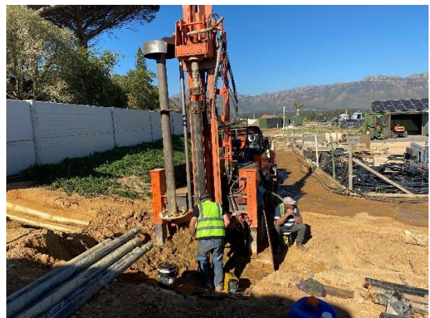
Borehole installation in progress towards the southeastern property boundary.
