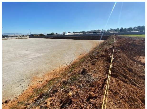
Field C embankment towards the east.
