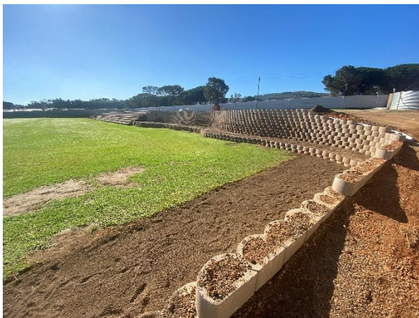
Condition and concrete retaining wall of Field B.
