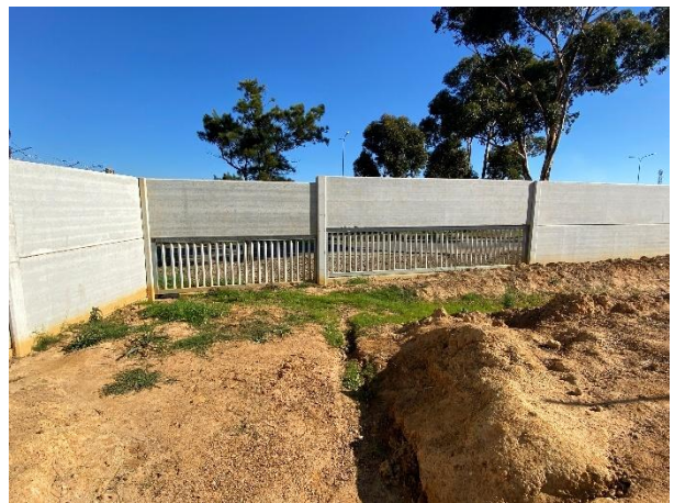
Stormwater outlet located in the western corner, along with the municipal water connection point
