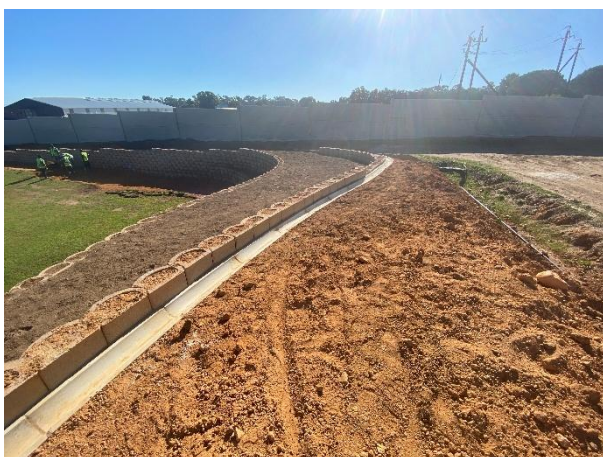
The northeastern embankment of Field B. Retention wall will be landscaped. Note the stormwater drain installed.
