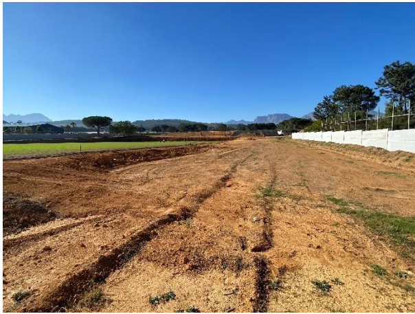
Southeastern property boundary adjacent to Field A, where the bulk stormwater pipeline will be installed.
