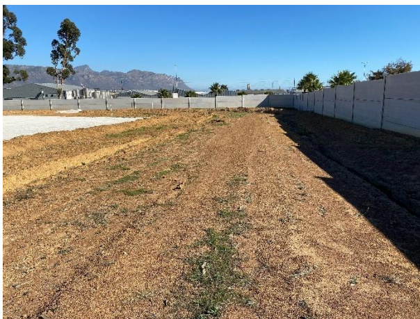
Cleared area designated for the reed bed and package plant installation.
