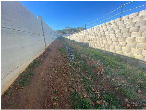
Temporary stormwater measures in place adjacent to the northern corner of Field B.
