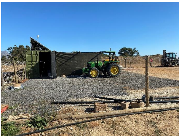
Condition of the demarcated and contained contractor's yard.
