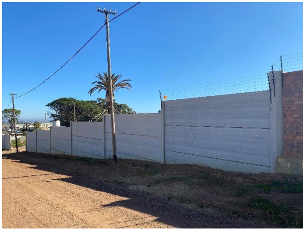
Entrance of the site off Mondeor Road where the boundary wall has been constructed.
