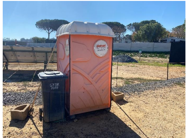
Secured chemical toilet and bins in place adjacent the current works area.
