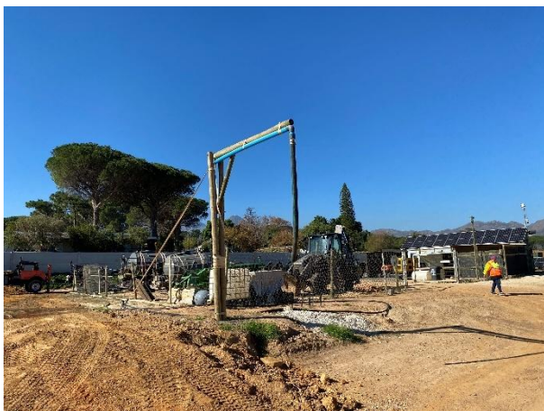
Water filling station for dust suppression.
