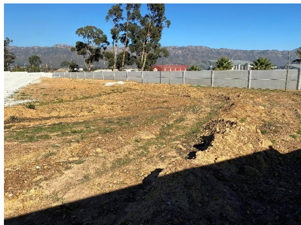
Area cleared and being levelled in preparation for attenuation pond construction.
