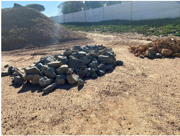
Rock stockpiles use for temporary stormwater mitigation where necessary.
