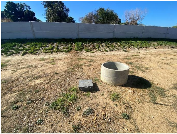
Southeastern borehole located at the entrance of the site towards the right.
