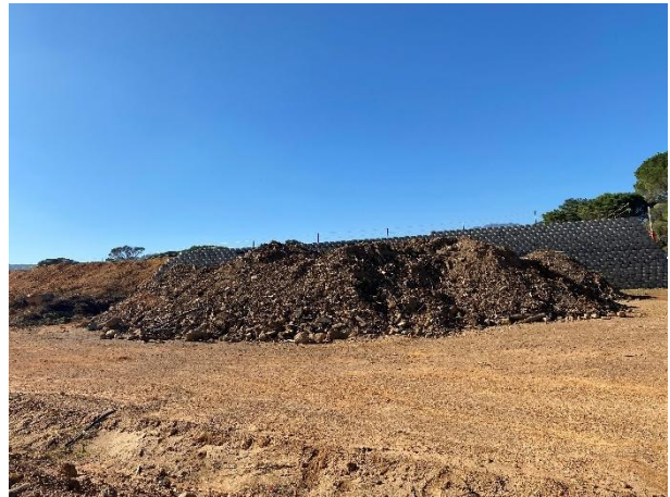
Temporary topsoil and mulch stockpiles continuously used.
