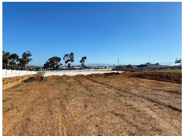
Field C embankment towards the east.
