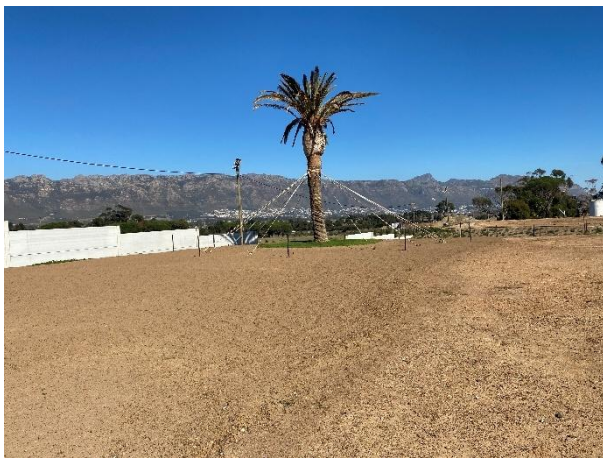
Towards the entrance of the site where the workshop will be located.
