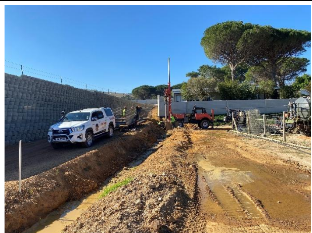
Borehole and stormwater installation in progress towards the southeastern property boundary.
