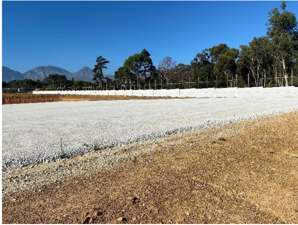
Field C prepared and cemented for sand-based astro field installation.
