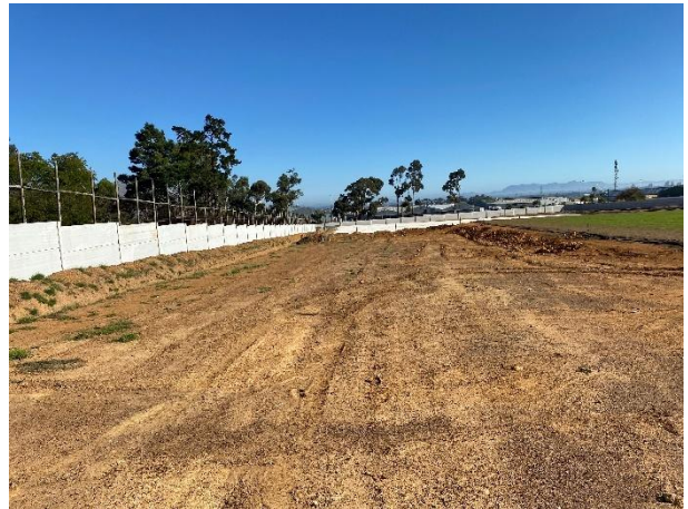
Field C embankment towards the east.
