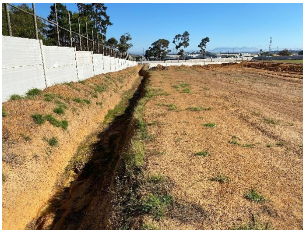
Preparation for the installation of the bulk stormwater pipeline along the eastern boundary of Field A
