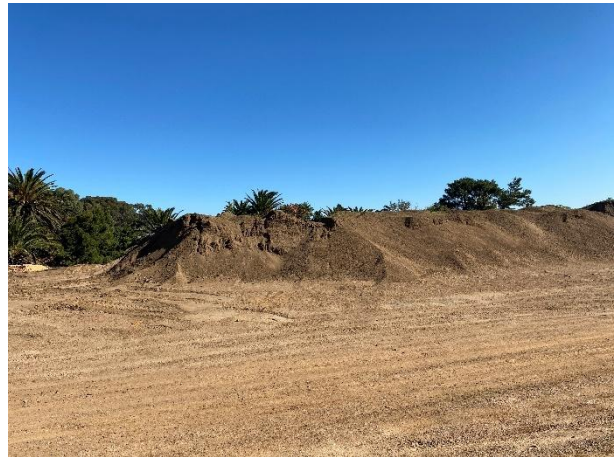
Temporary G5 material and topsoil stockpiles for layered road works and levelling of the sports fields.
