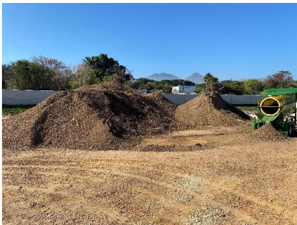
Sieved material stockpiles at the entrance of the site where the workshop will be located.
