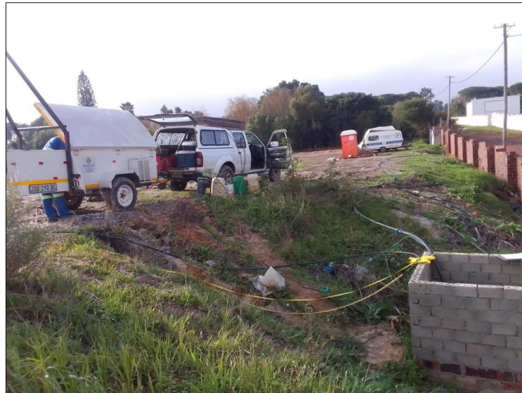
Figure 12: Borehole testing set up a few meters away from the HP_BH4.
