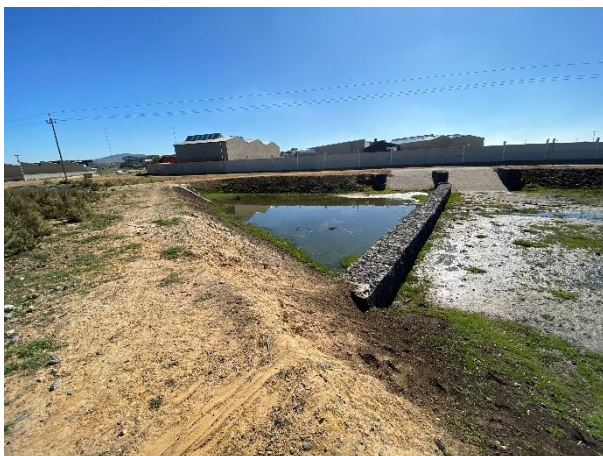
The new dry pond forebay.
