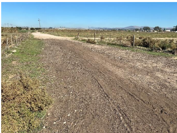
Composted and rehabilitated temporary access road.
