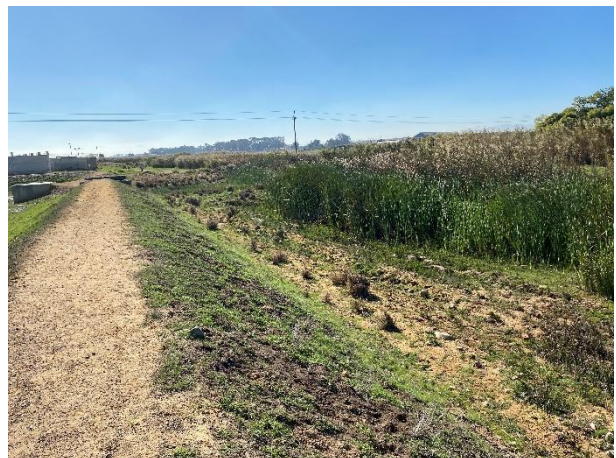
Eastern embankment of the dry regional pond adjacent to the wetland area of the Mosselbank River.
