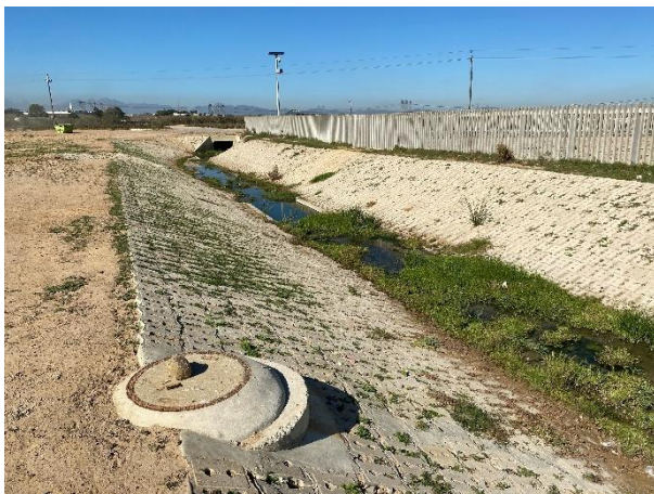
Construction and enlargement of Channel 1 along the existing outlet channel of the temporary pond.
