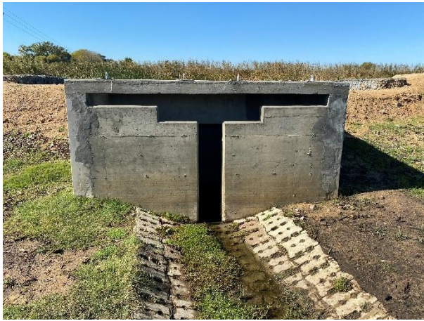
Outlet structure with weir openings and flapgate.
