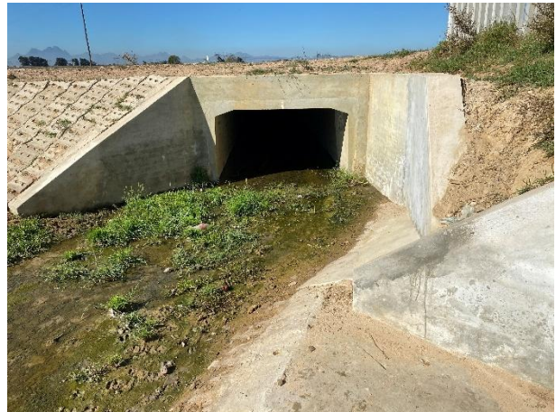
Culvert headwall along Channel 1 underneath Brass Avenue gravel access road.
