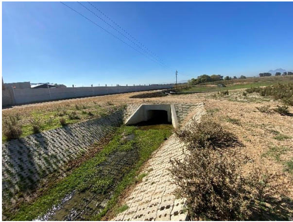
New box culvert inlet to the new dry pond forebay as seen towards the east.
