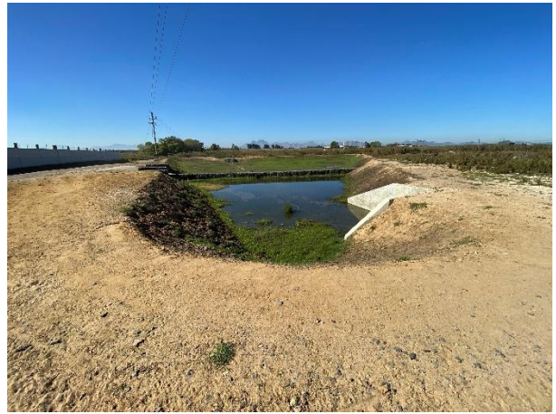
The new dry stormwater pond as seen from the west towards the east.
