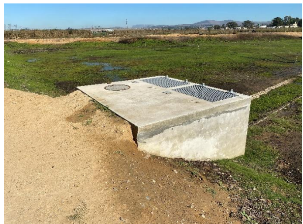
Outlet structure with weir openings and flapgate.
