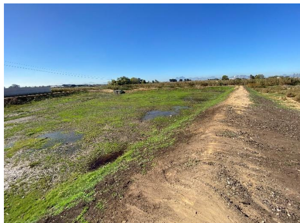
The new dry stormwater pond.
