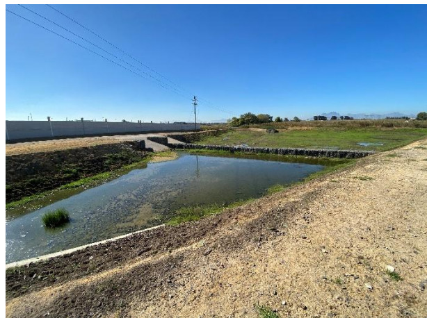
The new dry pond forebay.
