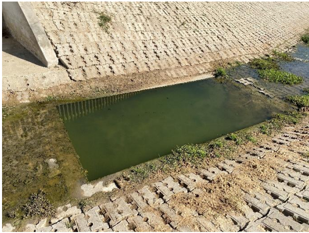
Central channel cunettes constructed along the enlarged Channel 1 to assist in low-flow conveyance and drainage.
