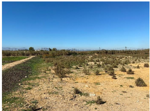
The condition of the temporary stockpile area as seen immediately south of the new pond towards the south.
