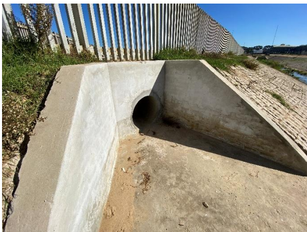
The stormwater culvert currently serving as an overflow diversion towards the decommissioned temporary pond.
