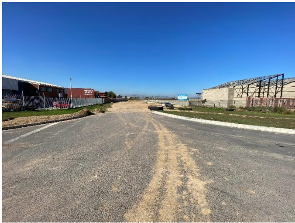
Access to the site off Darwin Road as seen towards the site. Some sand from the site is evident at the time.
