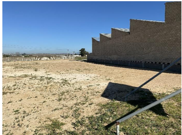
The previous temporary stormwater pond has been decommissioned and filled in.
