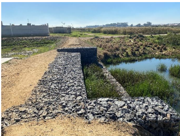
Gabion spillway drop structure with stilling basin as seen towards the east.
