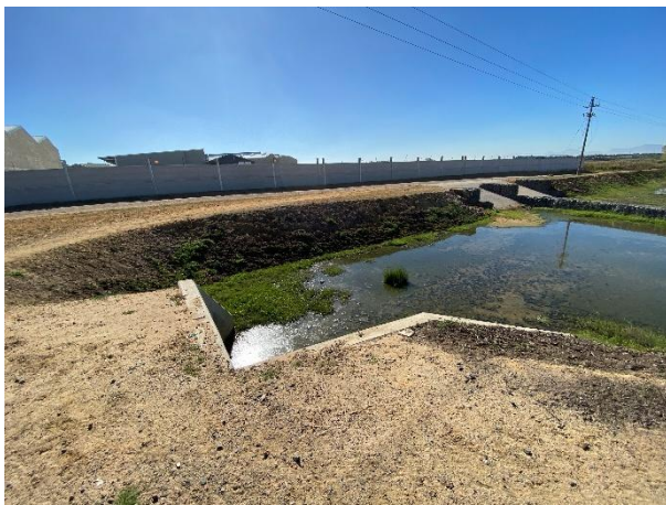
The new dry pond forebay.
