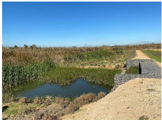
Gabion spillway drop structure with stilling basin as seen towards the south.
