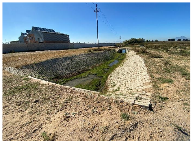
Channel 2 towards the box culvert inlet to the new wet pond forebay as seen towards the east.
