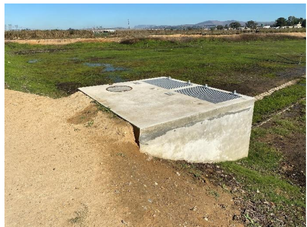
Outlet structure with weir openings and flapgate.
