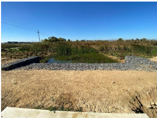
Gabion spillway drop structure with stilling basin.
