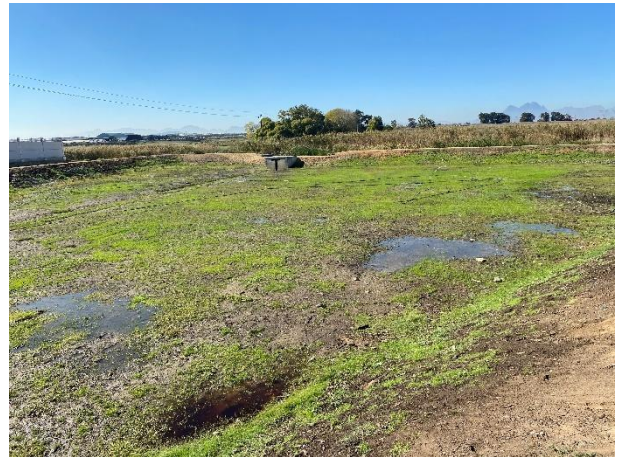
The permanent pool of the regional pond being irrigated, seeded with Bermuda grass.
