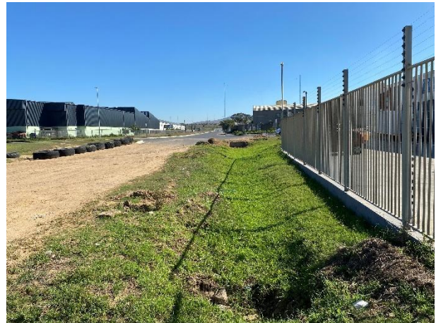
Roadside channels within the road reserve of Darwin Road.
