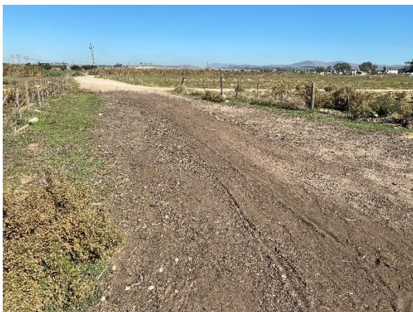
Composted and rehabilitated temporary access road.
