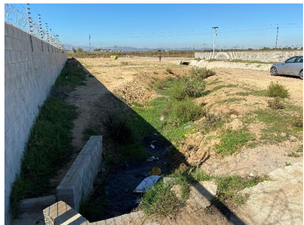
Roadside stormwater culvert channels within the road reserve of Darwin Road.
