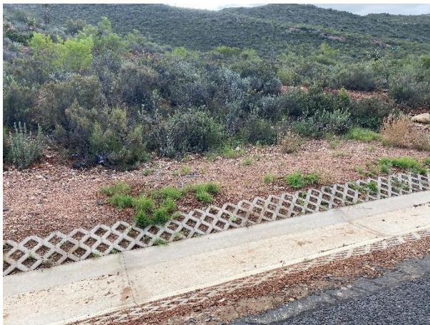
Upgraded side drains off MR 365.
