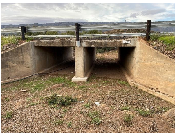
Removal of vegetation overgrowth and silt deposits.
