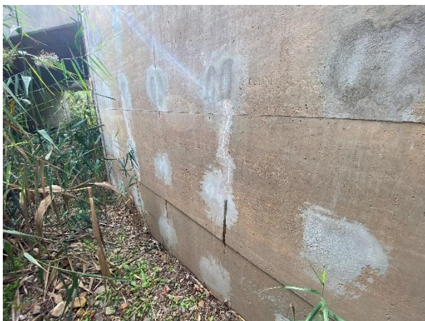
Repairing of cracks.
