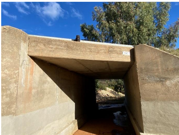
Replacement of the missing culvert number.
