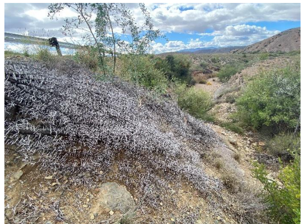
Condition of the vegetation surrounding the culvert.
