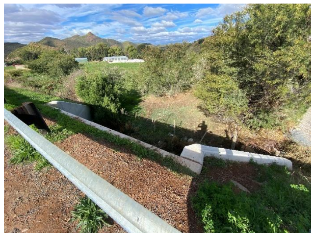
Condition of the vegetation surrounding the culvert. Fencing in place.
