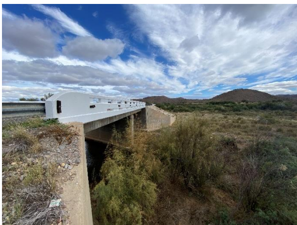
Condition of Bridge 4838.
