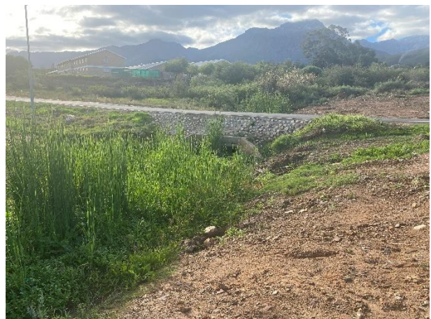
Overgrown vegetation due to the recent rainfall.
