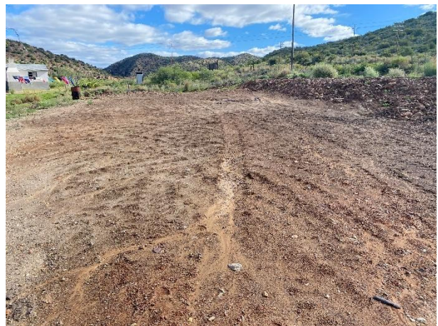
Condition of the former bitumen storage area within the construction camp.
