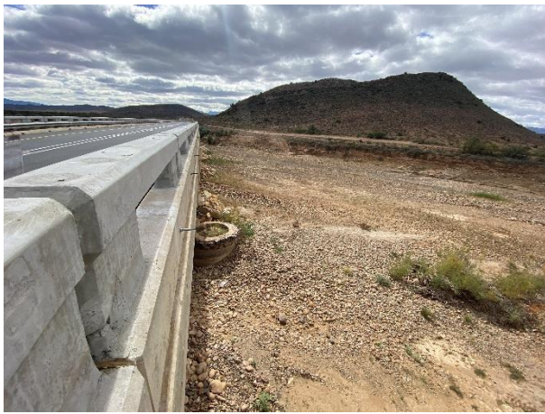
Condition of the vegetation surrounding the bridge.
