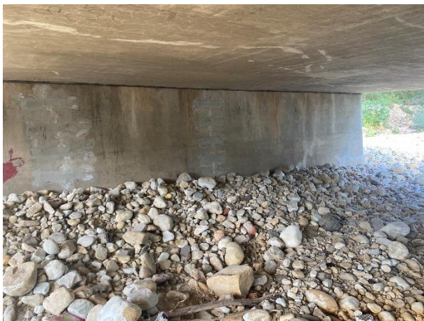
Removal of debris from the waterway.
