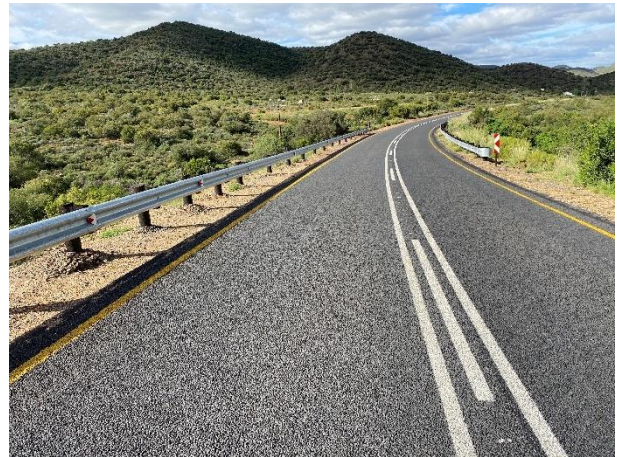
Condition of the newly installed guardrails and road surface.
