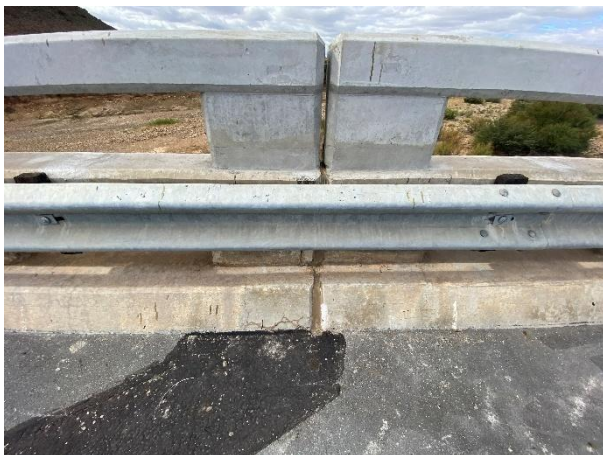
Replaced expansion movement joints at the piers and abutments with Thorma joints.
