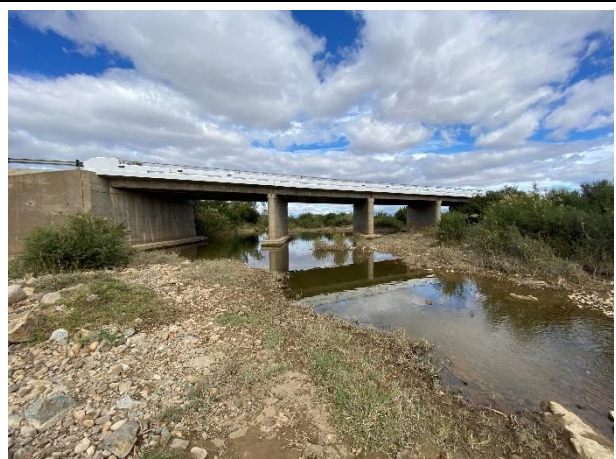
Condition of Bridge 4837.
