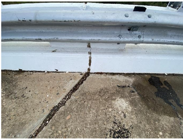
Concrete spalling repaired with an epoxy repair mortar.
