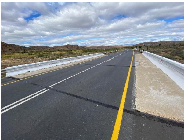
Replaced expansion movement joints.
