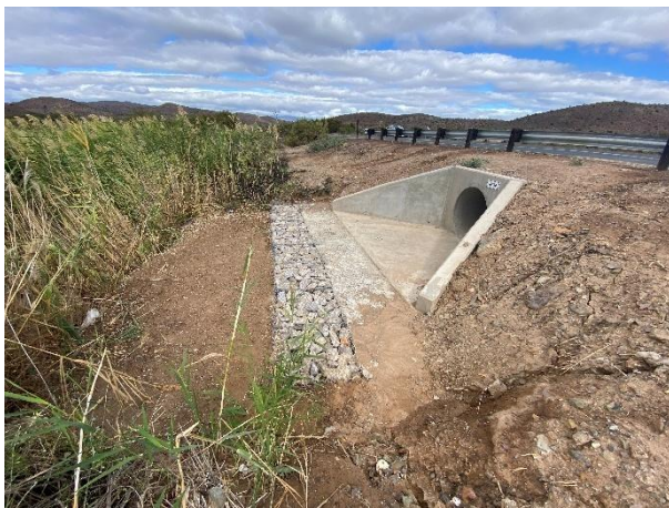
New gabion mattresses installed at the outlet.
