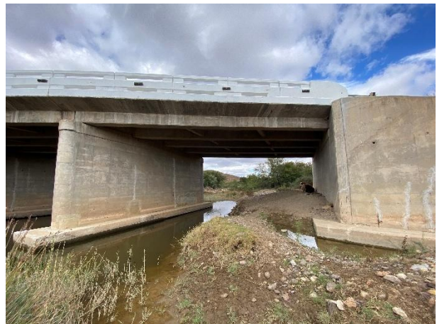
Repairs of vertical and horizontal cracks.
