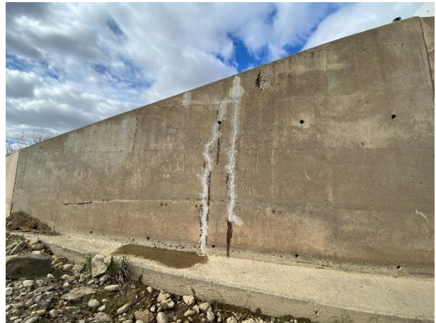
Repairs of vertical and horizontal cracks.
