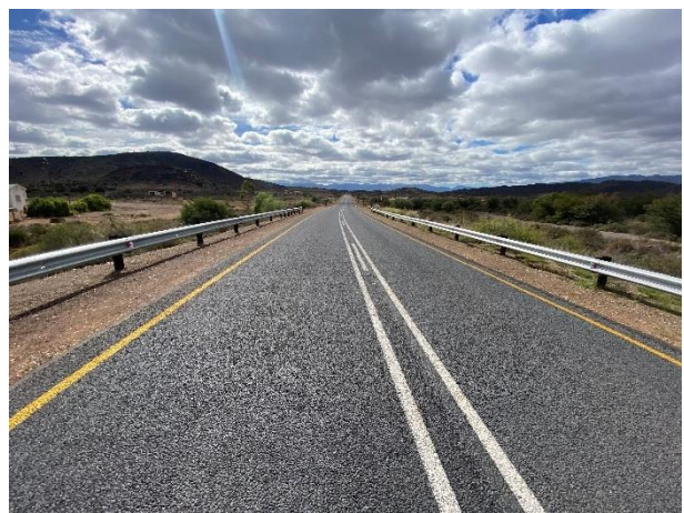
Condition of the newly installed guardrails and road surface at Culvert 10867.
