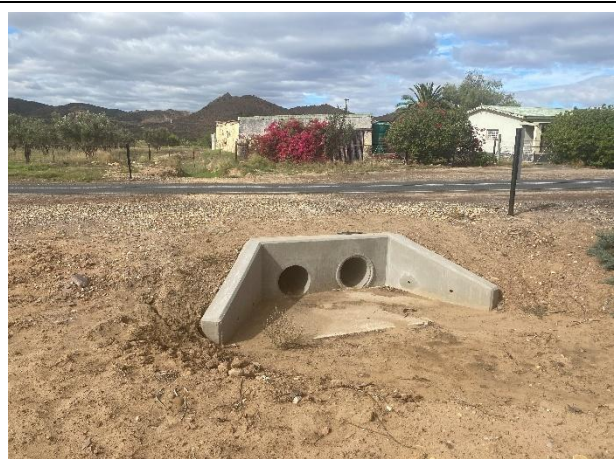
Small stormwater system adjacent to bridge 4837.
