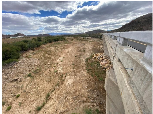
Condition of the vegetation surrounding the bridge.
