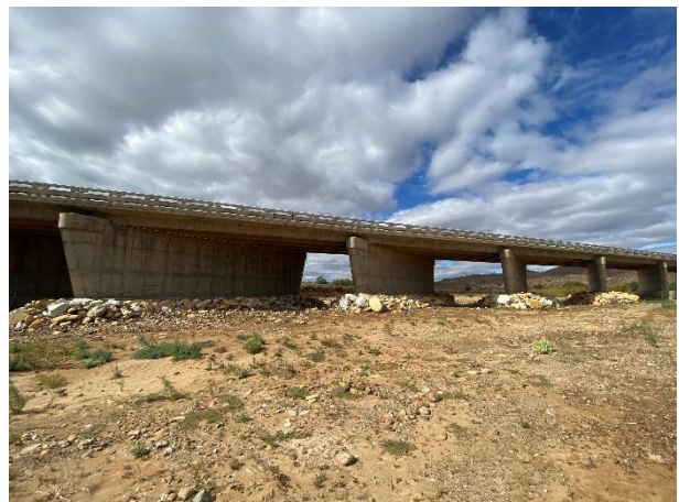
Condition of Bridge 5007.
