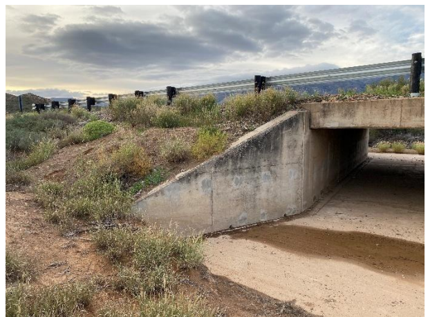
Repairs of vertical and horizontal cracks.
