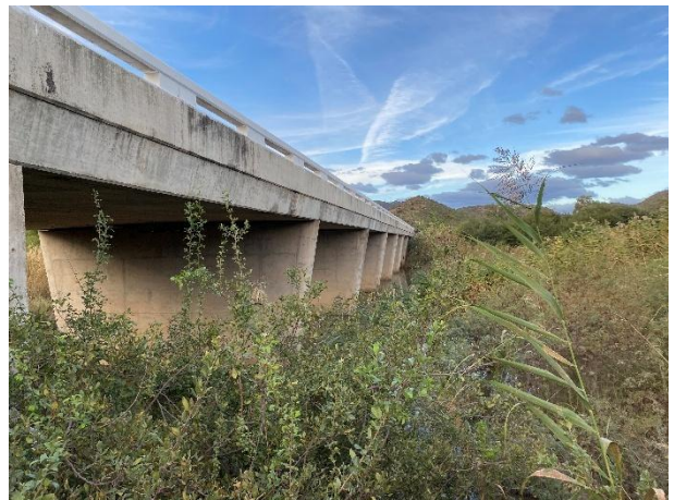
Condition of the vegetation surrounding the bridge.
