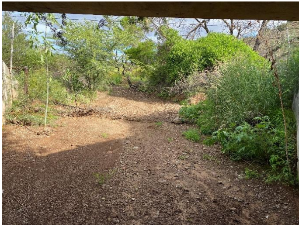
Clearance of dense vegetation and removal of the debris from the waterway. Fencing is in place.
