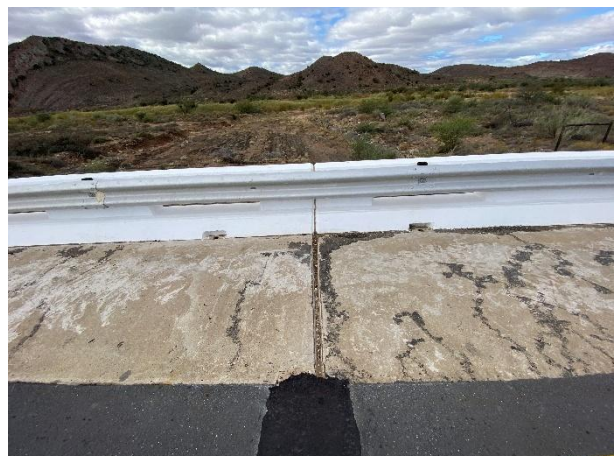
Replaced expansion movement joints
