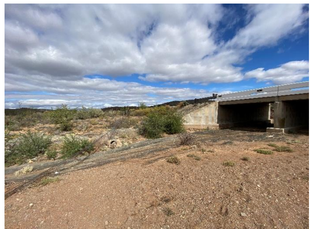
Condition of the vegetation surrounding the bridge.
