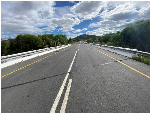
Replaced expansion movement joints.
