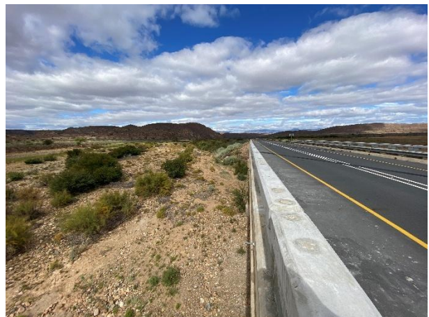
Condition of the vegetation surrounding the bridge.
