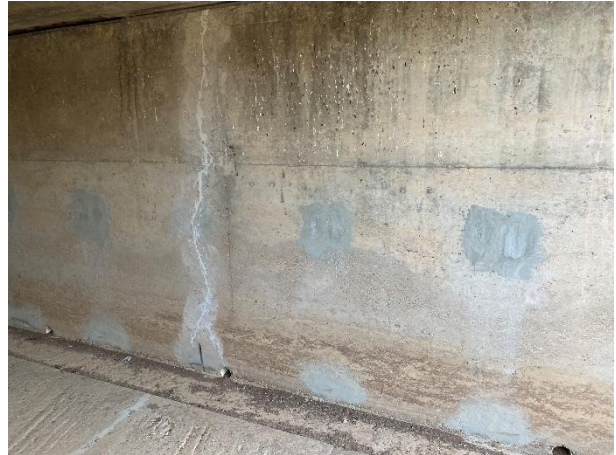
Repairs of vertical and horizontal cracks.
