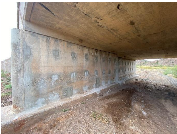
Repairing of cracks on the wingwalls and headwalls.
