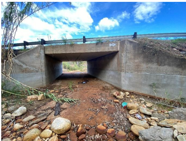
Removal of vegetation overgrowth and silt deposits.
