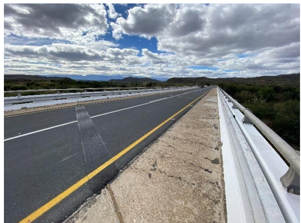
Replaced expansion movement joints.
