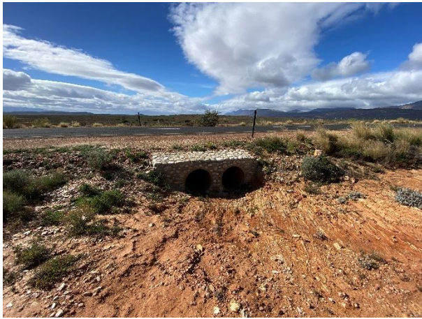
Culvert off TR 83/1 as km 29.
