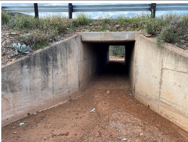
Removal of vegetation overgrowth and silt deposits.
