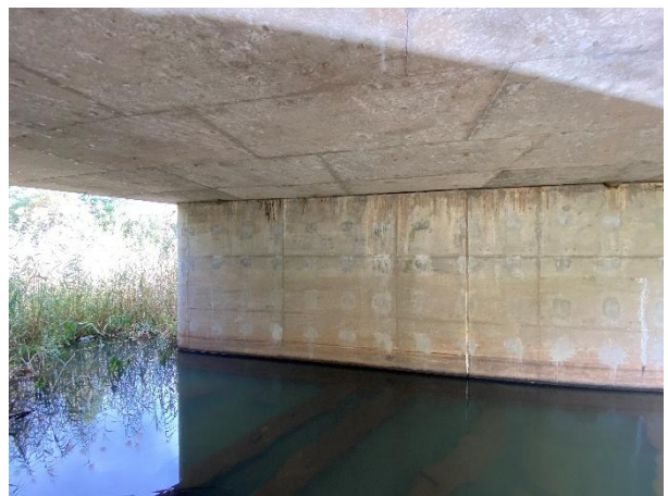
Repairing of cracks.
