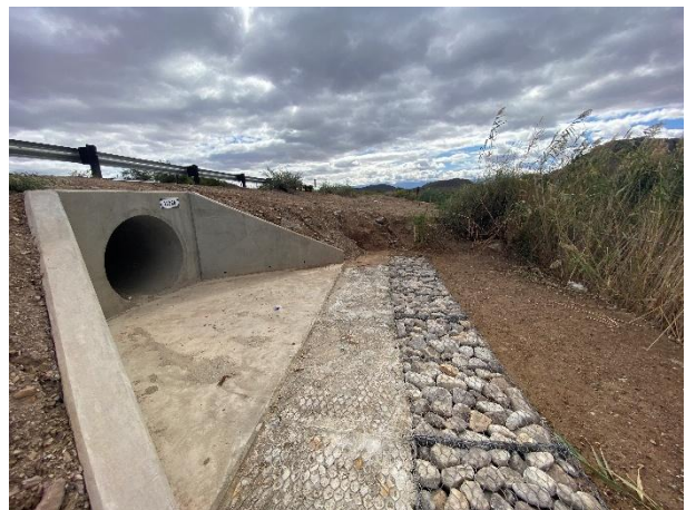
New prefabricated concrete pipe within the existing culvert.
