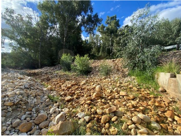
Condition of the vegetation surrounding the culvert.
