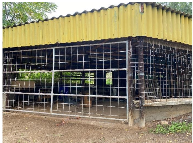
Previous site camp storage facility.
