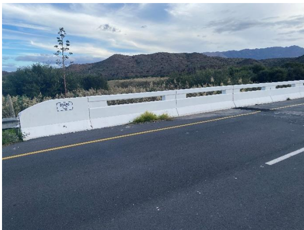
Replaced expansion movement joints.
