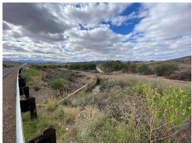
Condition of the vegetation surrounding the culvert.
