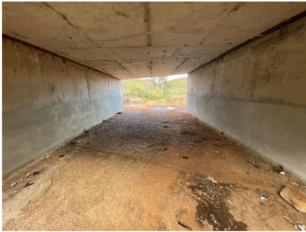
Removal of vegetation overgrowth and silt deposits.
