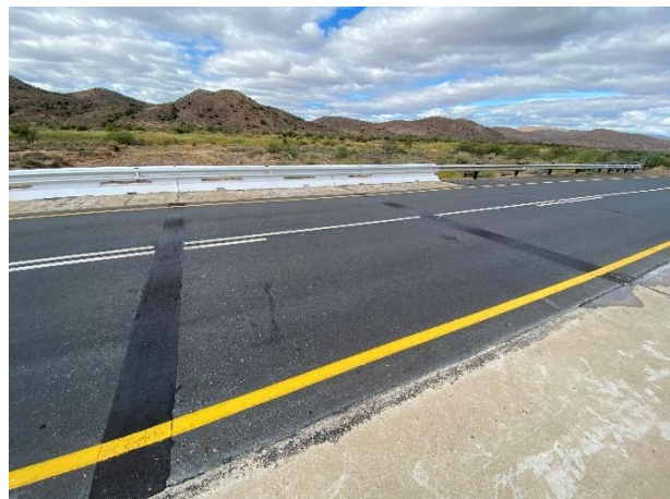
Replaced expansion movement joints
