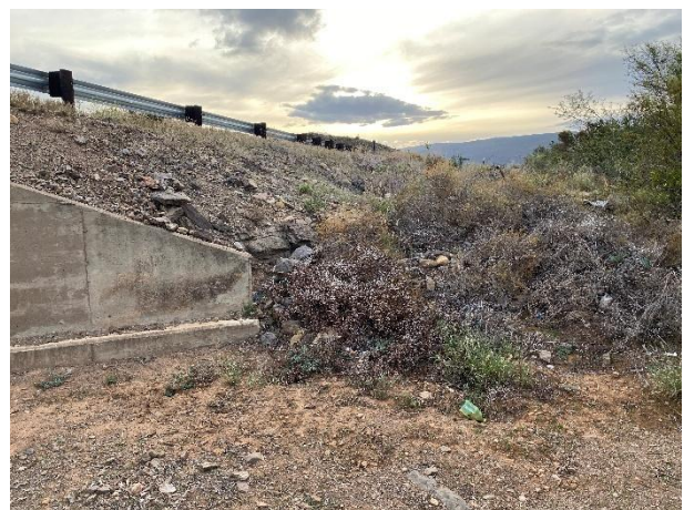
Backfill of the eastern and western cell.
