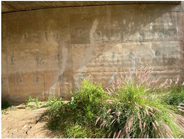
Repairs of vertical and horizontal cracks.
