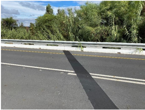
Replaced expansion movement joints.
