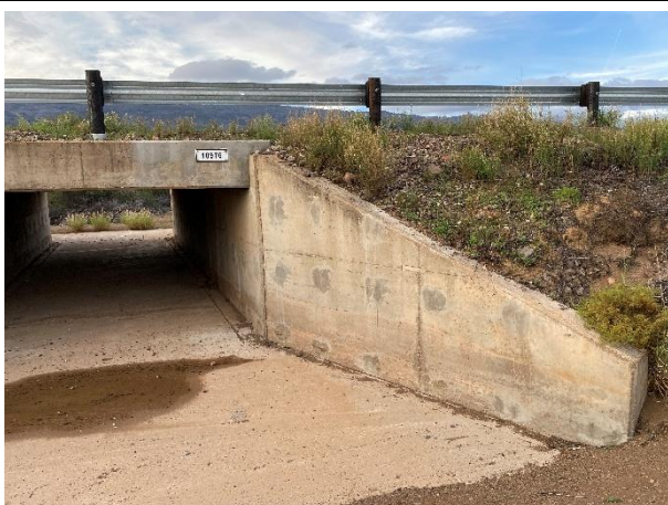
Repairs of vertical and horizontal cracks.
