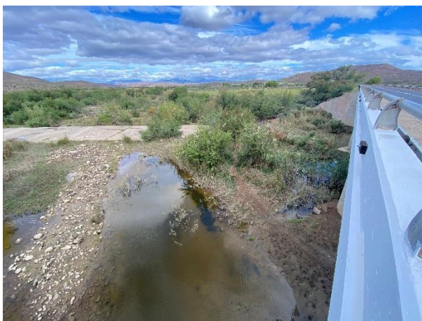
Removal of dense vegetation overgrowth and debris deposits.
