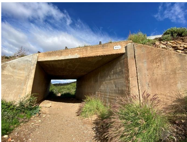
Condition of bridge 9061.
