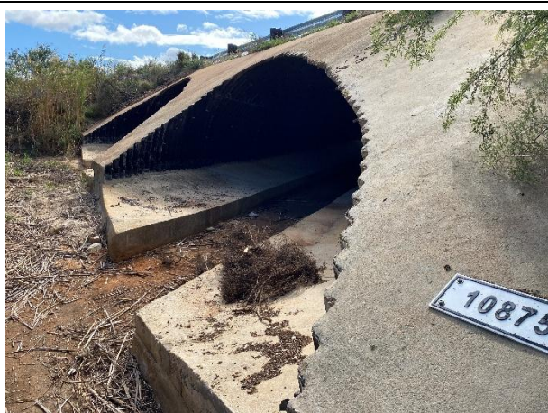
Trimming and removal of dense vegetation at the inlet and outlet and removal of silt deposits inside the barrel.
