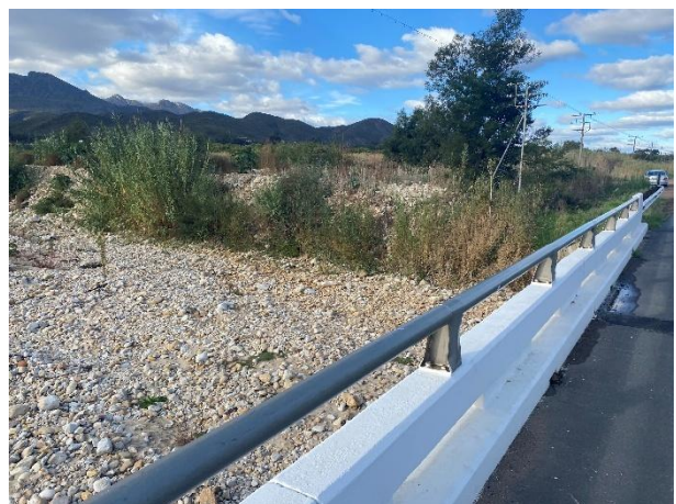
Condition of the vegetation surrounding the culvert.
