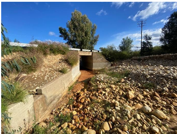
Condition of Culvert 10971.
