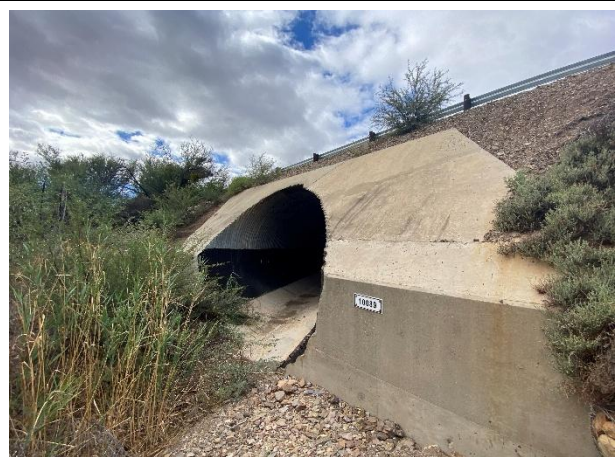
Clearance of dense vegetation and debris from the culvert.
