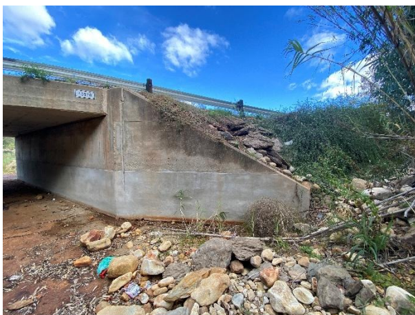
Repaired vertical and horizontal cracks in the abutment, piers, and wingwalls.
