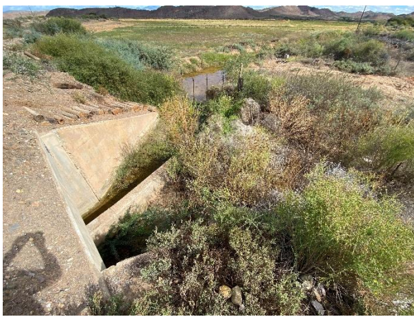
Condition of the vegetation surrounding the culvert. Fencing in place.
