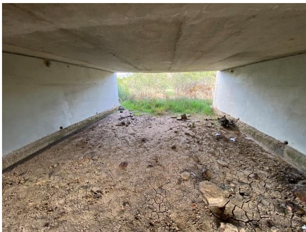
Removal of vegetation overgrowth and silt deposits.
