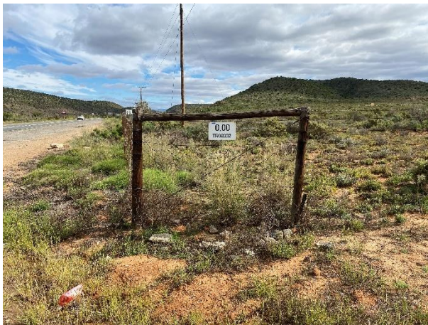
Condition of the road reserve at TR 83/2.
