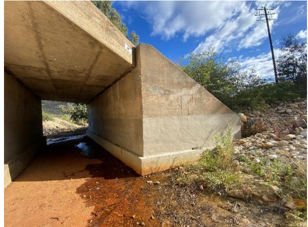
Removal of debris from the waterway.
