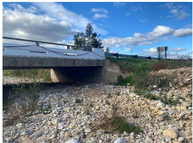
Condition of bridge 4515.
