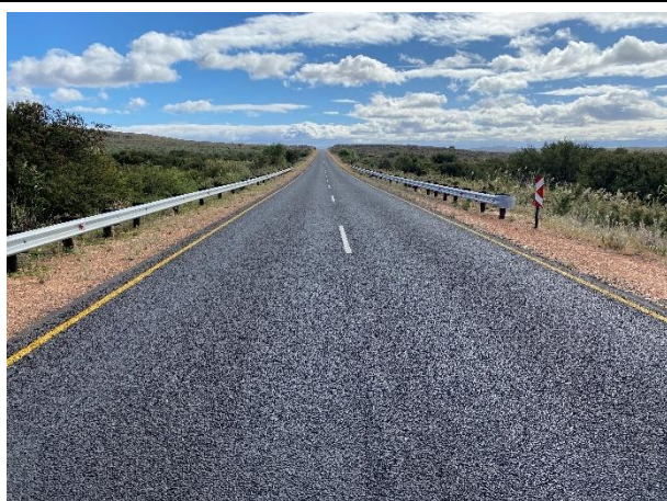
Newly surfaced and installed guardrails at culvert 10875 off TR 83/1.
