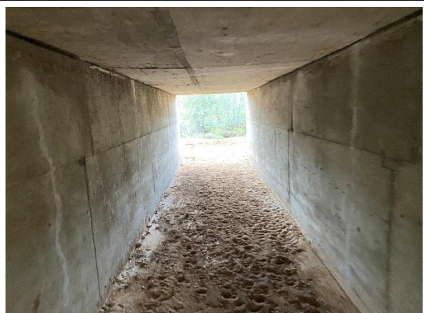
Removal of vegetation overgrowth and silt deposits.
