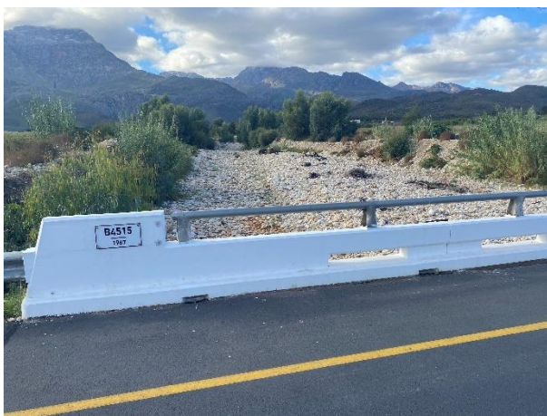
Condition of bridge 4515.
