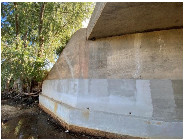
Repaired vertical and horizontal cracks along with concrete spalling in the abutment, piers, and wingwalls.
