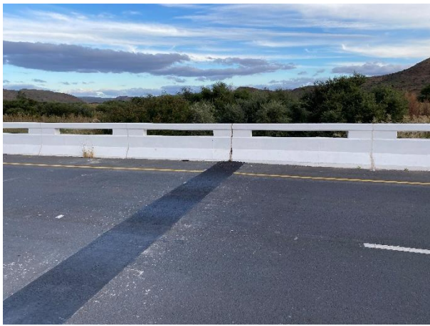
Replaced expansion movement joints.
