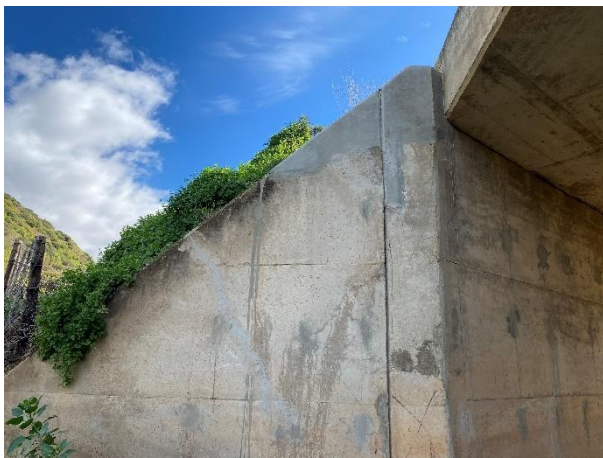
Concrete spalling repaired with an epoxy repair mortar.
