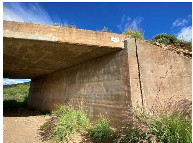
Repairs of vertical and horizontal cracks.
