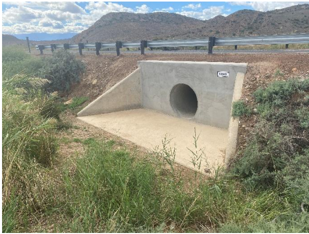
The construction of a new headwall, apron slab and wingwalls at the outlet.
