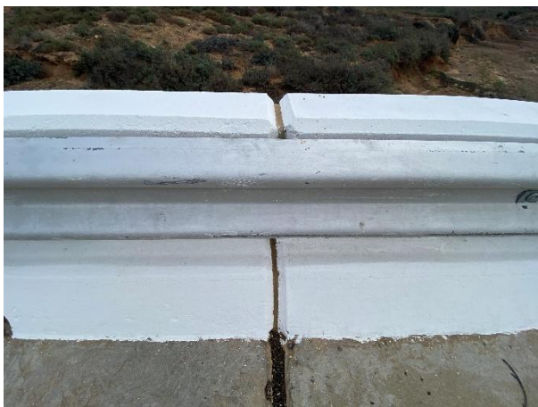
Replaced expansion movement joints
