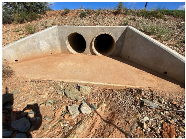
Culvert off TR 83/1 as km 29.
