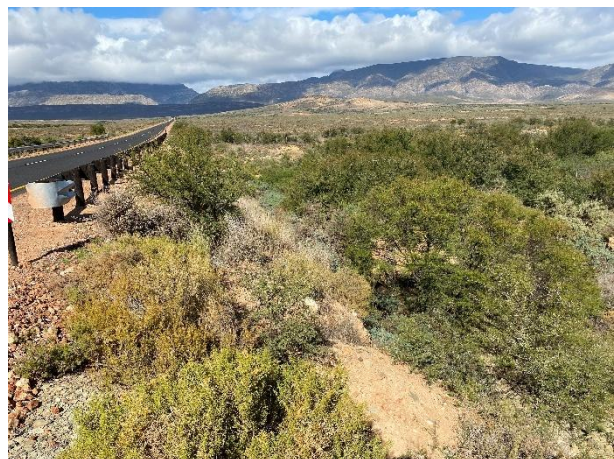
Condition of the vegetation along Culvert 10874.
