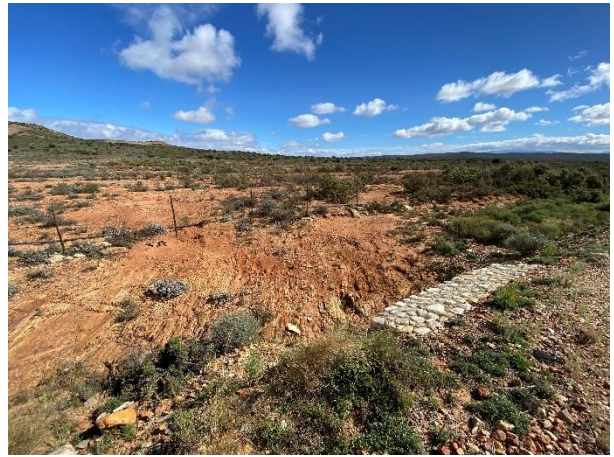
Removal and trimming of dense vegetation at the inlet and outlet.
