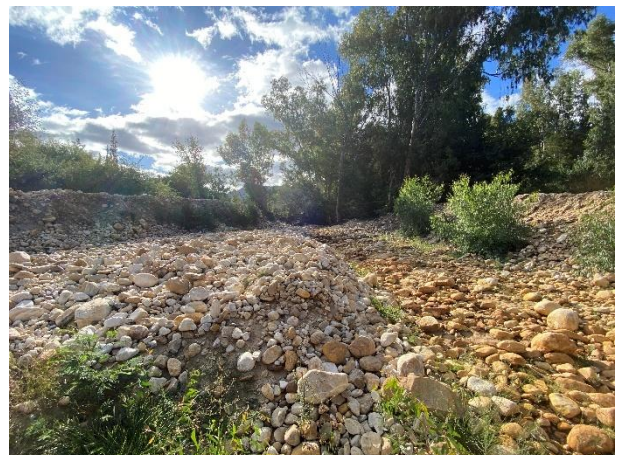
Condition of the vegetation surrounding the culvert.
