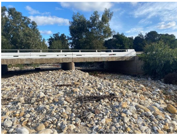
Condition of the vegetation surrounding the culvert.
