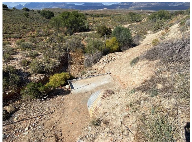
Condition of the vegetation surrounding Culvert 10692 at km 30.63
