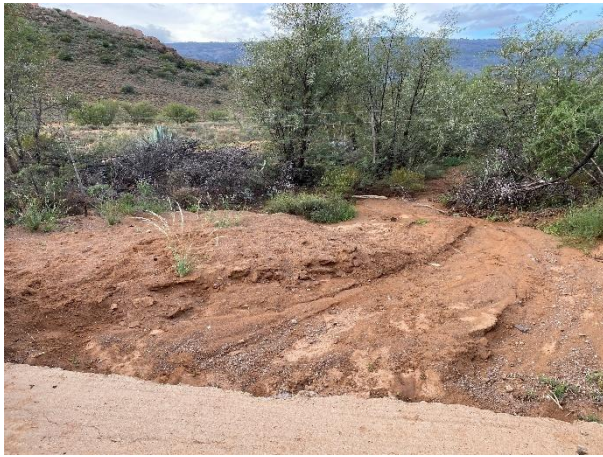
Removal of vegetation overgrowth and silt deposits.
