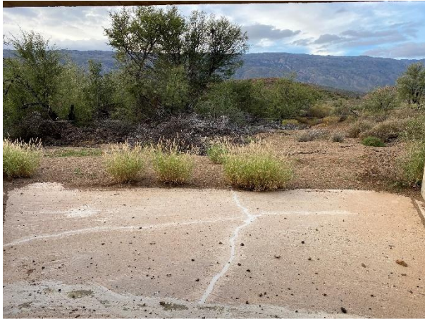
Removal of vegetation overgrowth and silt deposits.
