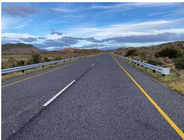
Condition of the newly installed guardrails and road surface at culvert 10976.
