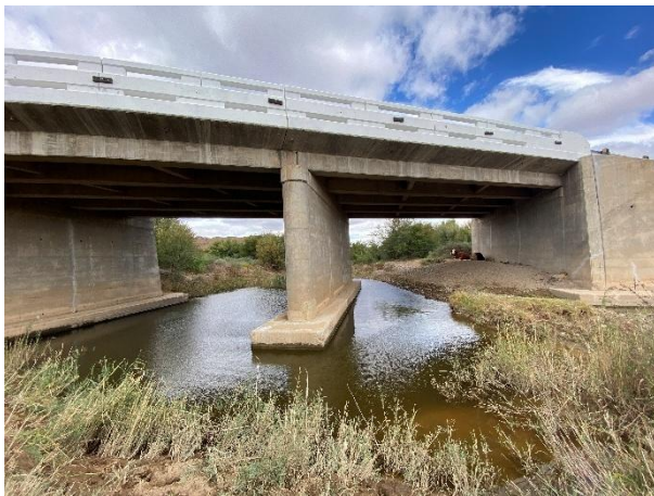
Removal of dense vegetation overgrowth and debris deposits underneath bridge 4838.
