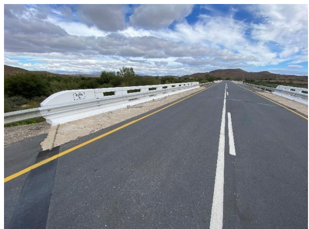
Replaced expansion movement joints.
