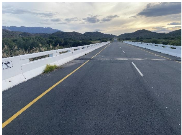
Replaced expansion movement joints.
