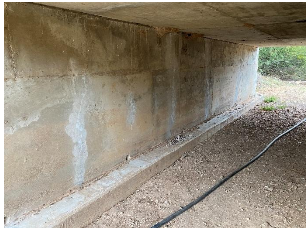
Repairs of vertical and horizontal cracks.
