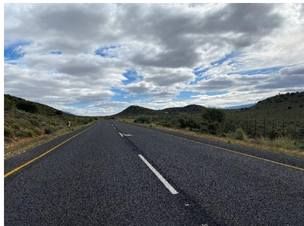
Condition of the road reserve at TR 83/2.
