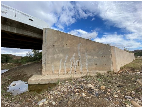
Repairs of vertical and horizontal cracks.
