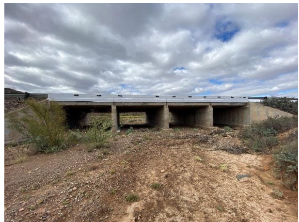
Removal of vegetation overgrowth and silt deposits surrounding Bridge 5090.
