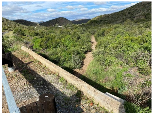
Condition of the vegetation surrounding the bridge.
