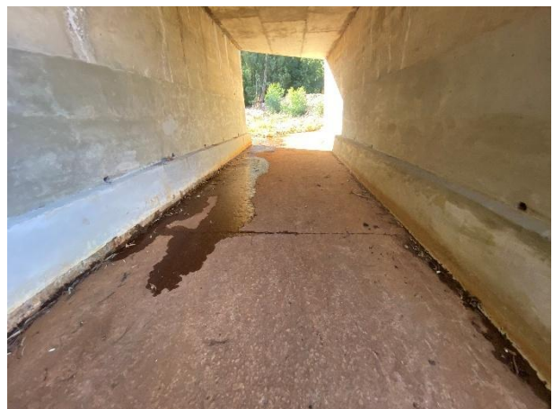
Removal of debris from the waterway.
