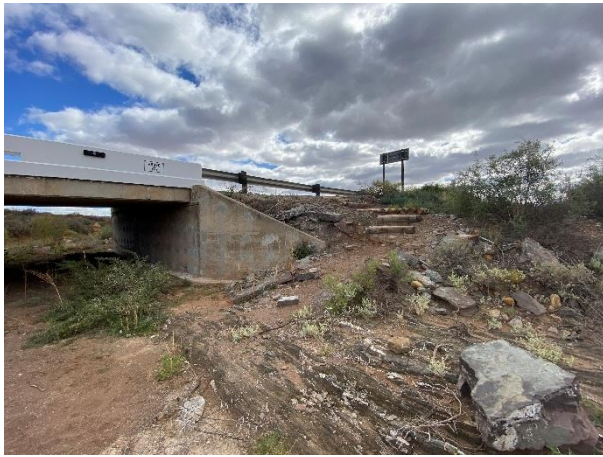
Condition of the vegetation surrounding the bridge. Some fencing is seen on the ground which has been replaced.
