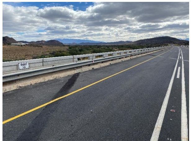
Replaced expansion movement joints.
