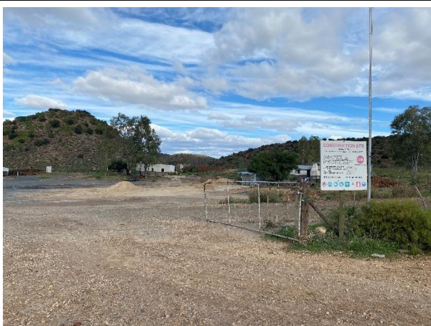
Entrance of the construction camp.
