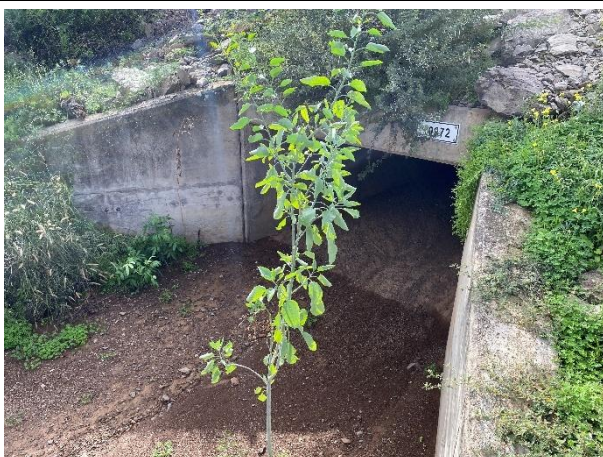
Clearance of dense vegetation and removal of the debris from the waterway.
