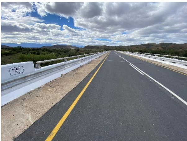
Condition of the newly installed guardrails and road surface at bridge 4837.
