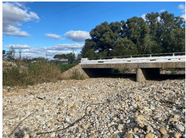
Condition of the vegetation surrounding the culvert.
