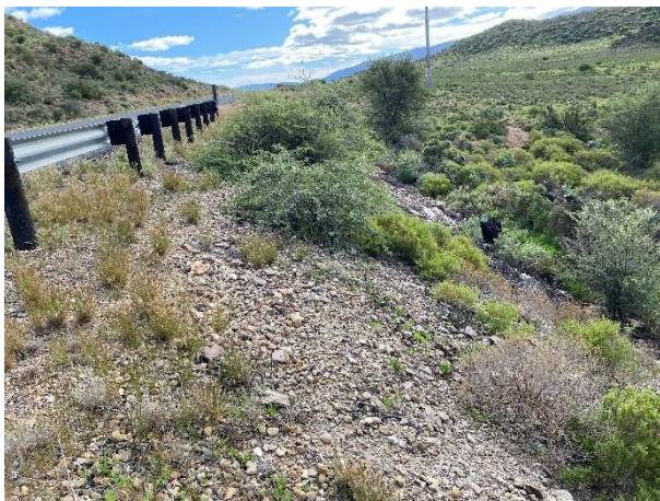
Regraded banks of the bridge.
