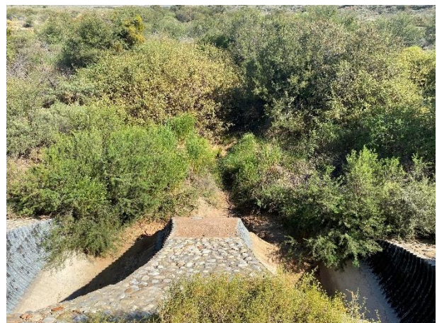
Condition of the vegetation along Culvert 10874.
