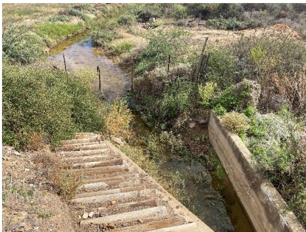
Timber-reinforced embankment slope.
