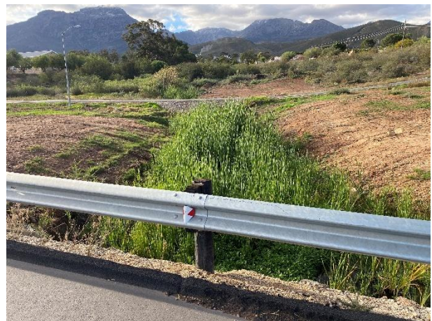
Overgrown vegetation due to the recent rainfall.
