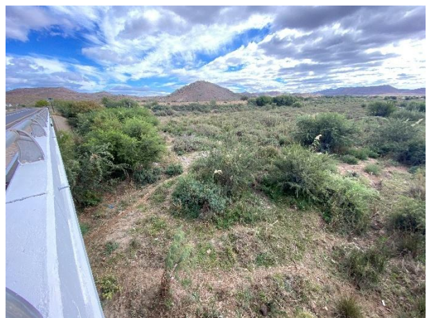
Condition of the vegetation surrounding the bridge.
