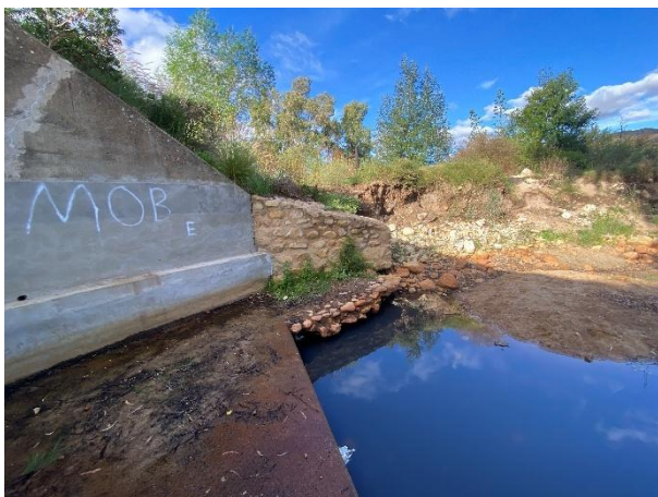
Condition of the vegetation surrounding the culvert.
