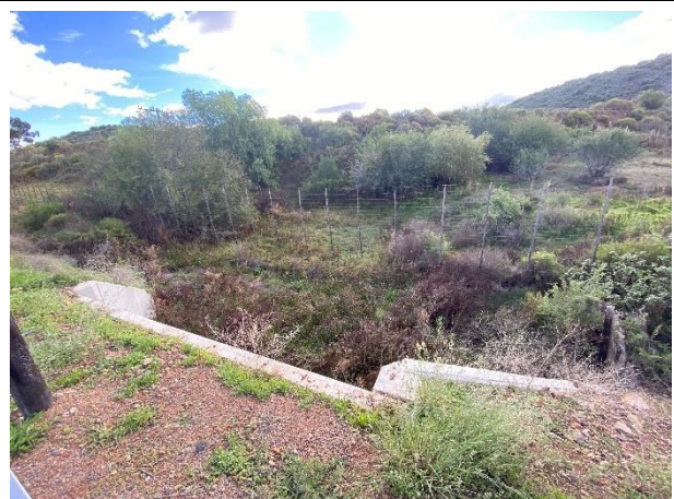
Condition of the vegetation surrounding the culvert.
