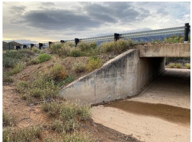
Repairs of vertical and horizontal cracks.
