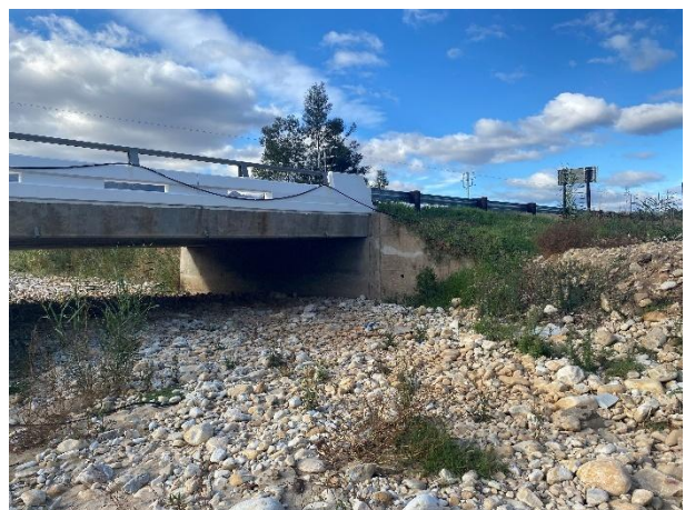
Condition of bridge 4515.
