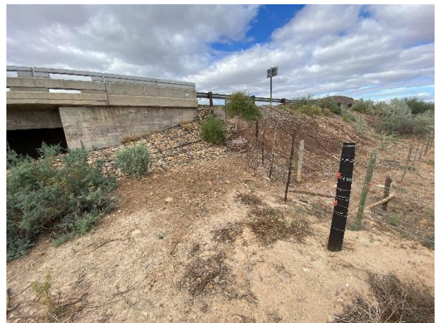
Condition of the vegetation surrounding the bridge. Fencing in place.
