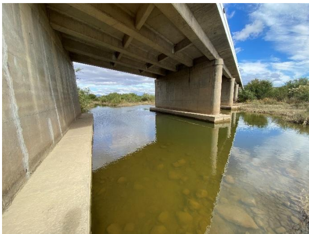
Repairs of vertical and horizontal cracks
