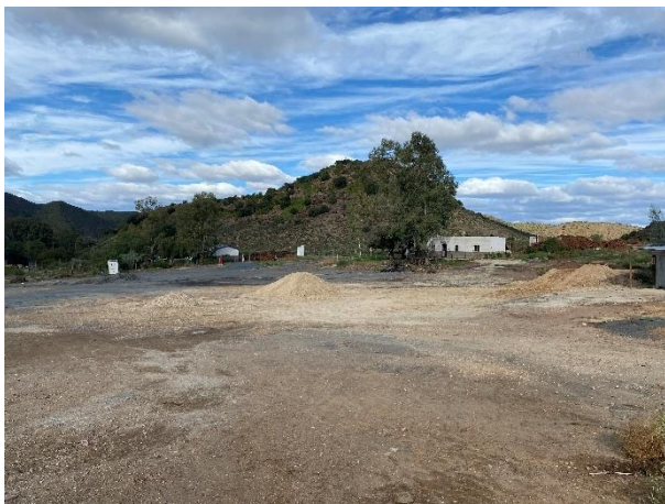
Remaining material stockpiles at the construction camp.
