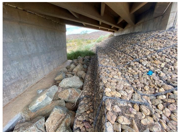
Installation of gabion baskets along the waterway and embankments to prevent further scouring and erosion.
