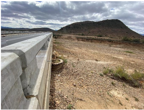
Condition of the vegetation surrounding the bridge.
