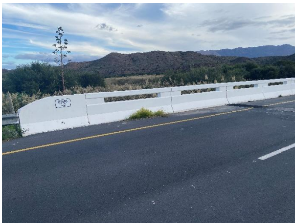
Replaced expansion movement joints.
