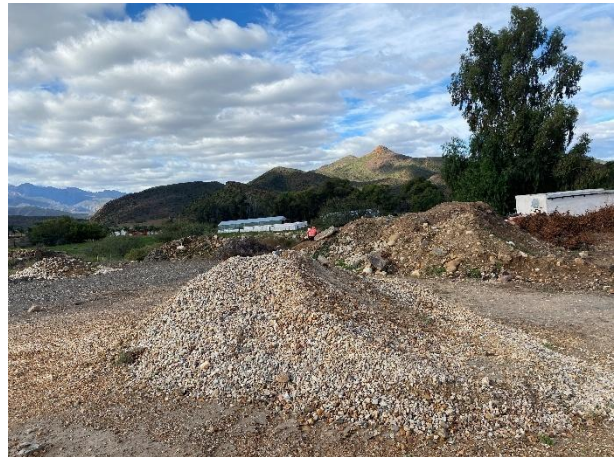
Remaining material stockpiles at the construction camp.
