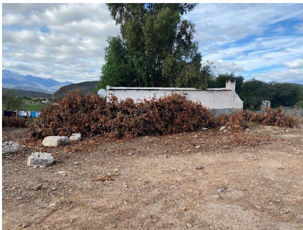
Vegetation debris located at the construction camp.
