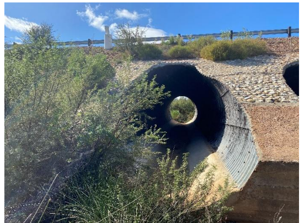
Condition of the vegetation along Culvert 10874.
