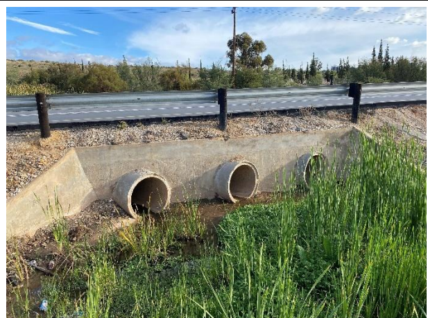
Repaired culvert.
