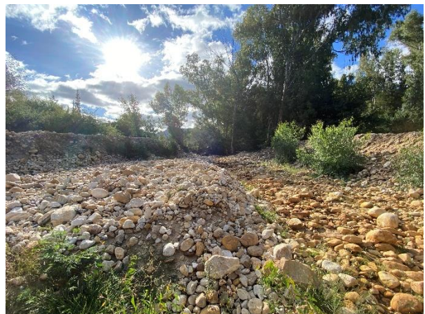
Condition of the vegetation surrounding the culvert.
