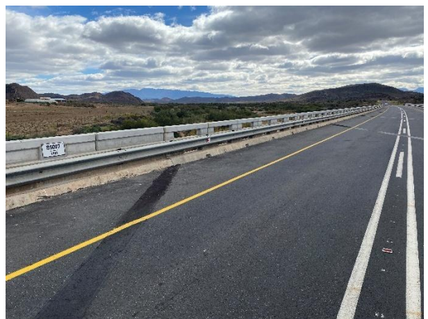
Replaced expansion movement joints.
