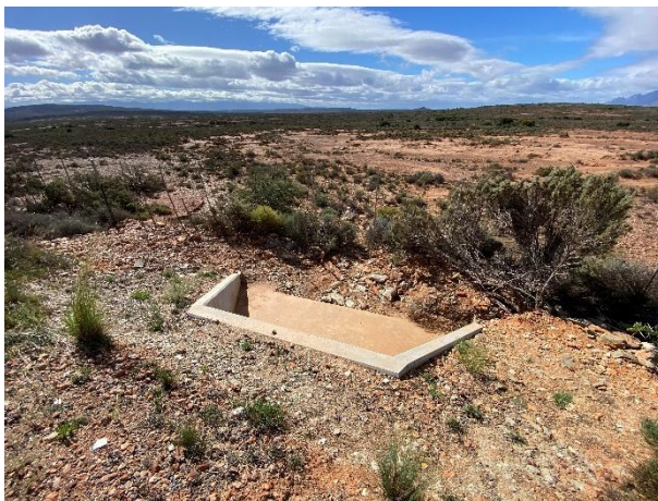
Culvert off TR 83/1 as km 29.
