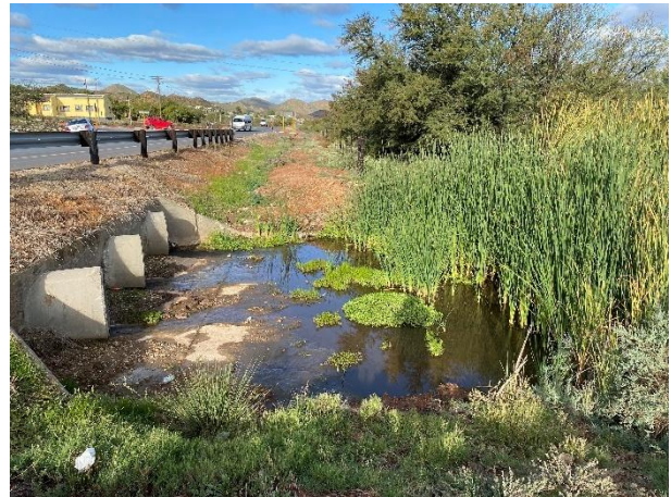
Removal of vegetation and debris from the waterway.
