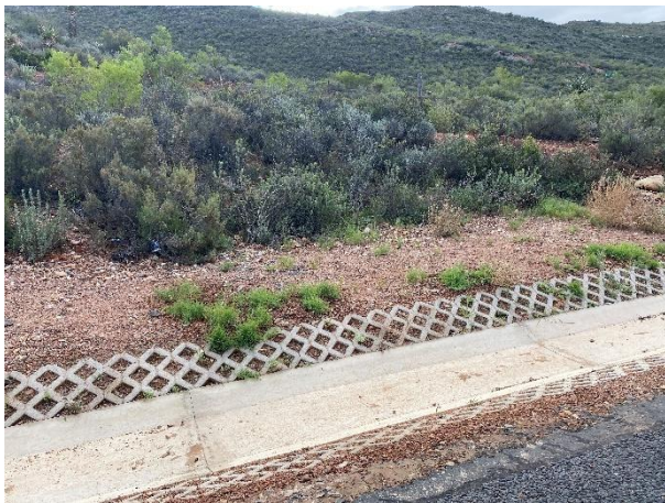
Upgraded side drains off MR 365.
