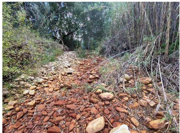
Removal of vegetation overgrowth and silt deposits.
