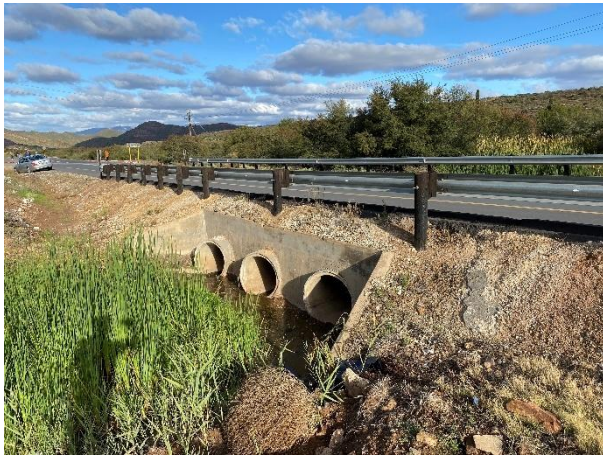
Repaired culvert.
