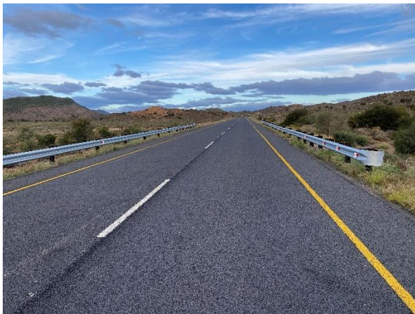
Condition of the newly installed guardrails and road surface at culvert 10976.
