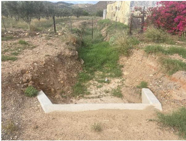
Inlet of the small stormwater system adjacent to bridge 4837.
