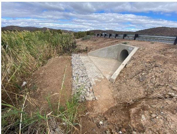
New gabion mattresses installed at the outlet.
