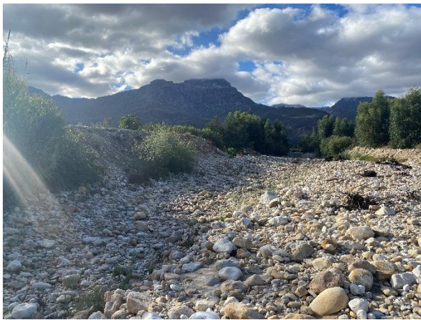
Condition of the vegetation surrounding the culvert.
