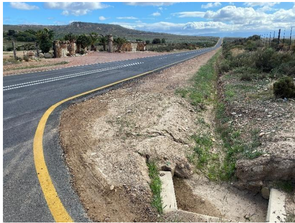
Condition of the road reserve at TR 83/1 km 25.78.
