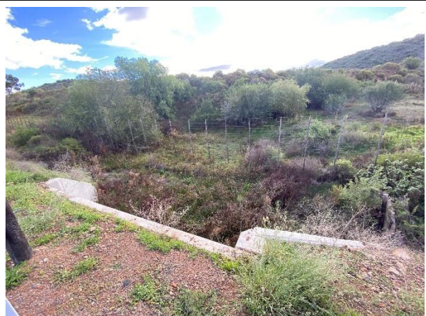
Condition of the vegetation surrounding the culvert.
