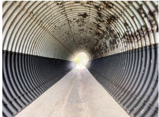
Clearance of the Armco barrel walls and the painting of affected corroded areas.
