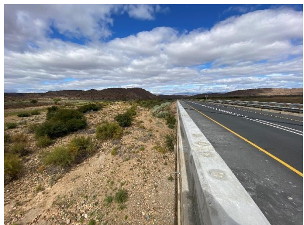
Condition of the vegetation surrounding the bridge.
