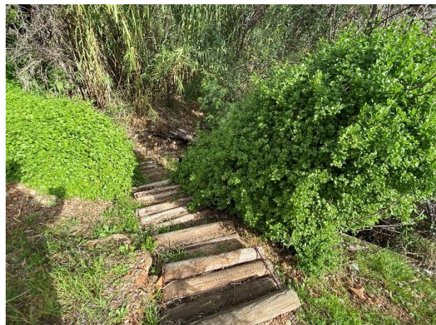
Timber-reinforced embankment slope.
