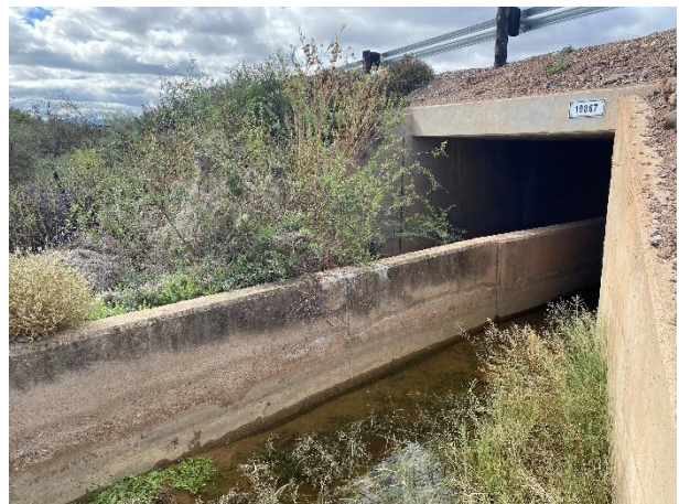
The existing deck at both the inlet and outlet demolished and reconstructed with a raised headwall.
