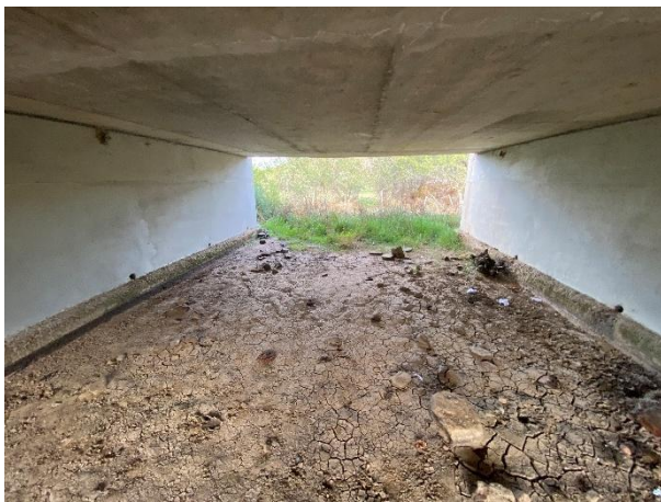
Removal of vegetation overgrowth and silt deposits.
