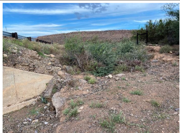
Backfill of the eastern and western cell.
