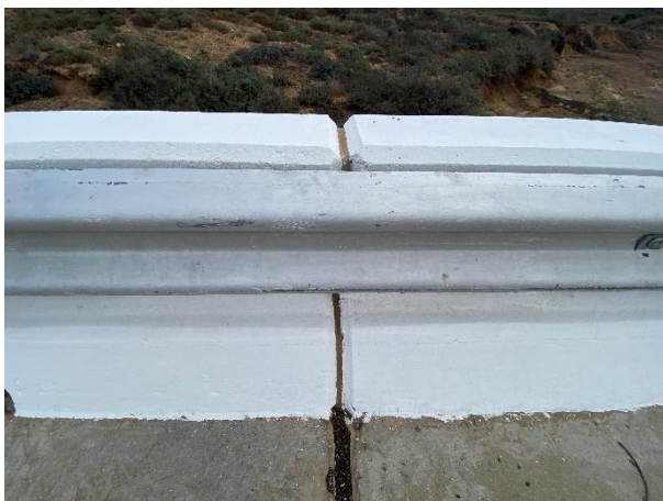
Replaced expansion movement joints
