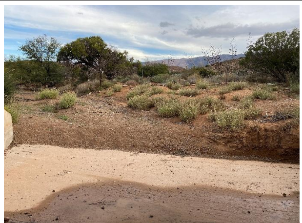
Removal of vegetation overgrowth and silt deposits.
