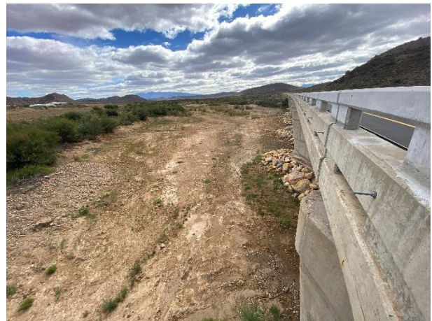
Condition of the vegetation surrounding the bridge.
