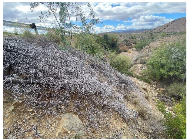
Condition of the vegetation surrounding the culvert.
