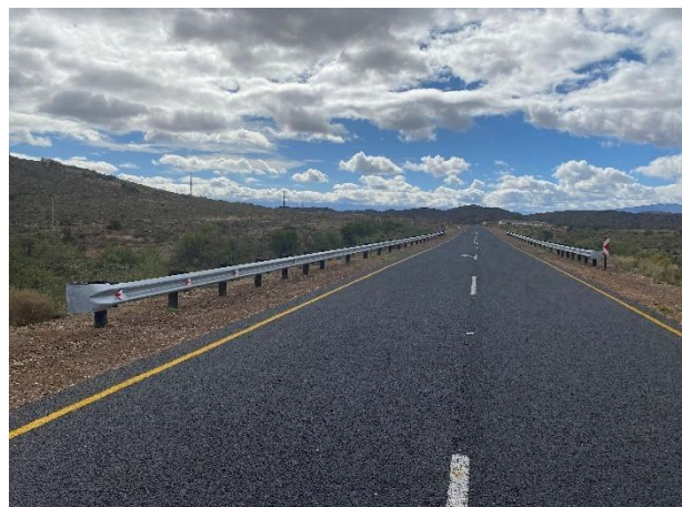
Condition of the newly installed guardrails and road surface at Culvert 10089.
