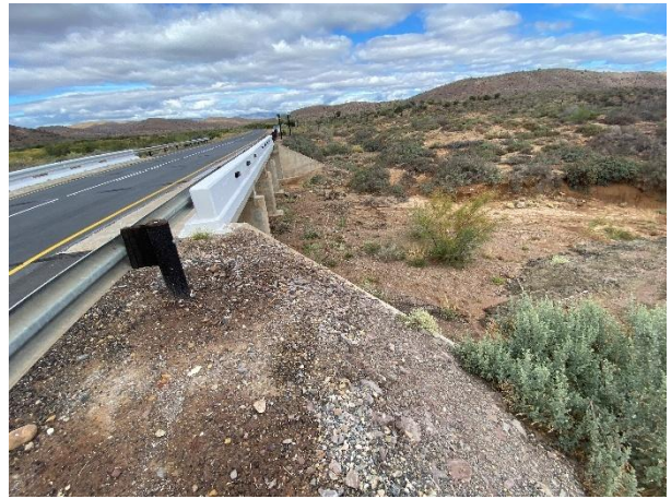
Condition of Bridge 5090.
