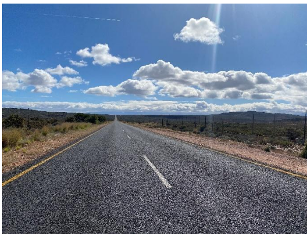
Condition of the newly surfaced road and road reserve at TR 83/1 km 29.
