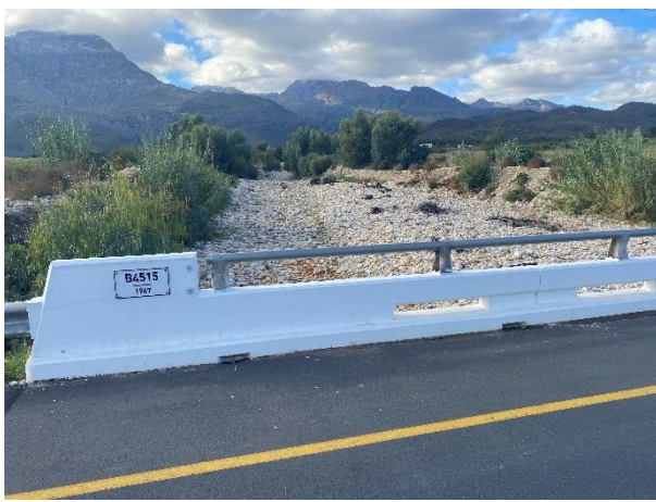
Condition of bridge 4515.
