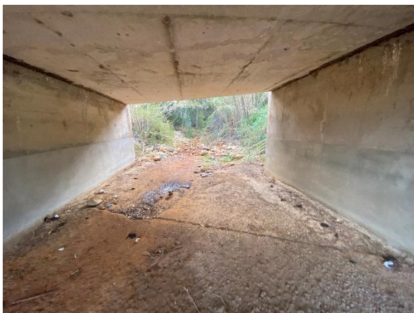
Removal of vegetation overgrowth and silt deposits.
