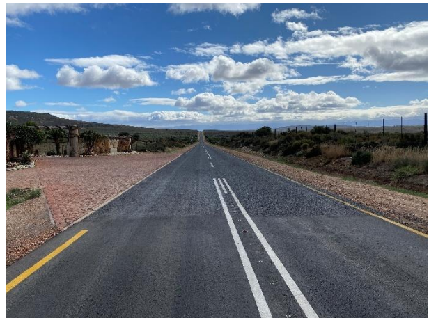
Condition of the newly surfaced road and road reserve at TR 83/1 km 25.78.
