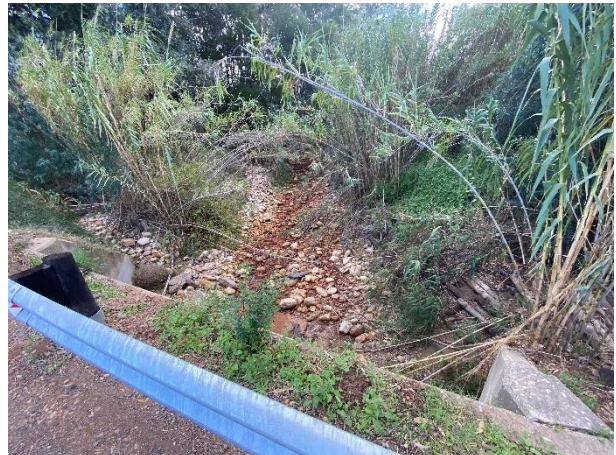
Condition of the vegetation surrounding the culvert.
