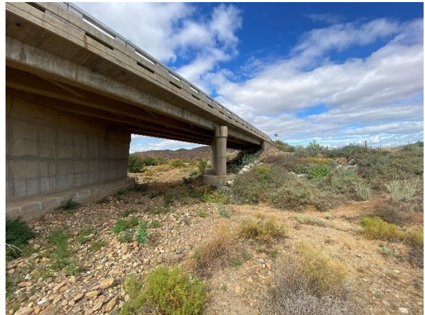
Removal of vegetation overgrowth and debris deposits on the foundations
