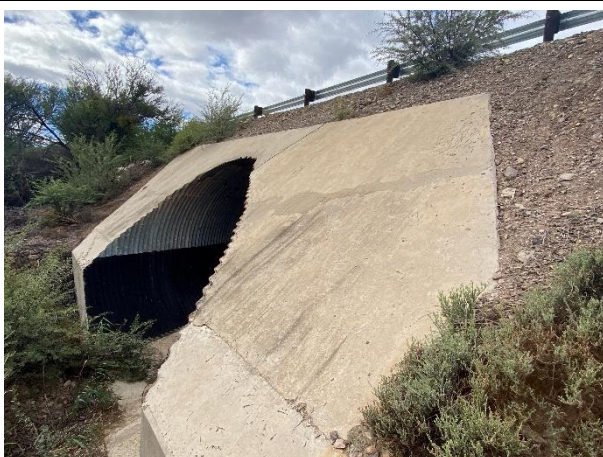
Sloping headwall sealed by injection, and cracks cut back and repaired using a cementitious repair compound.
