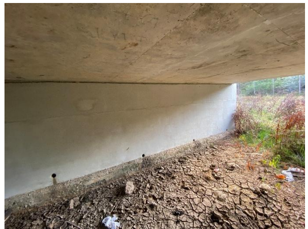
Concrete spalling and cracks repaired with an epoxy repair mortar.
