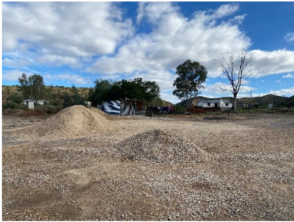
Remaining material stockpiles at the construction camp.
