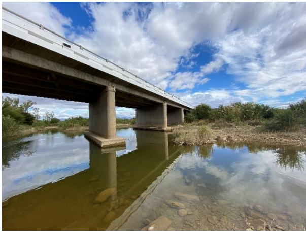
Condition of Bridge 4837.
