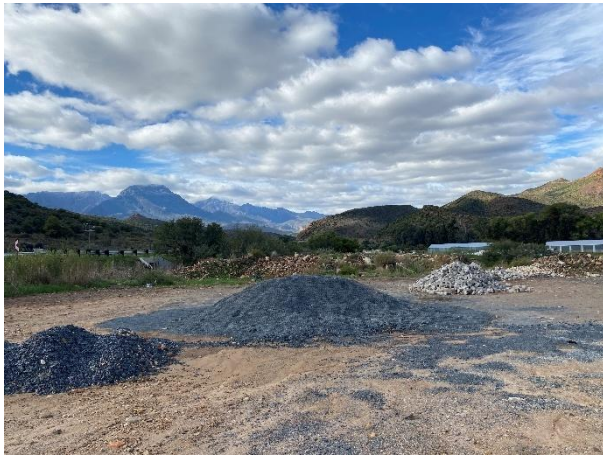
Condition of the construction camp with remained material stockpiles.
