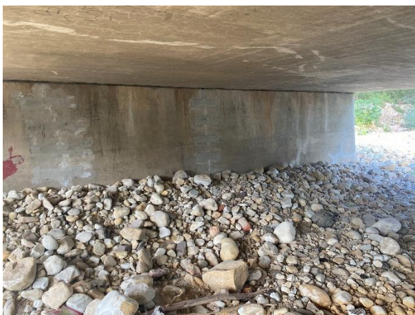
Removal of debris from the waterway.
