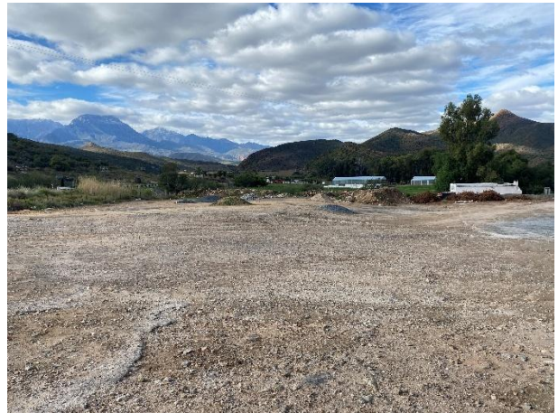
Remaining material stockpiles at the construction camp.
