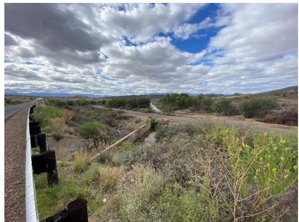
Condition of the vegetation surrounding the culvert.
