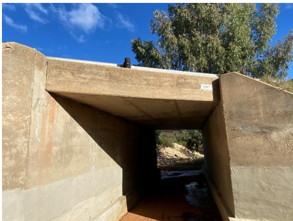
Replacement of the missing culvert number.
