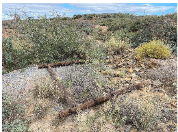
Condition of the vegetation surrounding the bridge. Fencing seemed to have been dismantled.
