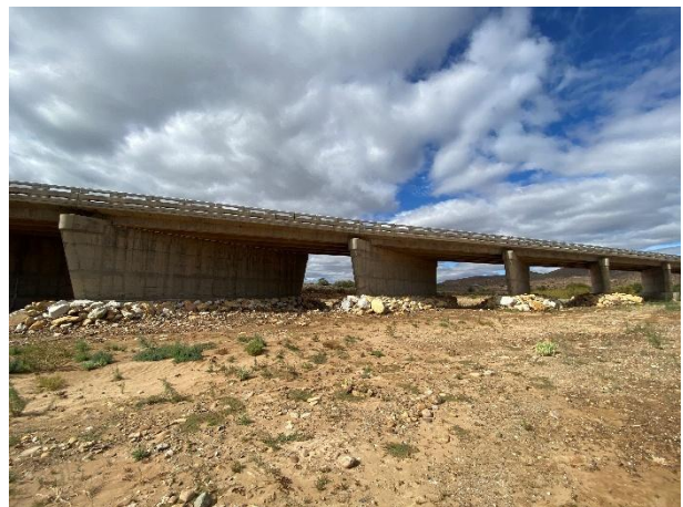
Condition of Bridge 5007.
