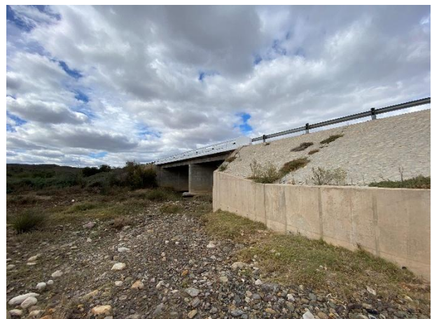
Backfilling and dump rock riprap around the piers and abutments.
