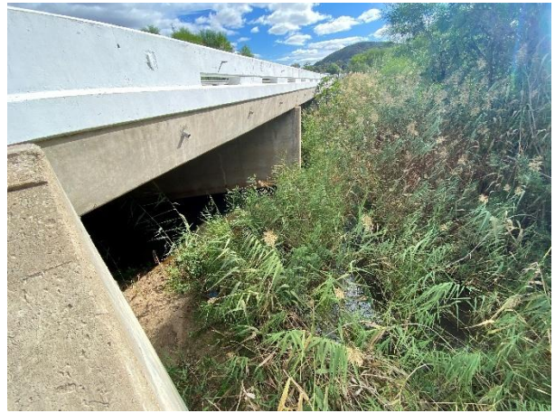
Condition of the vegetation surrounding the bridge.
