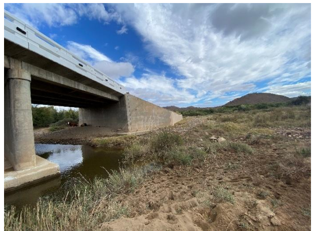
Condition of the vegetation surrounding the bridge.
