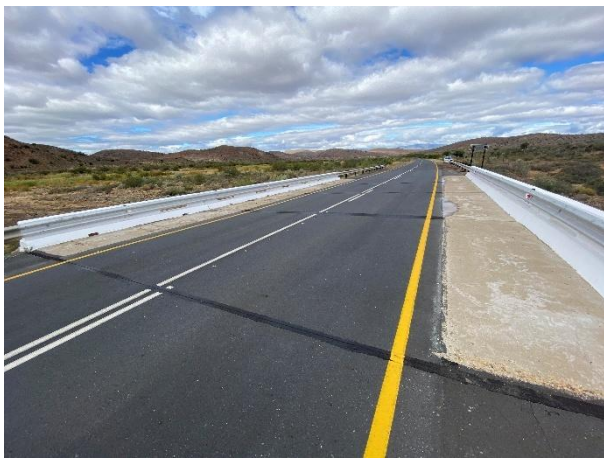
Replaced expansion movement joints.
