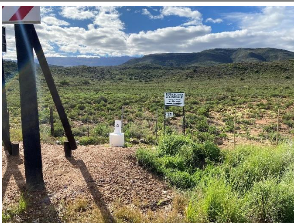
Condition of the road reserve at MR 365.
