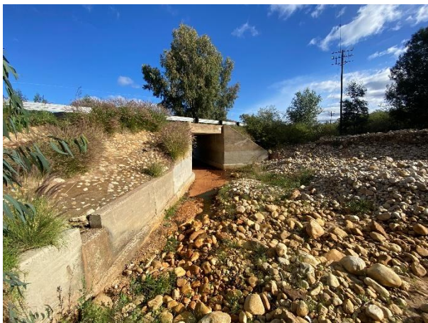
Condition of Culvert 10971.
