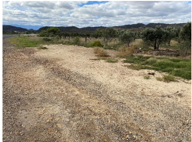
Condition of the vegetation surrounding the small culvert.
