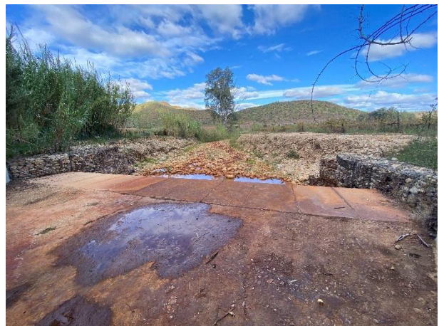
Removal of vegetation at wingwalls and the installation of gabion boxes.
