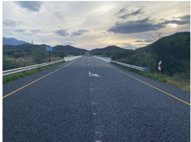
Condition of the newly installed guardrails and road surface at bridge 5490.
