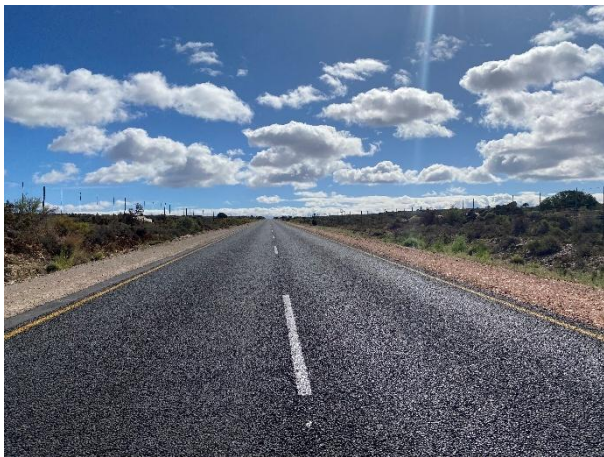
Condition of the newly surfaced road and road reserve at TR 83/1 km 30.
