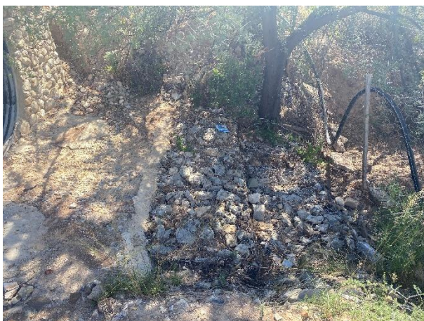
Gabion steps extending downward from the culvert to stabilise the slope and manage water flow.
