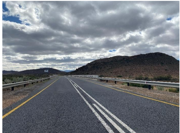
Condition of the newly installed guardrails and road surface at Bridge 5007.
