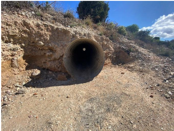
Clearance of accumulation of debris and silt deposits within the barrel.
