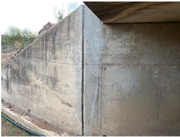
Cracks repaired with a cementitious repair compound.
