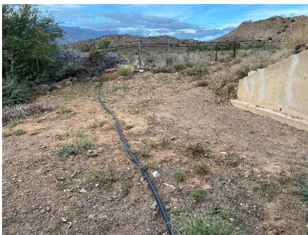
Condition of the vegetation surrounding the culvert.
