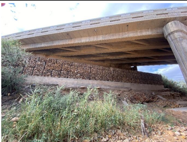
Installation of gabion baskets along the waterway and embankments to prevent further scouring and erosion.
