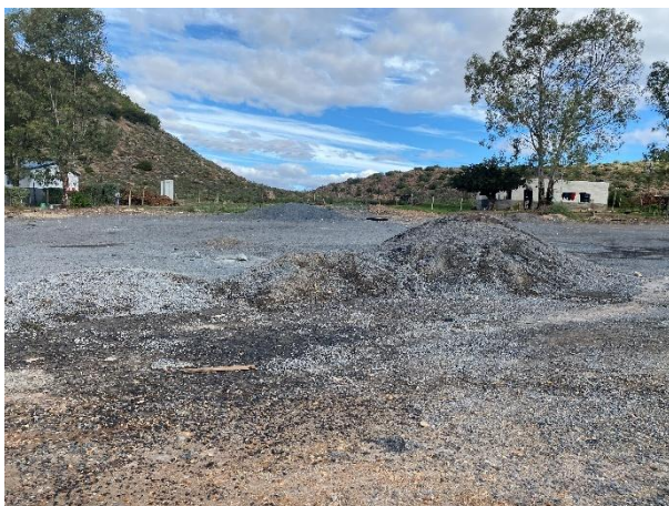
Remaining material stockpiles at the construction camp.
