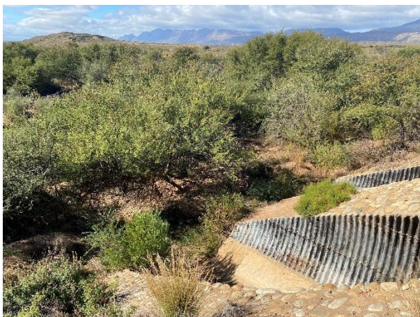
Condition of the vegetation along Culvert 10874.
