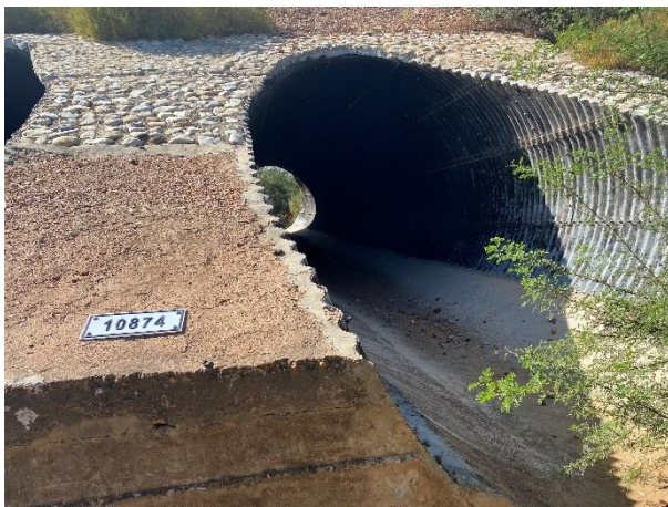
Removal of silt deposits inside the barrel and carting thereof to spoil.
