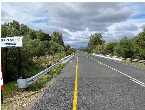
Condition of the newly installed guardrails and road surface at bridge 5359.
