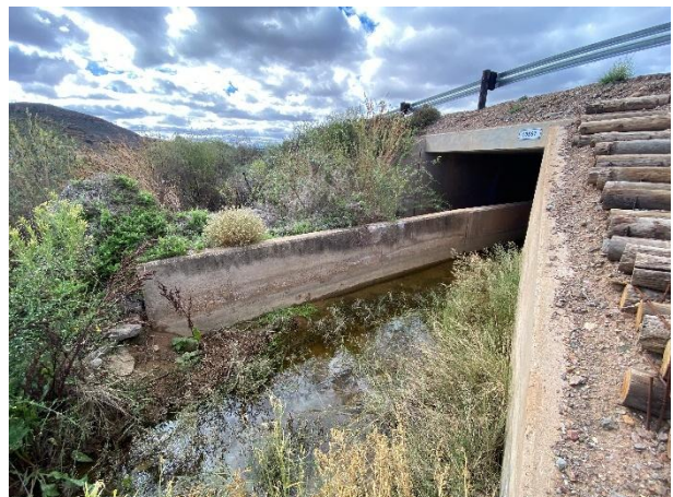
Concrete culvert outlet with vegetated channel and timber-reinforced embankment slope.
