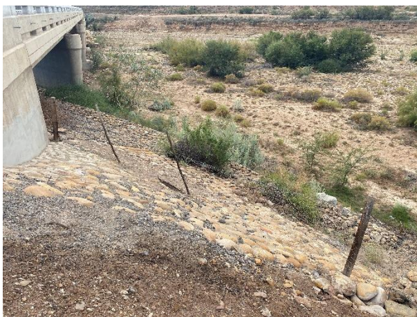
Condition of the vegetation surrounding the bridge. Fencing in place.
