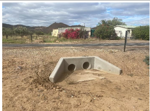
Small stormwater system adjacent to bridge 4837.
