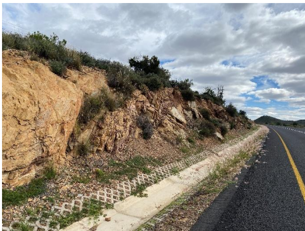
Upgraded side drains off TR 83/2.
