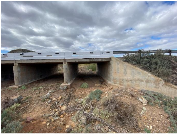
Condition of Bridge 5090.
