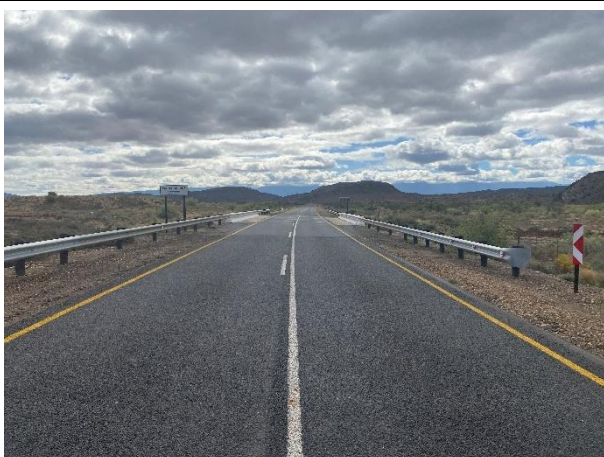
Condition of the newly installed guardrails and road surface at Culvert Bridge 5090.
