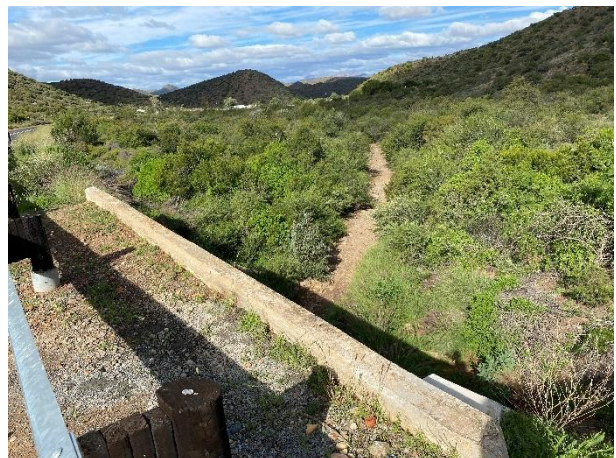
Condition of the vegetation surrounding the bridge.
