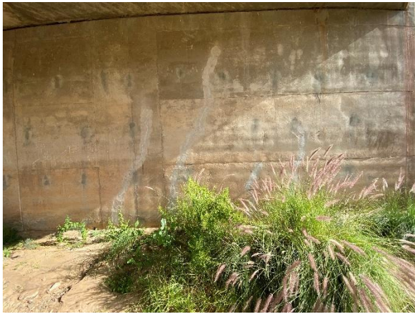
Repairs of vertical and horizontal cracks.
