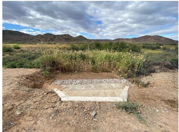
New gabion mattresses installed at the outlet.
