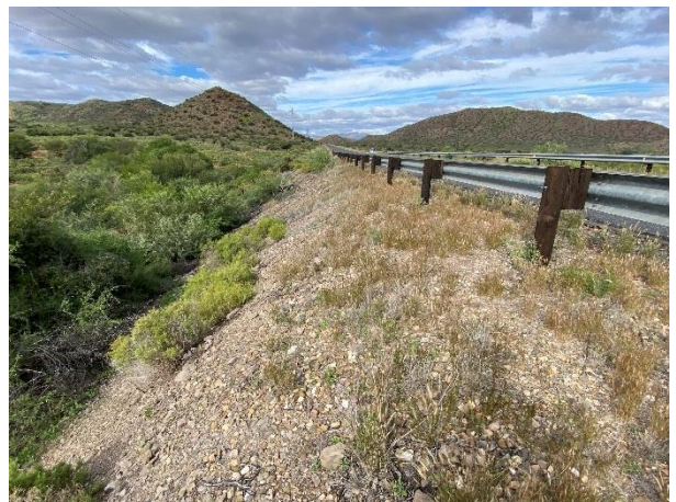
Regraded banks of the bridge.
