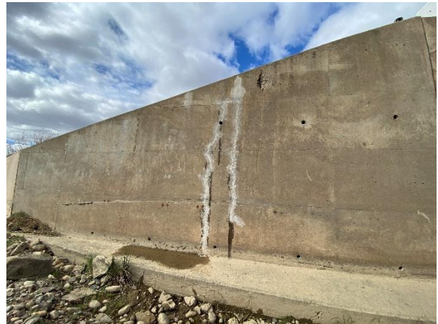
Repairs of vertical and horizontal cracks.
