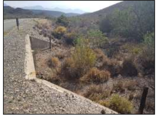
Figure 3: Typical pipe culvert with headwalls.
