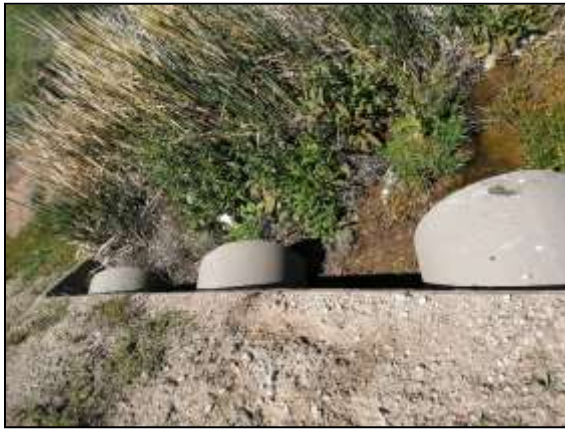
Figure 8: Existing bridge pipe culverts.
