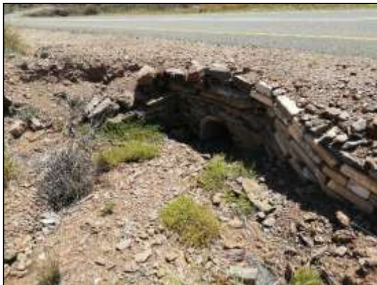
Figure 12: Pipe culvert with headwalls without apron slab.
