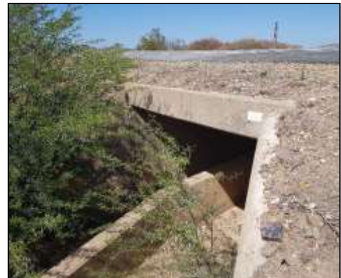
Figure 7: Large box culvert with headwalls and an apron slab.
