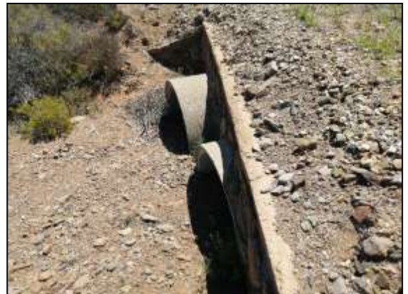
Figure 13: Pipe culverts without headwalls as well as an apron slab.
