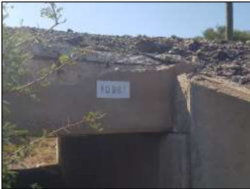
Figure 4: Large box culvert with headwalls.
