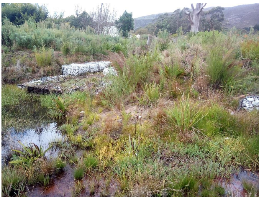
Picture of rehabilitated and established embankments along the same road; MR269; Done by GNEC
