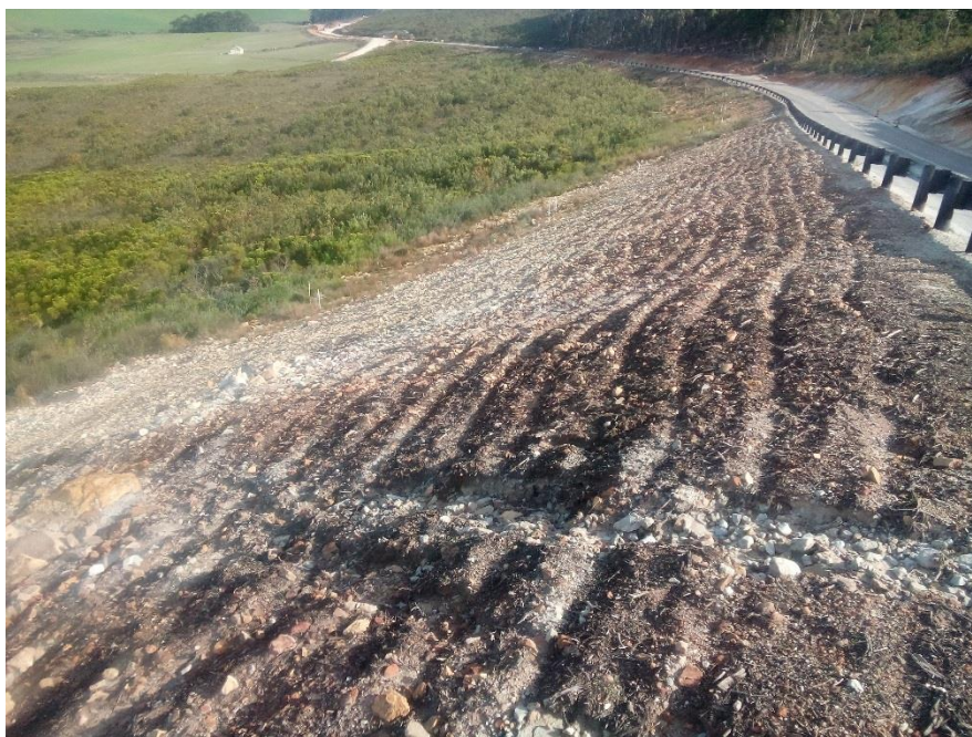
Example of horizontal terracing prior to planting to minimise vertical erosion
