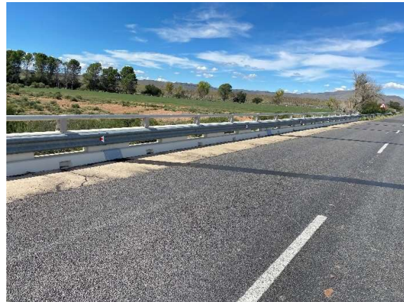
Condition of the completed Brakvallei River brige road surface as seen towards the northwest.
