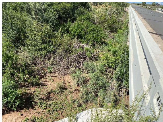
Bridge deck resealed, joints installed, with concrete and pier repairs. Condition of riverbed with spills removed.
