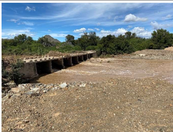
Current condition upstream of the old Buffalo River and the rehabilitated temporary bypass at Km 26.94.
