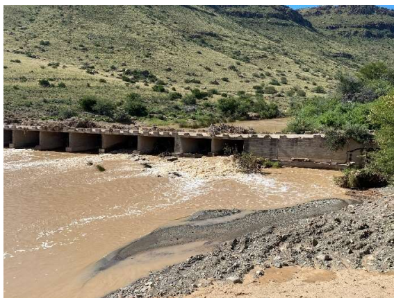
The rehabilitated temporary bypass upstream of the Buffalo River as seen from the southern bank
