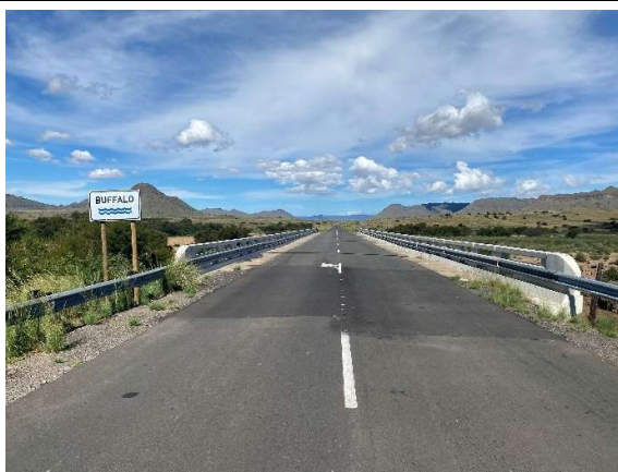
Condition of the Buffalo Bridge.
