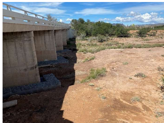
Concrete repairs and erosion protection works (gabion reinforcements) at piers and embankments.
