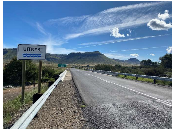
Condition of the Uitkyk Bridge.
