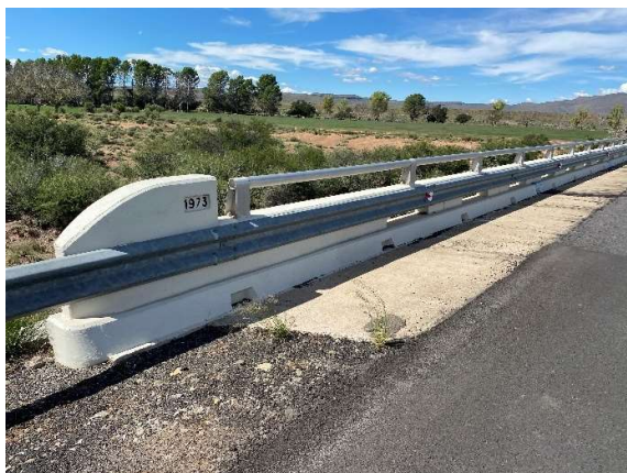
Condition of the new road surface and newly installed guardrails at Brakvallei River Bridge at Km 17.45.
