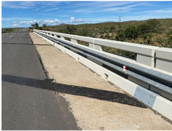
Bridge deck resealed, joints installed, with concrete and pier repairs.
