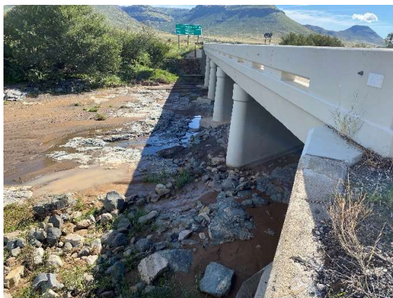
Newly upgraded culvert at the Uitkyk stream on TR 16/9.
