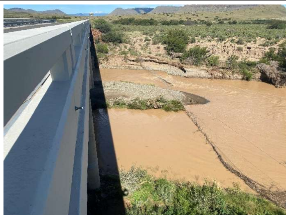
Condition downstream of the Buffalo Bridge.
