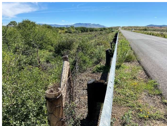
Condition of Gabriel River with newly installed wire fencing for debris.
