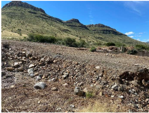
Upstream of the Buffalo River bridge where the temporary bypass road was in place.
