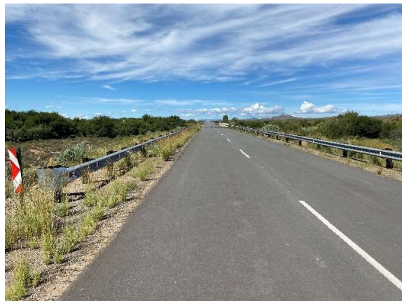
Condition of the completed road surface and road reserve along the TR 16/8 along with the guardrailings.
