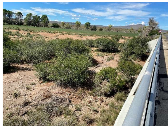
Downstream condition of the Brakvallei River bridge..
