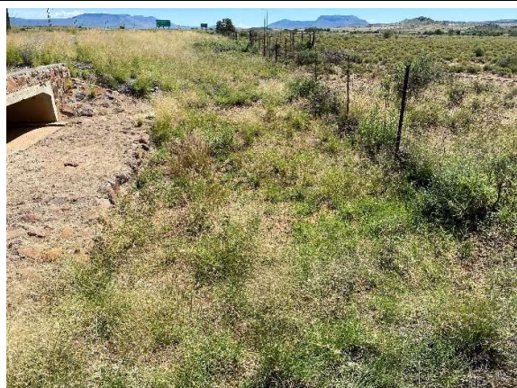
Condition of vegetation surrounding the upgraded culverts.
