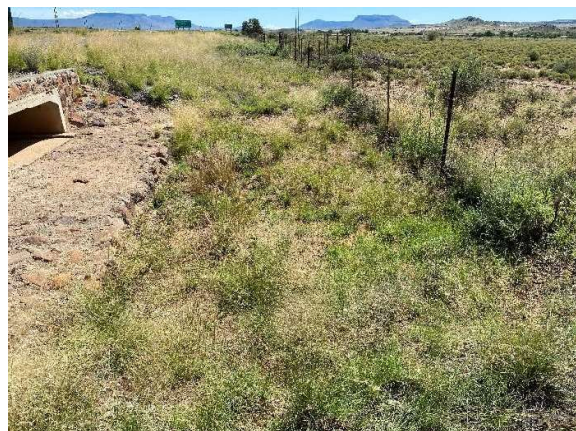
Condition of vegetation surrounding the upgraded culverts.
