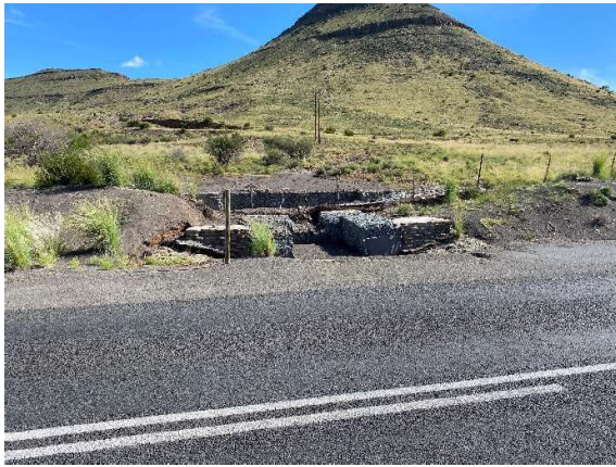
Newly installed gabion baskets for sediment within the road reserve at approximately Km 34.6 on TR 16/9.
