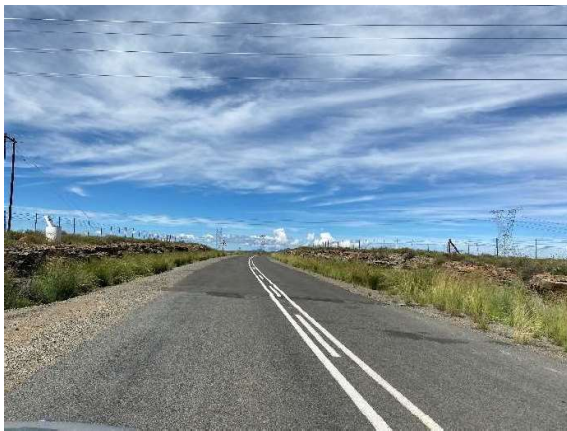
Northern end of the contract on the provincial border showing the upgraded road surface.
