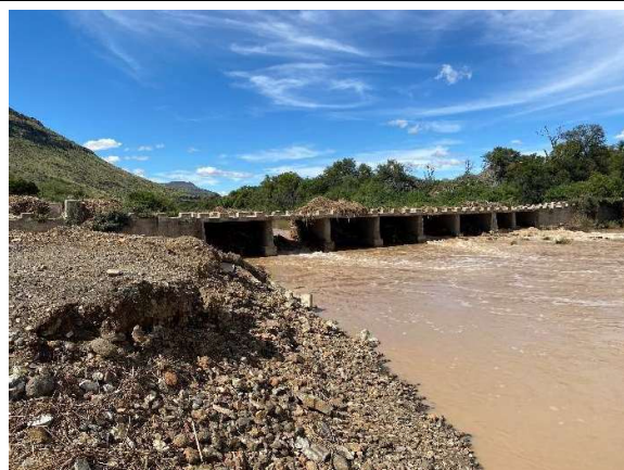
The old bridge upstream of the Buffalo River bridge as seen from the northern river bank towards the northeast.
