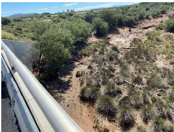
Upstream condition of the Brakvallei River bridge.
