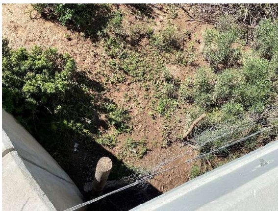
Condition of Gabriel Riverbed with newly installed wire fencing for debris.
