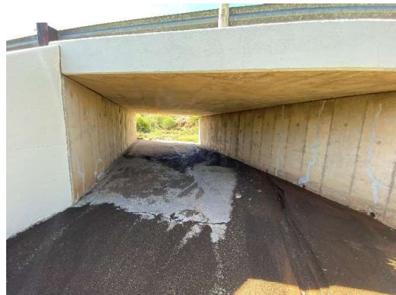
Culverts upgraded with new concrete structures, erosion control, and clearing of vegetation.
