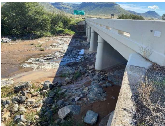
Newly upgraded culvert at the Uitkyk stream on TR 16/9.
