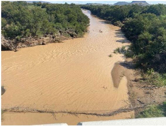
From the Buffalo River bridge seen downstream towards the southwest.
