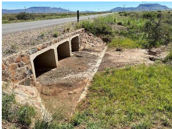
Culverts upgraded with new concrete structures, erosion control, and clearing of vegetation along TR 16/8.
