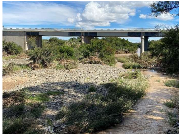
Upstream of the Buffalo River bridge as seen from the northern river bank to the southwest.
