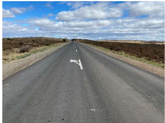
Condition of the completed road surface and road reserve along the TR 16/8.
