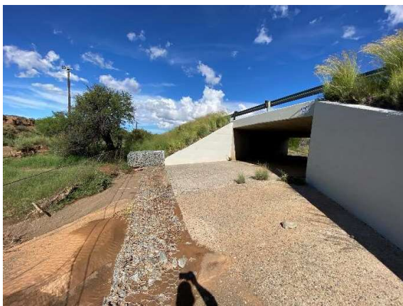
Culverts upgraded with new concrete structures, erosion control, and clearing of vegetation.
