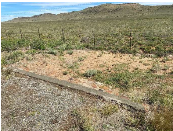
Culvert upgrading includes repaired concrete structures, stone-pitching, erosion control, and vegetation clearing.
