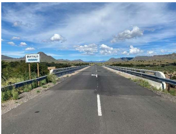
Condition of the Buffalo Bridge.
