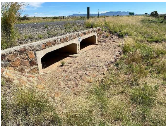
Upgraded culvert on TR 16/8 with repaired concrete and stone-pitching, daylighting and vegetation clearance.
