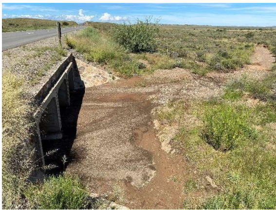
Culverts upgraded with new concrete structures, erosion control, and clearing of vegetation along TR 16/8.
