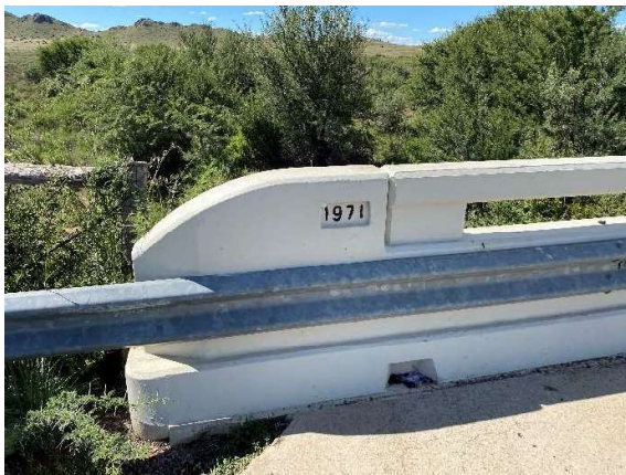
Newly installed guardrails at B4611: TR16/8 at Km 46.11 (Gabriel Stream).
