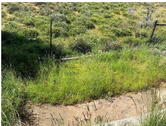
Culverts upgraded with new concrete stone pitch structures, and clearing of vegetation along TR 16/8.
