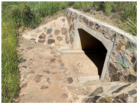
Culverts upgraded with new concrete stone pitch structures, , and clearing of vegetation along TR 16/8.
