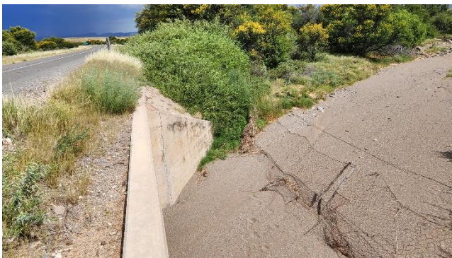
FIGURE 12: SITE PHOTO OF AN EXISTING CULVERT ALONG TR16/9.
