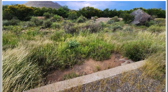
FIGURE 15: SITE PHOTO INDICATING VEGETATION IN THE AREA AT AN EXISTING CULVERT ON TRUNK ROAD 16/9.
