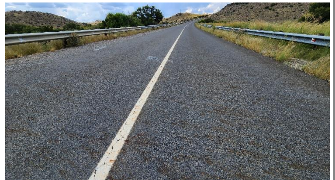
FIGURE 9: SITE PHOTO OF THE EXISTING TR16/9 ROAD BETWEEN MURRAYSBURG AND THE N1 NATIONAL ROAD.
