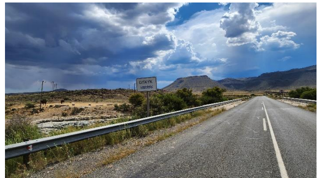
FIGURE 13: SITE PHOTO OF THE ROAD AT THE UTKYK RIVER / BRIDGE (TRUNK ROAD 16/9).
