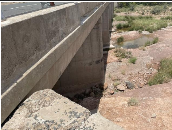
FIGURE 6: PHOTO OF THE EXISTING GABRIEL STREAM BRIDGE ON TR16/8 INDICATING A WATERCOURSE.
