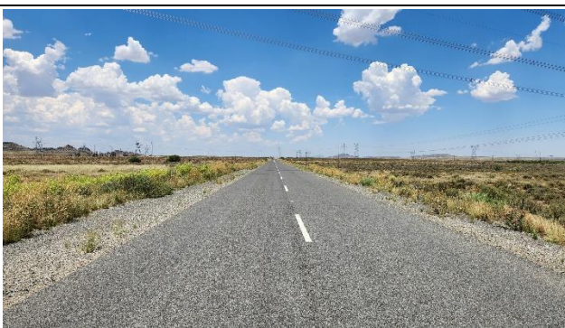
FIGURE 2: SITE PHOTO OF THE EXISTING TR16/8 ROAD.
