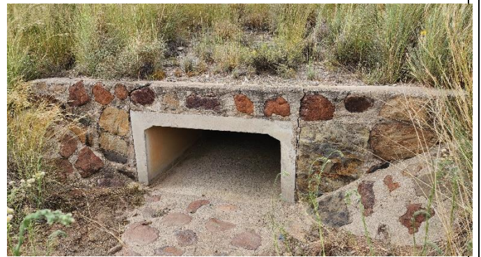
FIGURE 11: SITE PHOTO OF AN EXISTING CULVERT ALONG THE ROUTE OF TR16/9.
