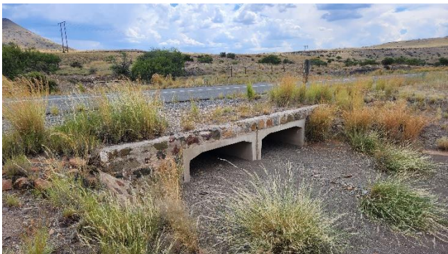
FIGURE 8: SITE PHOTO OF AN EXISTING CULVERT AT KM NO. 30.15 ON TR16/9.
