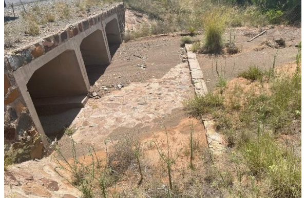
FIGURE 5: SITE PHOTO INDICATING BOX CULVERTS.
