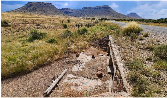
FIGURE 16: SITE PHOTO INDICATING AN EXISTING CULVERT ALONG THE ROUTE.
