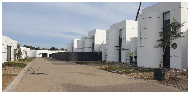
Condition of the first few constructed units off Hyacinth Lane.
