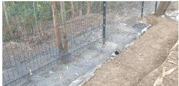
Contractors busy installing the gabion base along the low-lying sections of the buffer area.
