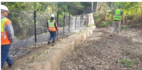
Installed hay bales and gabion mattresses towards the corner of the property.
