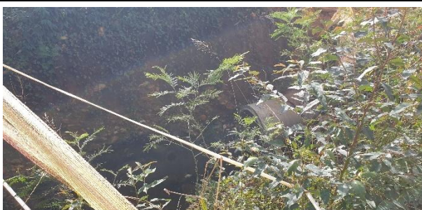
Stormwater outlet towards the riparian area.
