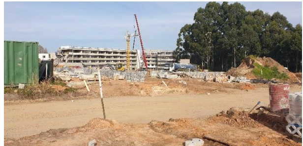
Construction laydown area where civil services are being installed.
