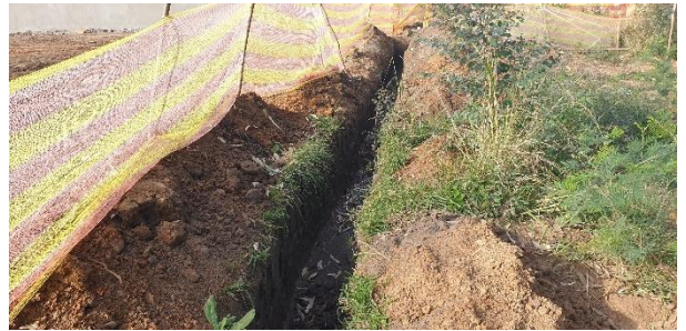
Electrical lines being installed.
