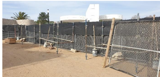
Screening around the construction area in place.
