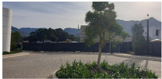
Construction area is screened at the entrance of the site along Soapberry Close and Nature Boulevard.
