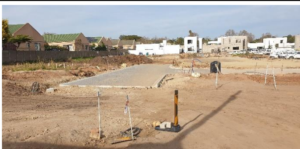
Civil services being installed along with the roads being paved.
