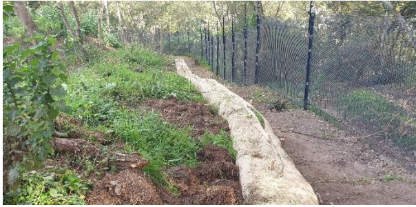
Newly installed hay bale along the riparian zone and security fence.
