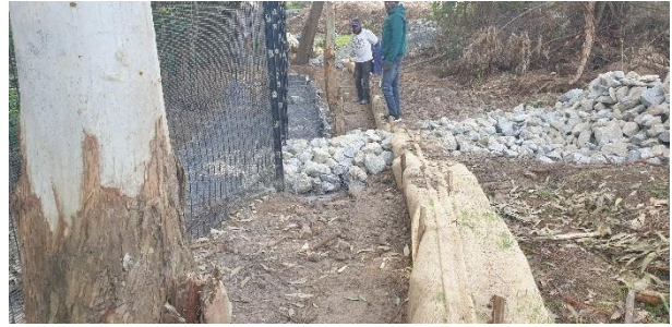
Contractors busy installing the gabion base along the low-lying sections of the buffer area.
