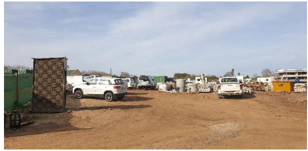
Construction site camp.
