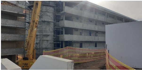
Demarcation in place around the construction of the apartment blocks.
