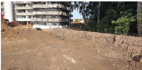
Topsoil temporary swale for stormwater diversion and will be used for rehabilitation.
