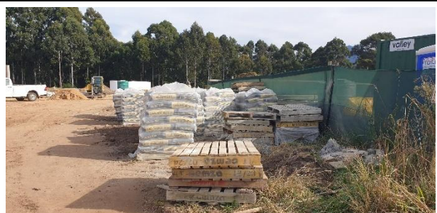
Laydown area adjacent to the site camp.
