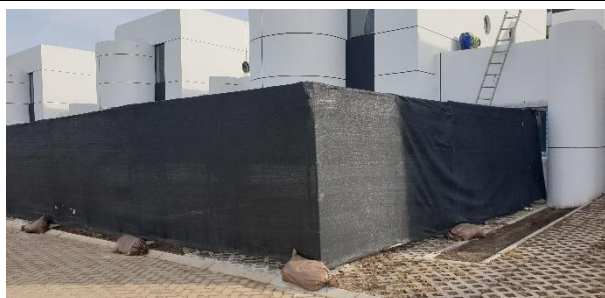
Screened construction area off Hyacinth Lane.
