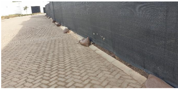
Screening held in place with sandbags.
