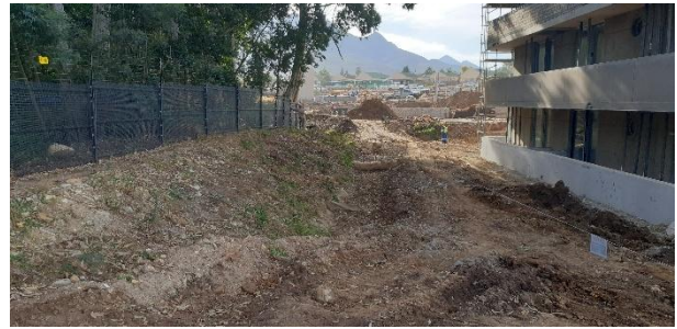
Temporary stormwater channels for surface flow.
