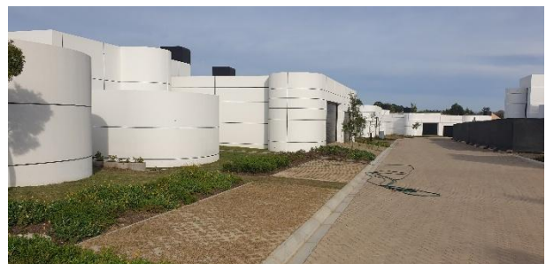
Permeable paving "grass block", SUDS intervention.
