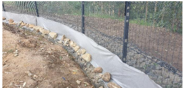
Gabion mattresses installed to prevent uncontrolled surface flow.
