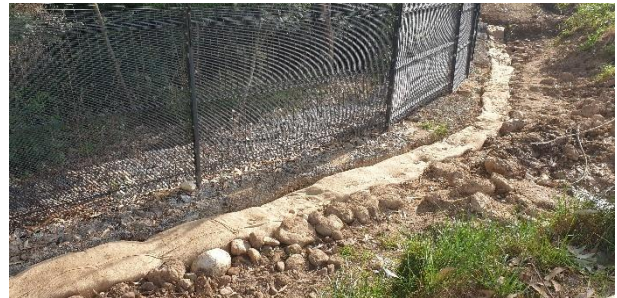
Installed hay bales along the security fence.
