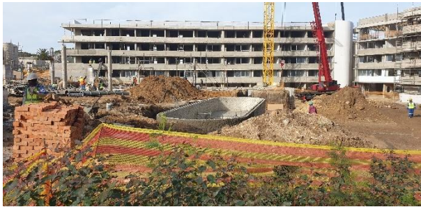
Clubhouse pool and associated infrastructure being constructed.
