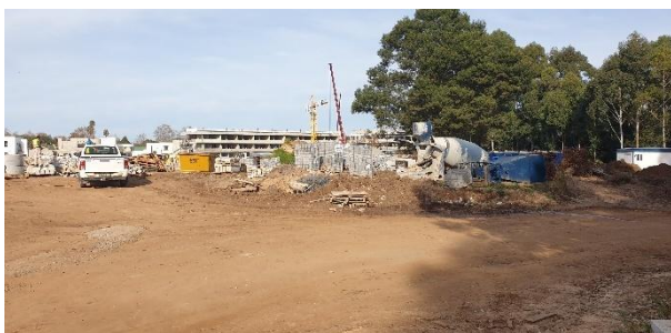
Temporary construction laydown area.
