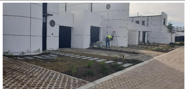
Permeable paving "grass block", SUDS intervention.
