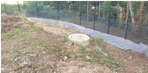
Security fence installed along with sewage service that has been tied into the municipal network.
