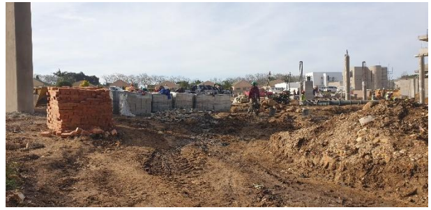
Construction area and temporary laydown area of construction material.
