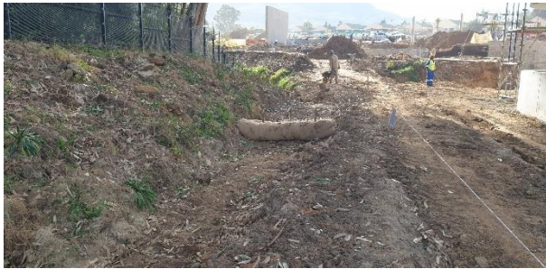
Temporary stormwater channels for surface flow with hay bales.
