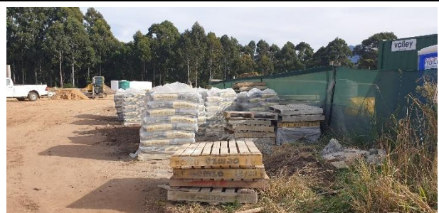
Laydown area adjacent to the site camp.
