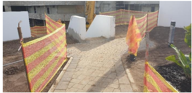
Demarcation in place surrounding the landscaping area and surrounding construction area.
