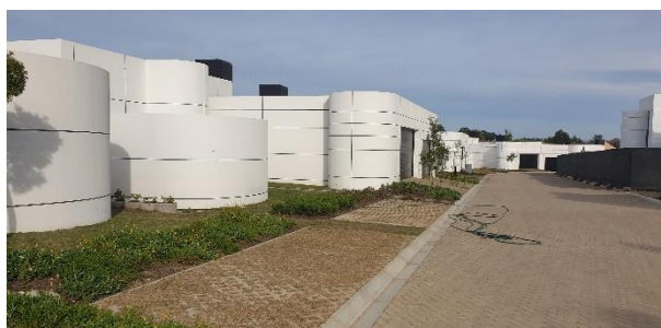
Permeable paving "grass block", SUDS intervention.
