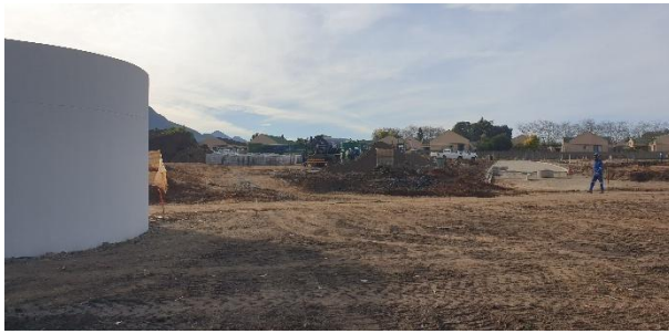
Water truck available for dust suppression.
