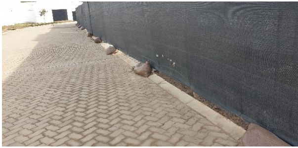
Screening held in place with sandbags.
