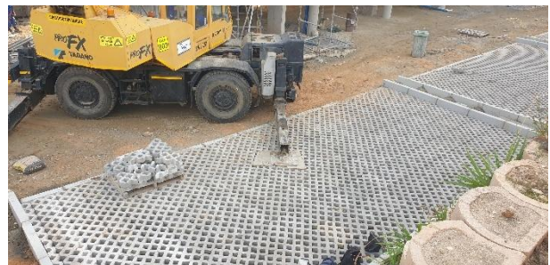
SUDS being installed.
