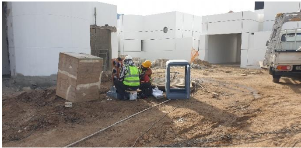
Electrical installations in progress at the individual units.
