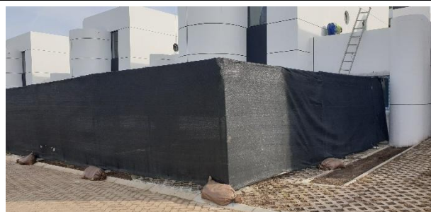
Screened construction area off Hyacinth Lane.
