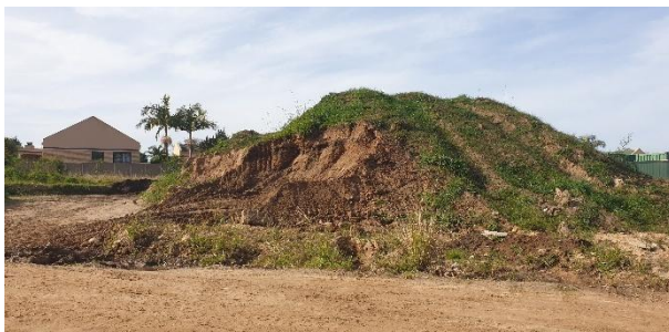
Topsoil and subsoil stockpiles were excavated after roadways were cleared.
