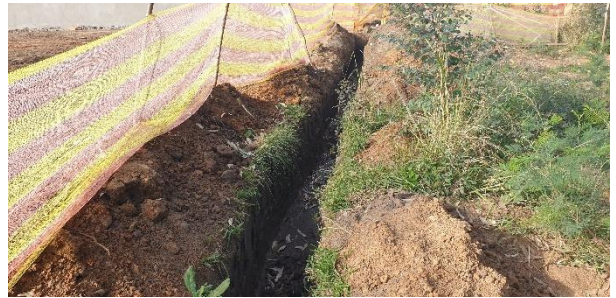
Electrical lines being installed.
