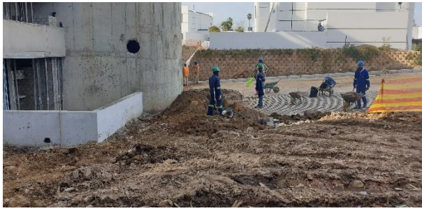
Civil services along the apartment block being installed.
