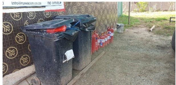
Fire extinguishers available at the site camp.
