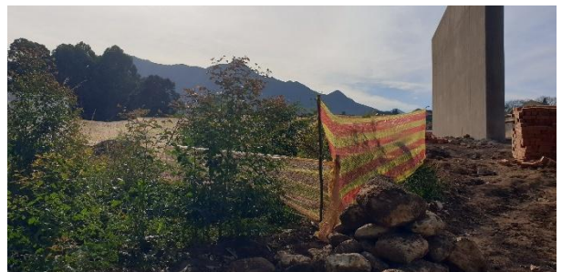
Demarcation surrounding the stormwater outline.
