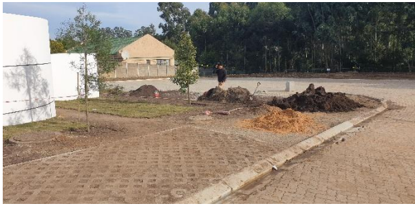
Landscaping of outside gardens in progress.
