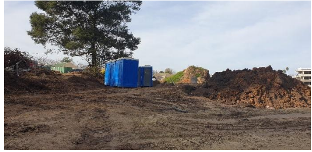
Chemical toilets in place along the construction areas.
