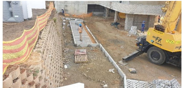
Demarcation in place around the construction of the apartment blocks.
