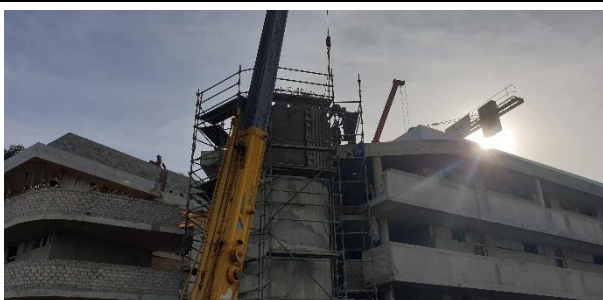
Construction of the apartment units.
