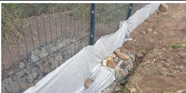
Gabion mattresses installed to prevent uncontrolled surface flow.
