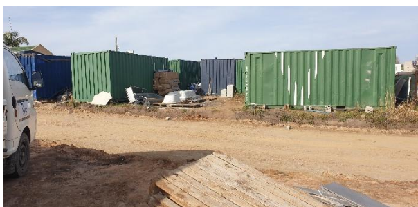
Lockable storage containers within the site camp.
