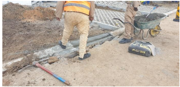
Curbs being installed.
