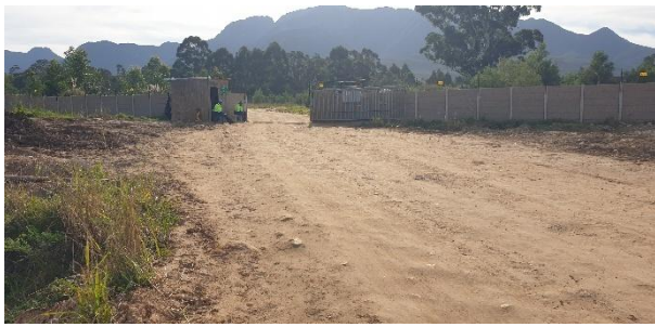
Temporary access road off plantation road.
