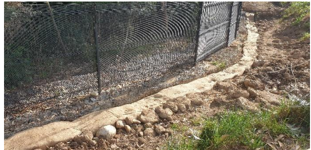
Installed hay bales along the security fence.
