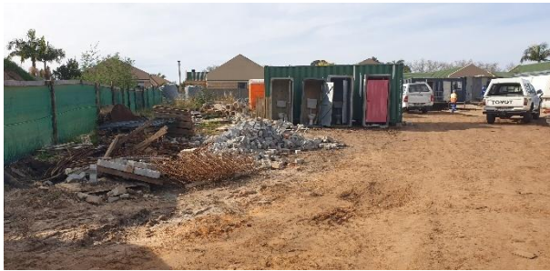
Construction site camp with build in toilets feeding into the sewage network on-site.
