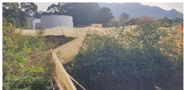
Demarcation surrounding the stormwater outline.
