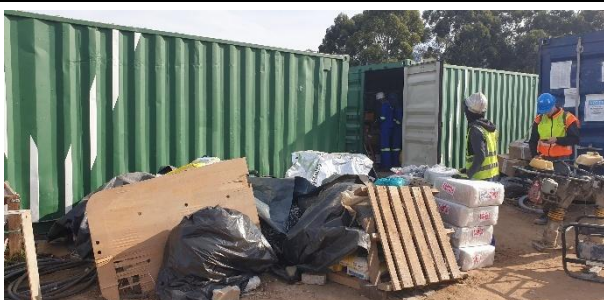
Lockable storage containers within the site camp.
