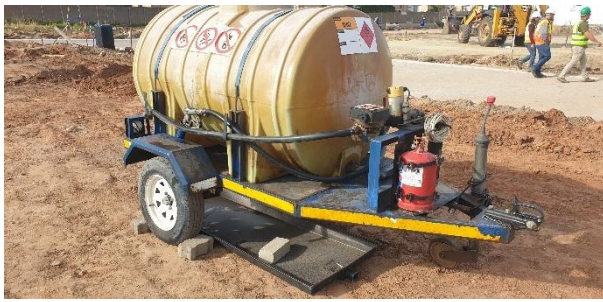
Drip tray in place below the fuel bowser.
