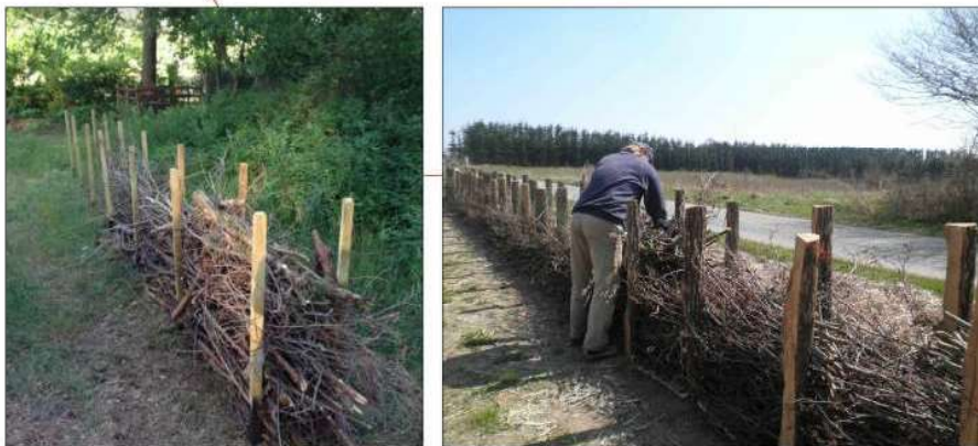
PROPOSED PACKED BRUSH FENCE 2m FROM RIVER BANK TO PROTECT REHABILITATION PLANTING
