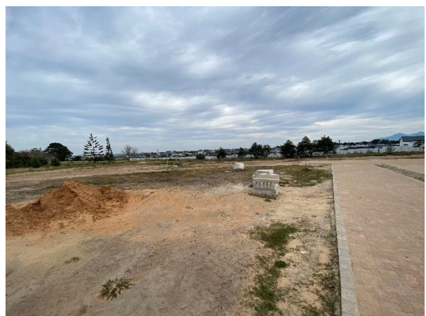
Cleared area for the next phase of development. Paving and curb installations in progress.
