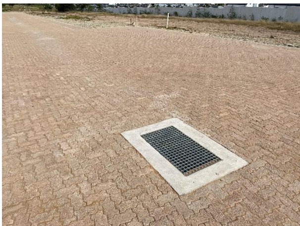
Central stormwater channel.
