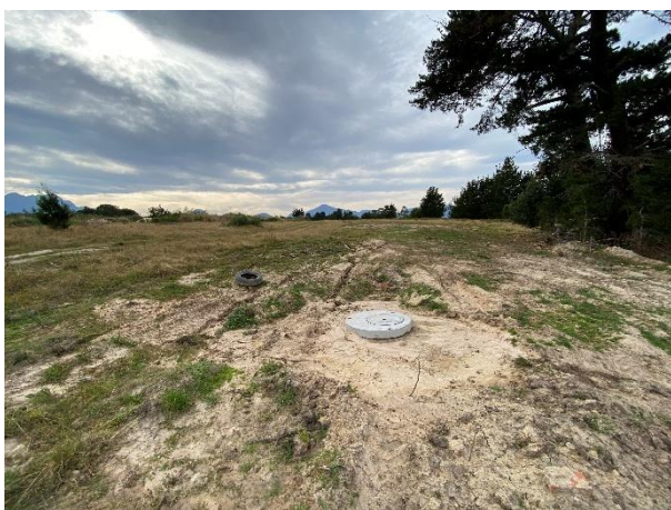
Successfully installed sewage pipeline towards the Modderrug River.
