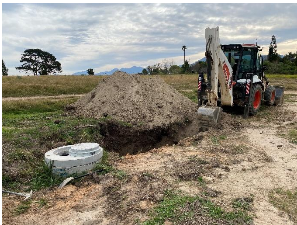
Sewage systems being installed towards the entrance of the site.
