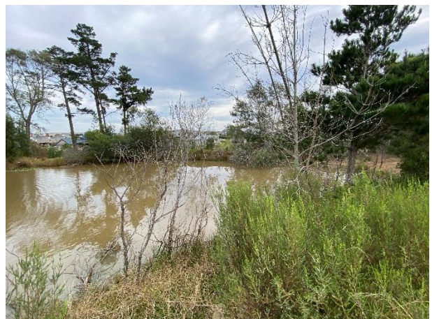
On-site dam to be reconstructed into a retention pond.
