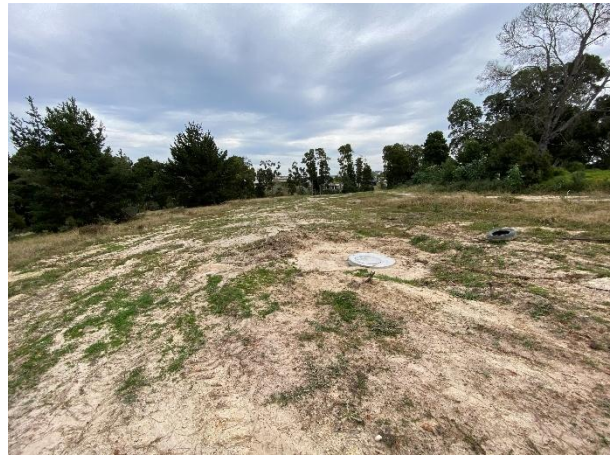
Successfully installed sewage pipeline towards the Modderrug River.
