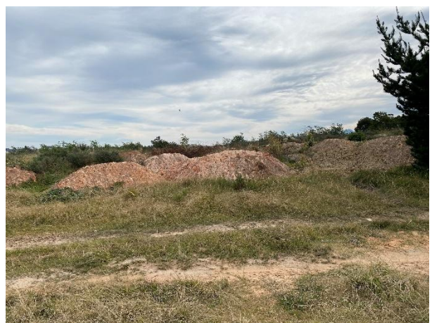
Stockpiled subsoil and topsoil after site clearance.
