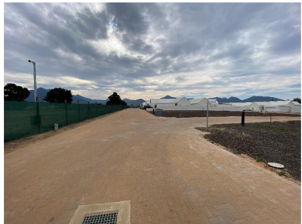
Condition of the first completed residential phase.
