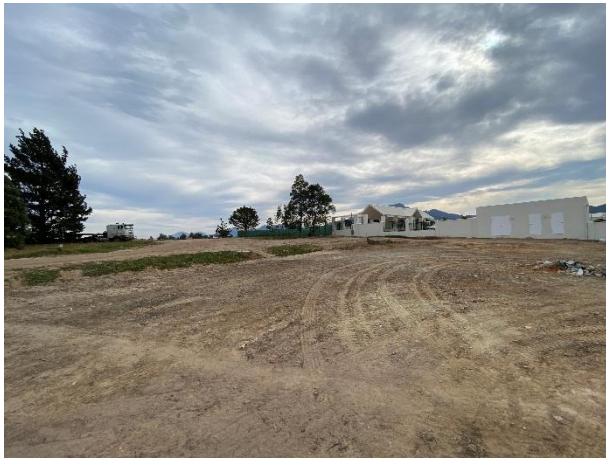
Cleared area for the next phase of development where services are being installed.
