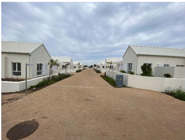
Condition of the first completed residential phase.
