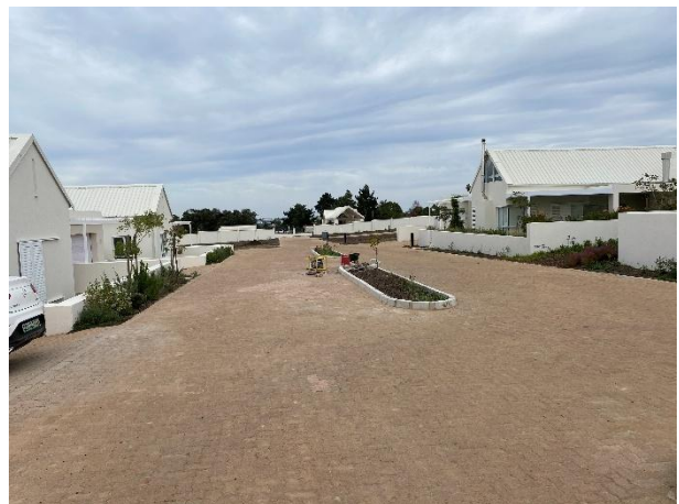
Condition of the first completed residential phase.
