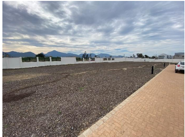
Cleared area for residential units mulched with woodchips.
