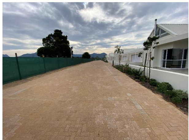
Condition of the first completed residential phase with screening in place.
