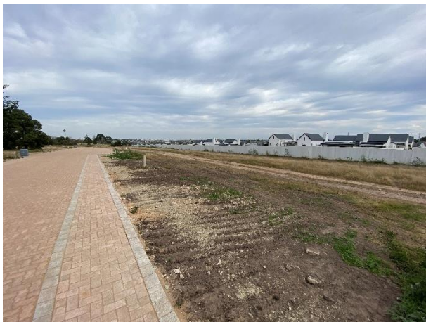
Condition of rehabilitated cleared sites where services were installed.
