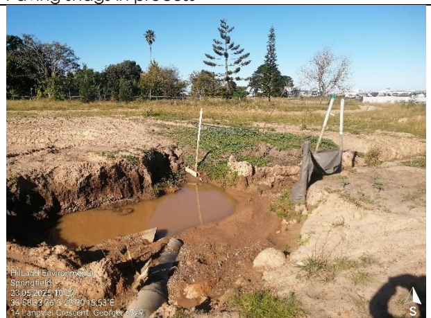
Temporary stormwater outlet shaping to be finalised. Silt fence is in place.
