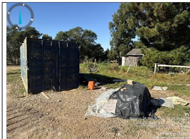
Site camp area
