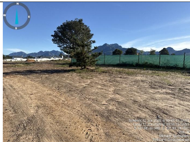
Construction material stockpile area still need to be rehabilitated.
