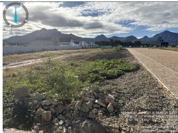
Paving snags in process. Invasive aliens as a result of construction activity to be removed by the contractor. Construction rubble to be disposed at the municipal disposal facility.
