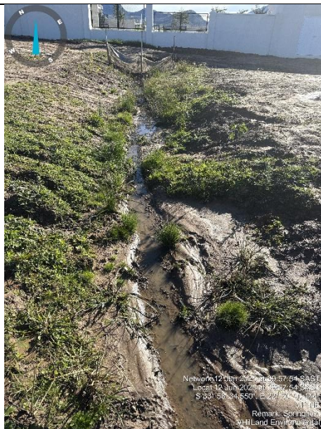
Silt fences are in place and must be maintained.
