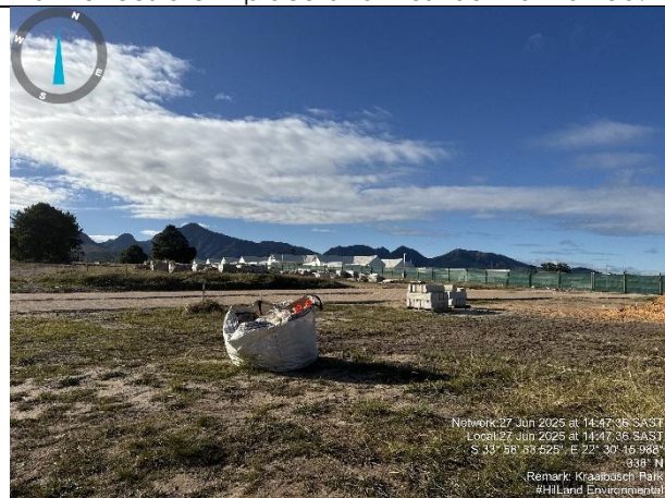
Litter / waste bags on site.
