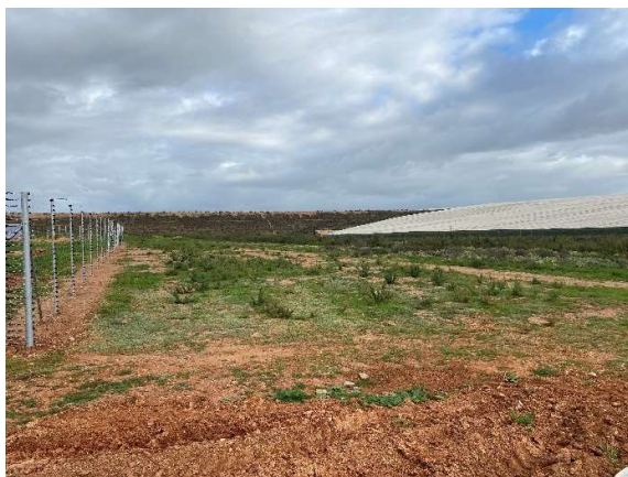
From the northwestern boundary of the site footprint as seen towards the south.
