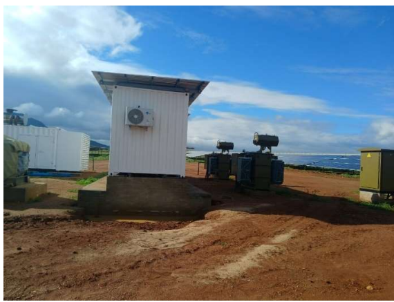
Completed electrical control stations.
