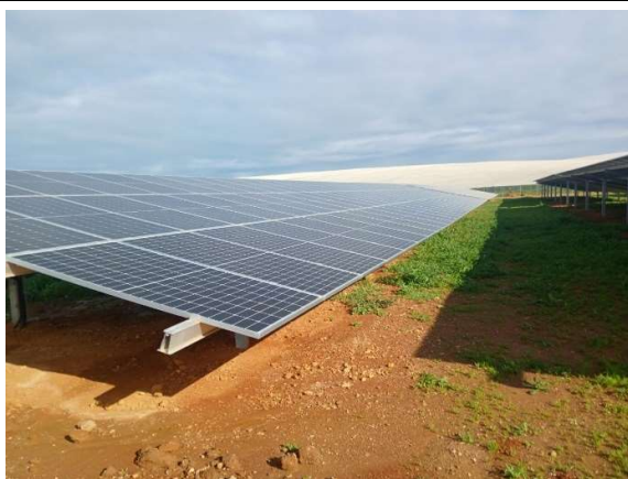
Condition of the completed panel structures as seen towards the west.
