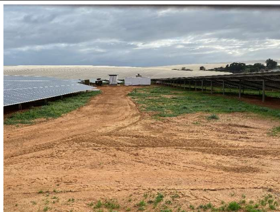
From the entrance gate to the site seen towards the west and the control station.
