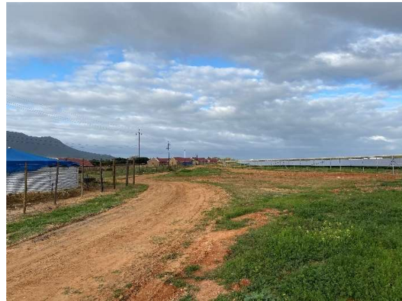
From the ring main unit as seen towards the east along the northern boundary access road.
