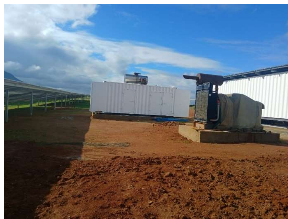
Completed electrical control stations.
