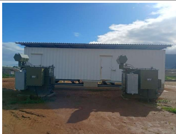
Completed electrical control stations.
