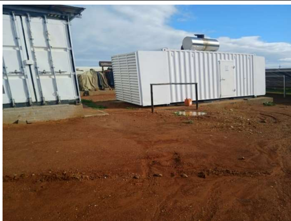
Completed electrical control stations.
