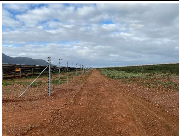
The access road along the southern boundary of the site as seen towards the east.
