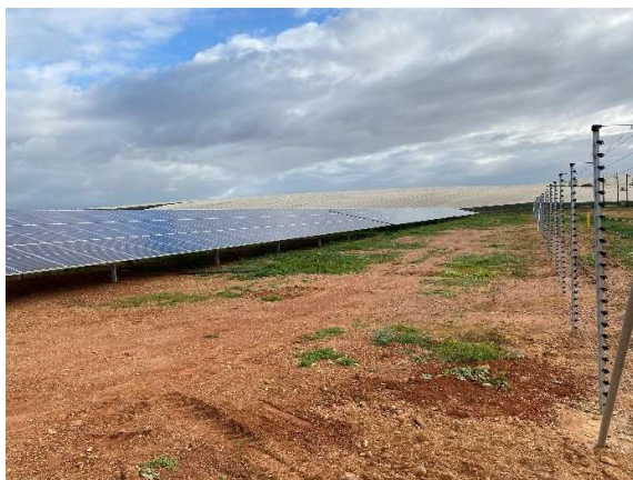
Along the inside of the northern fence as seen towards the west.
