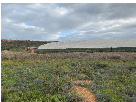
The location of the water pipeline within the no-go area has been overgrown again with indigenous veld.
