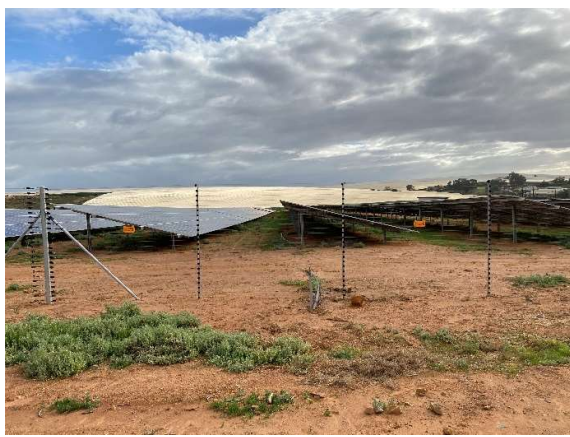
Condition of the completed panel structures as seen from the eastern boundary towards the west.
