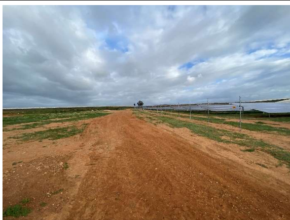
The access road leading around the site boundary along the east of the site seen towards the south.
