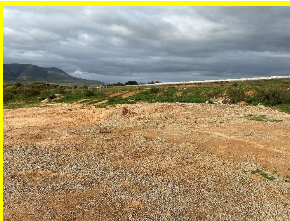
Adjacent to the site camp area, some remaining building sand and aggregate for mixing concrete is still in place.
