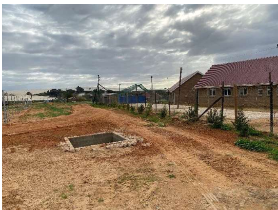
Stormwater catchpit along the northern boundary of the site between the footprint and the houses.
