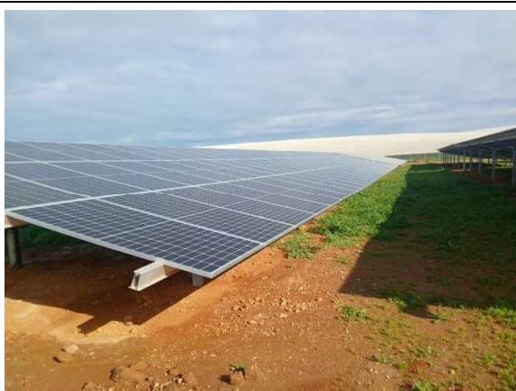
Condition of the completed panel structures as seen towards the west.
