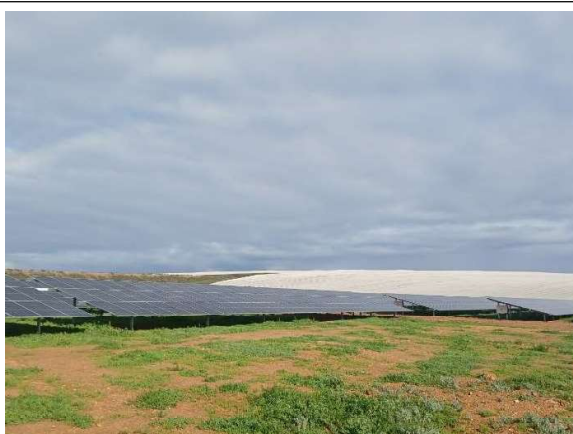
Solar panels and condition of completed works as seen from the northeastern corner towards the southwest.
