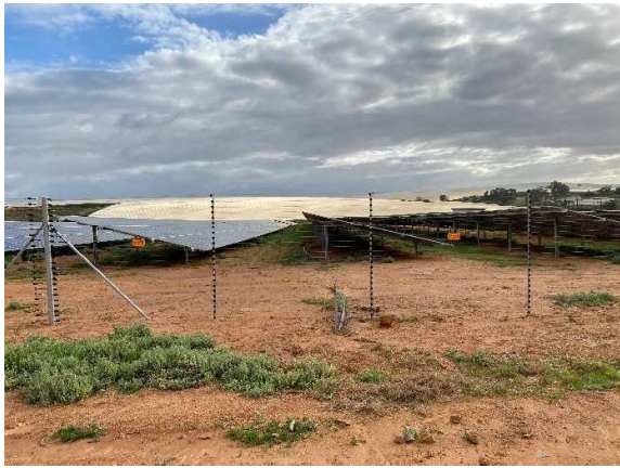
Condition of the completed panel structures as seen from the eastern boundary towards the west.
