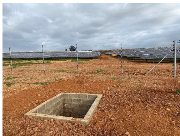
Completed stormwater catchpit along the northern boundary of the site as seen towards the south.
