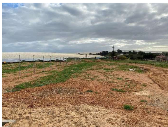
Along the northern boundary of the site as seen towards the west where stormwater measure were completed.
