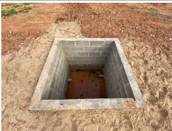
Condition of a completed stormwater catchpit along the northern boundary of the site.
