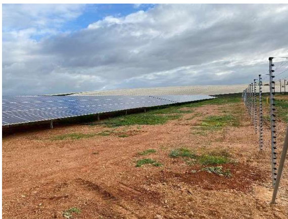
Along the inside of the northern fence as seen towards the west.
