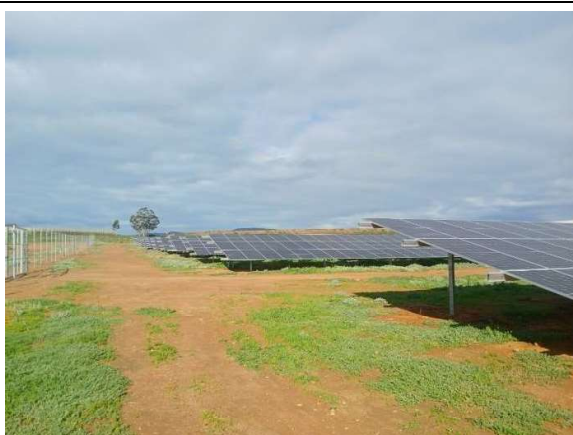
Condition of the completed panel structures along the eastern boundary as seen towards the south.
