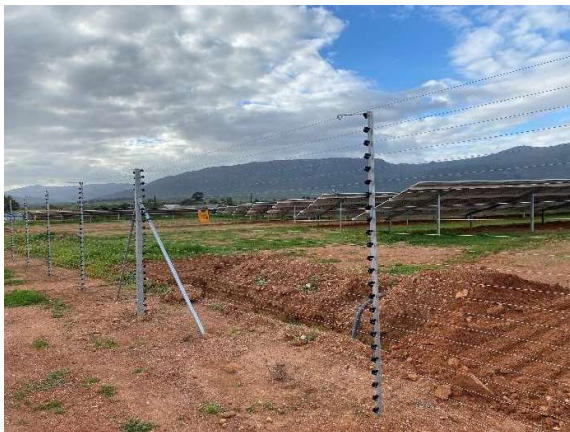
Along the western boundary of the site where the water pipeline connects to the internal water pipeline.
