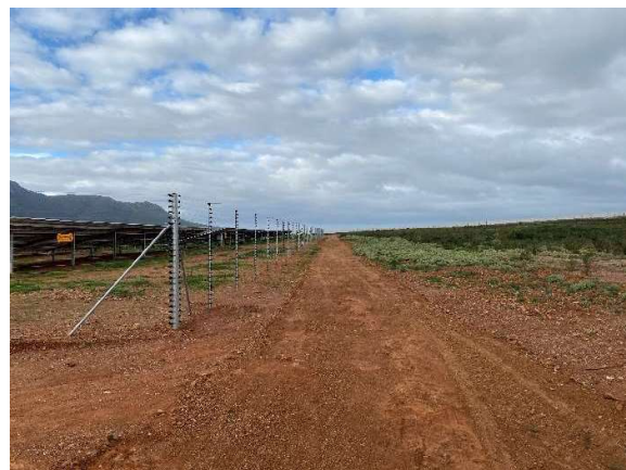
The access road along the southern boundary of the site as seen towards the east.
