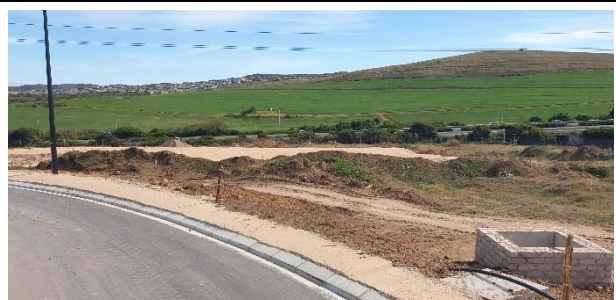
View of the construction area towards the school.
