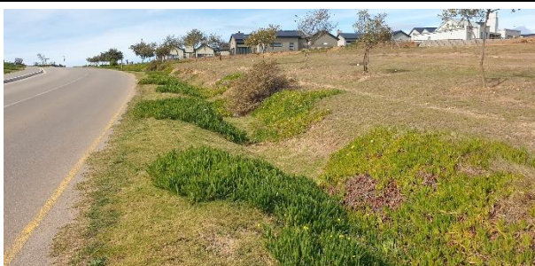
Rehabilitated stormwater channels along the roadside.
