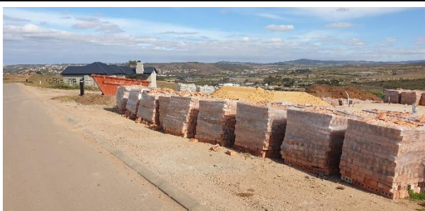
Construction of townhouses within Phase D.
