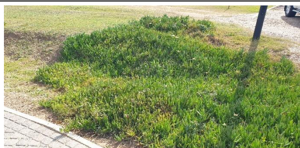
Rehabilitated stormwater channels along the roadside.
