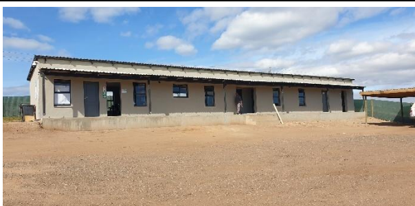
Site offices located within the screened site camp within Phase A adjacent to the N2.
