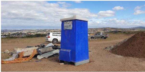
Chemical toilet located within the development area of Phase C – retirement village.
