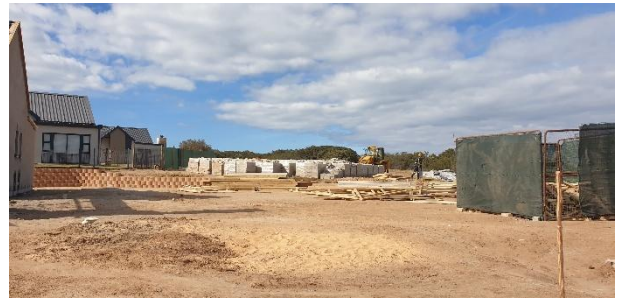
Construction of retirement units in Phase C.
