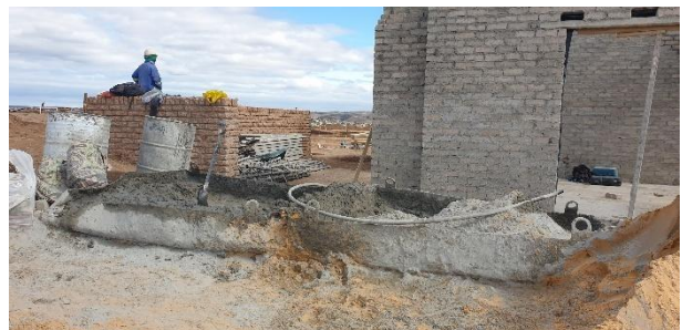
Cement batching active with large mortar boards in place.
