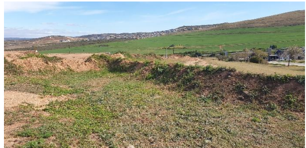
Temporary stormwater swales for natural stormwater diversion adjacent the entrance road of erf 7380.
