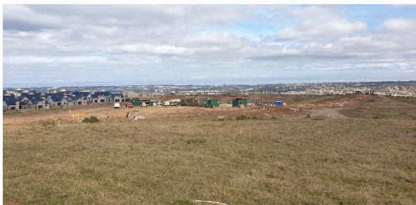
Phase B construction site camp.
