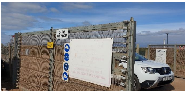
Site office being de-established adjacent to Erf 7380.
