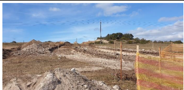
Main access road being constructed and services installed.
