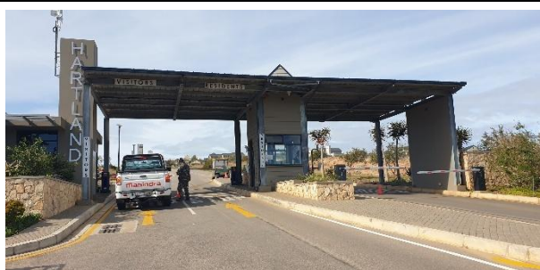
Current main entrance to Hartland Lifestyle Estate from the MR344 through the existing culvert under the N2.
