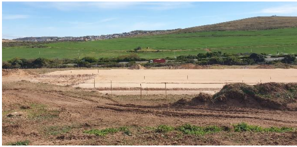
Levelled, shaped and cut school area.
