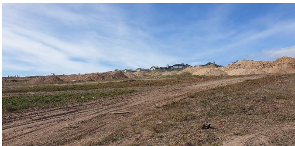
Topsoil and subsoil stockpiles of cleared erven within Phase D and A.
