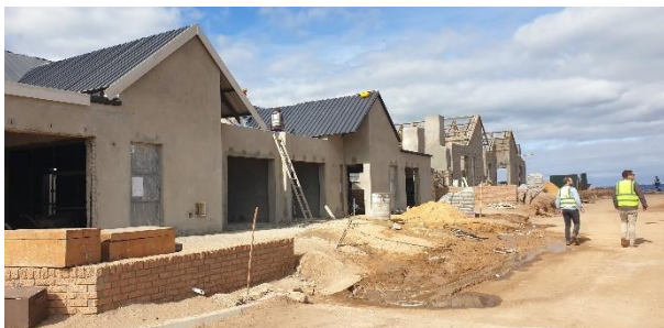
Condition of the construction area within the retirement village.
