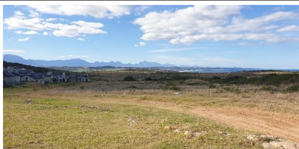
Ring road surrounding the development boundary.
