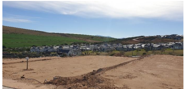
Installation of services and earthworks for erven within Phase A, with retaining walls being established.
