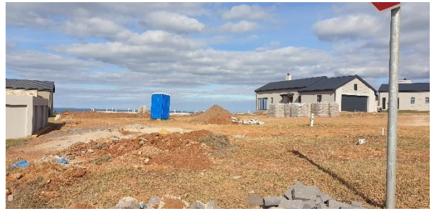
Condition of the development area of Phase H towards the North.
