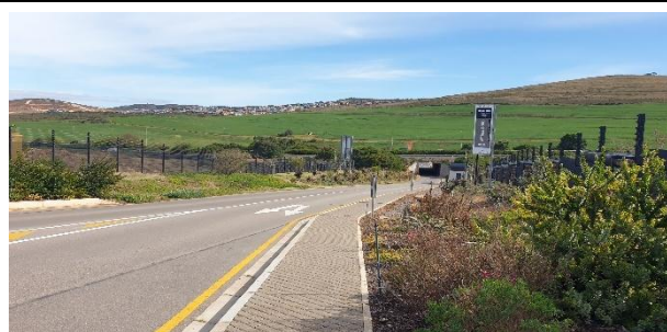
Entrance to Hartland Lifestyle Estate from the MR344. Landscaping within natural vegetation.
