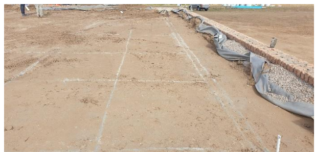
Setting out of foundation lines marked on site in preparation for excavation.
