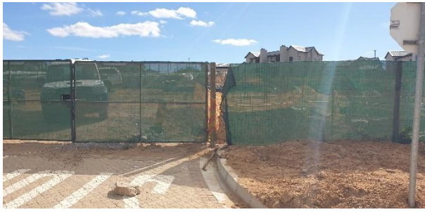
Construction area along Phase B screened within green netting to limit visual intrusion.
