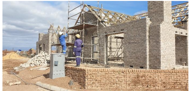
Construction of retirement units within Phase C.
