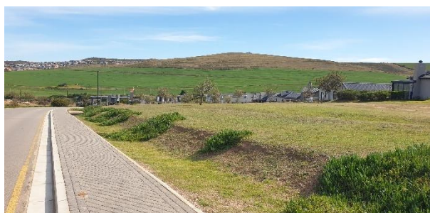
Stormwater is conveyed via natural roadside swales.
