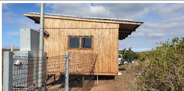
Guard building at the Kleinbrak Estuary access route.
