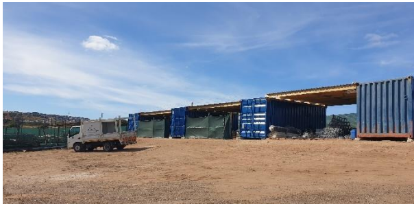
Storage containers available at the main site camp within Phase E adjacent to the N2.
