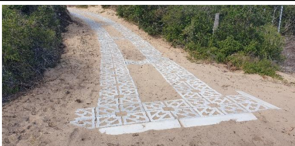
Permeable paving grids installed along the access track to stabilise sandy soils and prevent erosion.
