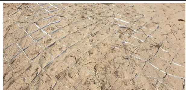
Geogrid netting installed to stabilise sand and manage erosion.
