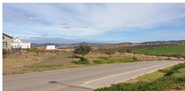
Condition of the site towards Phase A.
