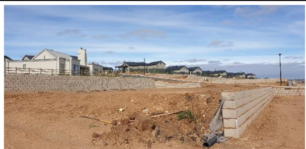
Installation of services and earthworks for erven within Phase A, with retaining walls being established.
