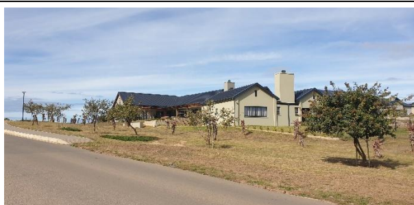
Landscaping with indigenous trees towards the showhouse.
