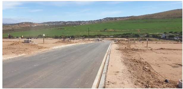
Kerbs are being installed along with the installation of services in Phase A.
