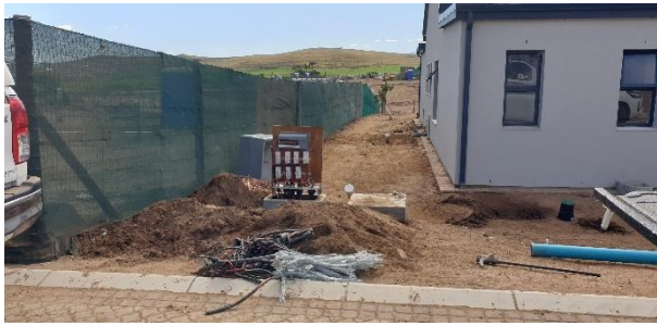
Electrical connections being prepared for distribution to various service points.
