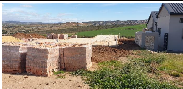
Construction of townhouses within Phase D.
