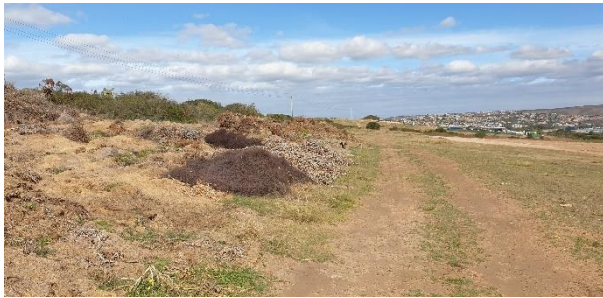
Stockpiles of vegetation and debris during the clearance of the site for the sports field and school area.
