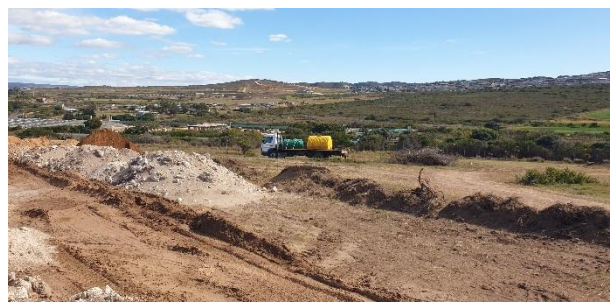
Main access road being constructed and services installed. Water truck available for dust fallout.
