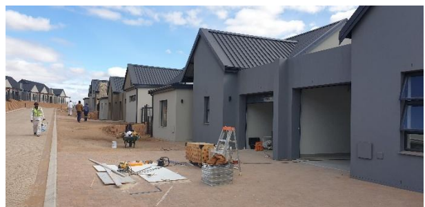
Final finishes of retirement units within Phase C.
