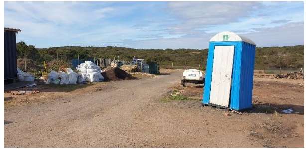
Condition of the construction camp adjacent to Erf 7380, chemical toilet in place.
