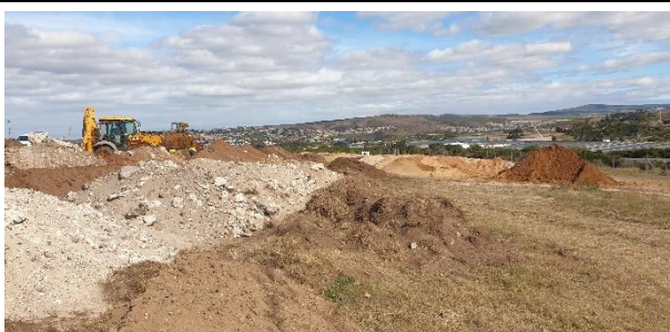
Topsoil and subsoil stockpiles separated during the excavation of the main access road and service installations.
