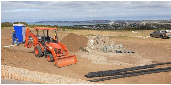
Material stockpiles within the construction area of Phase C.
