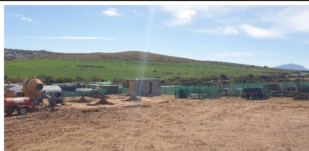
Condition of the main site camp within Phase E adjacent to the N2.
