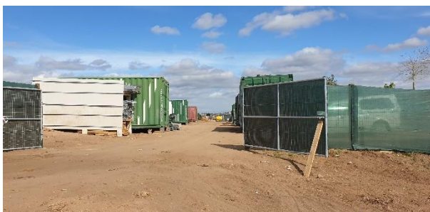
Condition of the main site camp within Phase E. Storage containers for each contractor currently commissioned.
