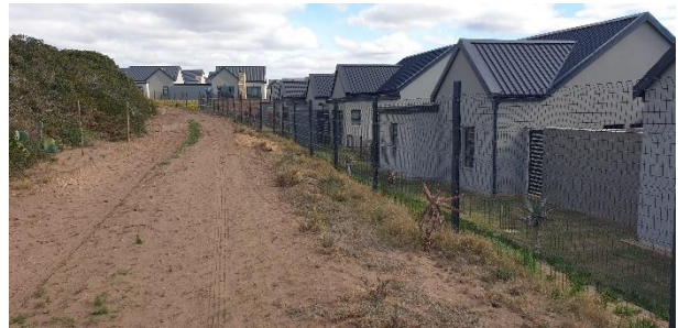
Phase C – Retirement Village boundary fence.
