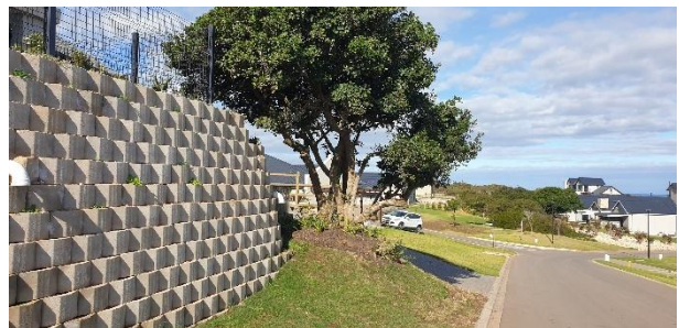
Existing Milkwood tree kept within the road designs.
