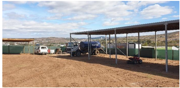
Water truck available at the main site camp within Phase E adjacent to the N2.
