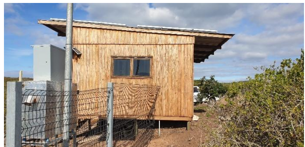
Guard building at the Kleinbrak Estuary access route.
