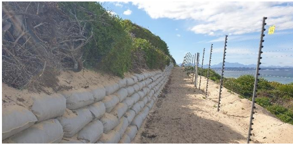
Sandbags placed along the property boundary to stabilise sections of unstable soil.
