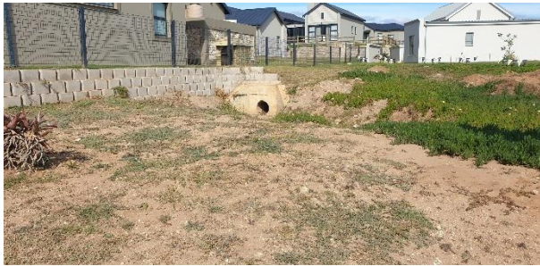
Stormwater outlet structure from Phase A and erf 7380.
