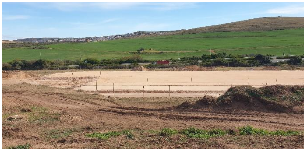
Levelled, shaped and cut school area.
