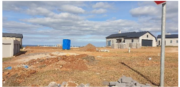
Condition of the development area of Phase H towards the North.
