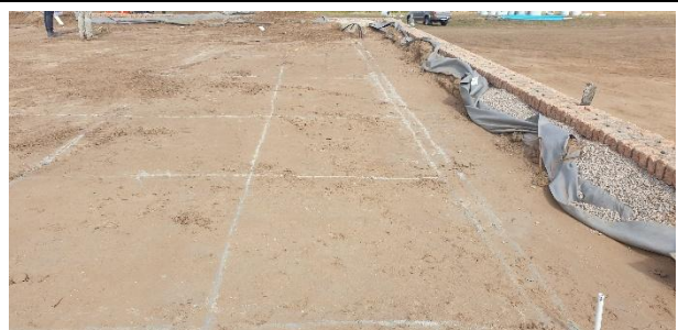
Setting out of foundation lines marked on site in preparation for excavation.
