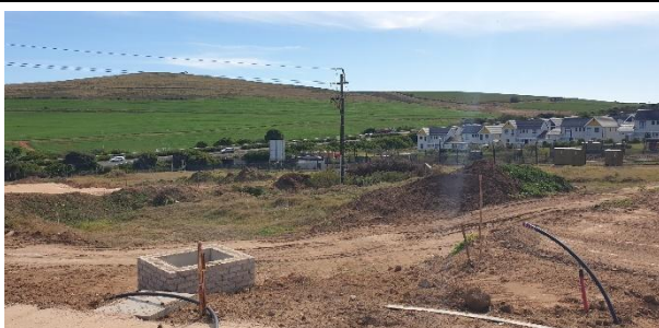
Topsoil stockpiles from the excavation site of the proposed school.
