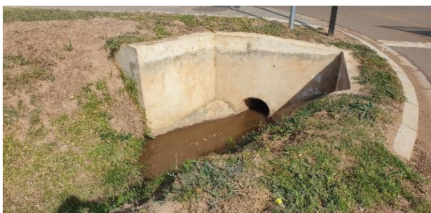
Stormwater inlet and outlet structure.
