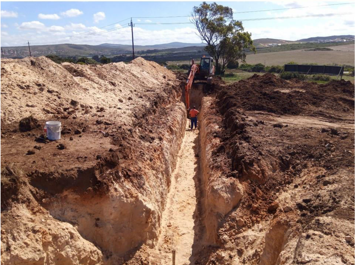
Figure 8. Hartland – Phase A – Klein Karoo Civils – vegetation stripping and excavations in progress.
