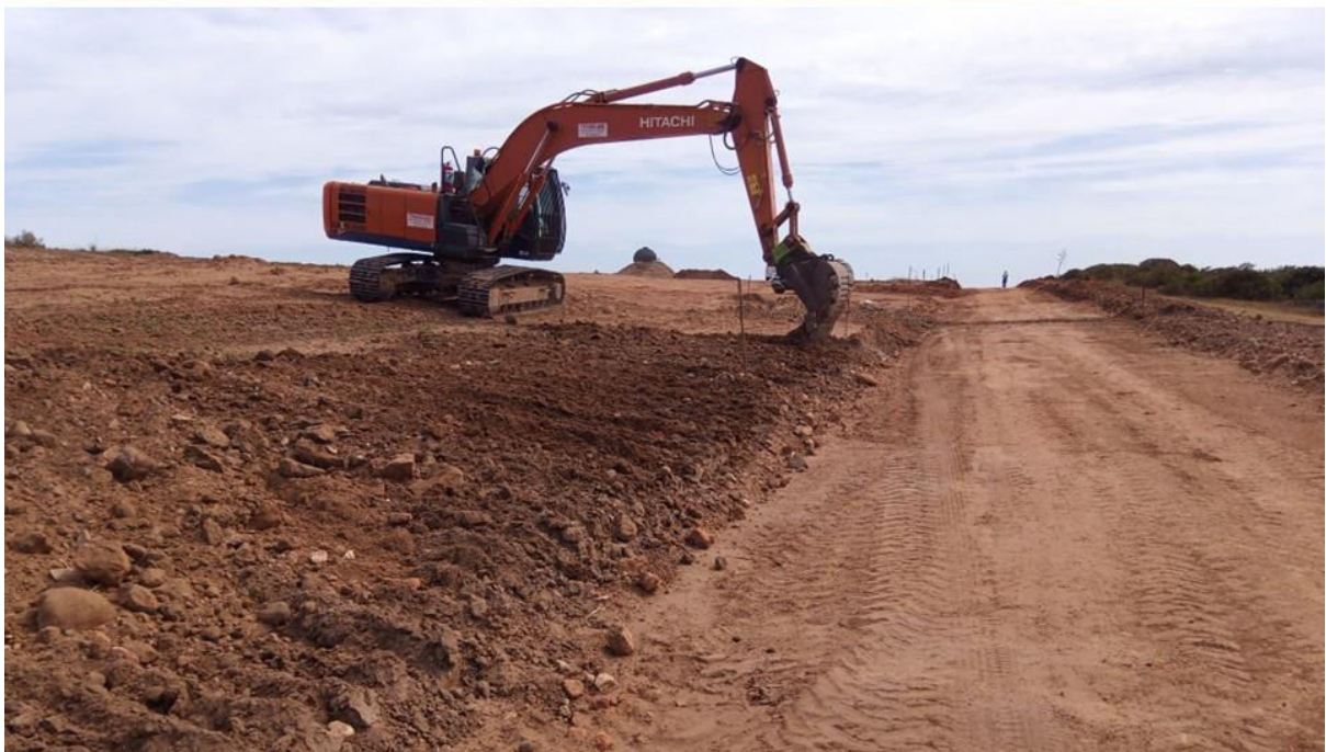
Figure 5. Hartland – Phase H2 Civils – road box cuts and verge “trimming” in progress.
