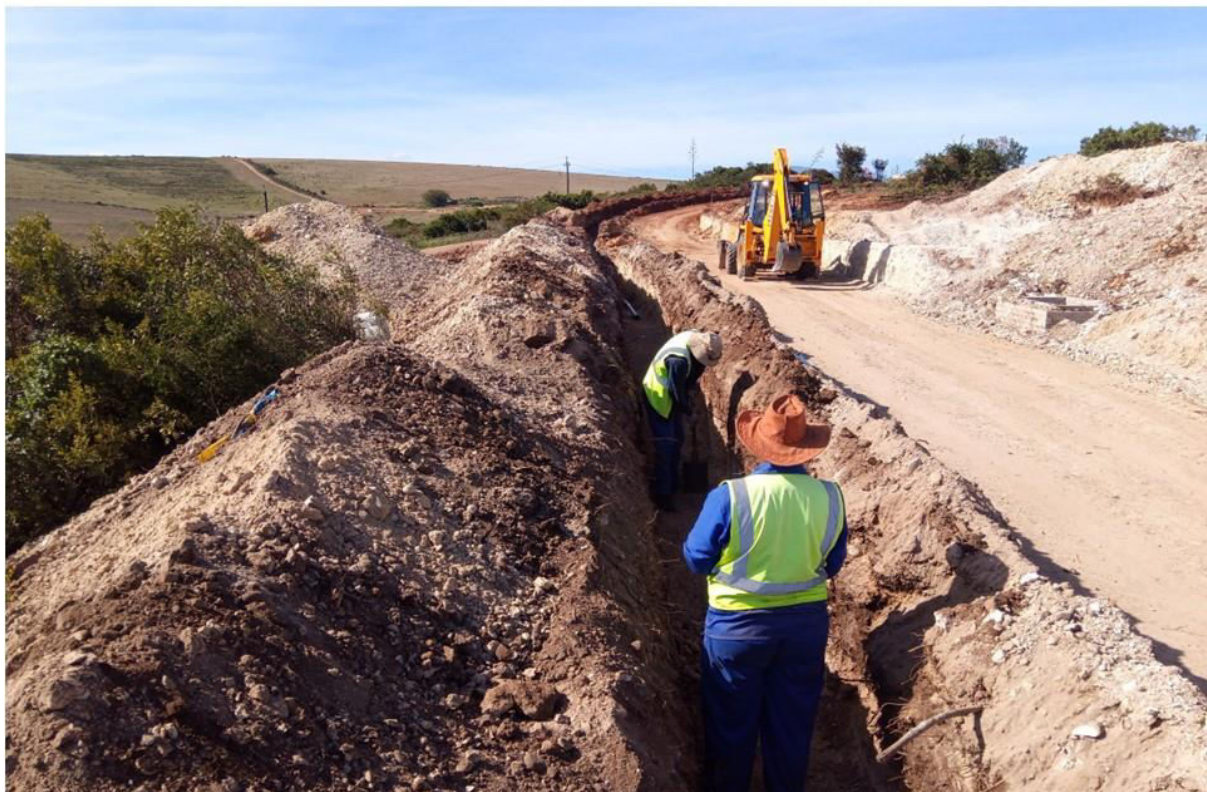
Figure 4. Hartland – Phase H2 Civils – excavation of road box cuts and trenches in progress.
