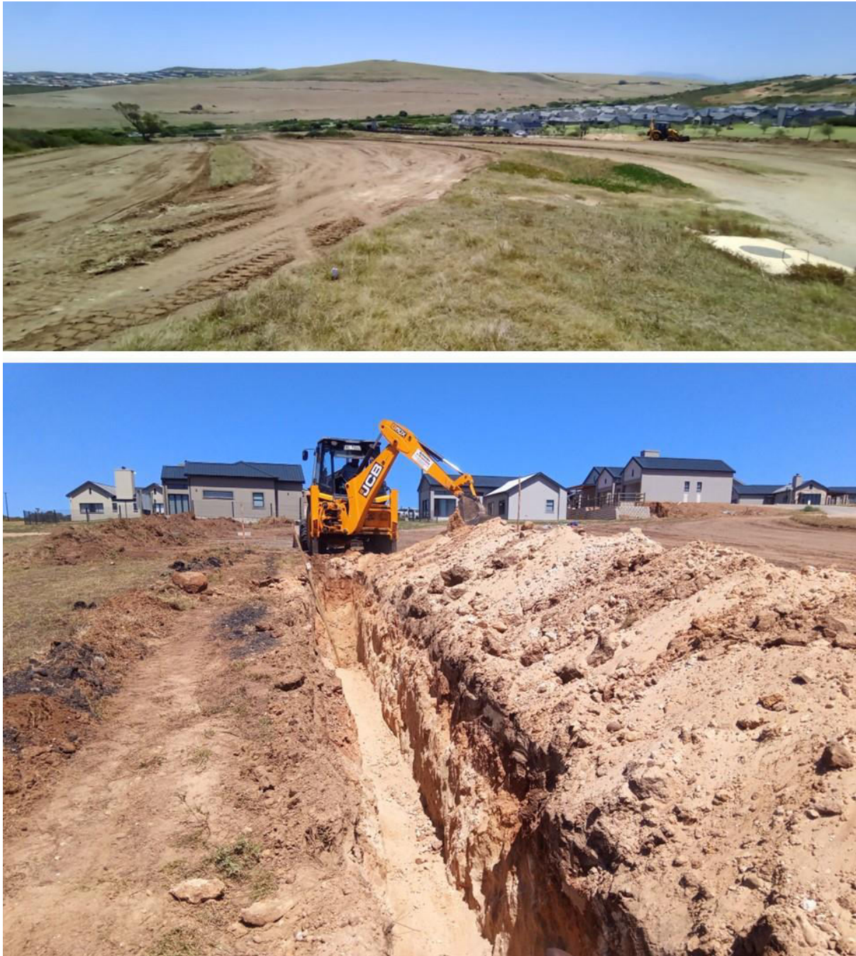
Figure 7. Hartland – Phase A – Klein Karoo Civils – vegetation stripping and excavations in progress.
