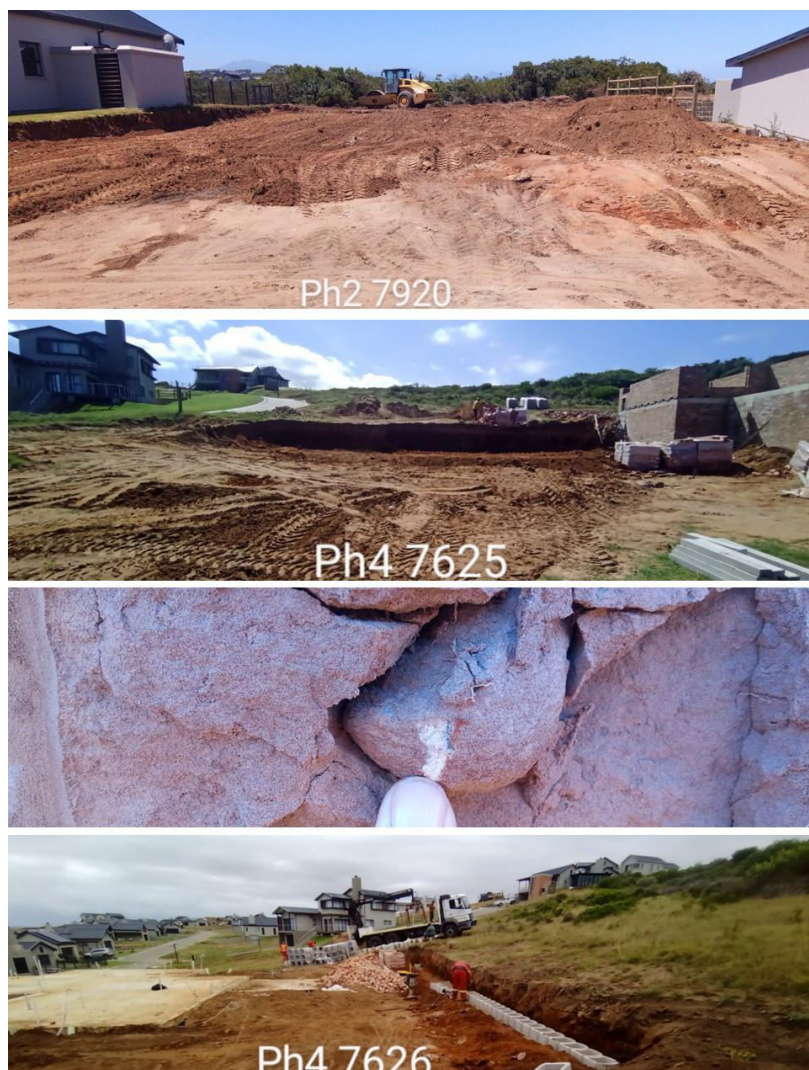
Figure 1. Hartland – Phases 2 and 4 – completed platforms and exposed manuport at Erf 7625.
