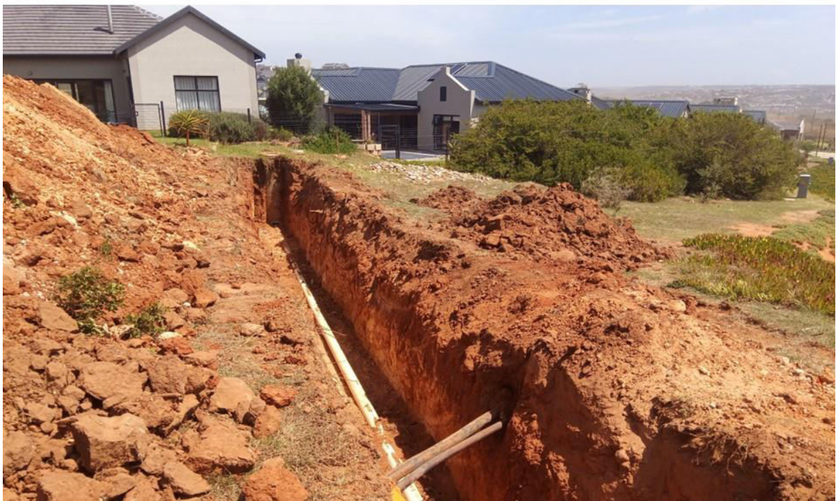
Figure 6. Hartland – Phase H2 Civils – water and sewer trenches.
