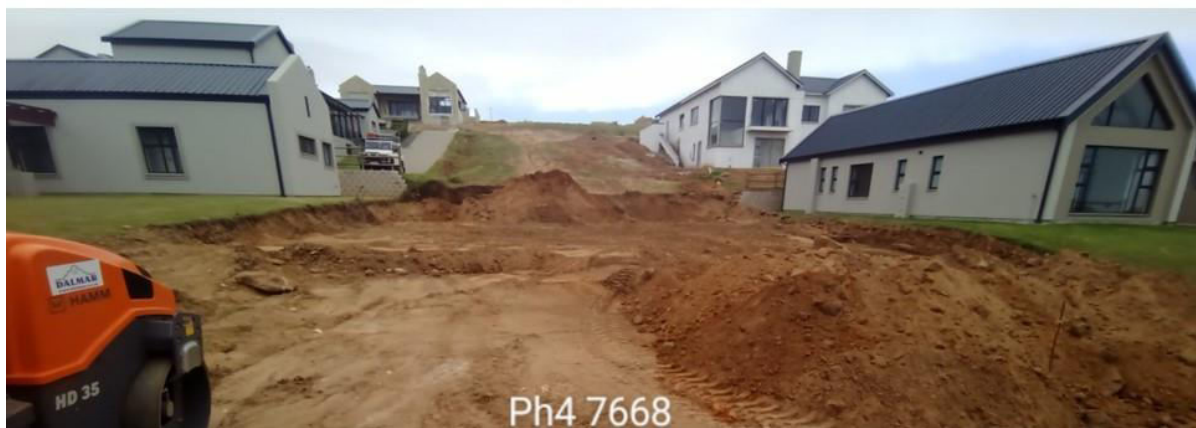
Figure 2. Hartland - Phase 4 – completed house platforms except for 7668.
