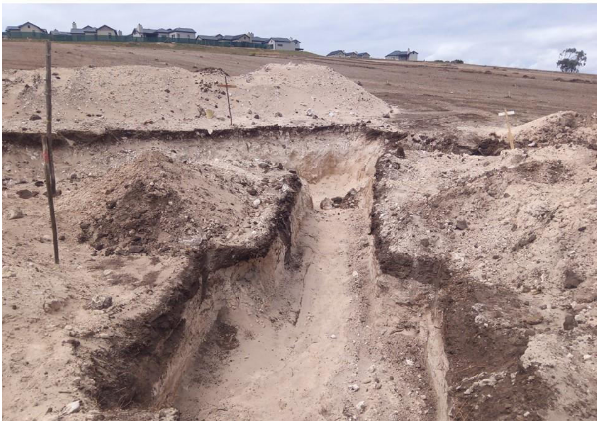
Figure 6. Hartland – Phase A – Klein Karoo Civils – storm water trench excavations in progress.
