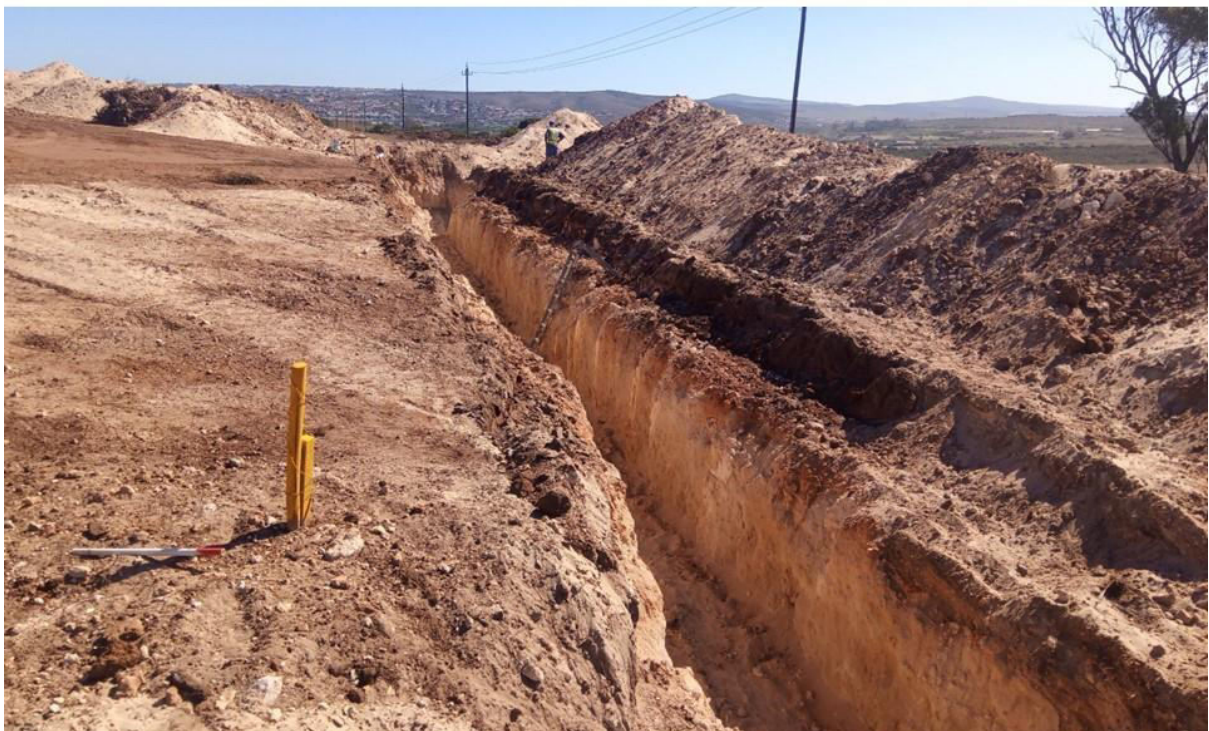
Figure 5. Hartland – Phase A – Klein Karoo Civils – storm water trench excavations in progress.
