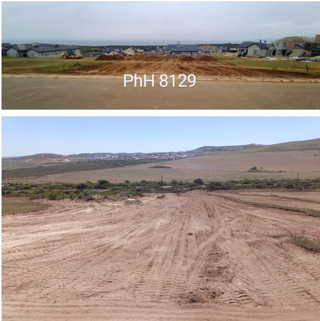
Figure 4. Hartland - Phase H, Erf 8129 cleared (top) and Phase A – Klein Karoo Civils, clearance of vegetation and topsoil (bottom).
