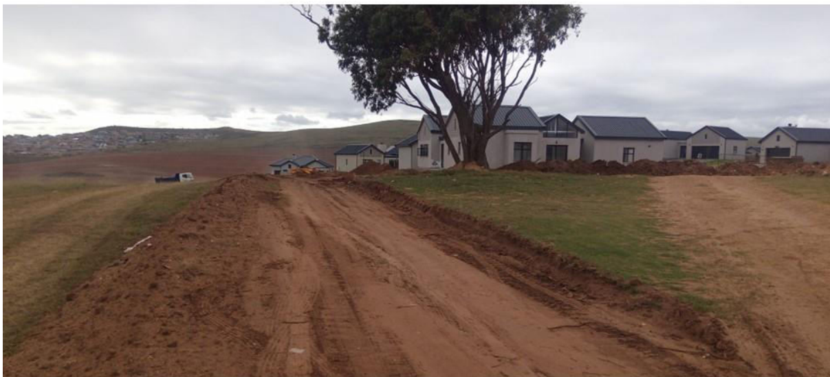
Figure 11. Hartland Development – opened / graded roads.
