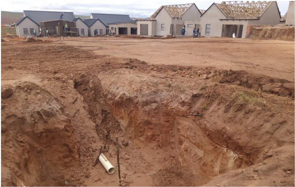
Figure 7. Hartland – HRV-Ph2 – cleared area and sewer trenching.
