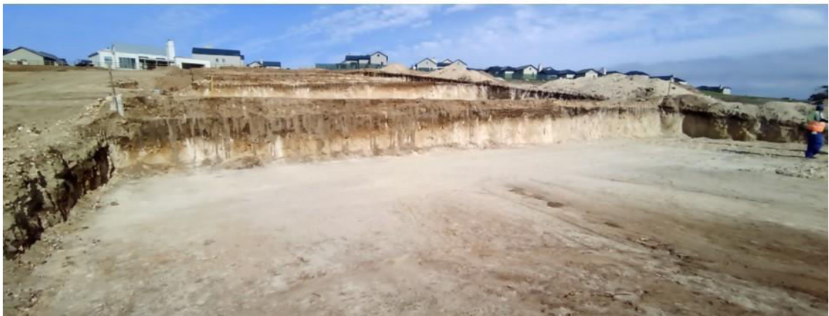
Figure 6. Hartland – Phase A – Klein Karoo Civils – platform / terracing excavations and grading in progress.
