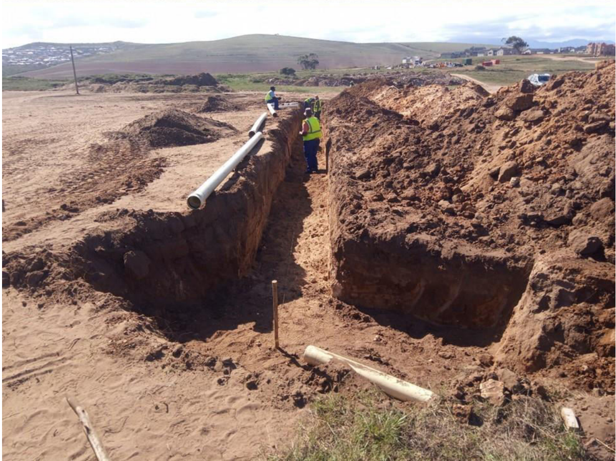
Figure 9. Hartland – HRV-Ph2 – road box cut and sewer trench excavations.
