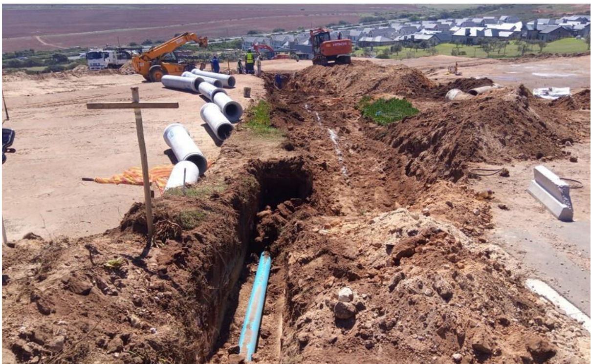
Figure 5. Hartland – Phase A – Klein Karoo Civils – water and storm water trench excavations in progress.
