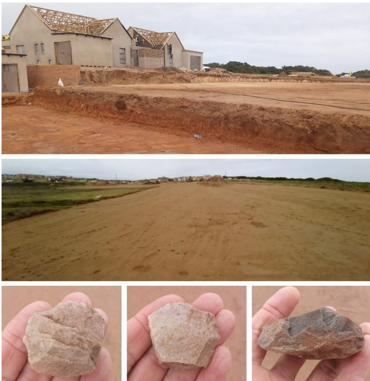
Figure 8. Hartland – HRV-Ph2 – platform excavations and cleared area with a few Stone Age pieces.
