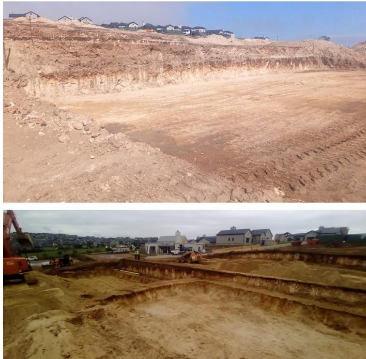
Figure 4. Hartland – Phase A – Klein Karoo Civils – terracing / platform excavations in progress.
