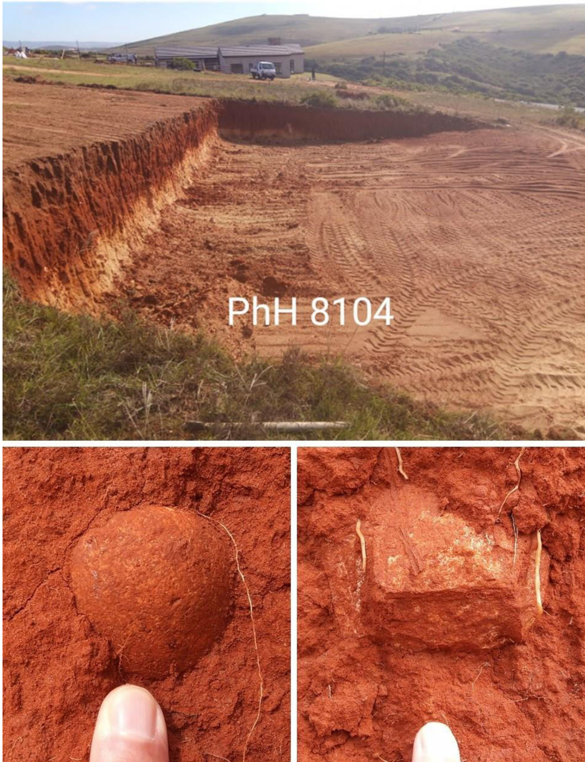
Figure 2. Hartland – Phase H – completed platform and Stone Age pieces in quartzite (middle).
