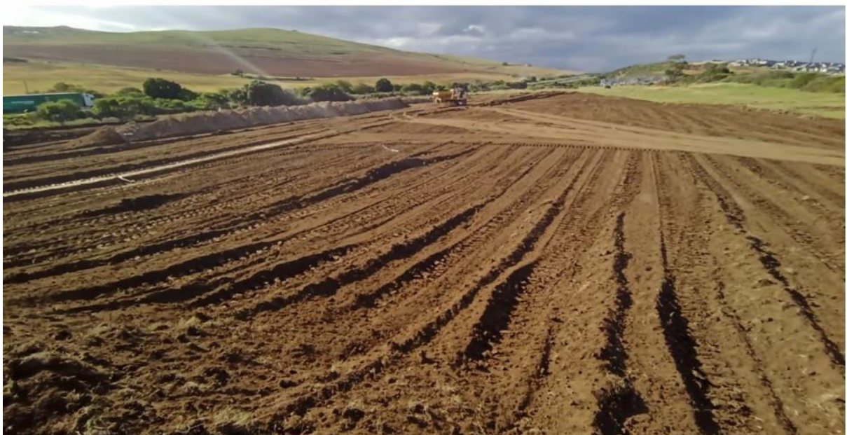
Figure 7. Hartland Development– future school sports field – earthworks in progress.
