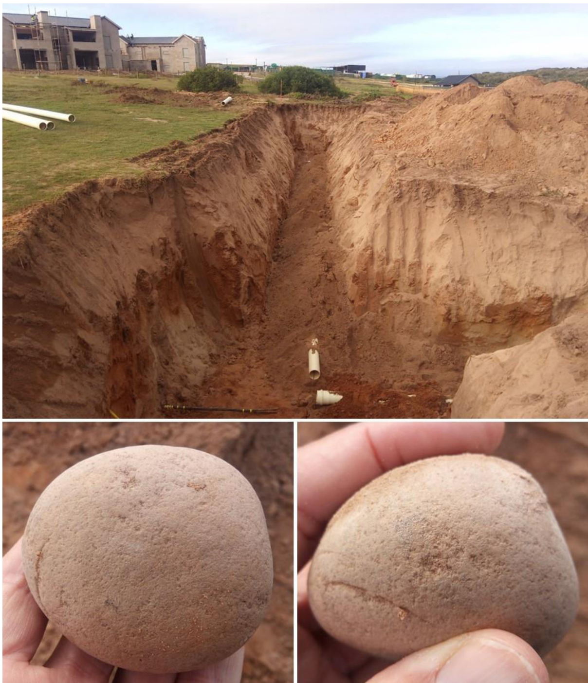
Figure 6. Hartland – HRV – sewer trench excavations and single Stone Age hammerstone in quartzite.
