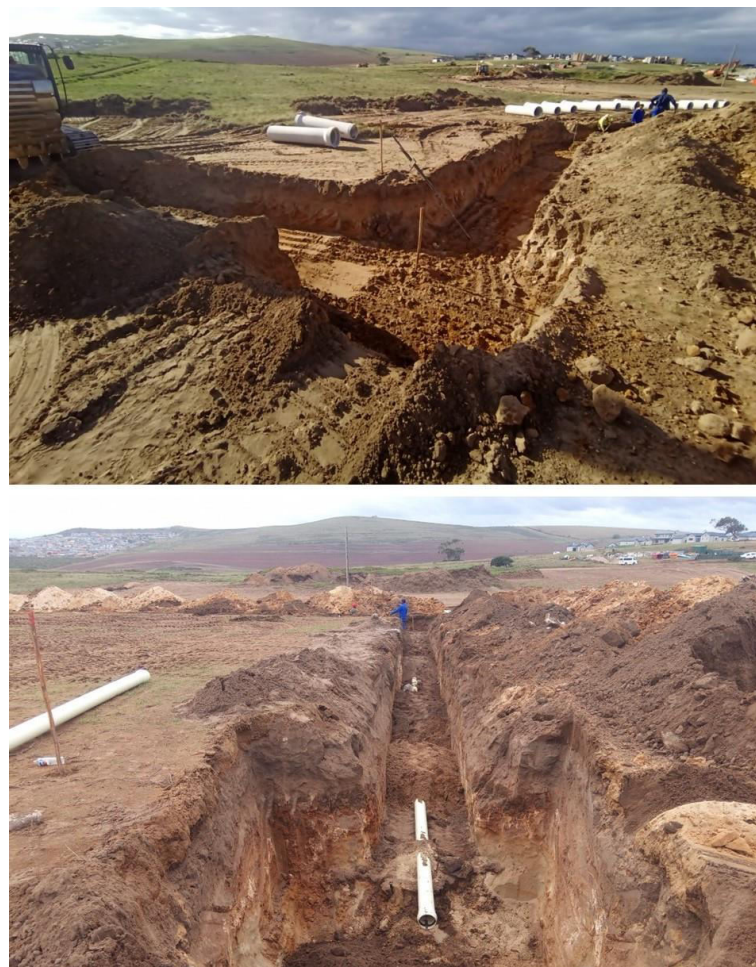
Figure 5. Hartland – HRV-Ph2 – storm water and sewer trenching.
