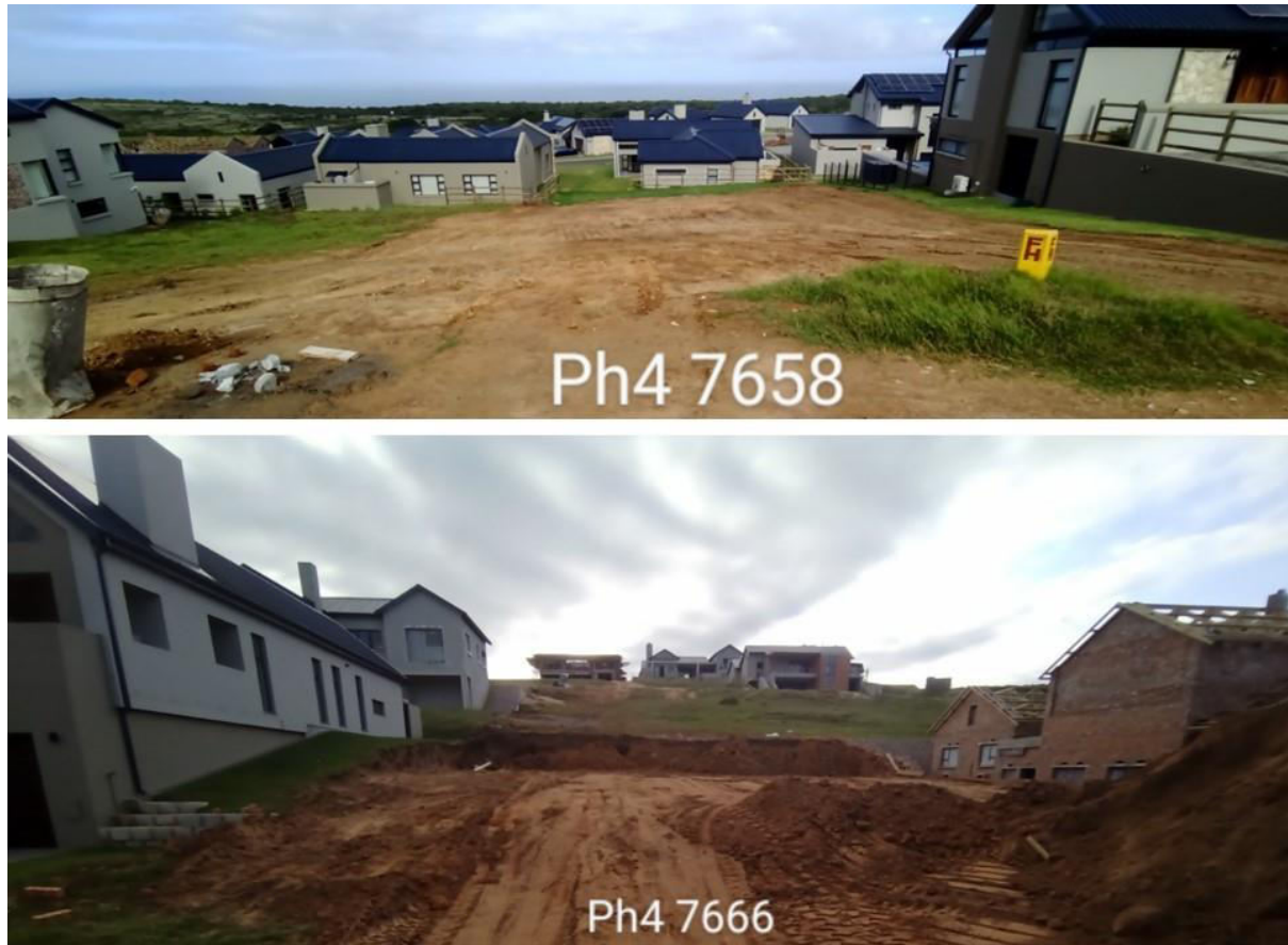
Figure 3. Hartland – Phase 4 – platforms in progress. 7659 is left of 7658 (top).
