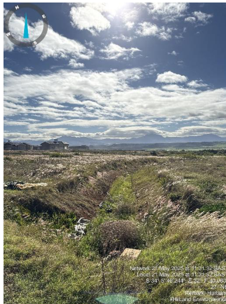
Rehabilitation progress of the stormwater outlets
