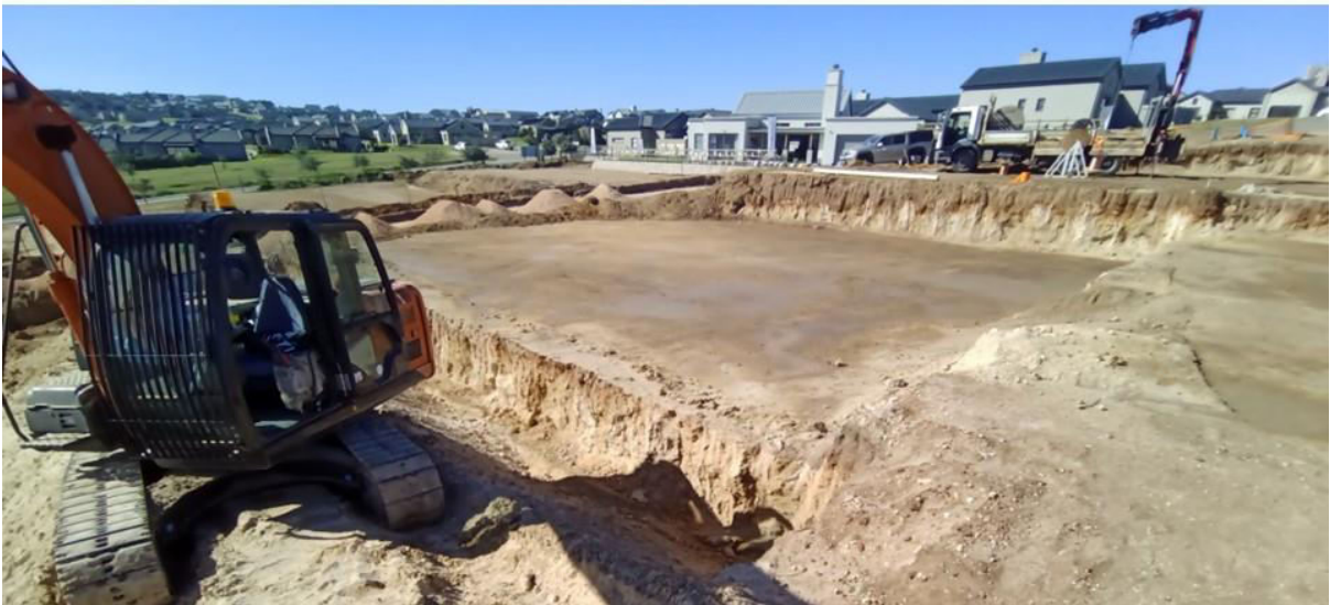
Figure 6. Hartland – Phase A – Klein Karoo Civils – road box cuts, road crossings and terrace repairs in progress.
