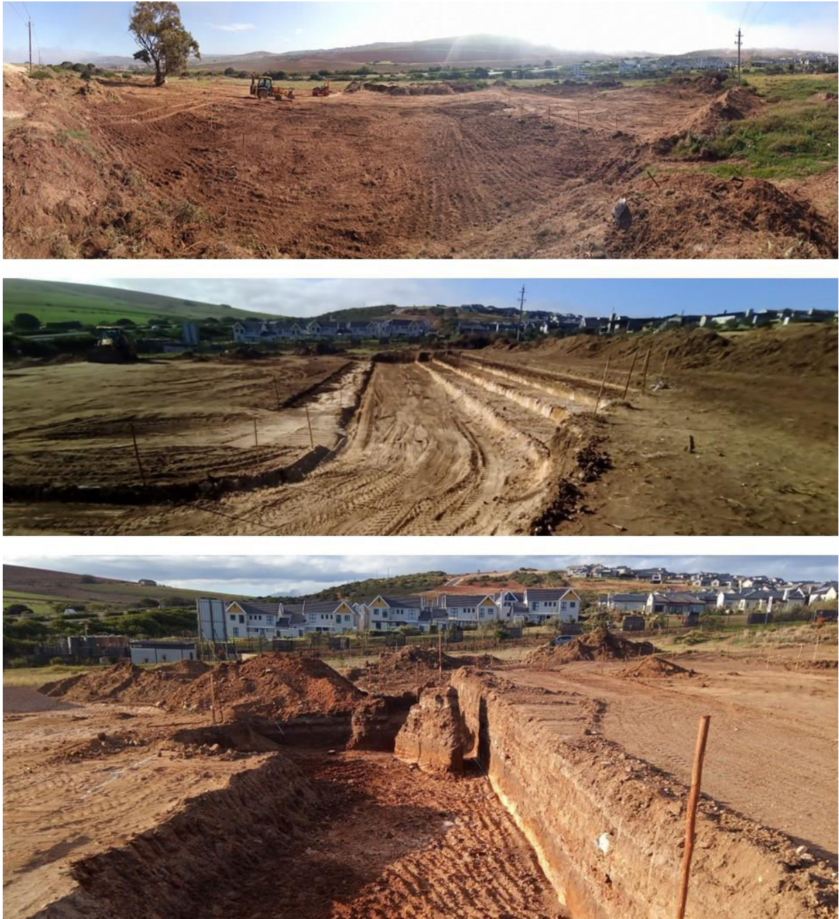
Figure 8. Hartland Development– future school site – earthworks in progress.
