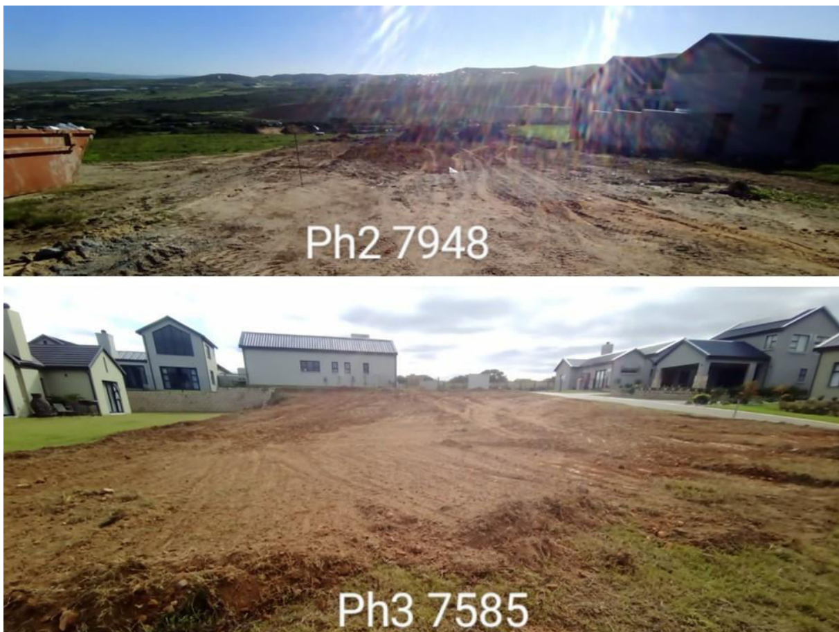
Figure 1. Hartland – Phases 2 and 3 – 7948 is cleared, filled and complete while 7585 is cleared but not excavated or complete.
