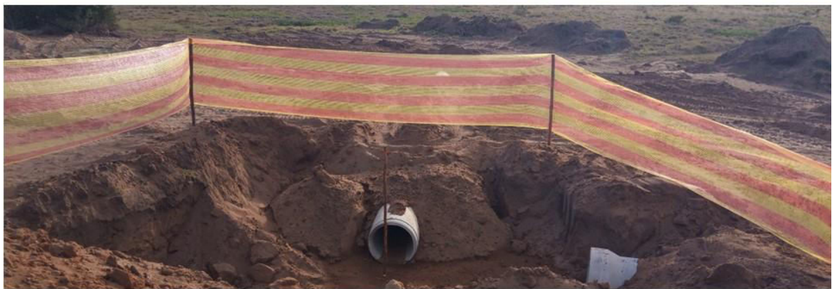
Figure 7. Hartland – HRV-Ph2 – earthworks in progress.
