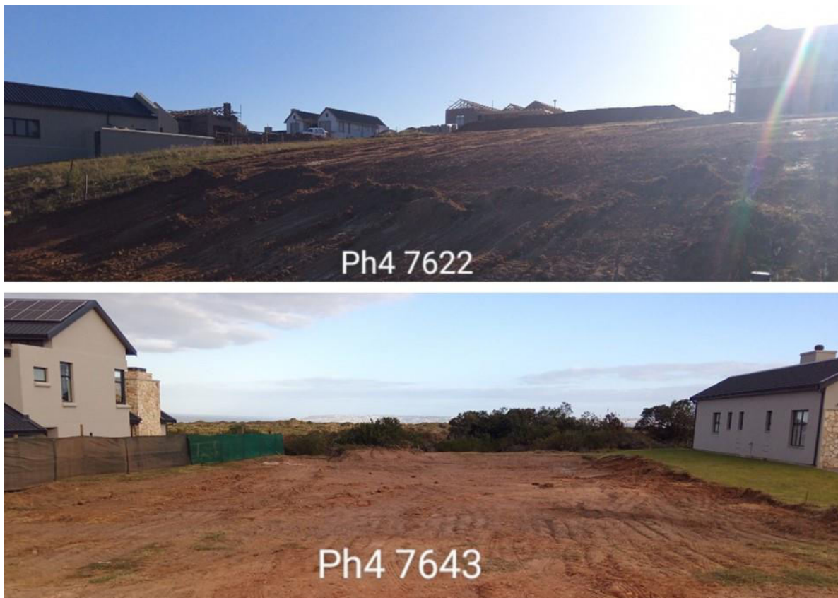
Figure 3. Hartland – Phase 4 – incomplete house platforms.
