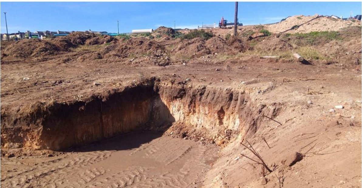
Figure 9. Hartland – School Site – works in progress.
