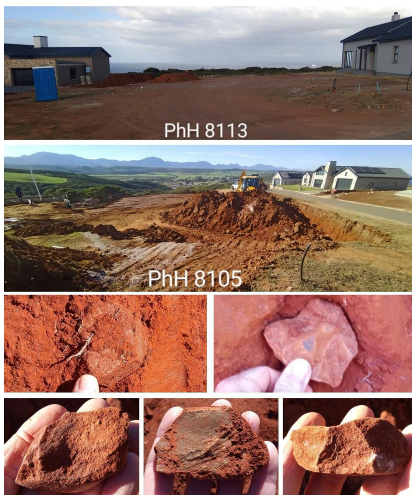
Figure 1. Hartland – Phase H – works in progress and Stone Age pieces recorded at 8105.
