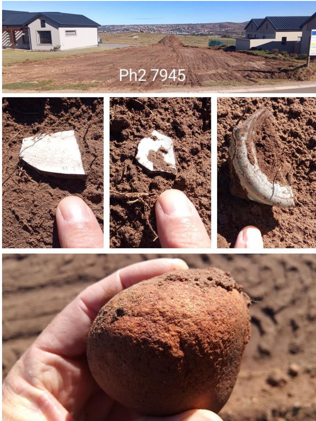
Figure 2. Hartland – Phase 2 – works in progress and modern / colonial period debris and a Stone Age hammerstone recorded at 7945.
