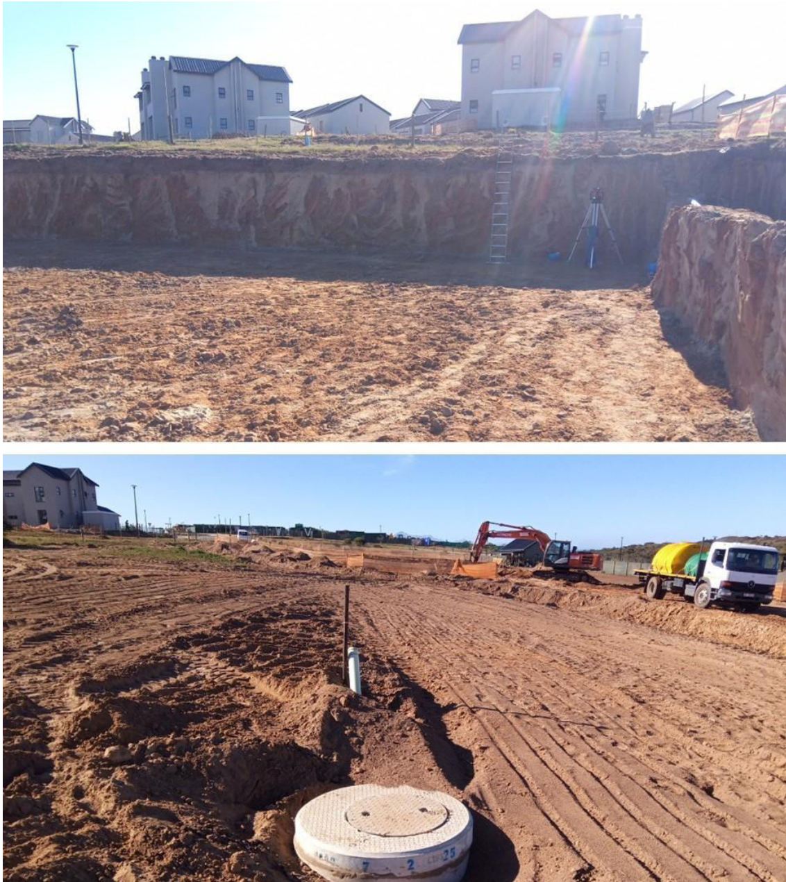
Figure 5. Hartland Retirement Village – works in progress.
