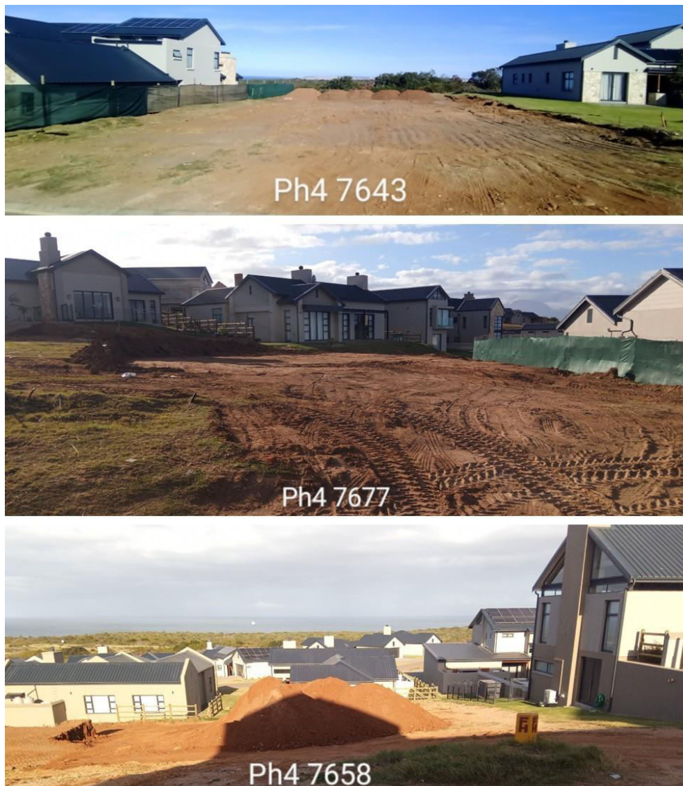
Figure 3. Hartland – Phase 4 – works in progress.
