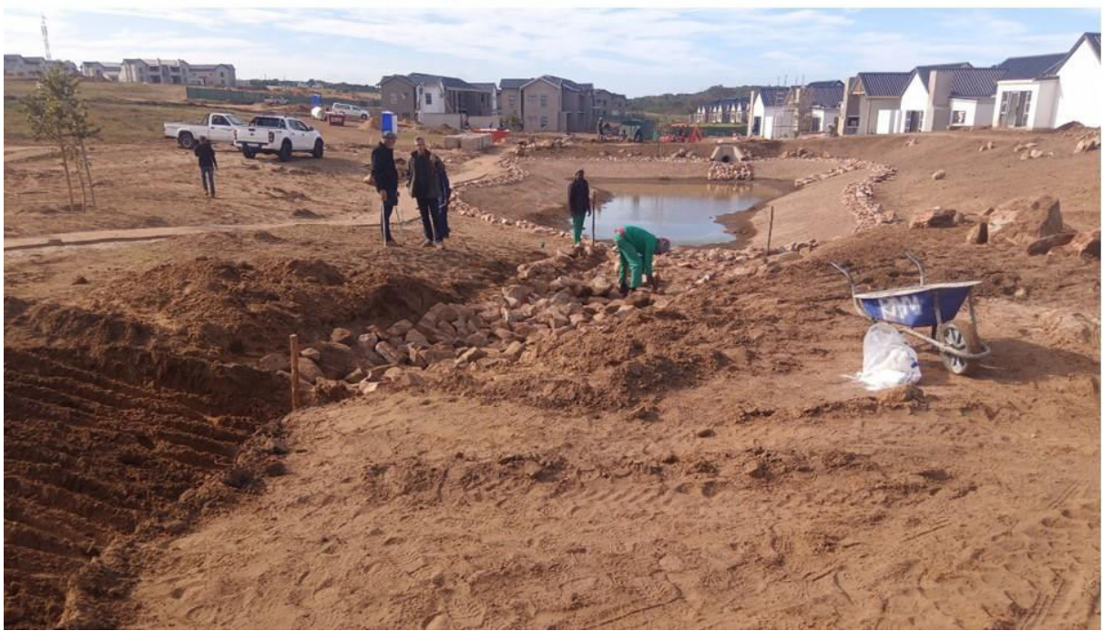
Figure 6. Hartland Retirement Village Phase 2 – works in progress.
