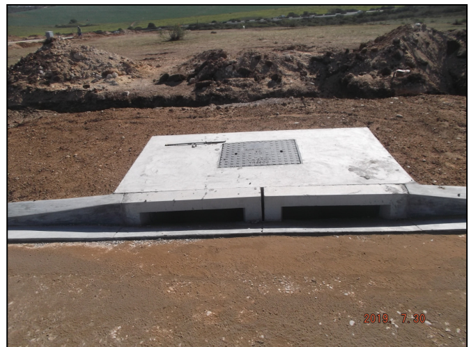
Image 4: Installed stormwater inlet within the development site
