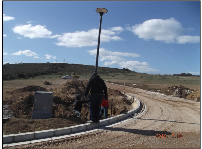
Image 6: Installation of new lamp posts within the development site
