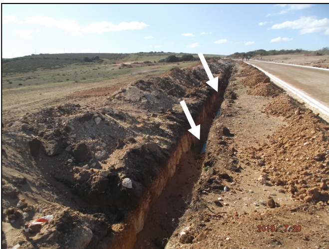
Image 3: Arrows indicating installed water pipes within the excavated trenches
