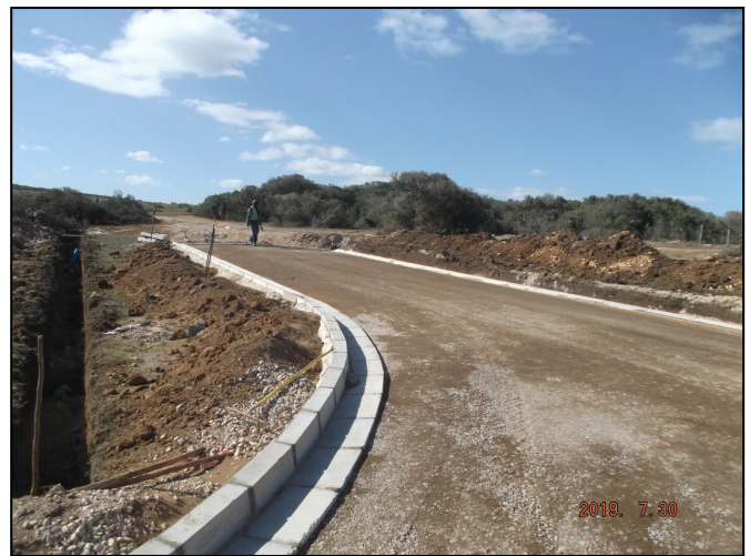
Images 1 & 2: Road network and installed kerbing within the development site
