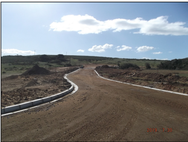
Images 1 & 2: Road network and installed kerbing within the development site
