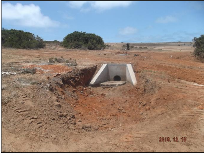
Image 5: New installed storm water culvert
