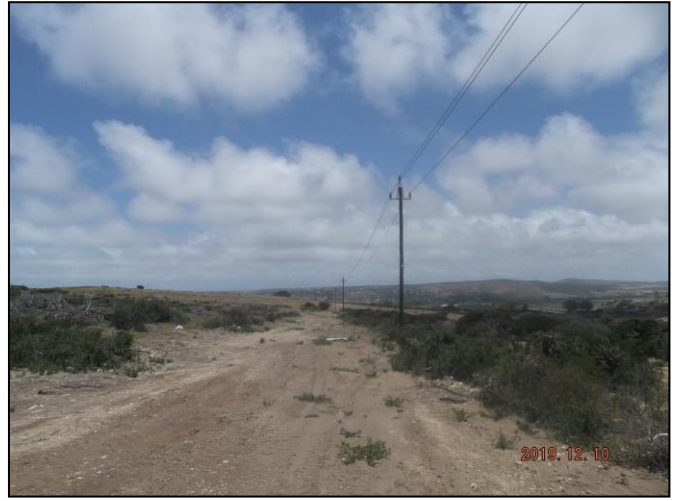
Image 6: New installed powerlines within the development site
