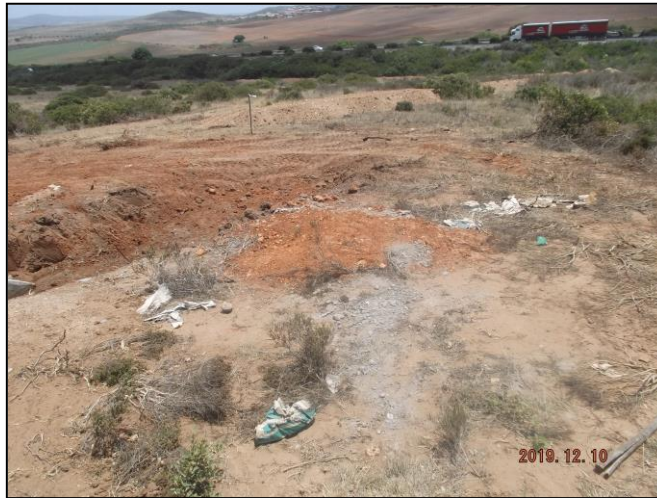
Image 15: The concrete rubble must be removed from the ground and disposed of at an appropriate registered facility
