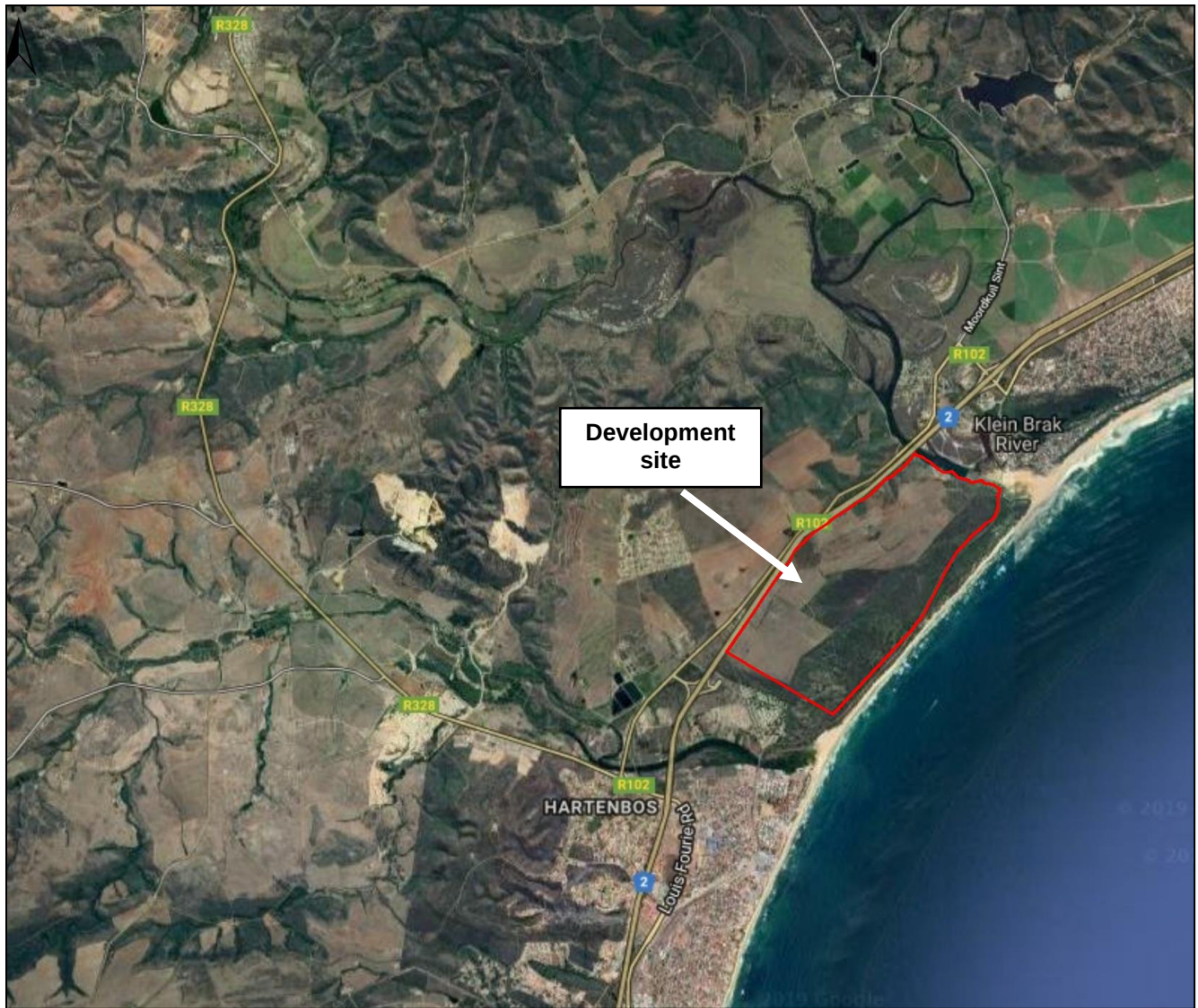
Figure 1: Google Earth Image depicting the development site
