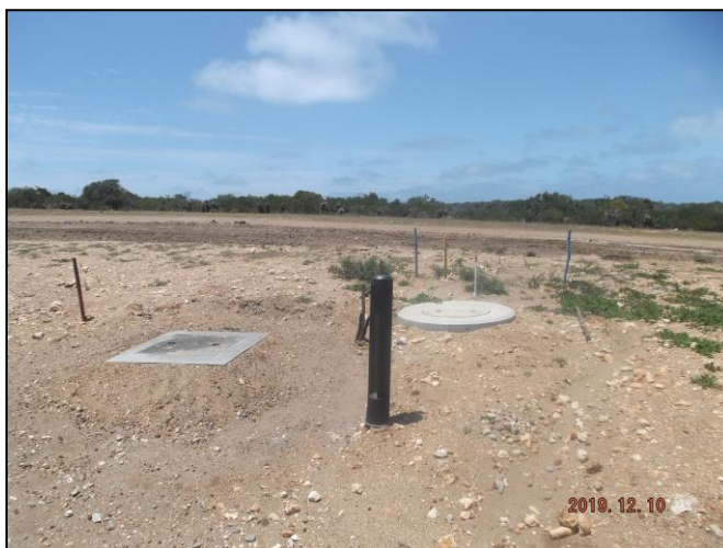
Image 4: New installed sewerage cesspit and valve chamber
