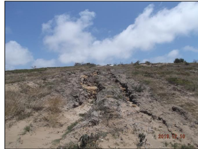
Image 16: The erosion gullies must be rehabilitated on site and further erosion must be mitigated
