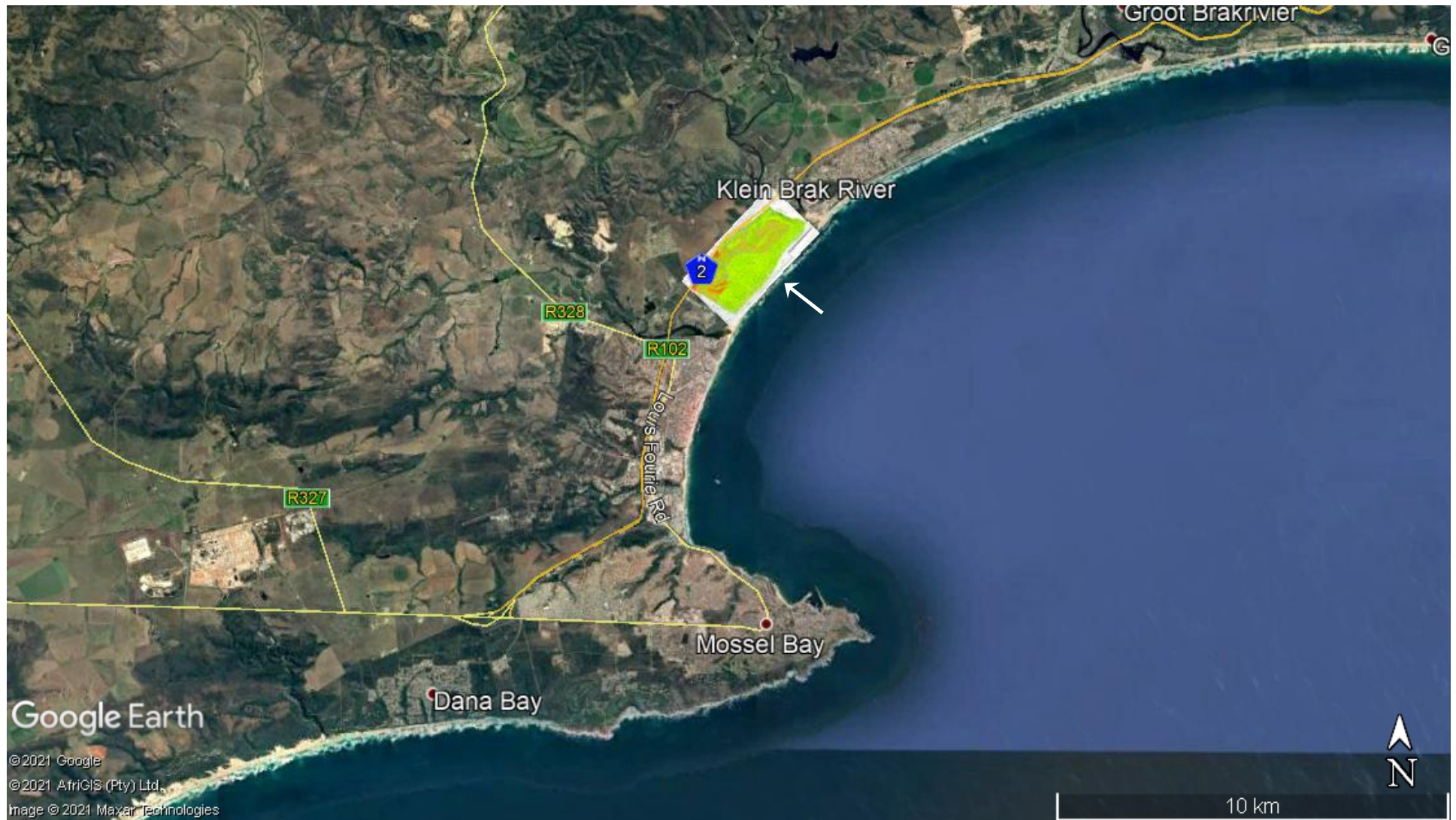
Figure 1. White arrow shows the location and extent of the Hartland Development relative to Mossel Bay and Klein Brak River in the Garden Route of the Western Cape Province. Courtesy of Dalmar Beleggings and Google Earth 2021 .
