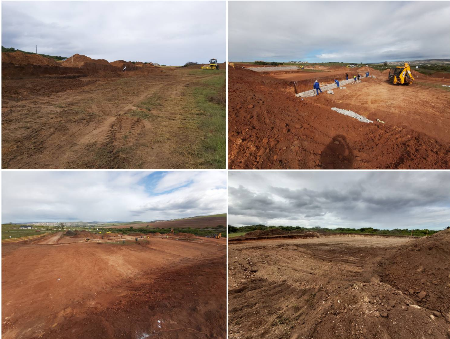
Plate 3. Excavations and earthworks in the north-eastern portion of the Hartland Villas phase, except for the bottom right image which shows a cleared plot at the north-eastern extent of Phase 1.
