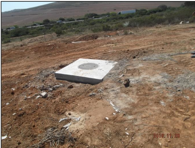
Image 12: The concrete powder and pieces must be removed from the ground and disposed of at an appropriate registered facility
