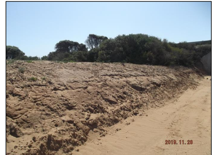
Image 14: The embankment on site must be revegetated with indigenous vegetation
