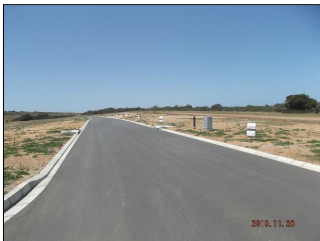
Image 2: Roads and kerbing have been constructed within the development site
