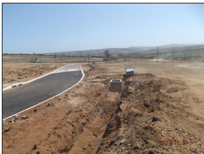
Image 6: Construction of valve chambers along the pipeline route within the development site
