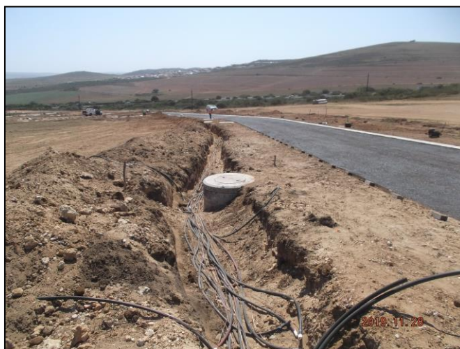
Images 3 & 4: Installation of electricity cables within the trenches
