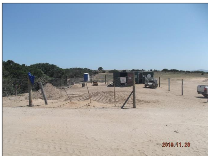
Image 1: The site camp has been fenced off along its perimeter
