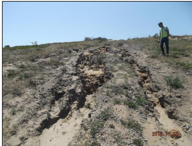
Image 13: The erosion gullies on site must be rehabilitated and further erosion must be mitigated
