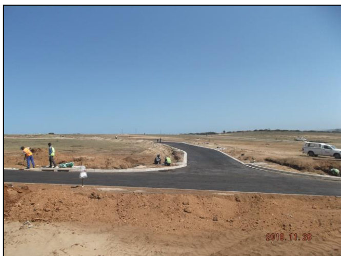
Images 5: Installed road network within the development site
