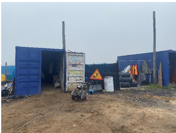
Concrete cutting saw stored at the site camp.
