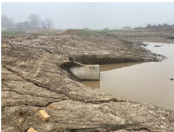
Stormwater pipeline installed in the large pond to direct water toward the main outlet along the Berg River.
