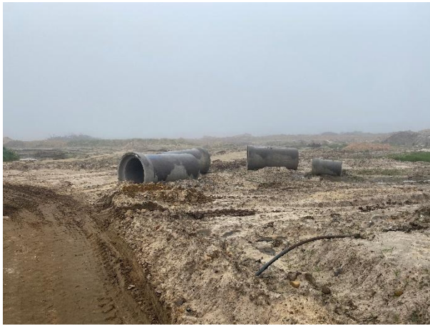
1.1m stormwater pipeline material adjacent to the large stormwater pond to be installed.
