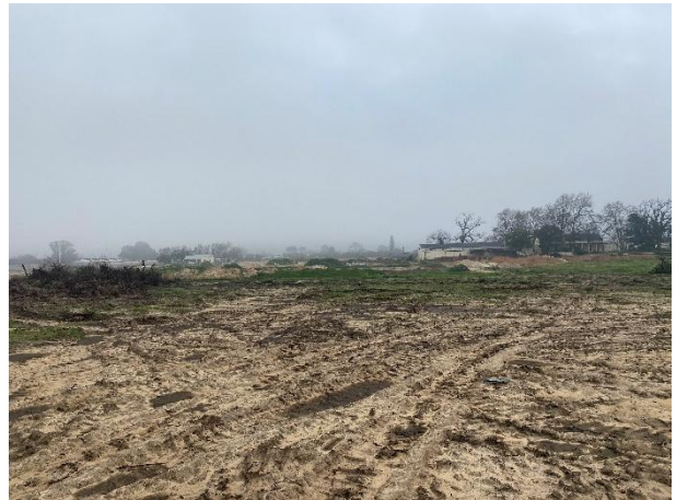
View of the existing Firwoods Homestead and stockpile laydown area towards the southwest.
