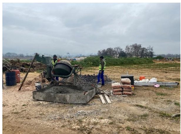
Asphalt mixing with a mortar board in place.
