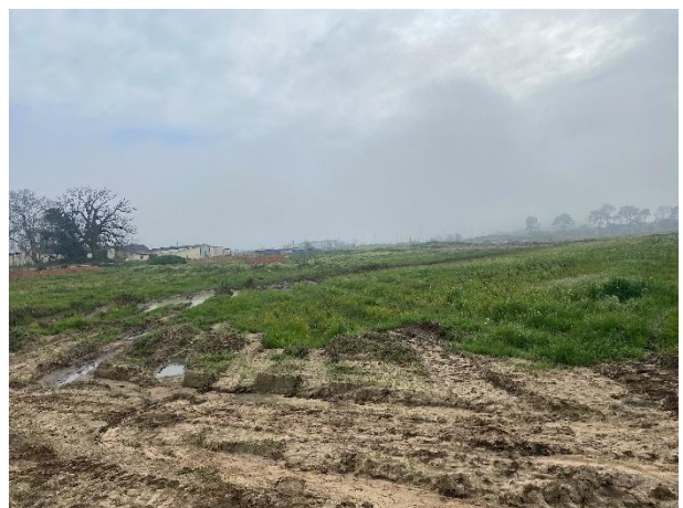
View of the site towards the site camp looking northwest.
