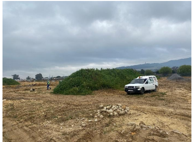
Revegetated topsoil stockpiles adjacent to the site camp.
