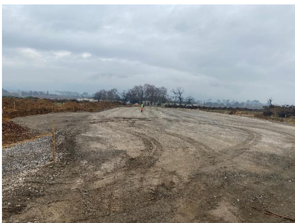
Internal road surfaces being chipped and sprayed. Entrance to the site towards the Firwoods Homestead.
