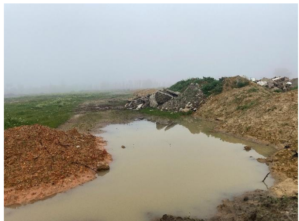
Demolished buildings crushed on-site for reuse as G7 material in road construction.
