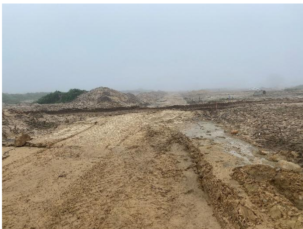
Road surfaces being prepared for asphalt.
