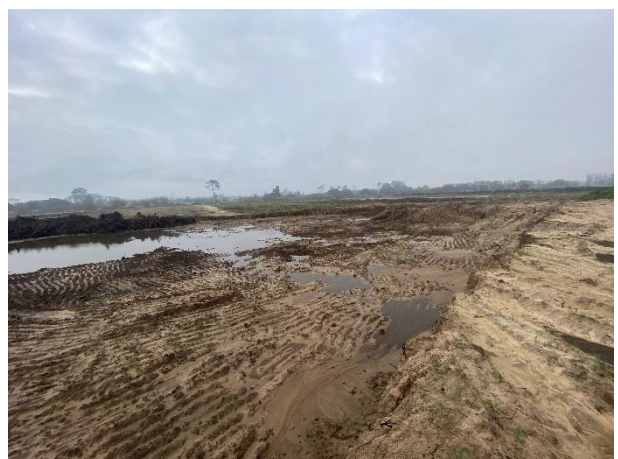
Cleared area adjacent to the Homestead and stormwater pond wet due to the recent rain.
