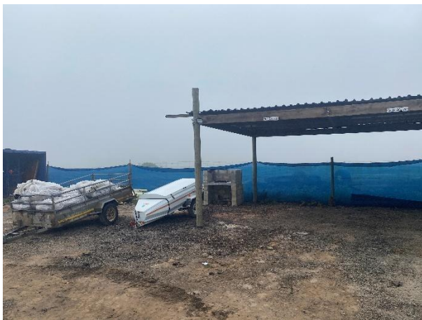
Site camp area with storage trailer, construction materials, and temporary shelter structure.
