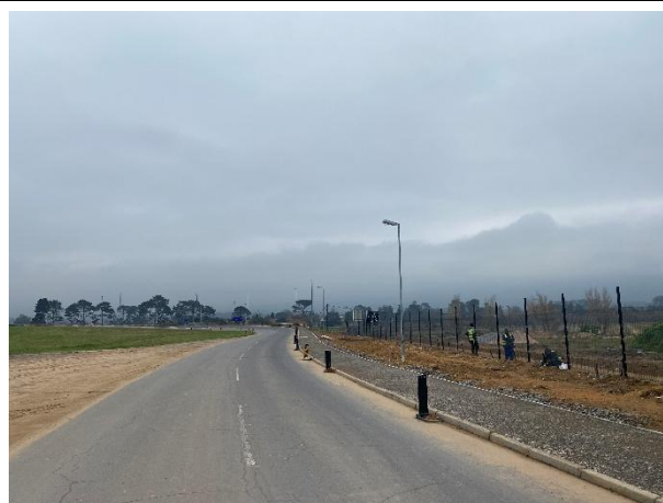
ClearVu boundary fence being installed along the western boundary of the site.
