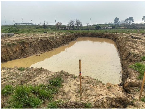
Smaller stormwater pond towards the north.
