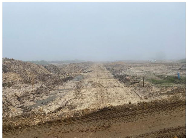
Road surfaces being prepared for asphalt
