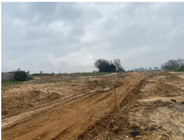
Roads being excavated and cut south of the foreman's house.
