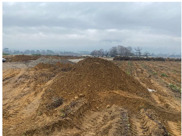
Stockpile area towards the southwest where roads are being excavated.
