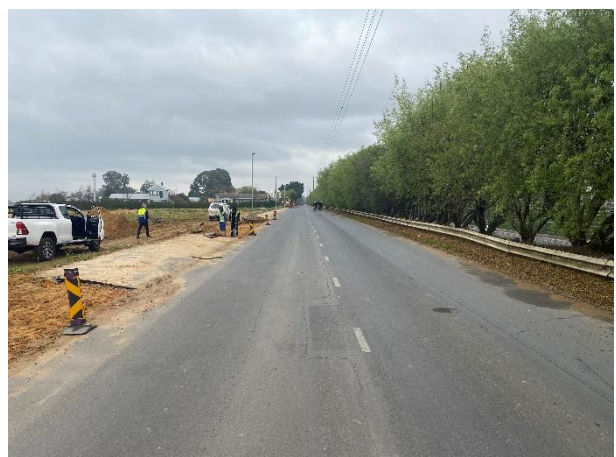
Fibre installations along New Eskdale Street.
