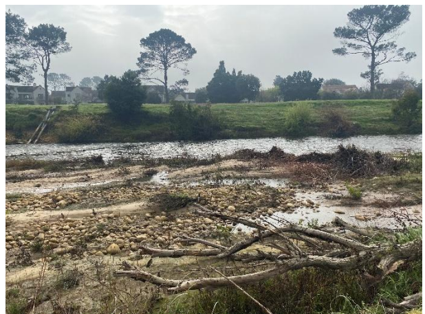
Condition of the Berg Riverbank north of the development site.
