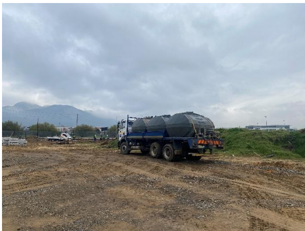
Water truck available for dust fallout on site.
