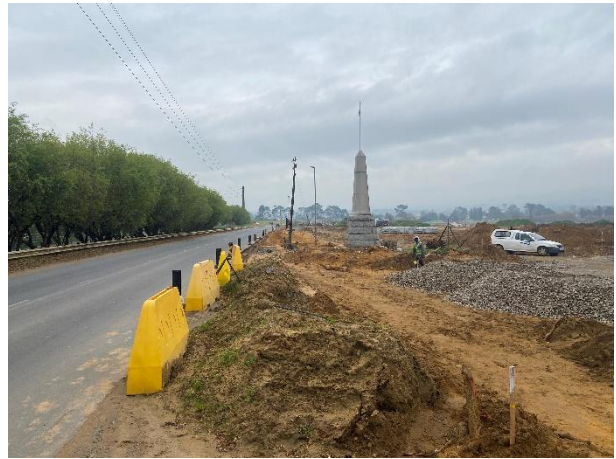
Condition of New Eskdale Street towards the North. Civil services being installed along the road.
