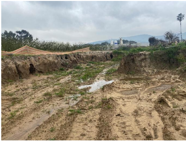
Excavated stormwater channel towards the southwest.
