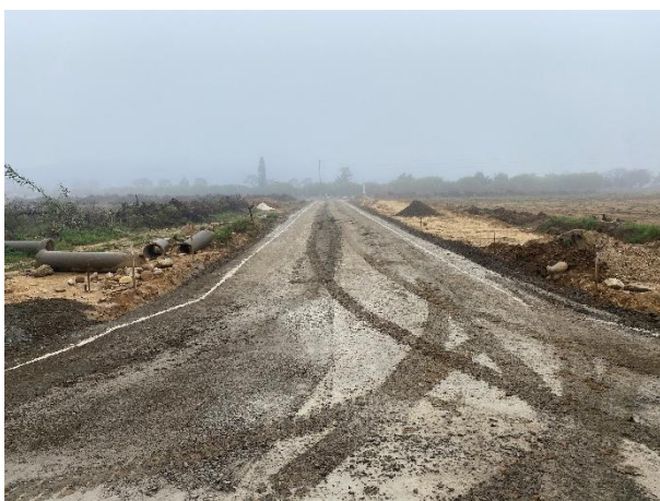
Access road off New Eskdale Street chipped and sprayed.
