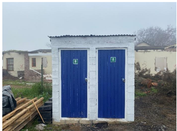
Toilets in place adjacent to the site camp.
