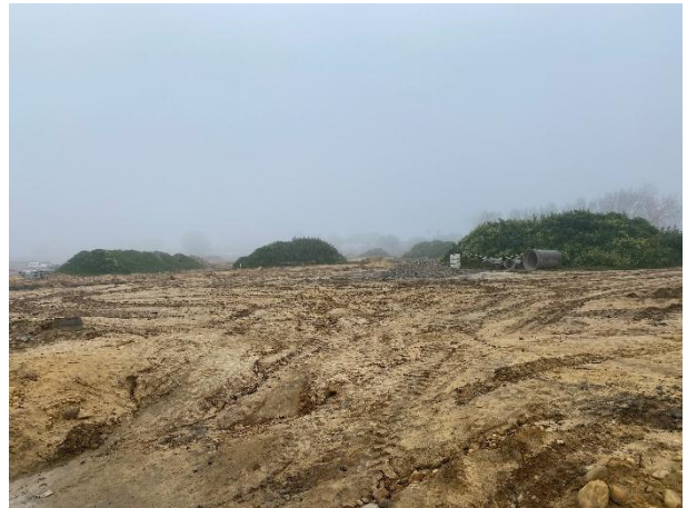
Topsoil stockpiles towards the southwest.
