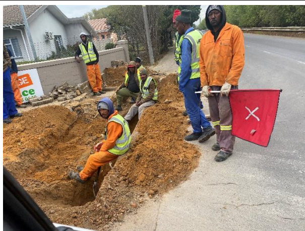
Fibre being installed along New Eskdale Street.
