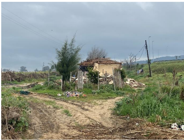
Workers' house still to be demolished and crushed.
