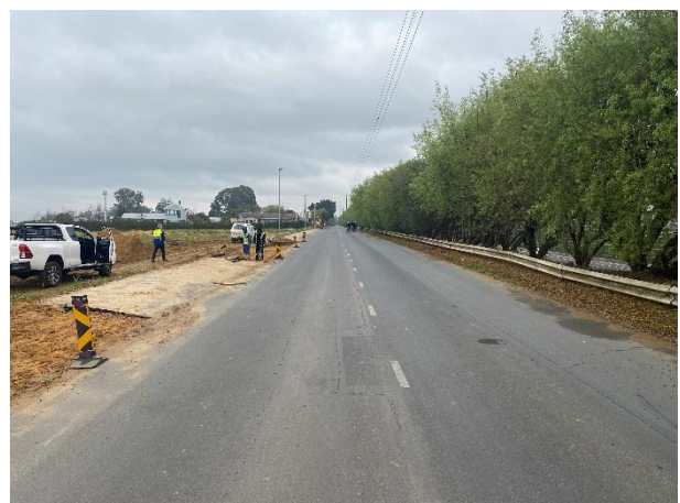
Fibre installations along New Eskdale Street.
