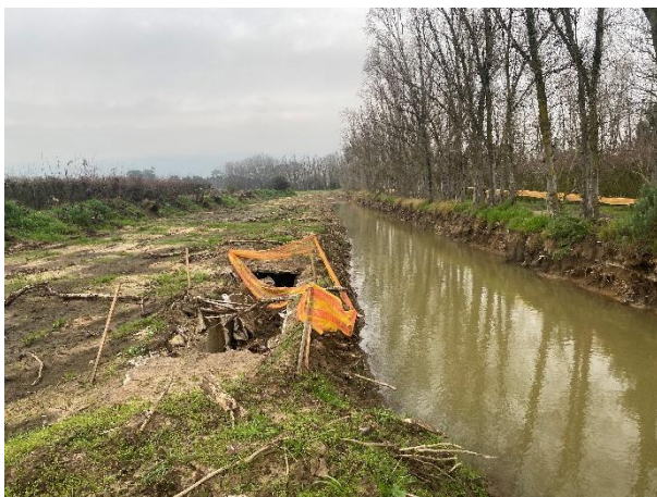
Stormwater channel being upgraded towards the southwest.
