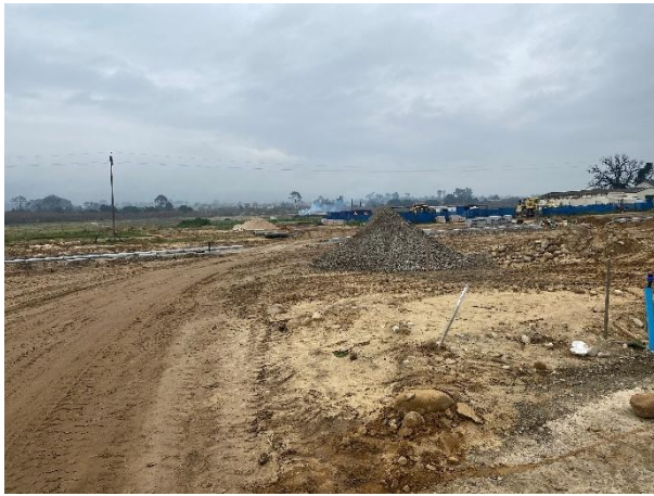
Internal road network being cut, shaped, and prepared.
