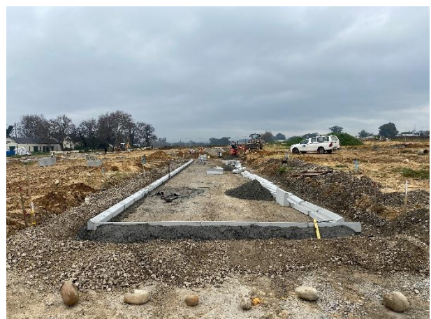
Civil services, kerbs, and road surface being prepared west of the site camp at the entrance to the site.
