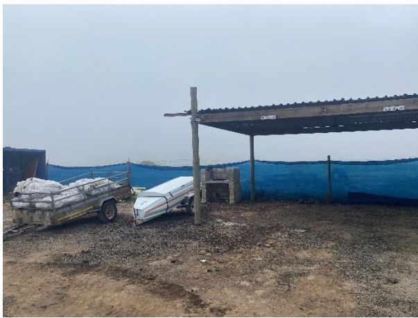
Site camp area with storage trailer, construction materials, and temporary shelter structure.
