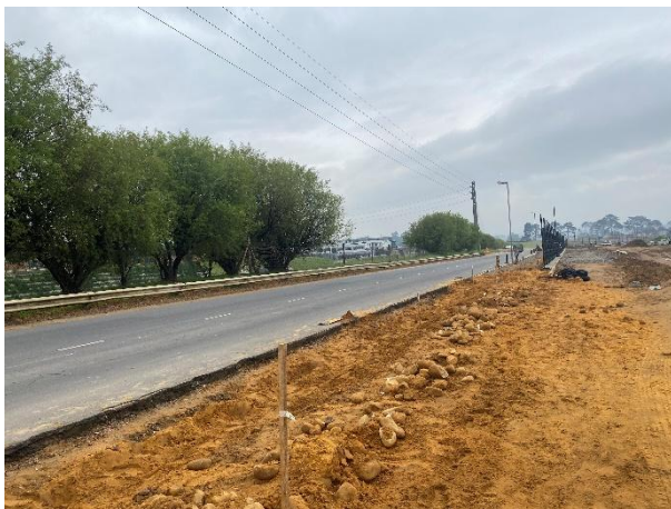
Condition of New Eskdale Street towards the southwest, where the ClearVu boundary fence is being installed.
