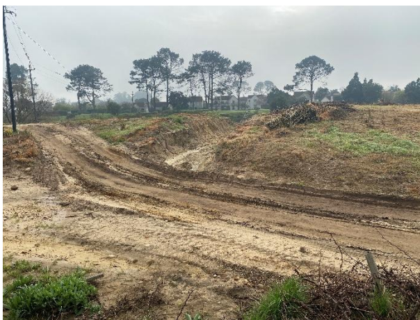
Excavated stormwater outlet channel north towards the Berg River.
