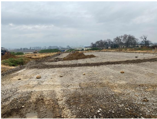
Civil services, kerbs, and road surface being prepared west of the site camp at the entrance to the site.
