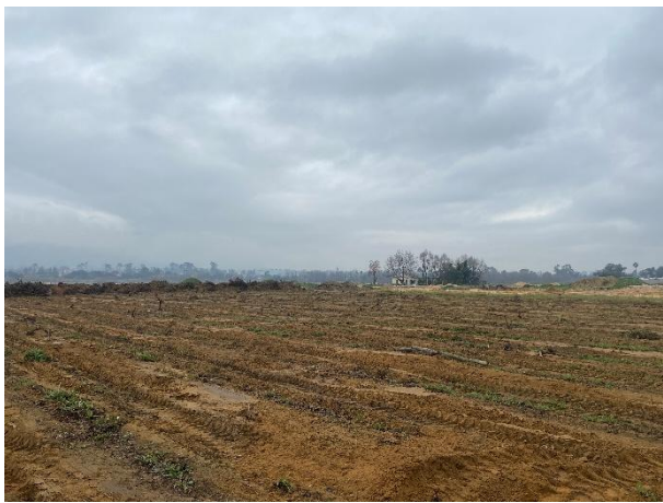
Cleared southern area where unproductive vineyards were removed, to be reinstated with new vines.
