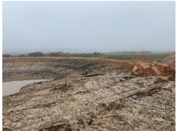
Large stormwater pond located east of the existing Firwoods Homestead.
