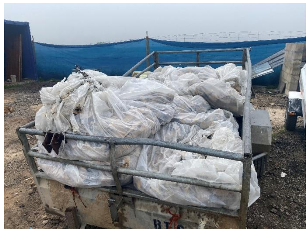
Construction waste stored in a trailer at the site camp, secured in plastic sheeting to prevent windblown litter.
