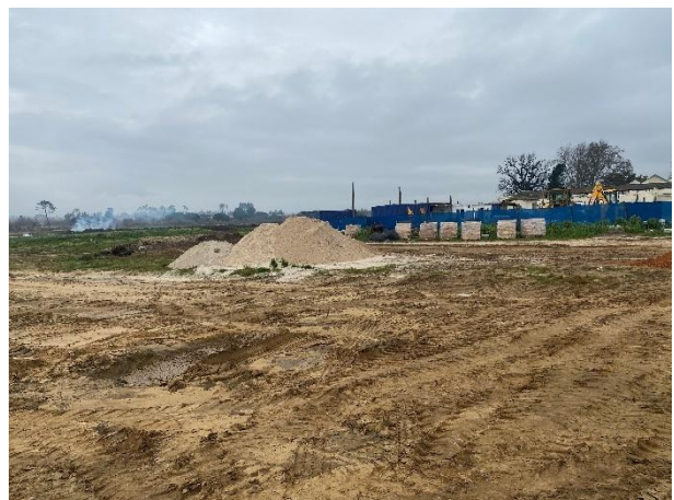
Stockpile material adjacent to the site camp towards the southwest.
