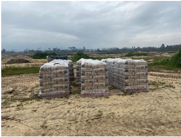
Ready mix cement for kerb installations.
