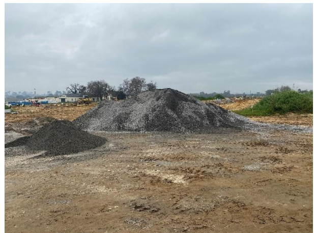
Asphalt material stockpiles adjacent to the site camp where roads are being chipped and sprayed.
