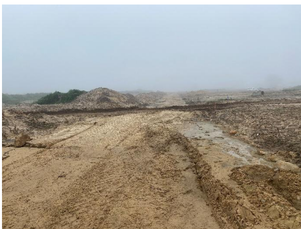
Road surfaces being prepared for asphalt.
