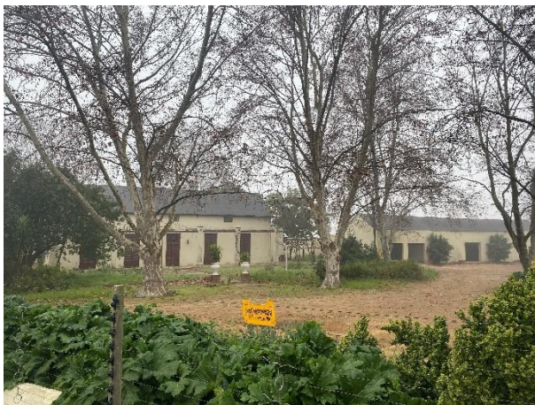
Workers' homesteads to be demolished and crushed; Firwoods Homestead to be retained.
