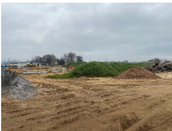
Topsoil and material stockpiles separated adjacent to the site camp.
