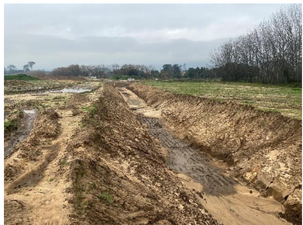
Stormwater channel being upgraded towards the southwest.
