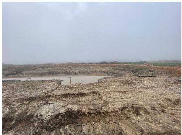
Condition of the large stormwater pond located east of the existing Firwoods Homestead.
