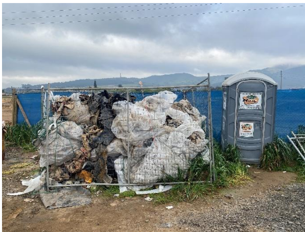
Wire structure available within the site camp for waste disposal.
