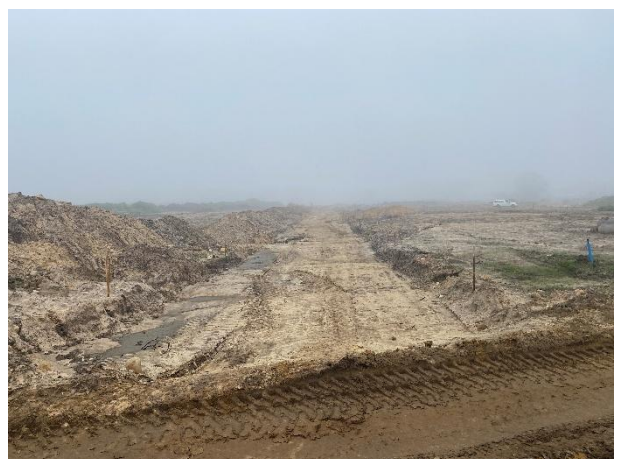
Road surfaces being prepared for asphalt
