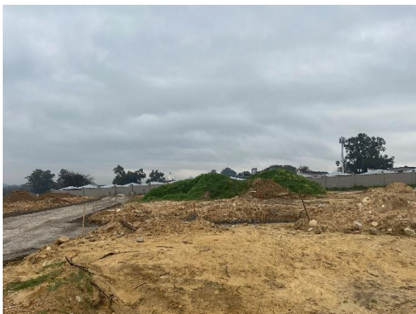
Topsoil stockpiles towards the southwest, adjacent to the foreman's house.
