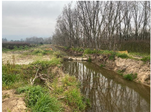
Collapsed stormwater channel with a new, formalised channel under construction.
