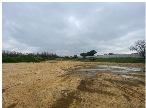
Stockpile area southwest of the site. Topsoil stockpiles have been revegetated.
