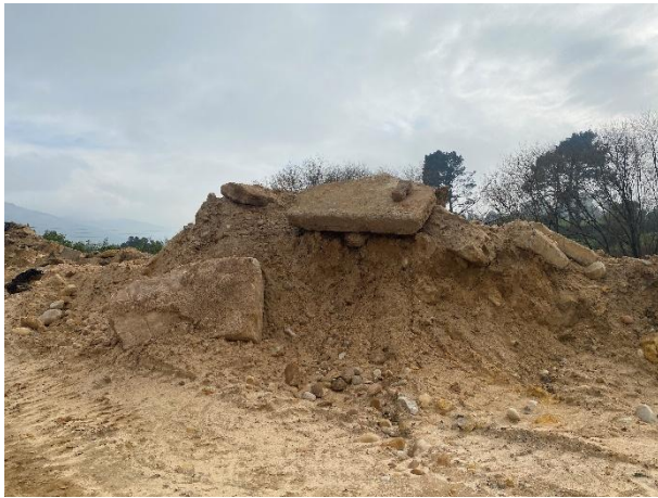
Dumped base material after the construction of the mall west of the development site, creating a quarry.
