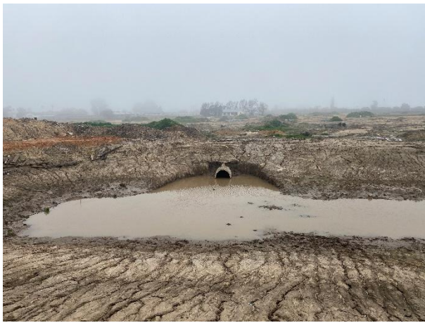
Stormwater pipeline installed in the large pond to direct water toward the main outlet along the Berg River.
