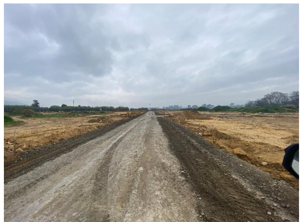
Roads being chipped and sprayed south of the foreman's house.
