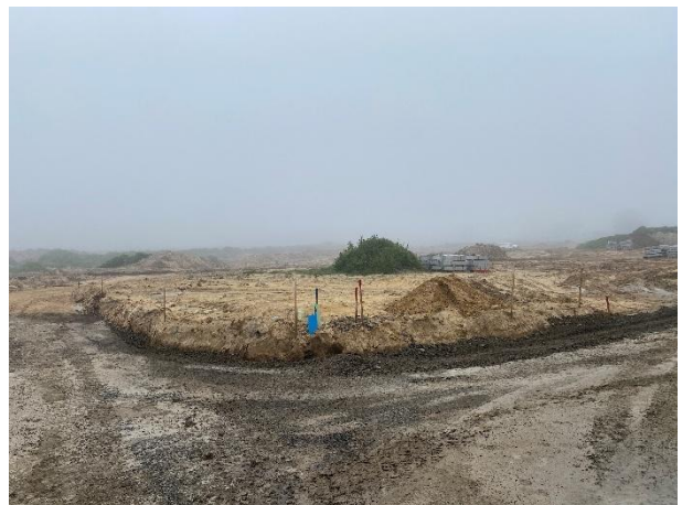
Towards the west, internal roads are being chipped and sprayed with material placed along the development.
