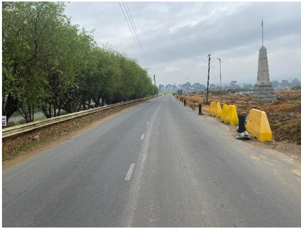
Condition of New Eskdale Street towards the North.
