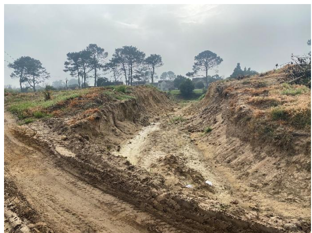
Excavated stormwater outlet channel north towards the Berg River.
