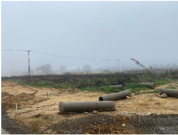
Stormwater pipeline material adjacent to the road being chipped and sprayed west of the Firwoods Homestead.
