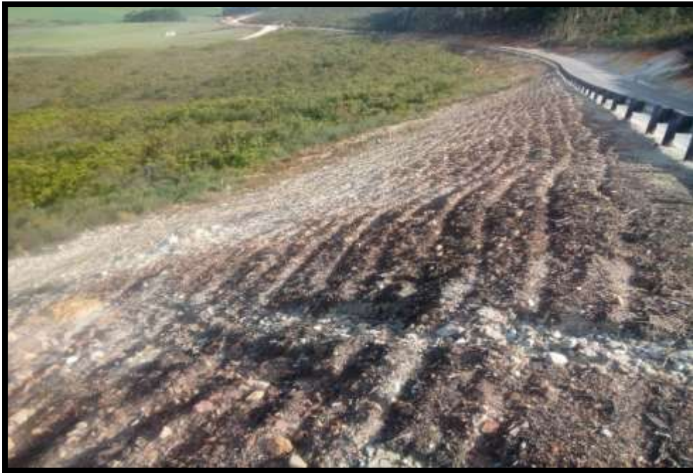
Figure 10: Example of horizontal terracing to reduce down slope erosion.
