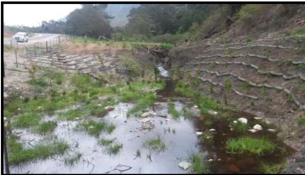
Figure 11: Example of horizontal terracing with biodegradable sausages to reduce down slope erosion.
