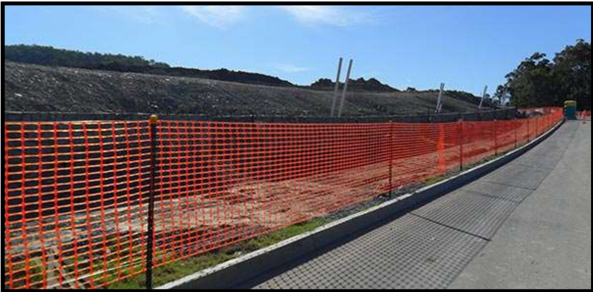
Figure 13: Example of a rehabilitated area cordoned off with danger netting.
