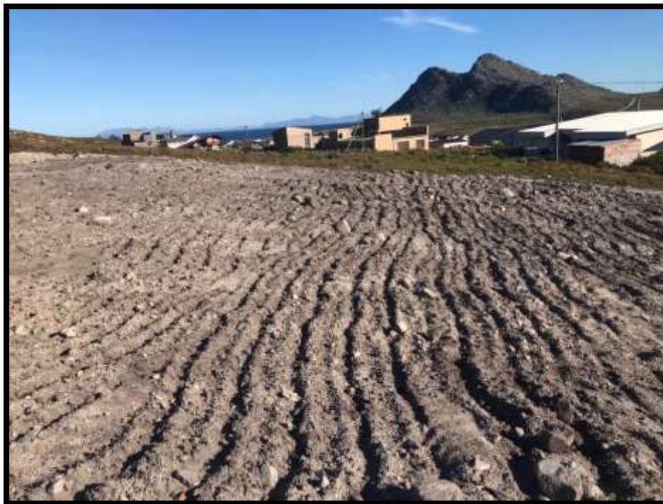
Figure 9: Example of a previously compacted area that has been ripped, shaped and topsoil spread over the affected area prior to rehabilitation.
