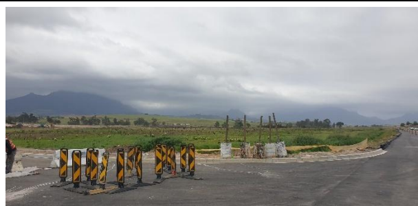
Construction of the main access road.
