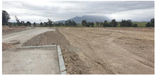
Civil services and internal roads being installed.
