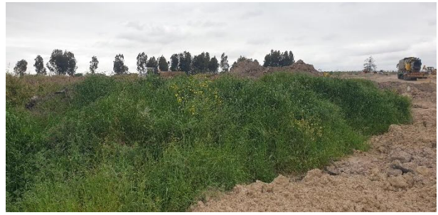
Vegetated topsoil stockpiles towards the north.
