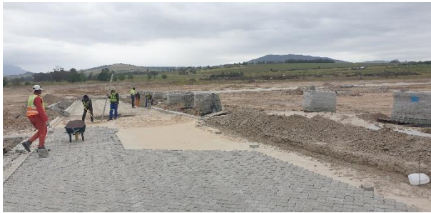
Internal roads are being paved, and kerbs are being installed.
