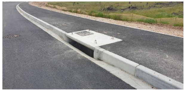
Stormwater inlet along the main access road.
