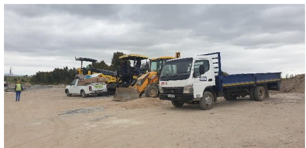
Material stockpiles have been placed adjacent to the site camp along with the machinery in use.
