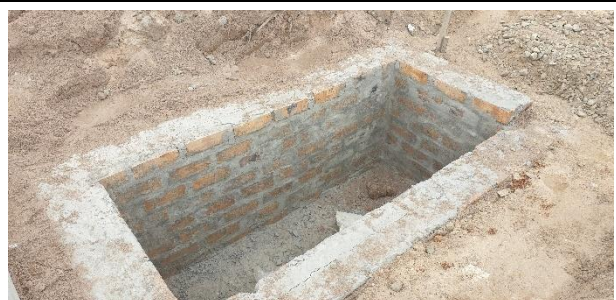
Stormwater inlet structures being constructed within the bus and visitor parking area.
