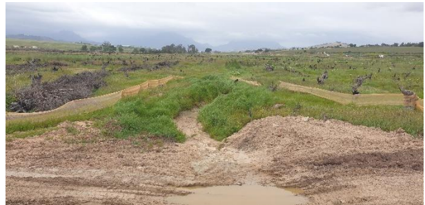
Box culvert outlet with shaped discharge channel directing stormwater toward the wetland.
