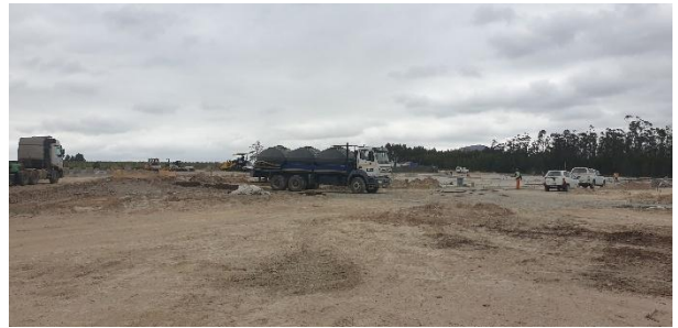
Water truck available on site near the works area.
