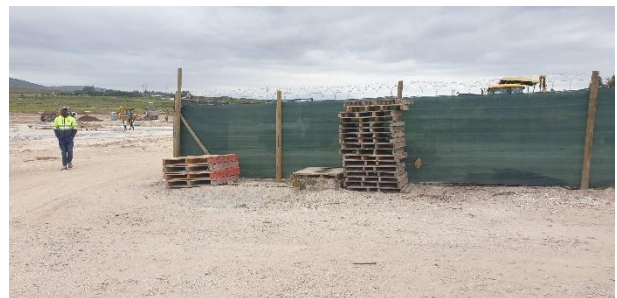
Screened site camp towards the northwest.
