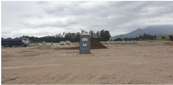
Chemical toilet adjacent to the parking construction area.
