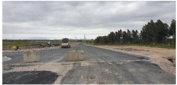
Main access road towards the west, bitumen surfacing in progress.
