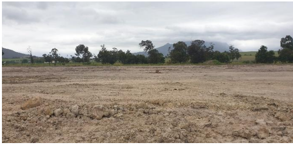
View towards the east, where the staff housing, maintenance yard, and stock nursery will be located.
