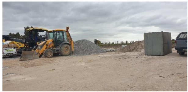
Material stockpiles have been placed adjacent to the site camp along with the machinery in use.
