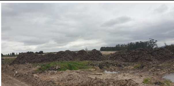
Cleared biomass has been chipped and stockpiled separately in the eastern portion of the site.
