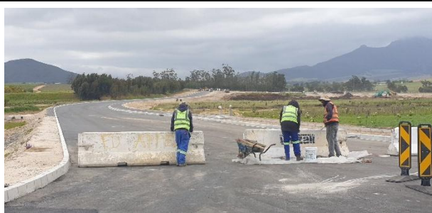
Construction of the main access road.
