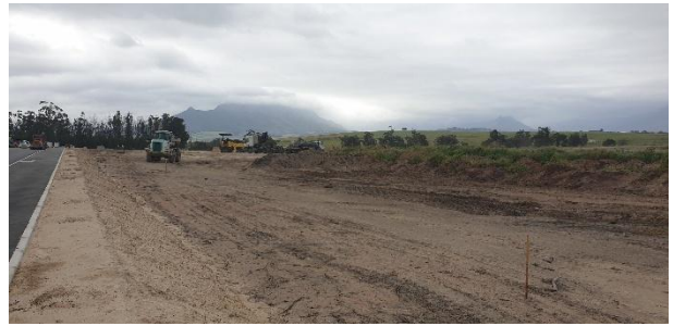
Cleared topsoil stockpiles towards the northeast.
