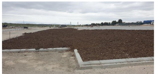
Gardens being landscaped at the parking area.
