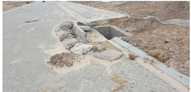
Sandbags placed alongside stormwater inlets to prevent sediment runoff.
