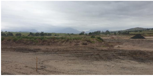
Cleared topsoil stockpiles towards the northwest.
