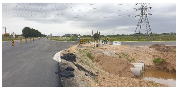
Entrance to the site off the main access road. Traffic management is being implemented.
