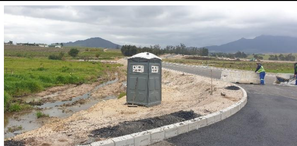
Chemical toilet in place at the construction site of the main access road.
