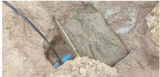
Civil services being installed.
