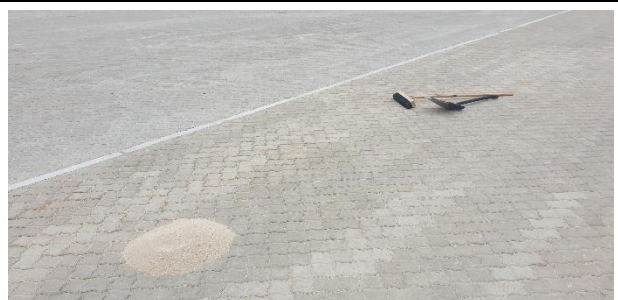
Sand grouting in progress on newly paved internal roads.
