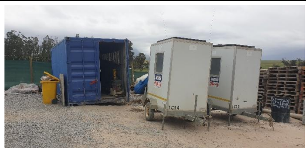
Condition of the site camp.
