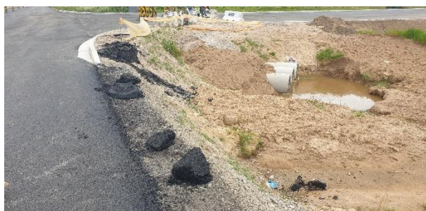
Access road and civil services (stormwater) being installed. Bitumen remains must please be removed.
