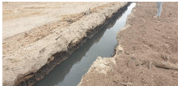
Drainage channels being shaped across the site.
