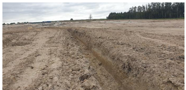
Drainage channels being shaped across the site.
