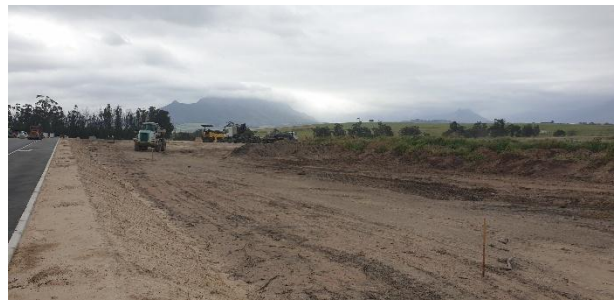
Cleared topsoil stockpiles towards the northeast.
