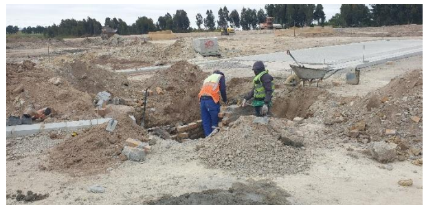
Stormwater inlet structures being constructed within the bus and visitor parking area.
