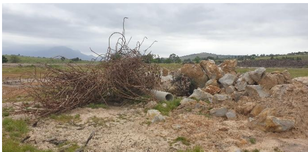
Construction rubble to be removed.
