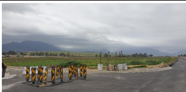
Construction of the main access road.
