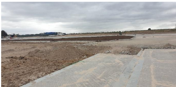
Gardens being landscaped at the parking area.
