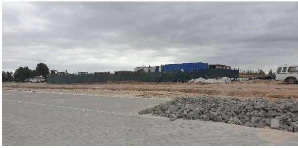
View of the site camp towards the north.
