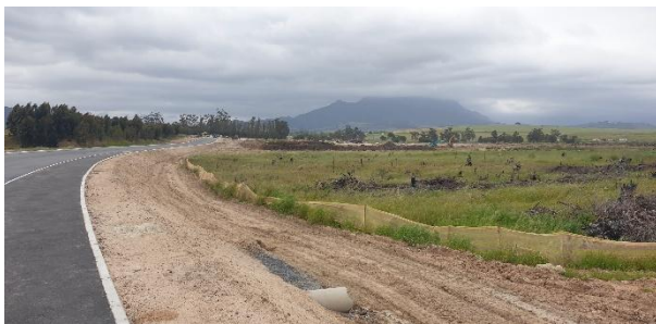
Demarcated wetland area along the main access road.
