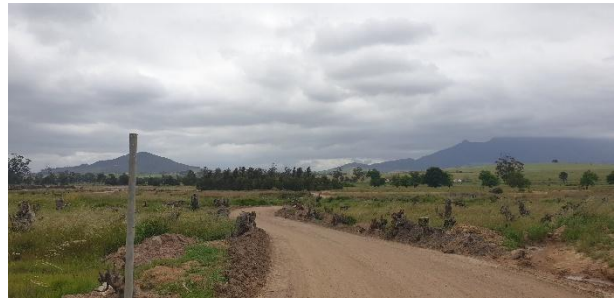
Haul roads demarcated from the access road towards the construction site.
