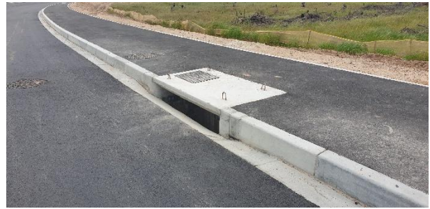
Stormwater inlet along the main access road.
