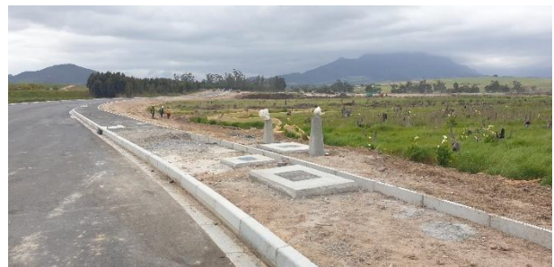
Pedestrian walkways under construction alongside the main access road.
