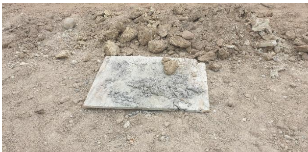
Cement batching occurring on site on the appropriate mortar boards.
