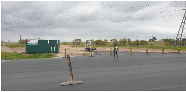
Main access road under construction, with adjoining access road upgrades in progress.
