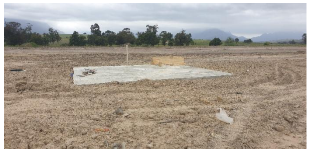
Concrete service chamber under construction as part of the site's civil infrastructure network.
