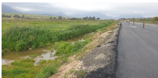
Drainage channel adjacent to the R44 to Stellenbosch.
