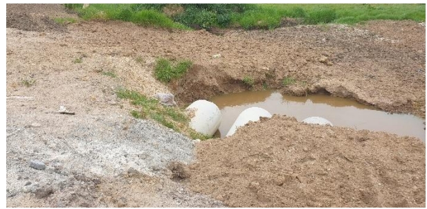
Outlet stormwater services being installed into the drainage channel adjacent to the R44 to Stellenbosch.
