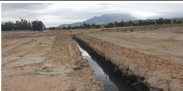
Drainage channels being shaped across the site.
