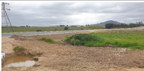
Condition of the main access road towards the north.
