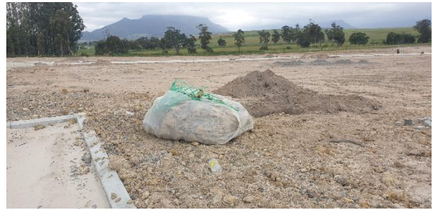
Empty cement bags securely wrapped in plastic sheeting to prevent dust dispersion.
