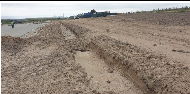
Drainage channels being shaped across the site.
