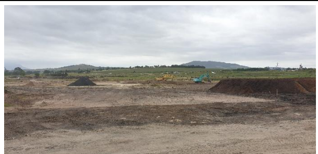
Stockpile area towards the northwest.
