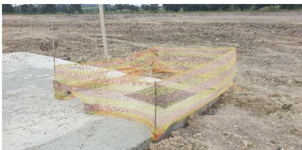
Concrete service chamber under construction as part of the site's civil infrastructure network.
