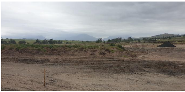
Cleared topsoil stockpiles towards the northwest.
