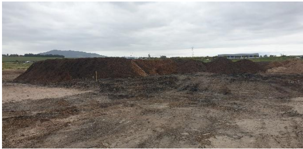
Stockpile area towards the northwest.
