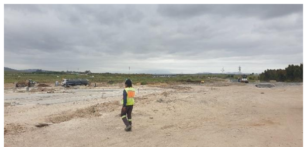
Bus and visitor parking being constructed towards the north.
