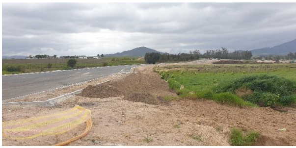
Shaped and sloped road embankment prepared for erosion control.
