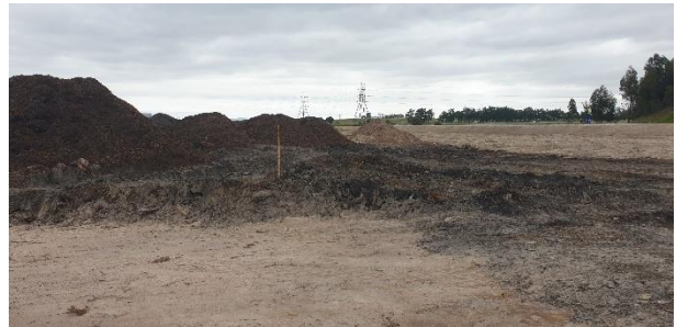
Stockpile area towards the northwest.
