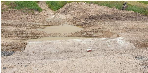
Box culvert installed beneath the main access road to facilitate stormwater flow.
