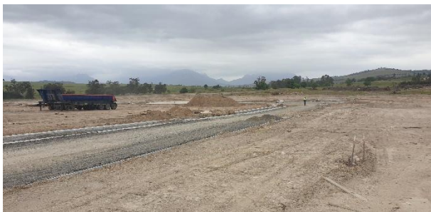
Civil services and internal roads being installed.
