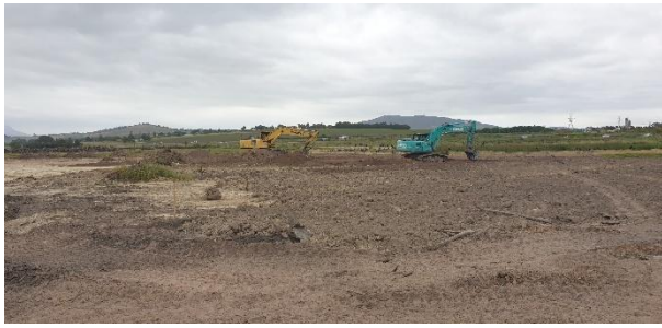
Location of the traditional headstone grave site. Topsoil and composting are being spread across the site.
