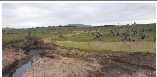
Rehabilitation/Wetland area fully demarcated. Contractor is reminded to install sediment traps where necessary.
