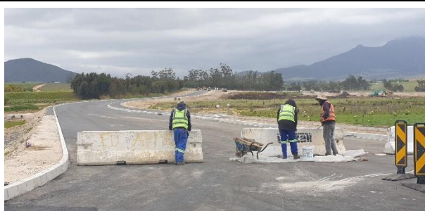
Construction of the main access road.
