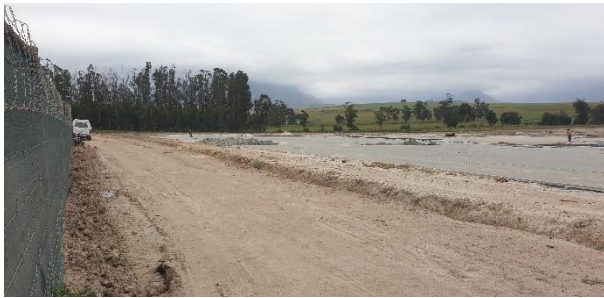
Bus and visitor parking being constructed towards the north.
