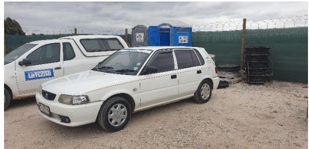
Chemical toilets present within the site camp.
