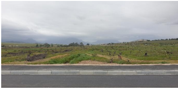
Box culvert outlet with shaped discharge channel directing stormwater toward the wetland.
