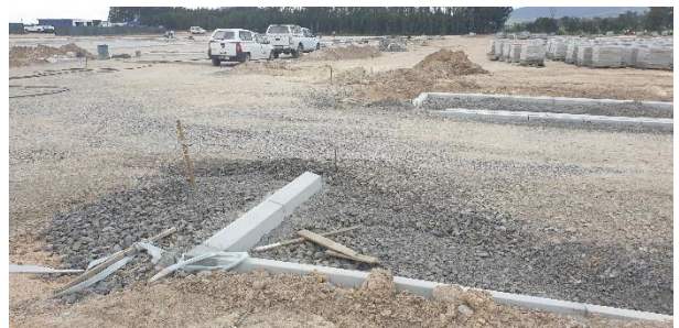
Kerbs being installed within the bus and visitor parking area.
