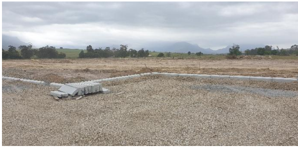
Kerbs being installed within the bus and visitor parking area.
