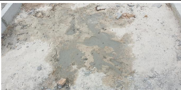
Pedestrian walkways under construction alongside the main access road.
