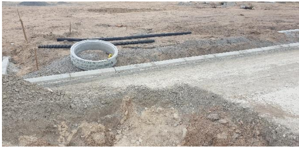
Civil services and internal roads being installed.
