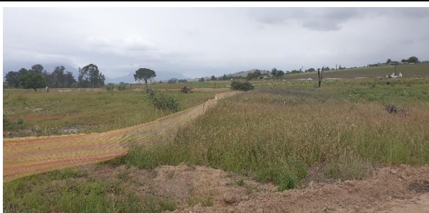
Buffer and wetland/rehabilitation areas have been demarcated with orange netting and danger tape.
