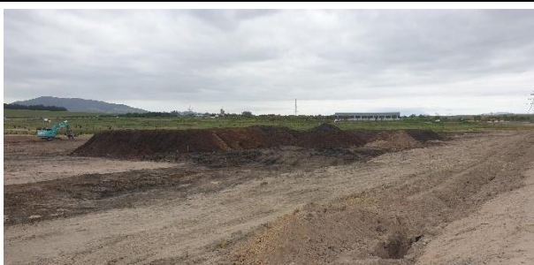
Stockpile area towards the northwest.
