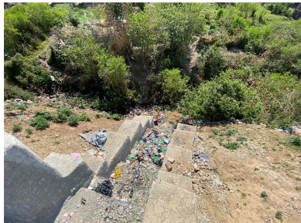
New gabion/mattress flood attenuation works completed. Local residents responsible for dumping.
