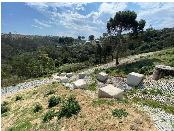
Completed armorflex stormwater channel.
