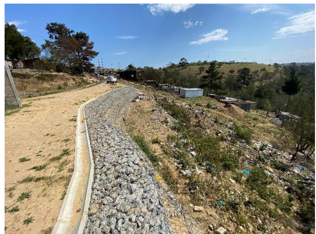
Backfilling completed with rehabilitation (topsoil and grass seed/sods) finalised.
