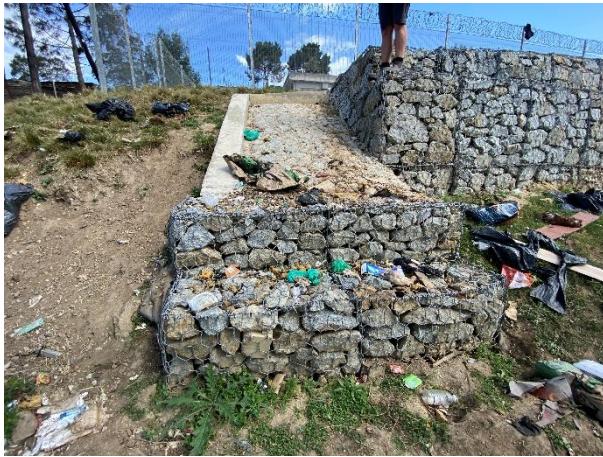
Shaping and tie in at the ends of the gabion structure completed. Local residents responsible for dumping.
