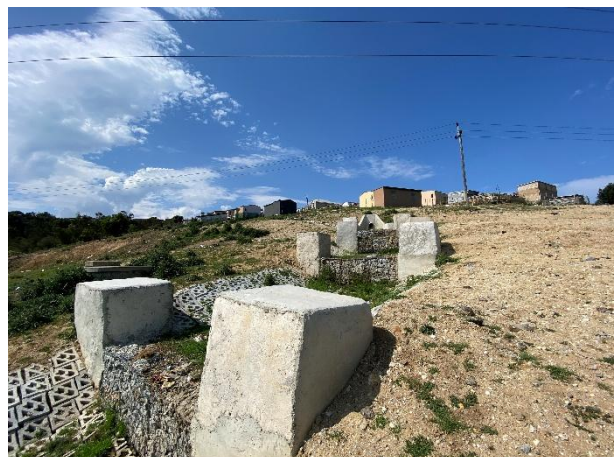
New terramesh and gabions constructed for main drainage channel
