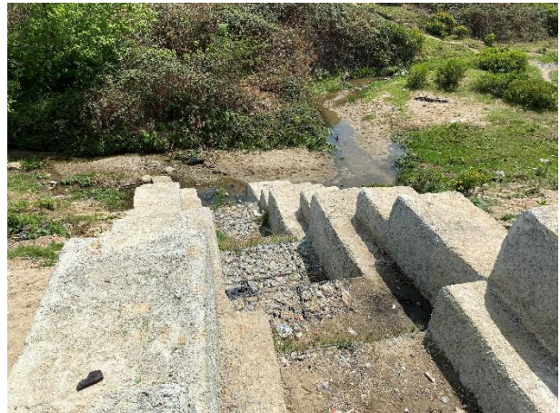
New gabion/mattress flood attenuation works completed.
