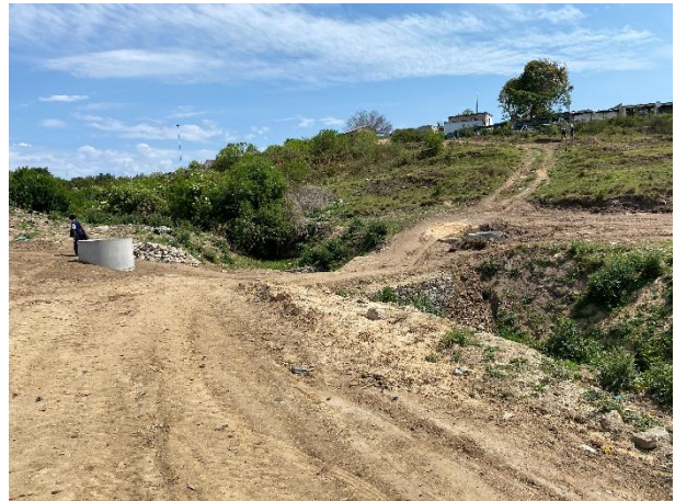
Replaced stormwater and manhole infrastructure.
