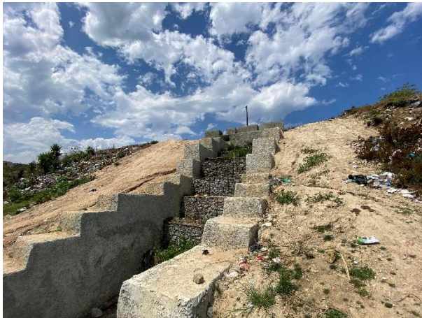
Backfilling and shaping of area adjacent to the works completed.
