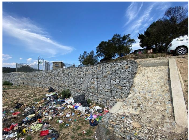
Completed reconstruction of gabion retaining wall. Local residents responsible for dumping.
