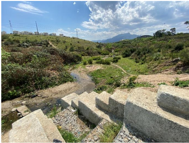
New gabion/mattress flood attenuation works completed.
