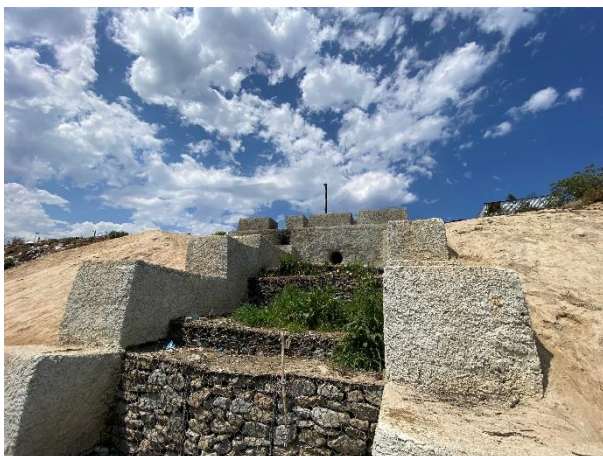
New gabion/mattress flood attenuation works completed.
