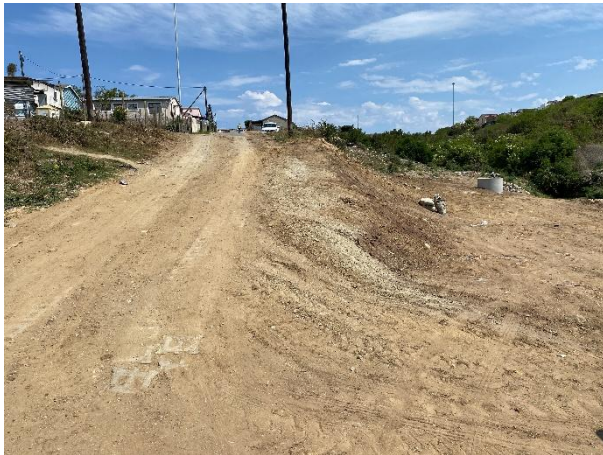
Access road towards the construction area.
