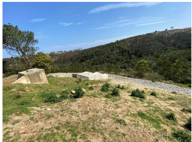
Completed armorflex stormwater channel.
