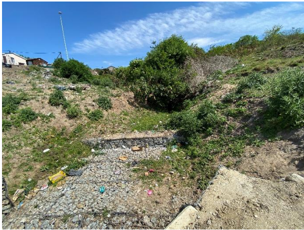
New gabion/mattress flood attenuation works outlet completed.
