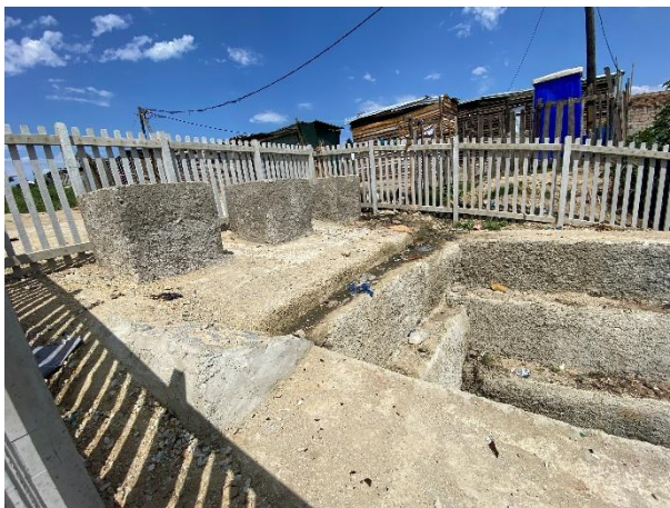
Completed upgraded/replaced SW outlet structure.
