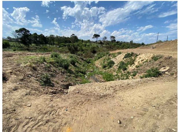
Upgraded stormwater outlet infrastructure.
