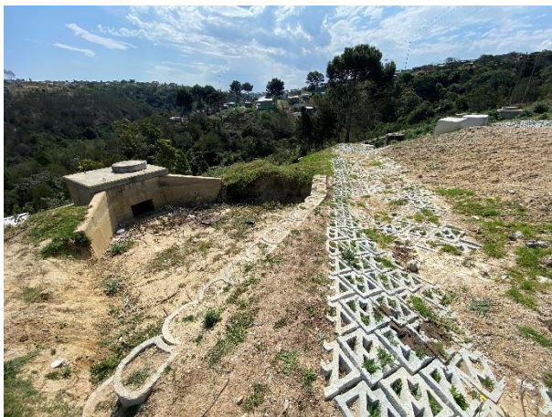
Completed armorflex stormwater channel, inlet and manhole infrastructure.
