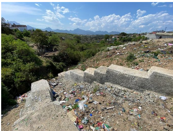
New gabion/mattress flood attenuation works outlet completed. Local residents responsible for dumping.
