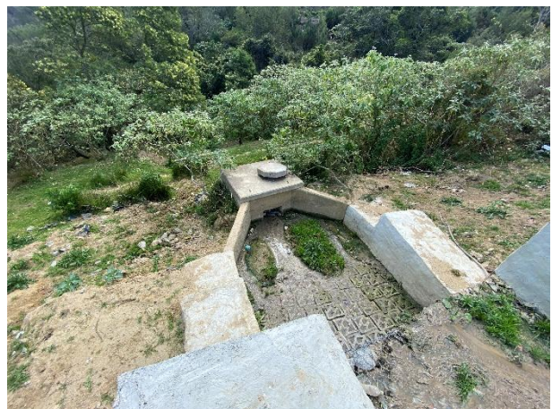
Replaced stormwater inlet infrastructure.
