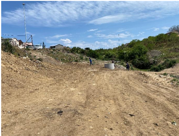
Replaced stormwater and manhole infrastructure.
