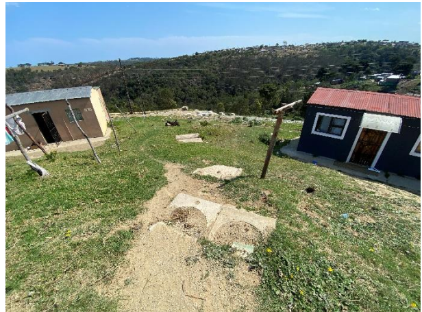
Newly constructed manhole infrastructure.
