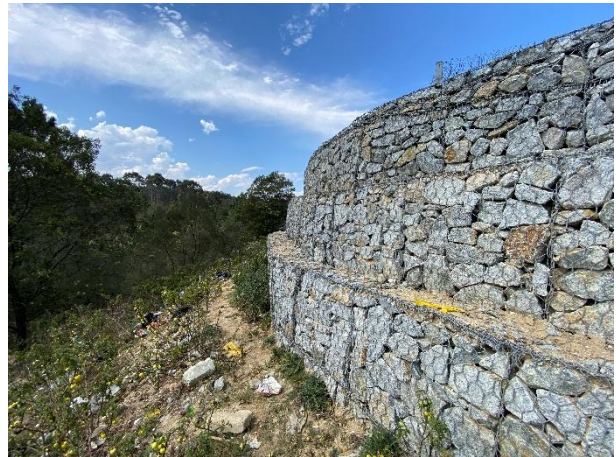
Completed reconstruction of gabion retaining wall.
