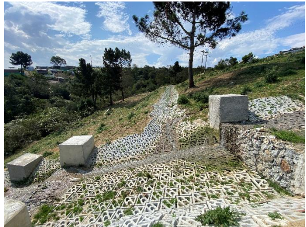
Completed armorflex stormwater channel and mitre drains.
