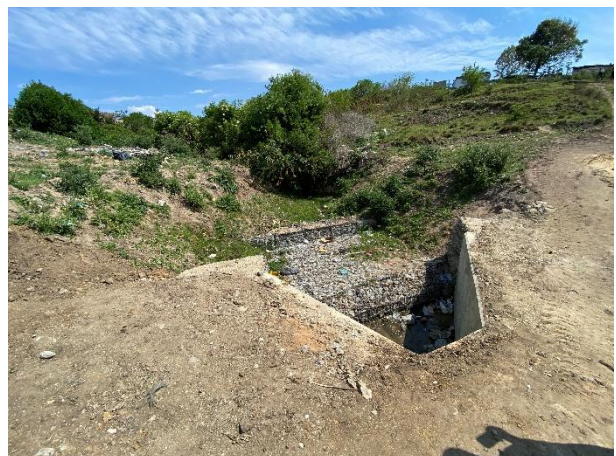
Upgraded stormwater outlet infrastructure.
