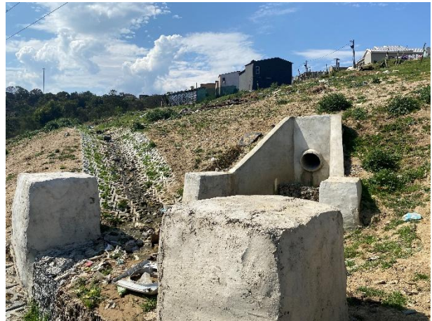
Newly construction stormwater outlet infrastructure.
