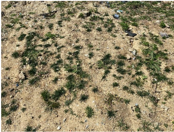
Slopes adjacent to the drainage channels have been shaped and rehabilitated, erosion backfilled.
