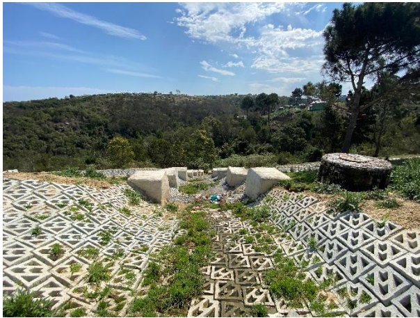
Completed armorflex stormwater channel.
