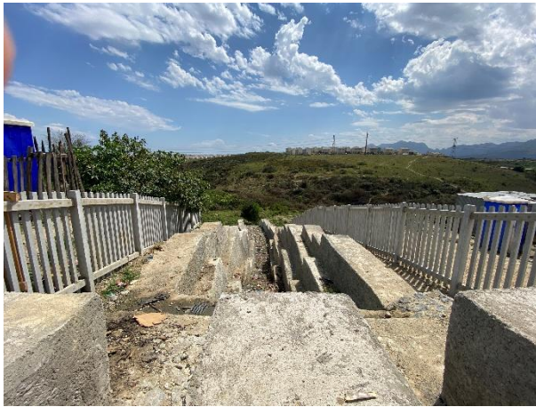
Completed upgraded/replaced SW outlet structure.
