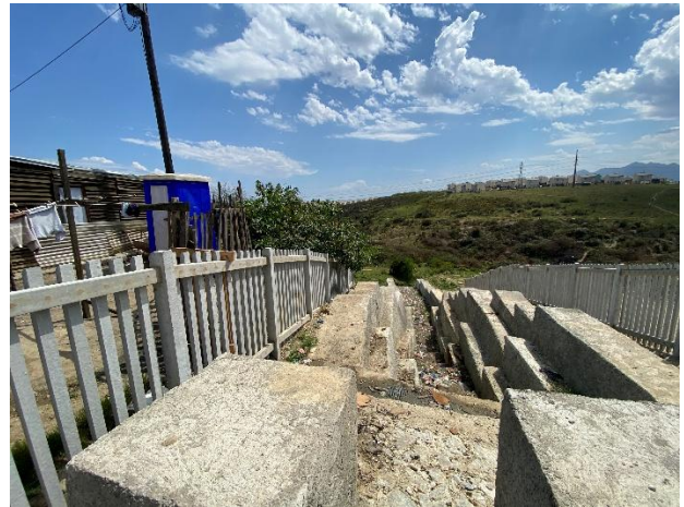
Chemical toilet available adjacent to the works area.
