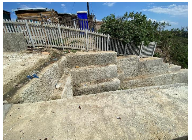
Completed reconstruction of stormwater outlet structure headwall.
