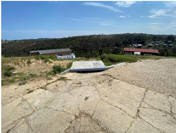
Newly constructed stormwater inlet infrastructure.
