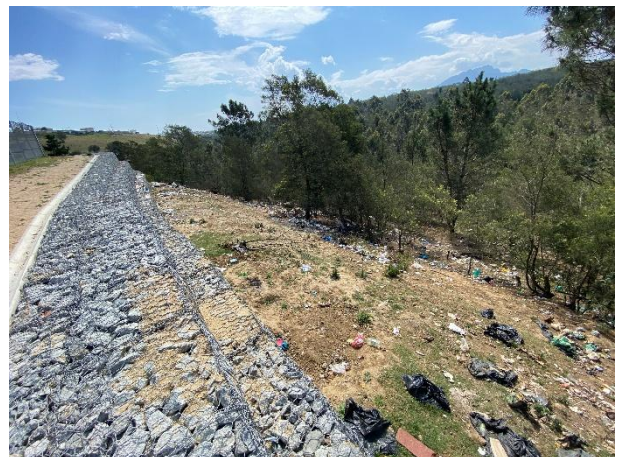
Completed reconstruction of gabion retaining wall. Slope below the retaining wall has been shaped.
