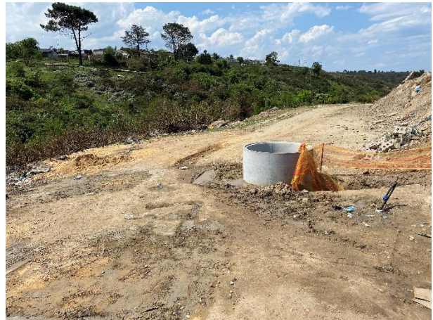
Replaced stormwater and manhole infrastructure.
