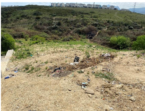
Backfilling and shaping of area adjacent to the works completed.
