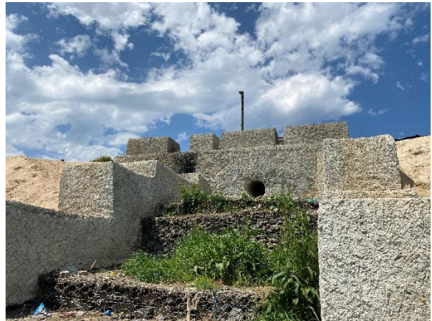
New gabion/mattress flood attenuation works completed.
