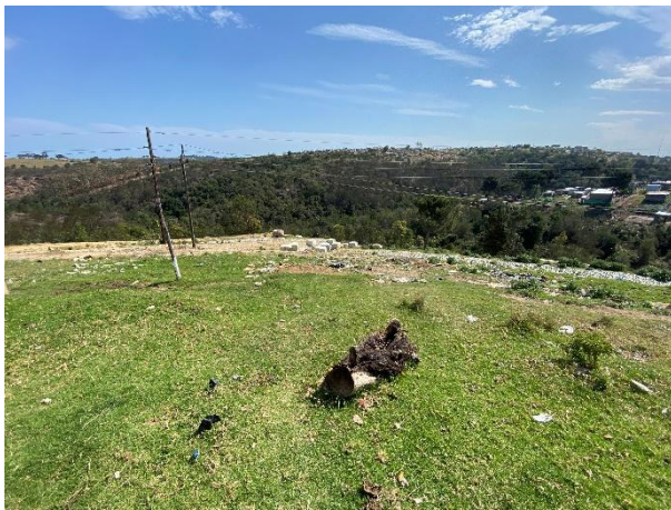
Slopes adjacent to the drainage channels have been shaped and rehabilitated, erosion backfilled.
