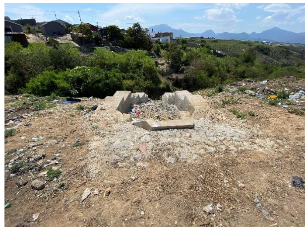
New gabion/mattress flood attenuation works outlet completed. Erosion damage fix and rehabilitated.
