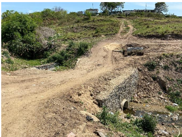
Access road adjacent to the works area.
