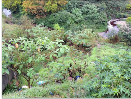
Figure 6: Photographs of Site 2 showing eroded, incised channels below existing gabion structures. Channels are bordered by Cenchrus clandestinus and invaded by Ricinus communis and Solanum mauritanum .
