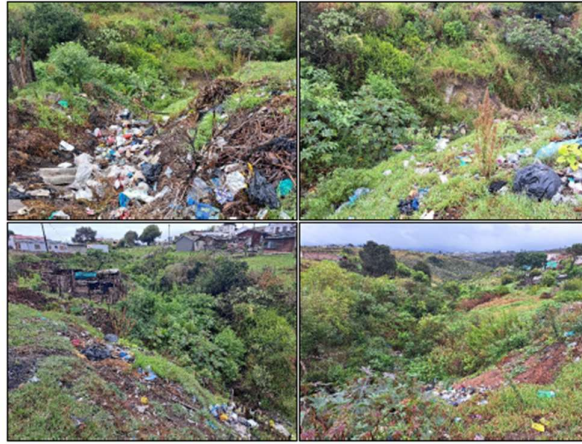
Figure 9: Photographs illustrating the steep embankment down to the eroded non-perennial drainage line.
