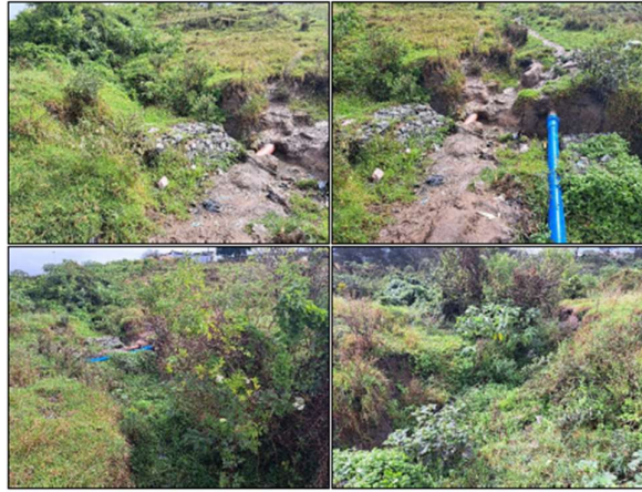
Figure 12: Photographs at Site 77 illustrating the exposed sewage pipeline, eroded bed and banks and incised channel.
