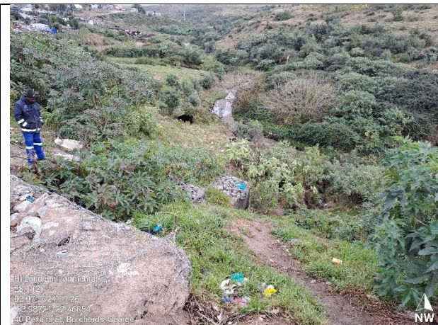
Site condition before commencement
