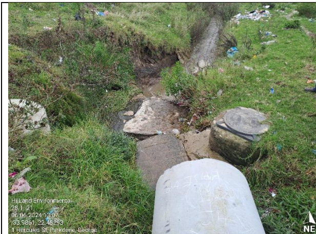
Site condition before commencement
