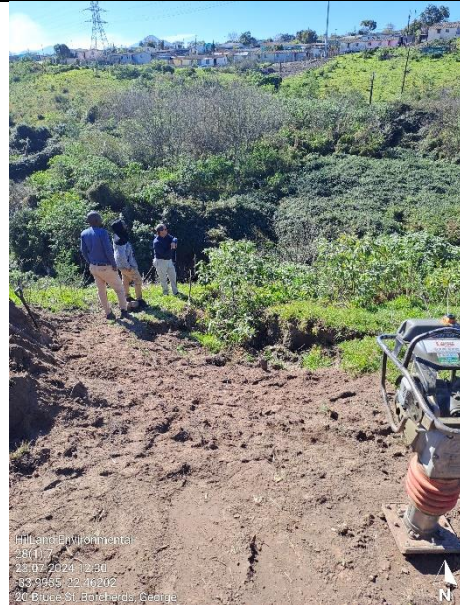
Backfilling and compacting within the demarcated (pegged) footprint
