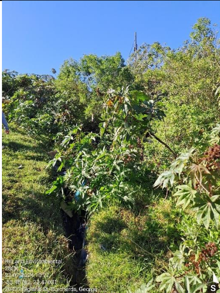
Construction footprint pegged out
