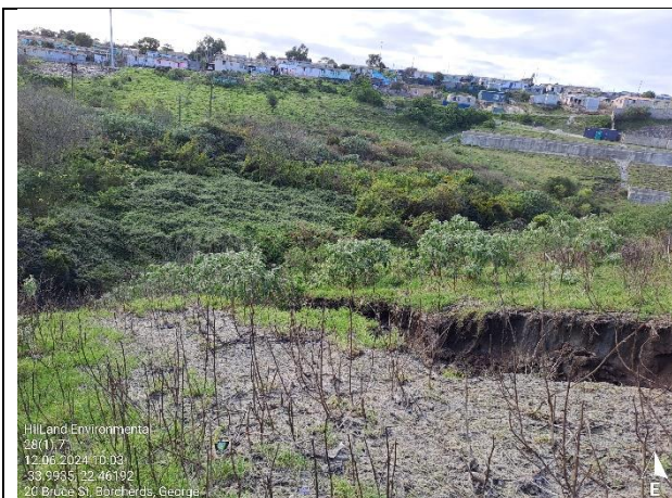
Site condition before commencement
