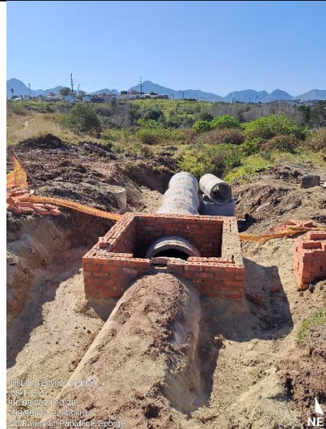
Construction progress – new manhole
