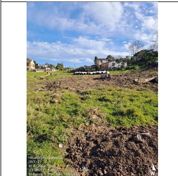
Construction material stockpile
