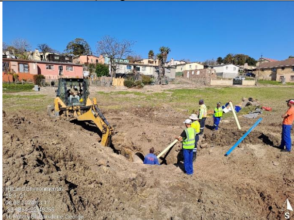
Construction progress – tie in with existing stormwater line
