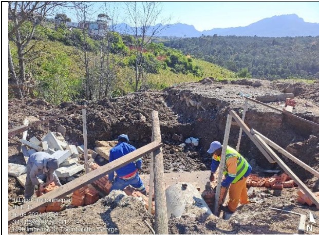
Construction progress – headwall construction
