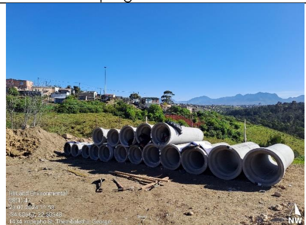
Construction material stockpile on existing disturbed area (historic dump area)
