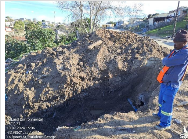
Exposing existing stormwater infrastructure and excavation within the pegged working zone.
