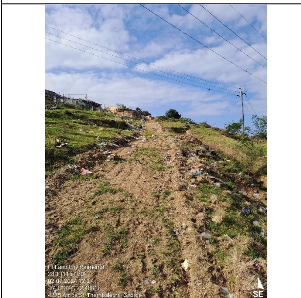
Site condition before commencement Proposed access to the site
