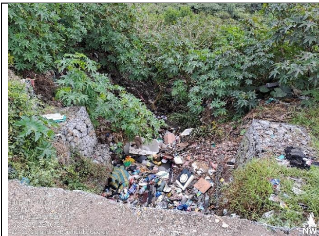
Site condition before commencement
