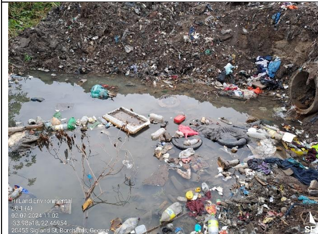
Exposing the existing stormwater pipe
