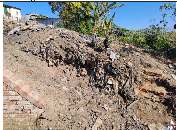
Final shaping to be done
