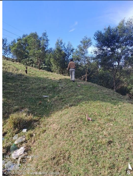
Construction footprint pegged out
