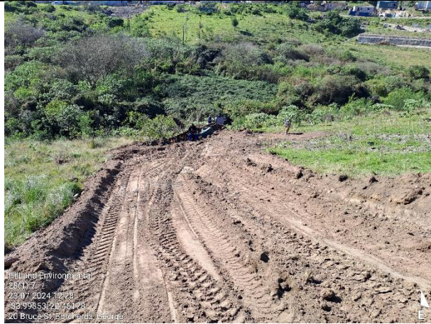
Temporary construction access
