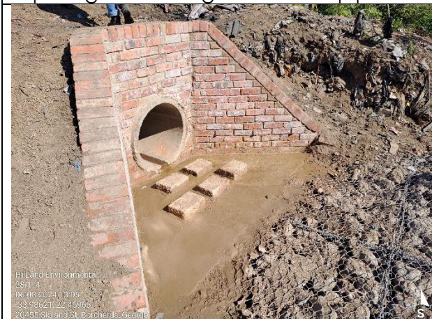
New headwall and gabion/reno protection complete
