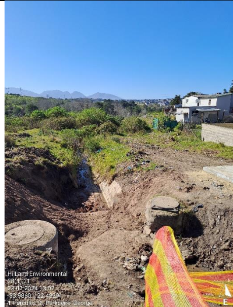
Construction progress – note the demarcation is in place which gets vandalized and/or stolen when the contractor leaves the site
