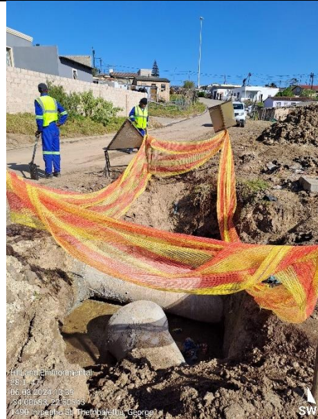
Construction progress – note the demarcation is in place at the time of the inspection
