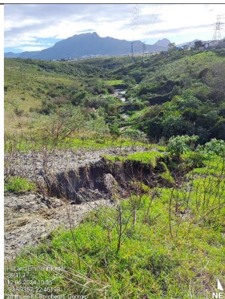
Site condition before commencement
