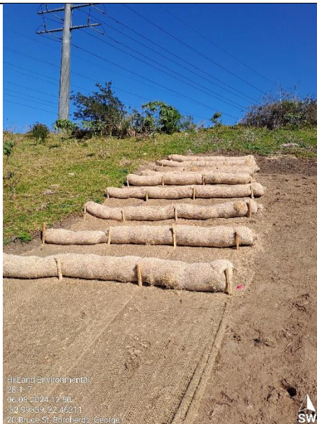
Rehabilitation complete – erosion protection installed
