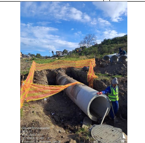
Exposing existing stormwater infrastructure
