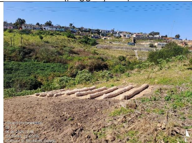
Rehabilitation complete – erosion protection installed
