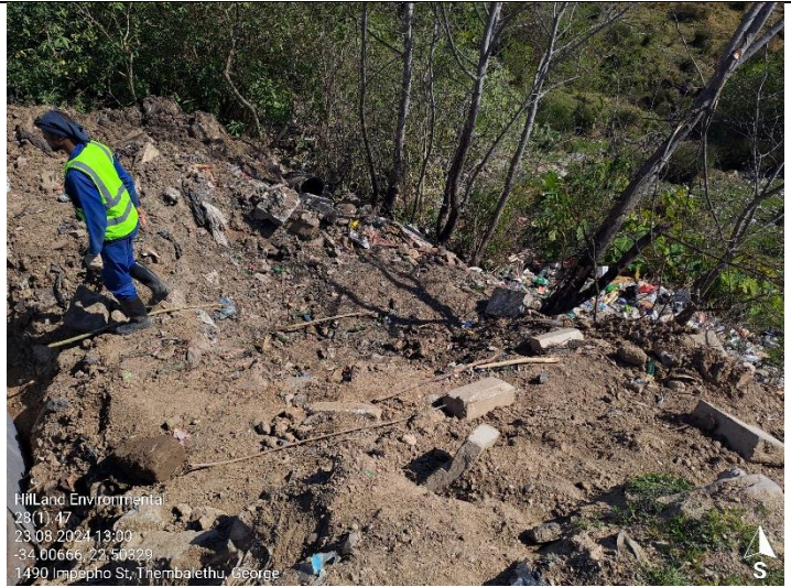
Working within the construction zone
