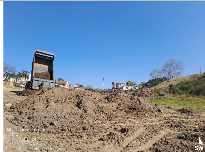
Topsoil for rehabilitation and shaping
