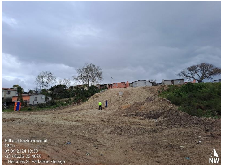
Shaping of the slope around the stormwater infrastructure is complete, and rehabilitation in progress.
