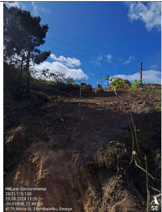
Site preparation – silt fences will be required if the slope is left exposed for a prolonged period
