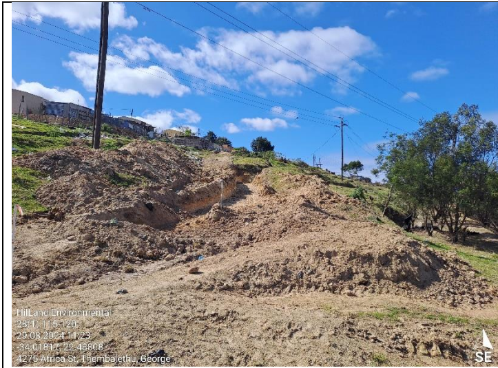
Site preparation in progress.
