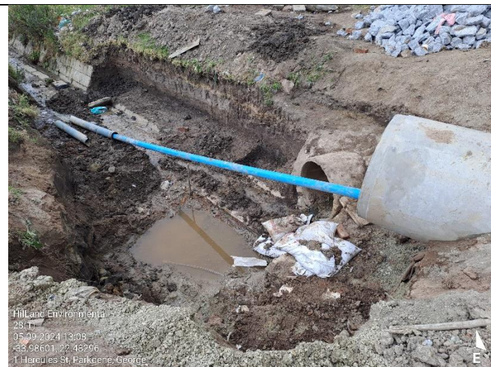
Construction of the stormwater headwall.
