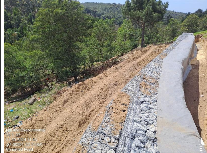
Backfilling behind the gabion structure in progress.
