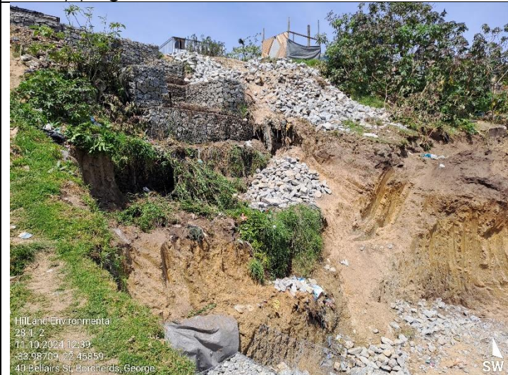
Construction material stockpile area – road reserve.
