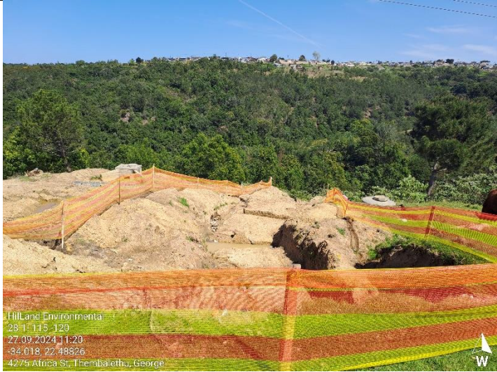
Construction progress – site demarcation in place.
