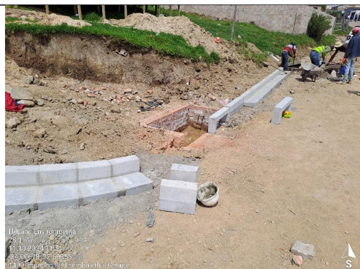
Construction progress – stormwater inlet
