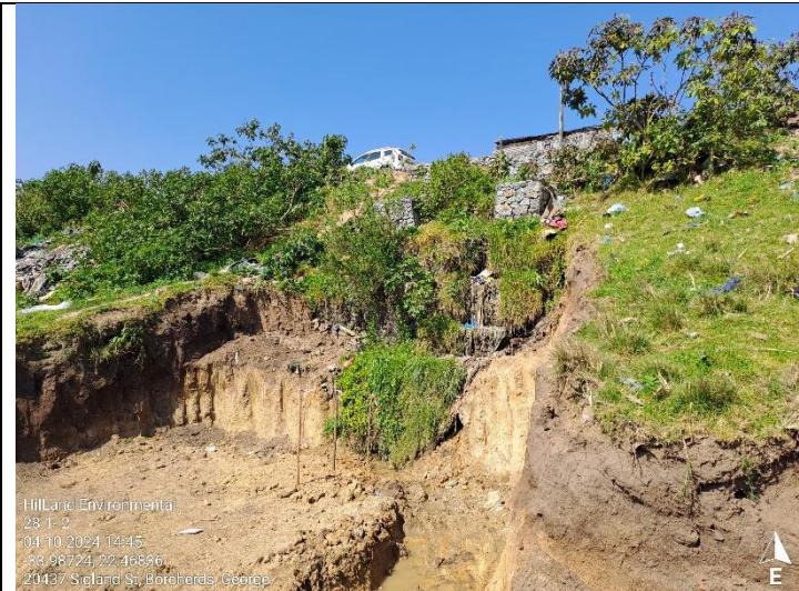
Construction progress – rubble removed, and survey pegs installed.
