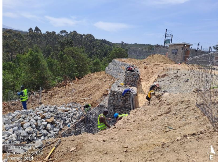
Construction progress – gabion retaining structure.
