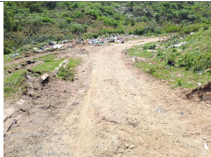
Existing access track is used.
