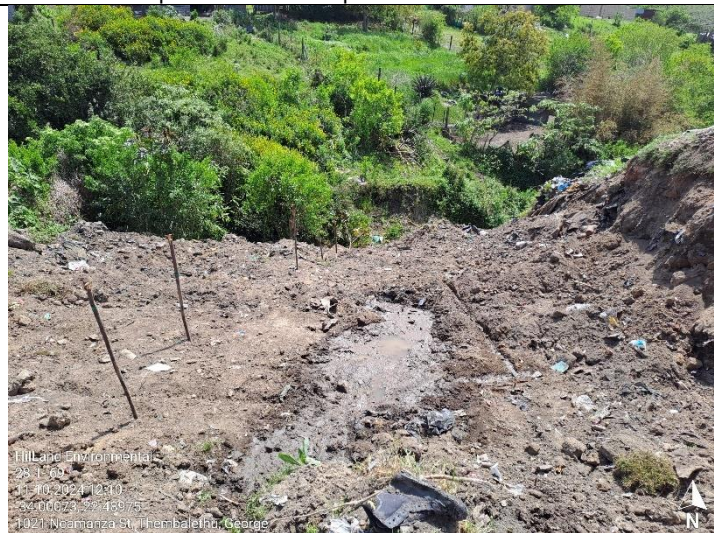
Construction footprint – silt fence to be installed below the last gabion position to prevent silt movement into the stream.
