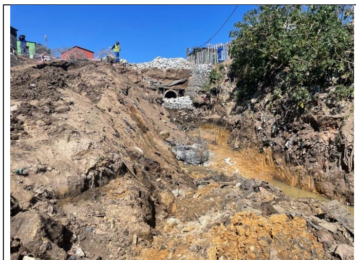
Photo by WEC – 19.09.2024 – construction progress. Access (left) as per the contractor's method statement.
