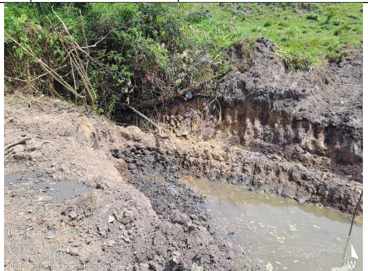
Excavation in progress. Silt fence to be installed and maintained to prevent silt movement downstream.
