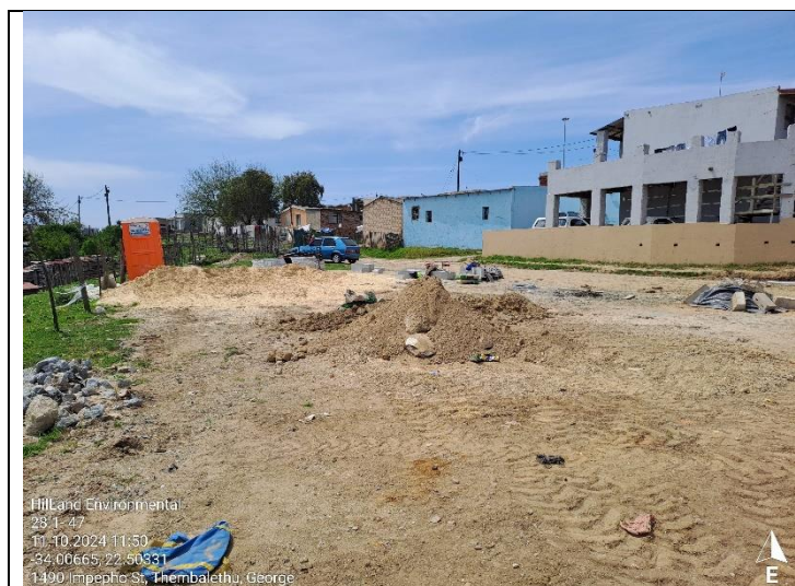
Portable toilet on site. Material stockpile area – previously transformed area.
