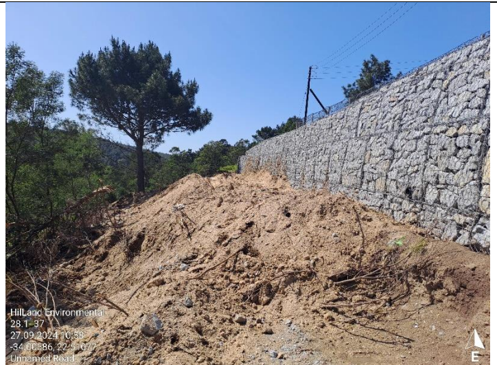
Shaping/sloping below the gabion structure in progress.
