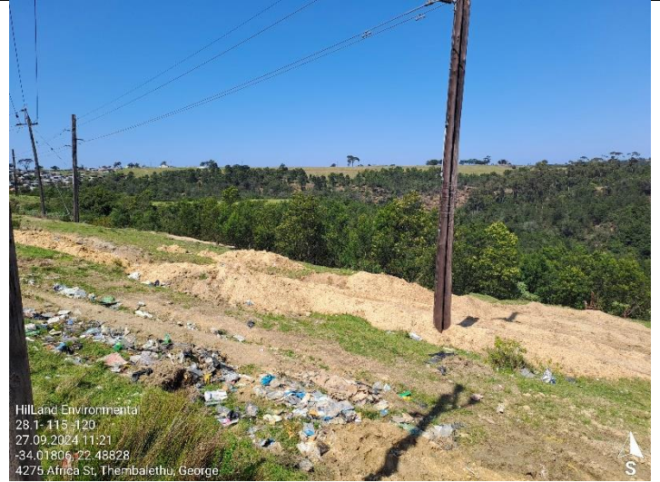
Site preparation and construction progress.
