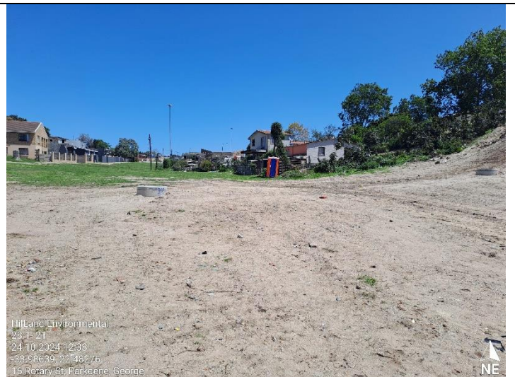
Compacted soil was loosened.
