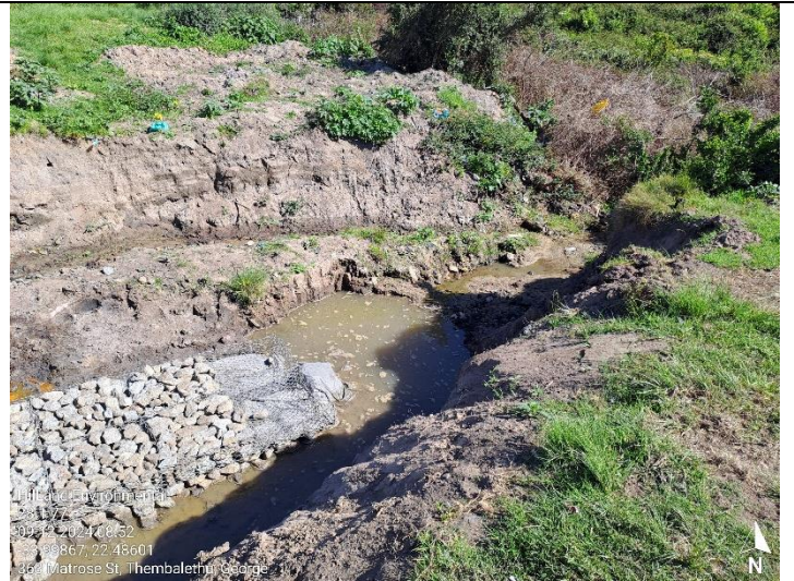
Temporary stream diversion in place during gabion construction.
