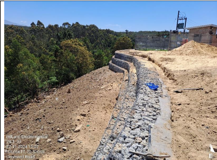
Gabion retaining wall construction completed.
