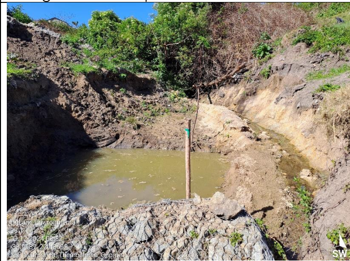
Temporary stream diversion in place.
