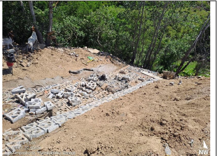
Working within the construction zone outside of the 32m buffer.
