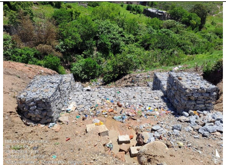
Contractor progress – note litter/rubble dumped after hours (not the contractor).
