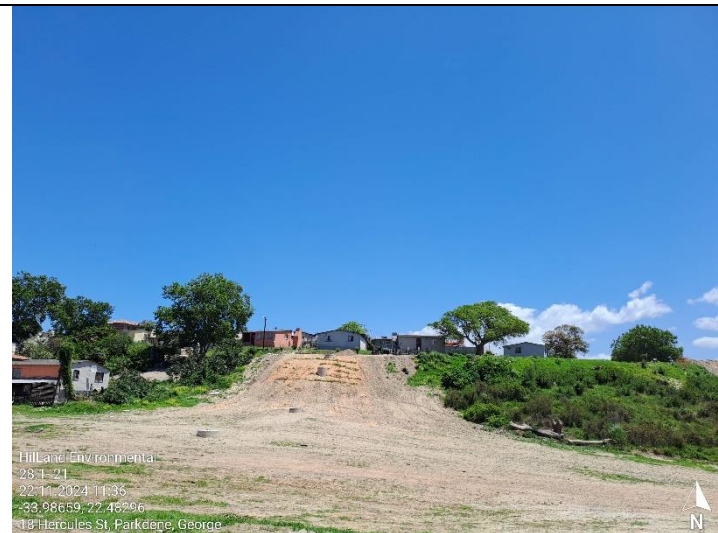
Shaping of the slope around the stormwater infrastructure and rehabilitation is complete.
