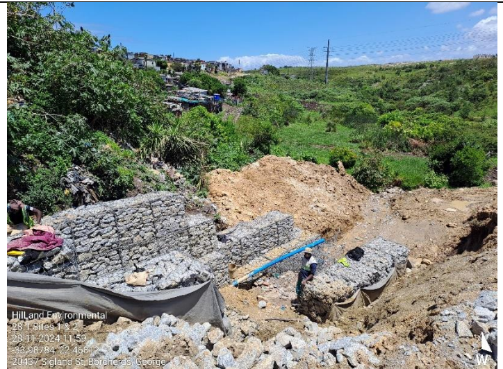
Construction progress. Excavated soil consists of historic dumped material (litter/rubble etc).
