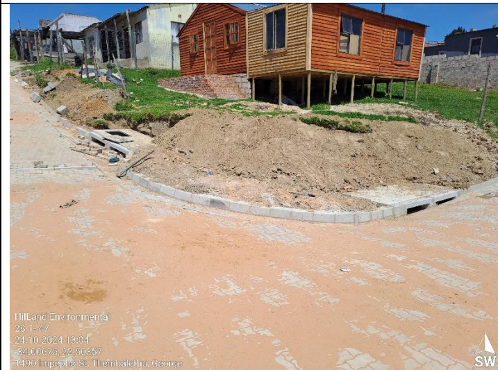
Construction progress – stormwater inlets.
