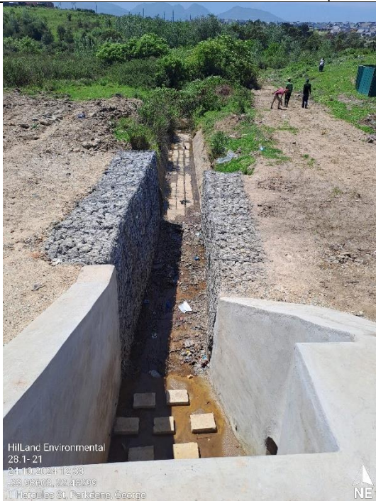
Headwall construction completed
