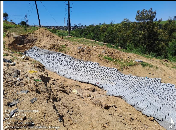
Construction progress – armorflex stormwater channel.
