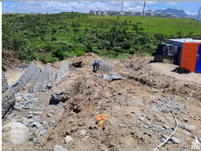
Construction progress. Gabion installation in progress.
