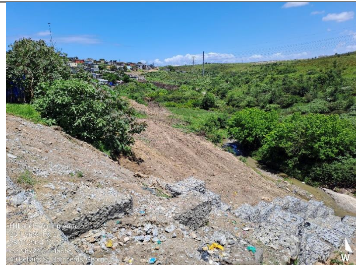
Gabion structure construction completed – final clean up to be done.
