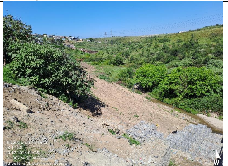
Backfilling completed – final clean-up to be done.
