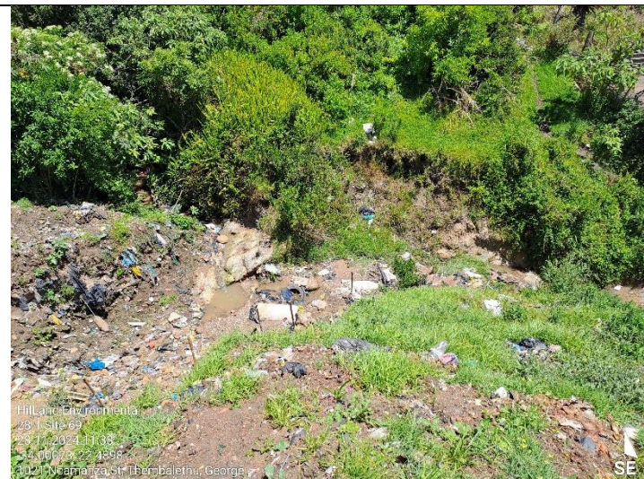
Construction footprint – silt fence to be installed below the last gabion position to prevent silt movement into the stream, however, note the degraded condition of the stream prior to commencement.
