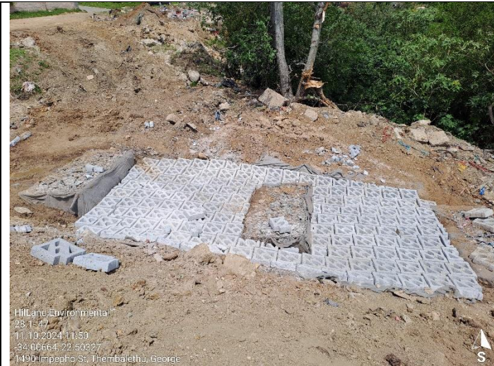
Construction progress of the stormwater outlet.
