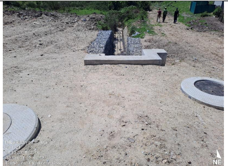
Compacted soil was loosened.
