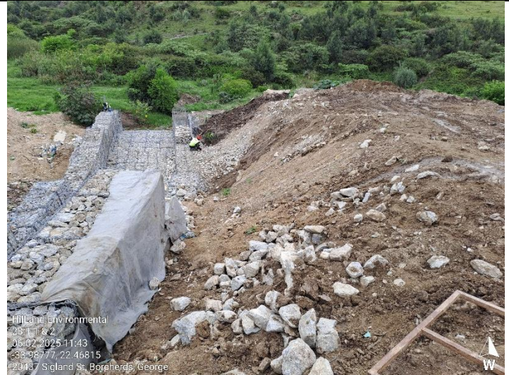
Construction progress and showing the stockpile area (RHS of the gabion structure).
