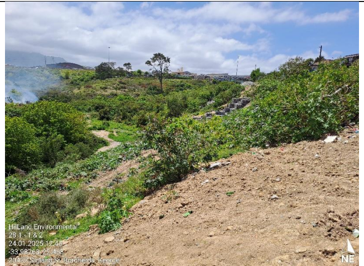
Access track shaping is done.
