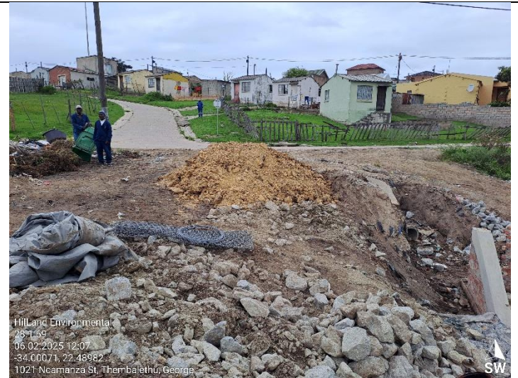
Contractor progress (69a) and construction material stockpile area. Note local residents busy dumping waste out of a wheely bin.
