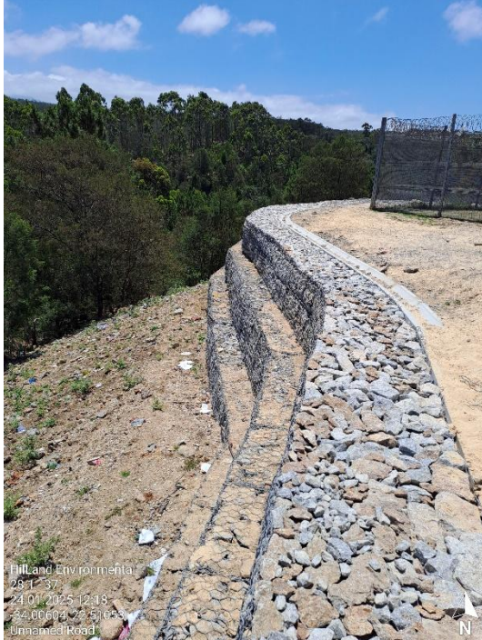
Gabion retaining wall construction completed.
