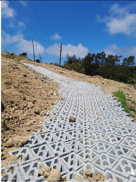
Construction progress – armorflex stormwater channel.
