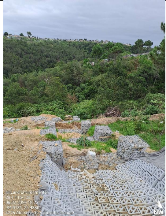
Construction site – silt is captured in the armorflex.
