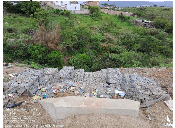
Construction footprint (69b). backfilling completed
