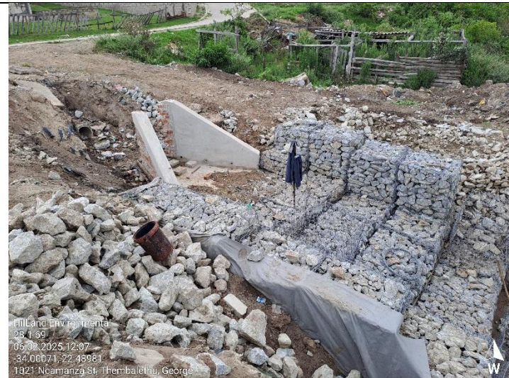
Construction progress (69a).
