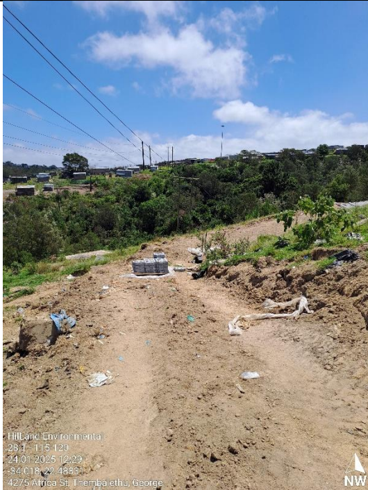
Temporary construction haul route.
