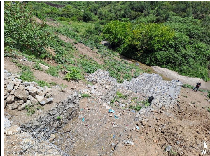
Gabion structure construction completed – tie in and clean-up in progress.
