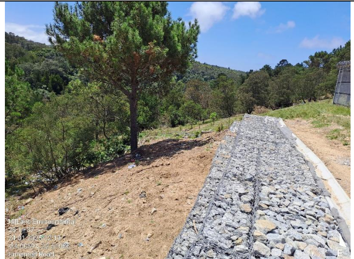
The slope below the gabion structure has been shaped to the satisfaction of the ECO.
