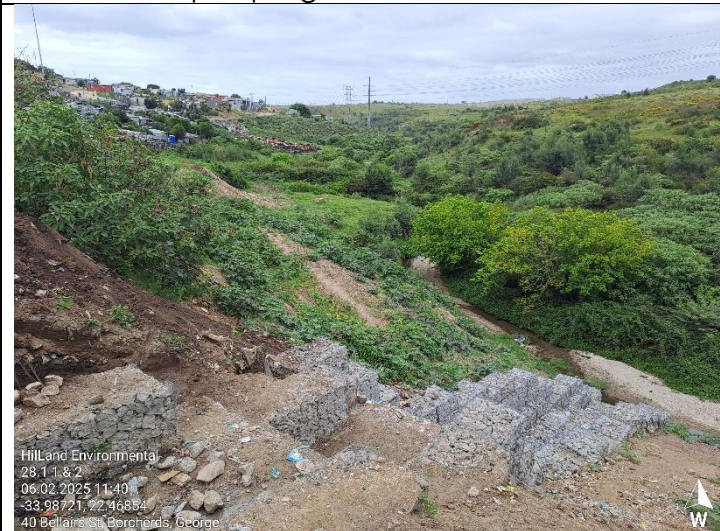
Access area to be rehabilitated with grass seed/sod mix and erosion protection (small silt fences). The invasive alien plants on the access slope must be removed.
