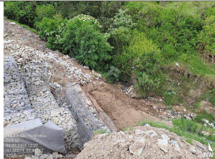
Construction progress (69a).
