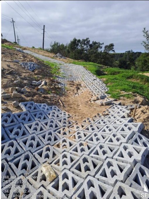
Construction progress – armorflex stormwater channel.
