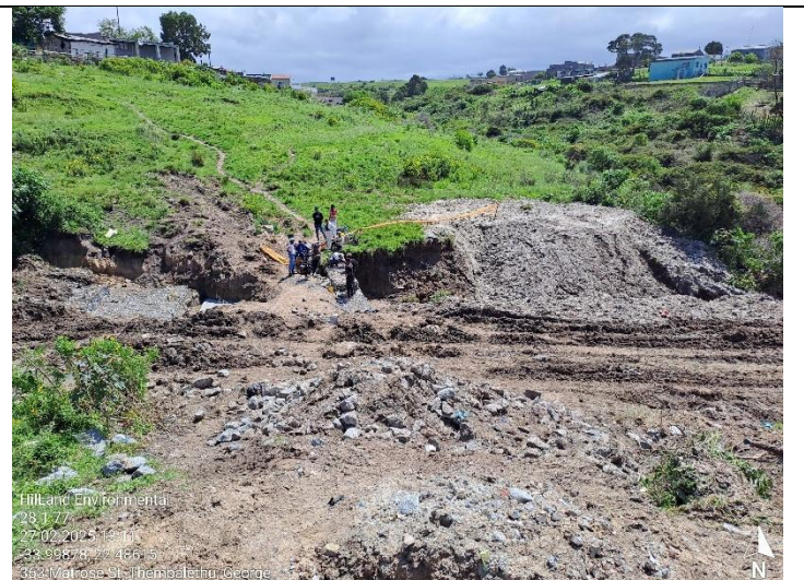
Construction site – pedestrians still use the walkway.
