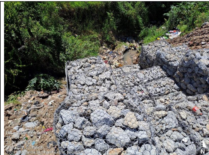
Construction progress (69a).
