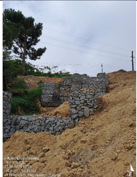
Construction progress – gabion installation. The slope will be shaped to tie in with the armorflex channel.
