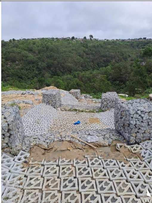
Construction site – silt is captured in the armorflex.
