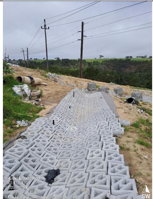
Shaping and installation of the armorflex in progress.
