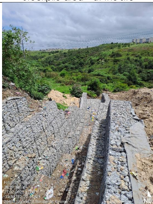
Construction progress – backfilling behind the gabion structure and shaping will start in due course.
