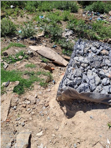
Final shaping and tie in at the ends of the gabion structure to be finalised – small concrete channel.
