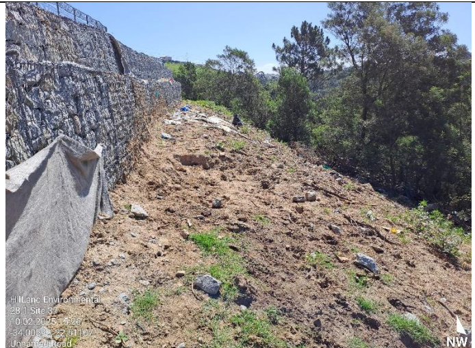
The slope below the gabion structure has been shaped.
