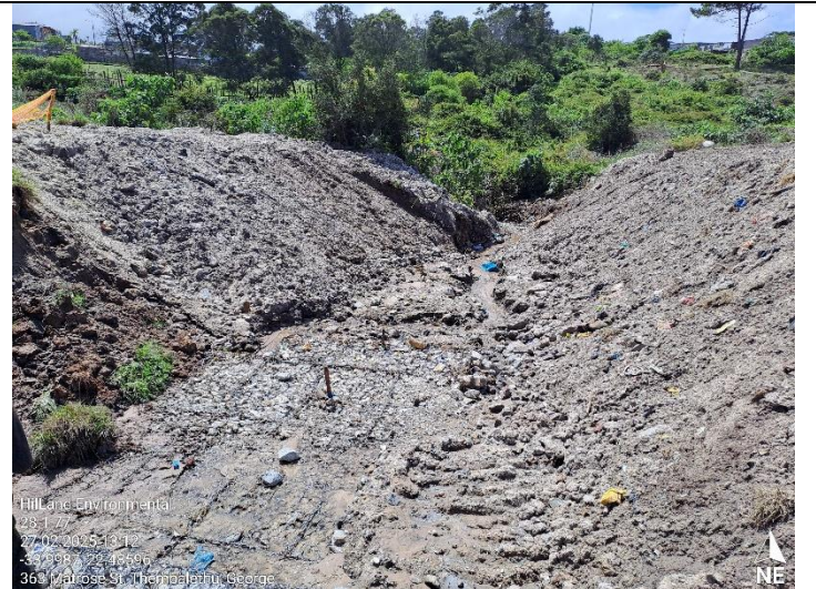
Downstream – gabion installed. Side slopes to be rehabilitated (topsoil) and erosion protection (mulch bags/ sandbags etc.) at the end of construction.
