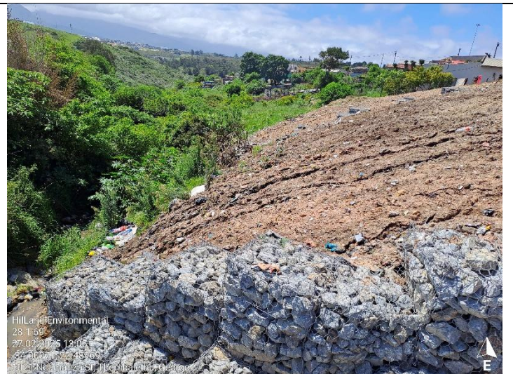
Contractor progress (69b) backfilling and shaping done – additional erosion protection (mulch bags or sandbags) to be used – where feasible.
