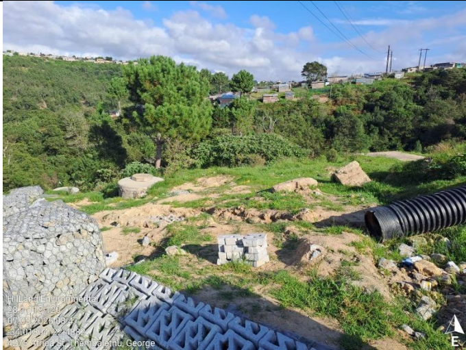
Construction site – existing erosion trenches will be rehabilitated at the end of construction.
