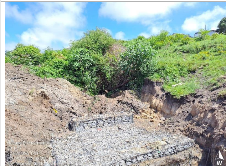
Upstream – gabion installed.
