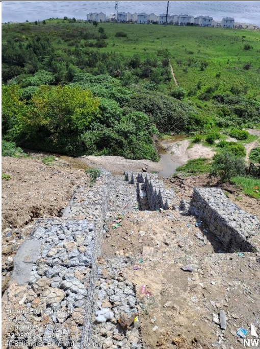
Gabion structure construction is completed. Note that the reno-mattress section captures silt as designed.
