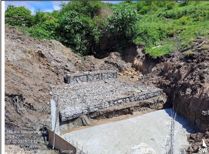
Construction in progress – temporary diversion in placed (left).
