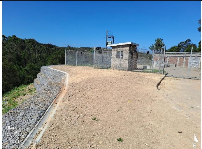
Backfilling completed – rehabilitation (topsoil and grass seed/sods) still to be completed.
