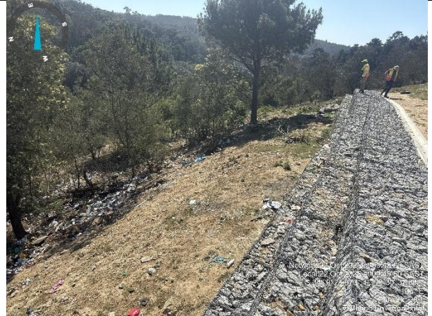
Backfilling completed – rehabilitation (shaping) has been done.
