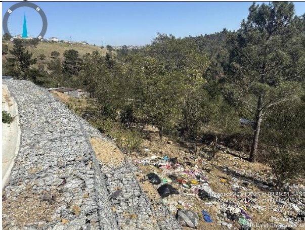
Final shaping and tie in at the ends of the gabion structure have been finalised.
