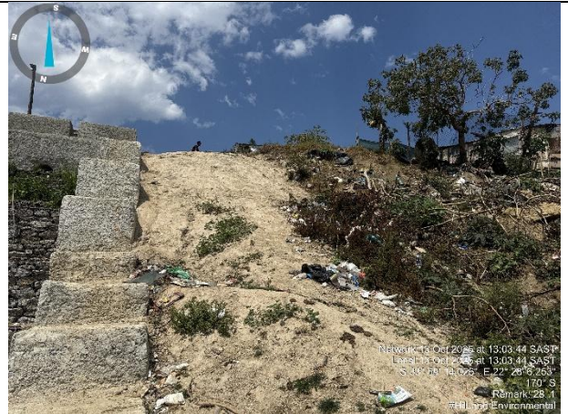
Erosion damage on the sides of the gabion structure has been backfilled and rehabilitated. Additional erosion protection has been installed (soil berms).
