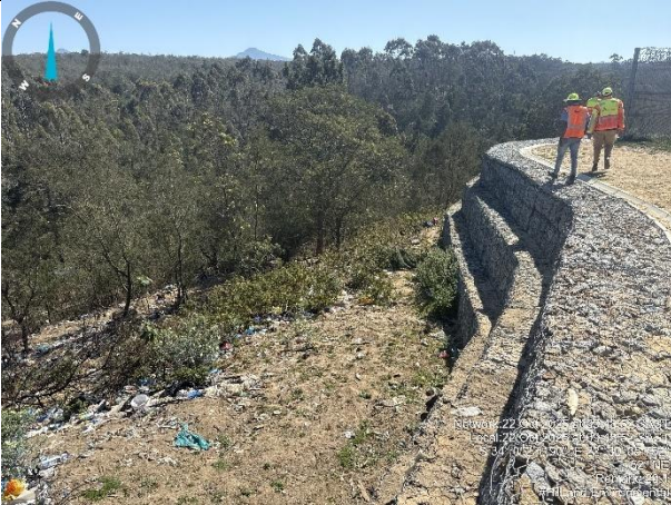
Gabion retaining wall construction completed. Continual dumping of waste and litter remains an ongoing issue.
