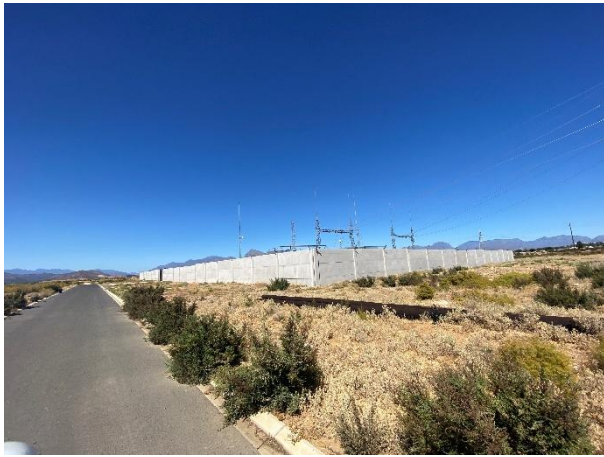
Condition of the site surrounding the Transhex substation.
