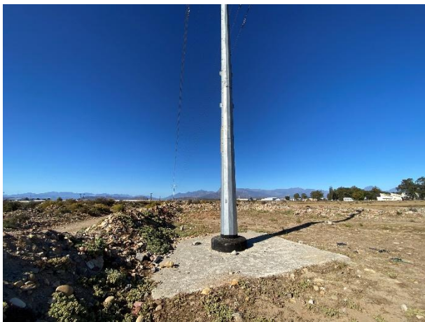
Completed Pylon 10 and footing as seen towards the south with public rubble dumping evident.
