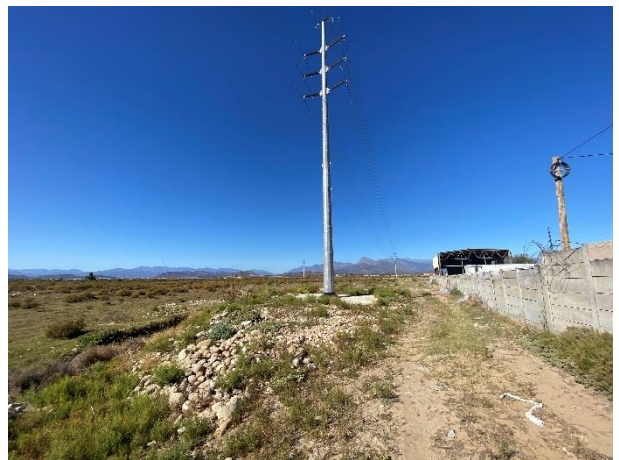
Completed Pylon 14 along the eastern boundary of the Worcester Industrial area.
