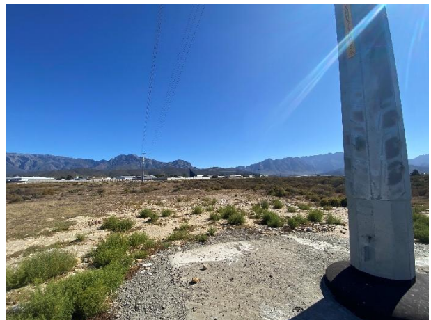
Completed Pylon 16 seen towards the north towards Pylon 15 and the Worcester Industrial area.
