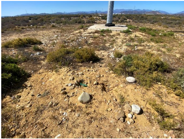
Completed Pylon 17 as seen towards the south. Pylon 17 is located immediately south of the R60.
