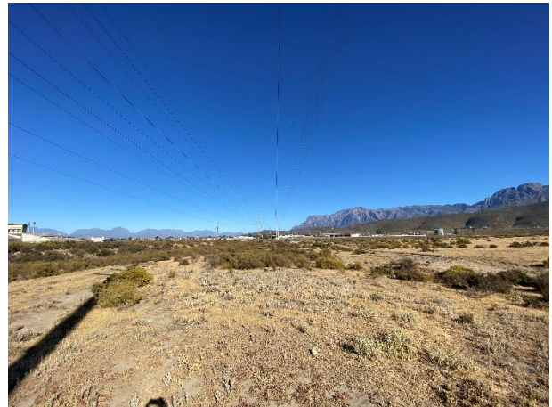
Completed Pylon footing 7 per Figure 3 as seen towards the west towards Pylon 6.
