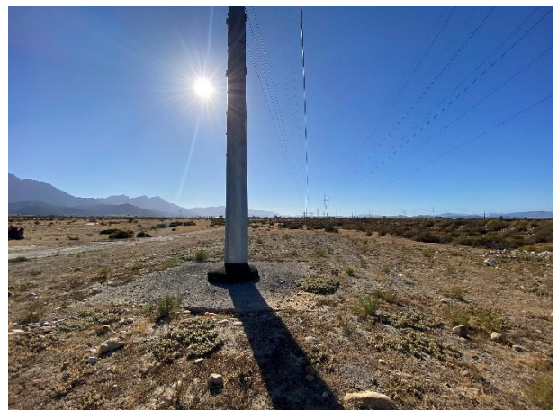
Completed Pylon footing 6 per Figure 3 as seen towards the east towards Pylon 7.
