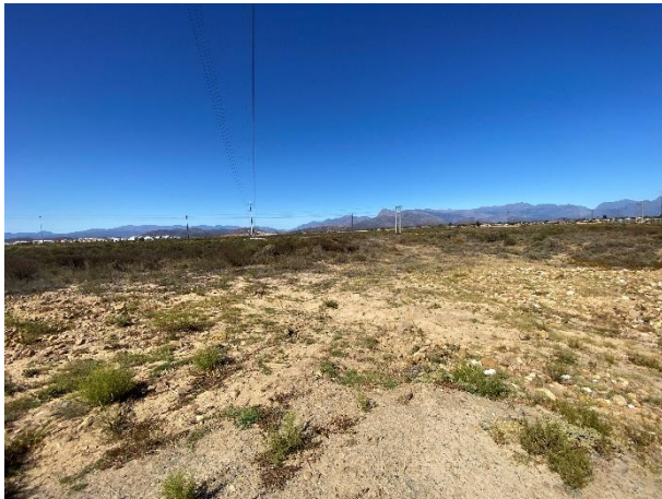
From completed Pylon 19 as seen towards the south towards Pylon 20.
