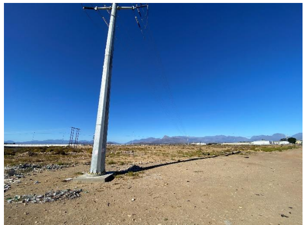
Completed Pylon 11 footing seen towards the south towards Raymond Pollet Drive.
