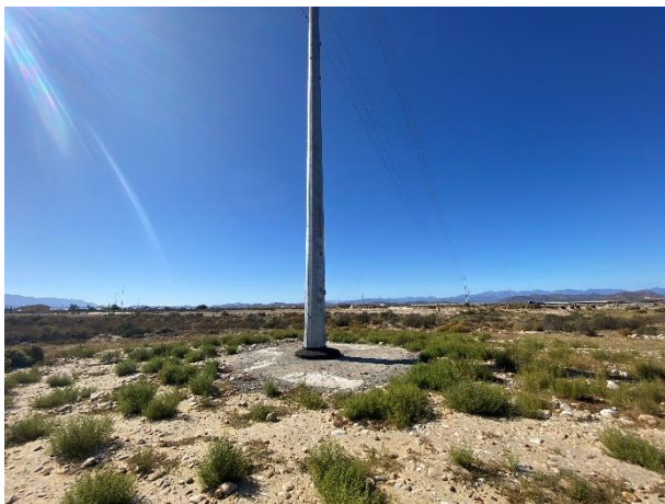
Completed Pylon 16 seen towards the southeast towards the R60.
