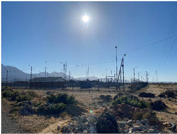
The Worcester Industrial substation, where the contractors camp was located.
