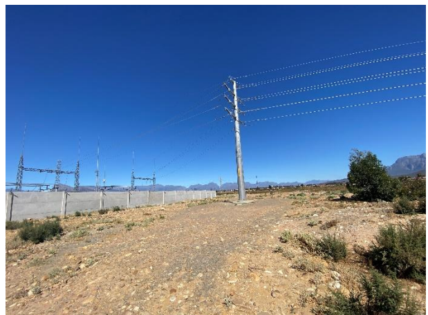
Completed Pylon 21 and footing immediately north of the Transhex Substation as seen from the tar road.
