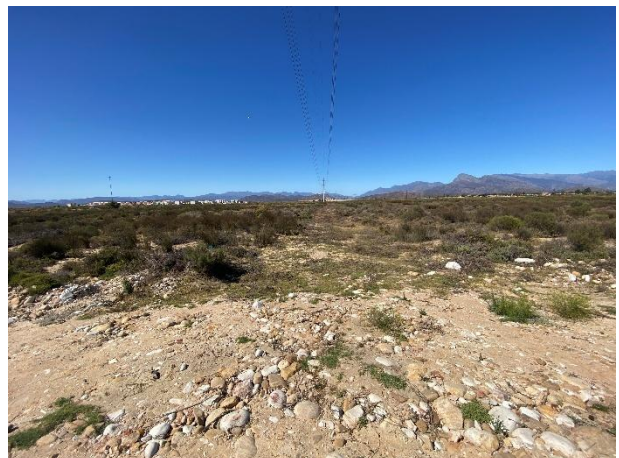
Brush cut vegetation between Pylon 20 and Pylon 21 as seen towards the south towards Pylon 21.
