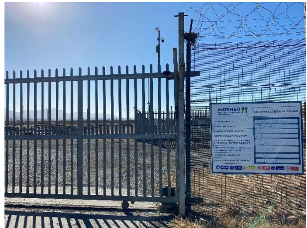
Notice board at the entrance to the Worcester Industrial substation.
