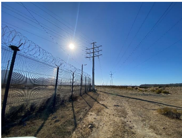
Completed Pylon 5 as seen along the substation fence in an eastern direction.
