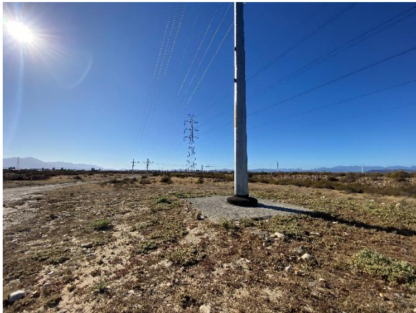
Completed Pylon footing 7 per Figure 3 as seen towards the east.
