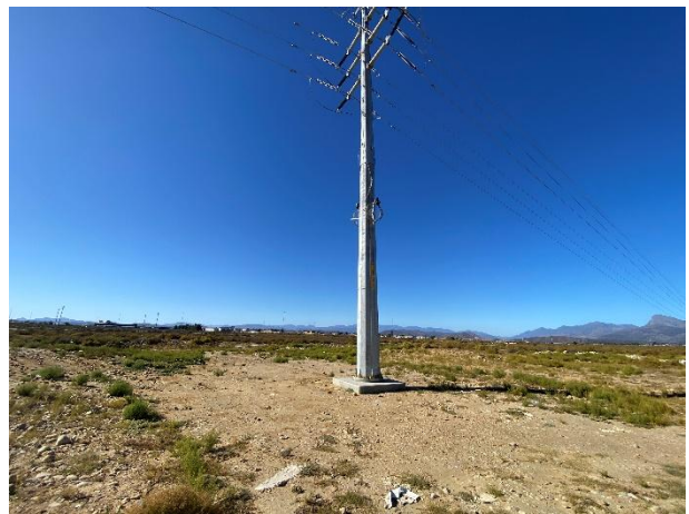
Completed Pylon 12 and footing seen towards the east towards the Hex River.
