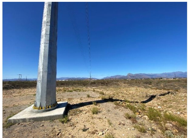
Completed Pylon 18 as seen towards the south towards Pylon 19.
