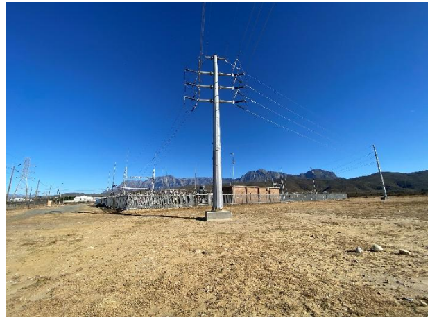
Pylon 5 adjacent to the Worcester Industrial substation erected as seen towards the northwest.
