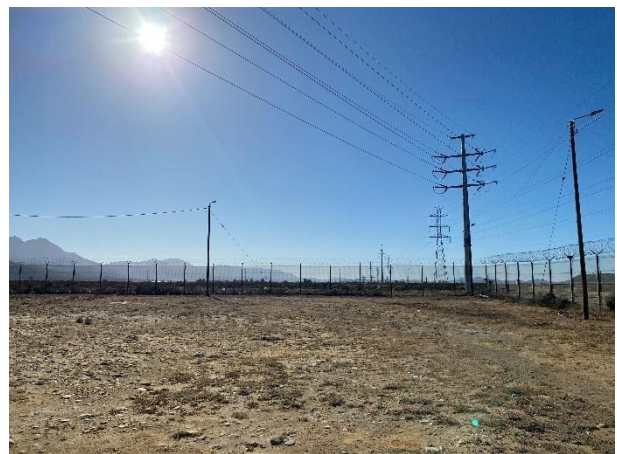
Contractors camp has been deestablished, and area rehabilitated.
