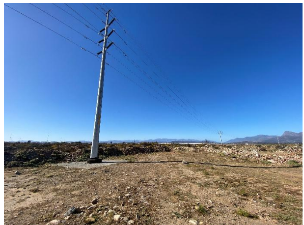
Completed Pylon 10 and footing as seen towards the east with public rubble dumping evident.
