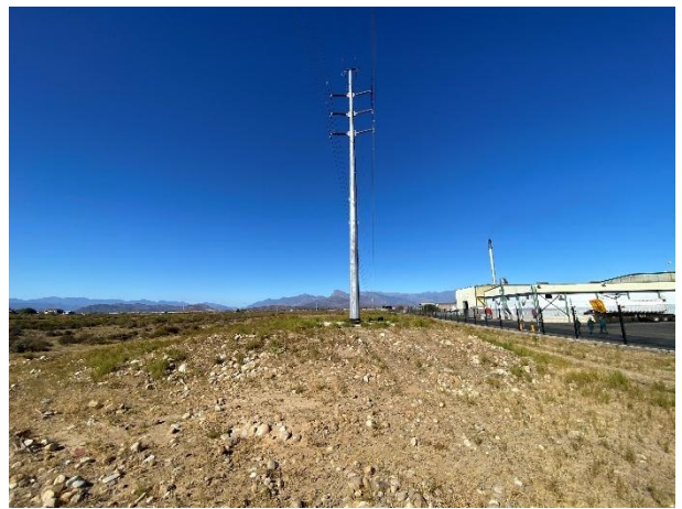
Pylon location 13 erected on a small platform along the boundary of Ceres Fruit Processors seen to the south.
