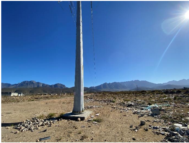
Completed Pylon 11 footing seen towards the north towards Pylon 9.
