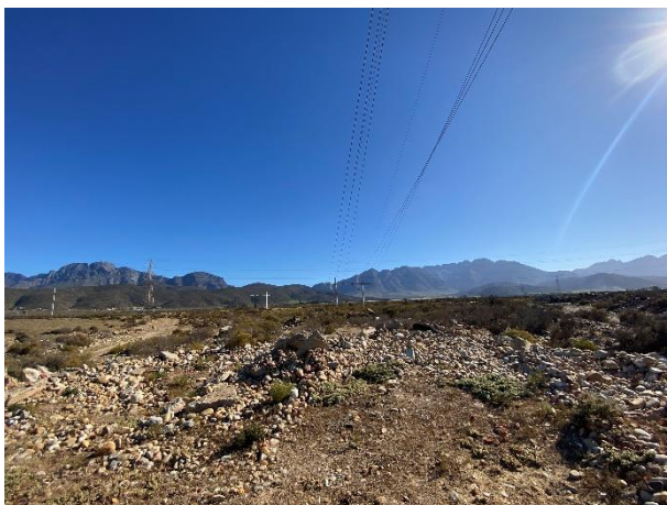
Condition of the site as seen from Pylon 10 towards Pylons 9 seen towards the north.
