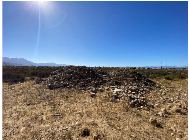
Excavated rock and stockpile on site north of Pylon 13 as seen towards the east.
