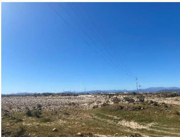
South of completed Pylon 16 seen south across the Hex River towards the R60 and Pylon 17 in back of picture.
