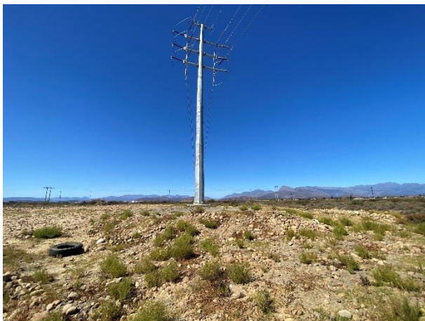
Pylon 18 footing and surrounds as seen towards the south.
