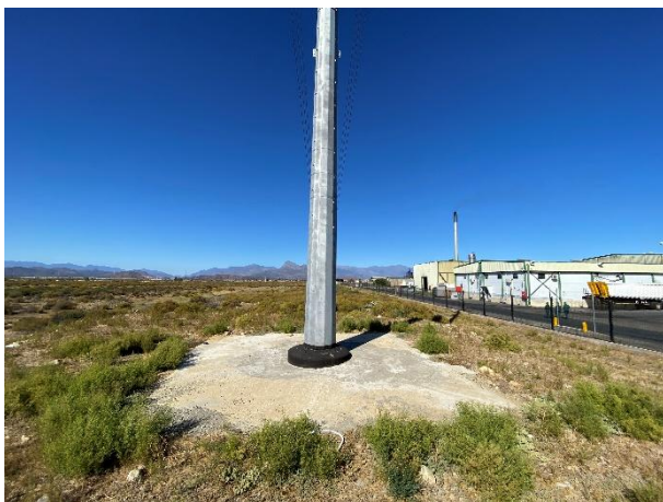
Completed Pylon 13 erected on a small platform along the Ceres Fruit Processors as seen to the south.
