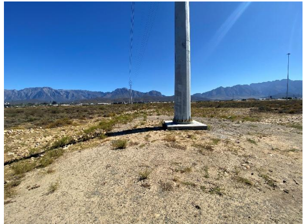
From completed Pylon 19 as seen towards the north towards Pylon 18.
