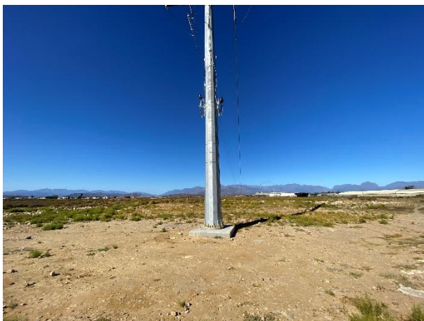
Completed Pylon 12 and footing seen towards the south towards Pylon 12.
