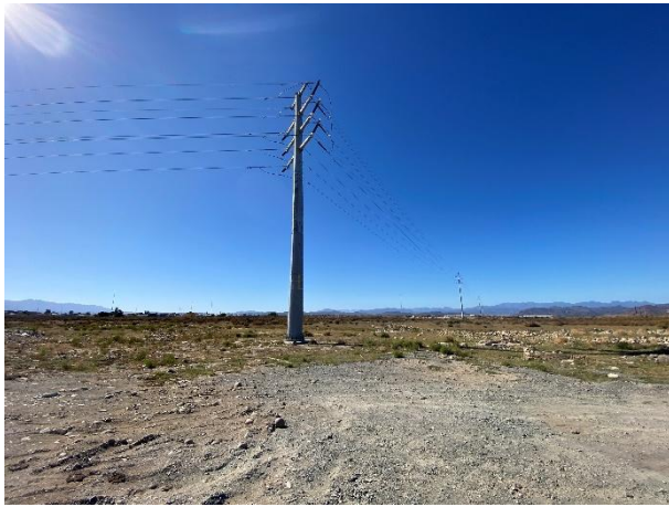
Pylon 15 as seen towards the southeast towards Pylon 16. An existing gravel access road in front of picture.
