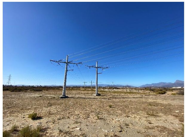
The condition of the site as seen from Pylon 8 southeast towards Pylon 9, area has been rehabilitated.
