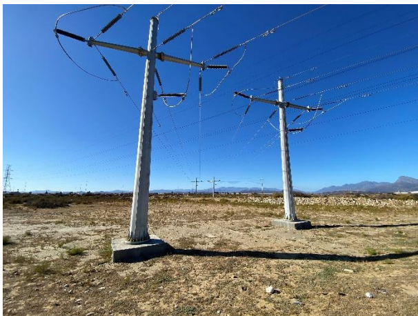
Completed Pylons 8 as seen towards the southeast towards Pylon 9.
