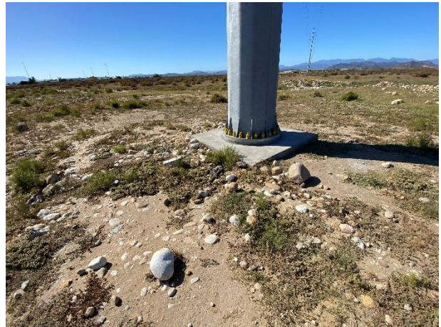
Completed footing of Pylon 15 as seen towards the southeast towards Pylon 16.
