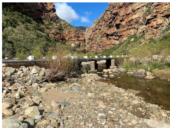
Maintenance of Causeway No 15 B2694 with cleared watercourse flow path.
