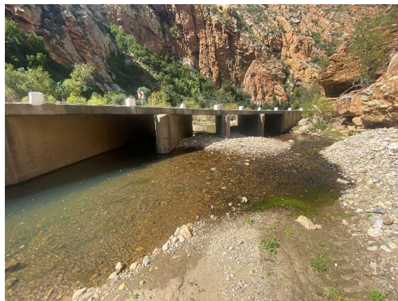
Downstream of causeway No 5 B2698A with cleared watercourse flow path.
