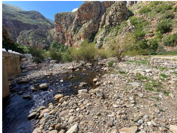
Upstream of causeway No 4 B2689 with a cleared watercourse flow path.
