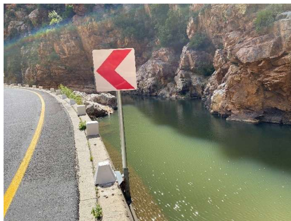
Damages of guard railings and notice boards repaired upstream of causeway 8.
