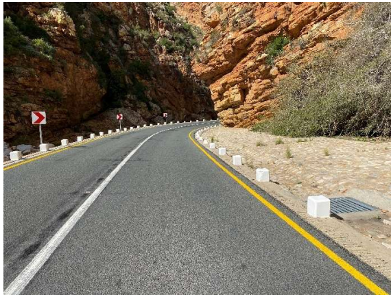
Newly installed stone-pitched side drains upstream of causeway 8.
