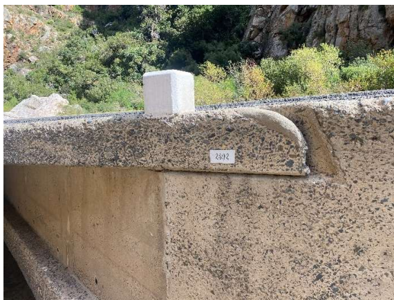
Newly installed structure number plate.
