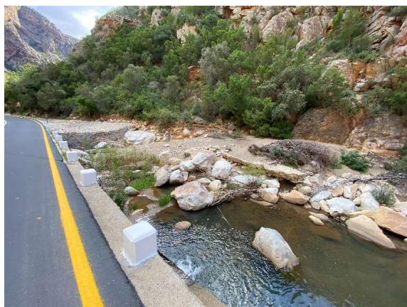
Upstream of Causeway No 7 B2698C with cleared watercourse flow path.
