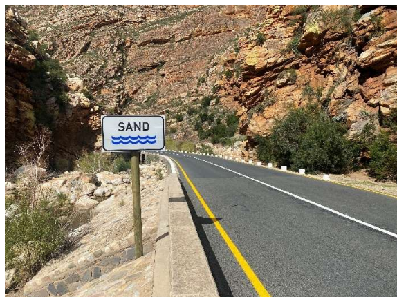
Indication of the sand river causeway.
