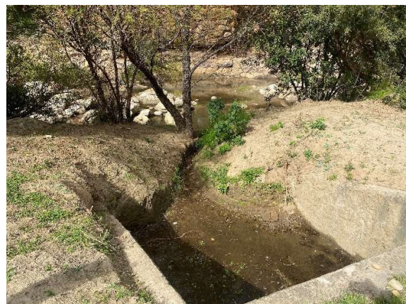
Cleared pipe culvert adjacent the causeway.
