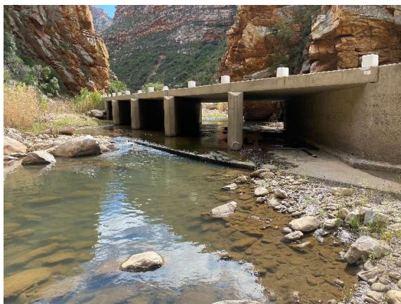
Downstream of Causeway No 10 with cleared watercourse flow path.
