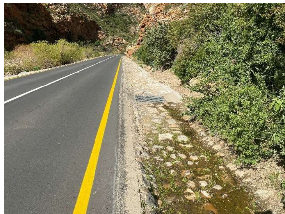
Stone-pitched side drains upstream of causeway 15.
