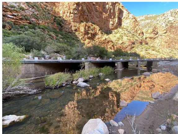
Sedimentation and vegetation debris removed downstream of causeway 16.
