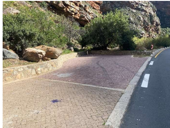
Repaired public parking area at causeway 11.
