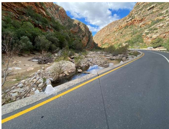
Cleared vegetation upstream of causeway 11.
