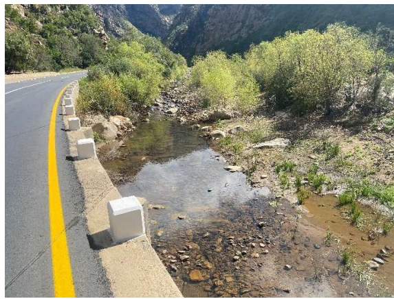
Vegetation debris cleared upstream of causeway 6.
