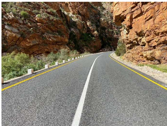
View of the road surface towards causeway no. 8.
