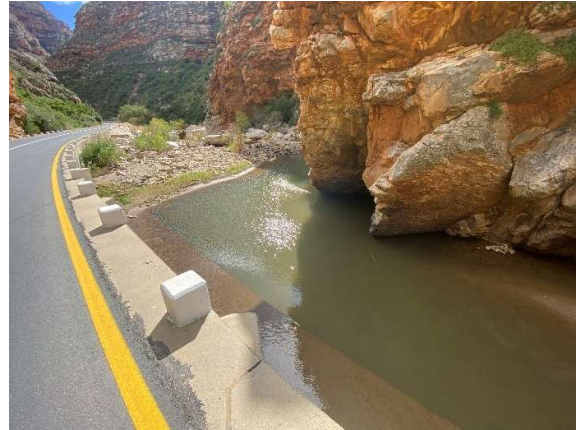
Evidence of reinstated cell joint fillers, and sealed deck expansion joints upstream of causeway 10.
