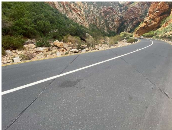
Evidence of strengthened bridge decks, reinstated cell joint fillers, and sealed deck expansion joints.
