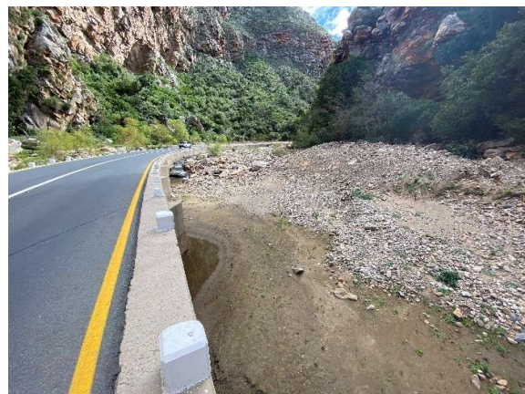
Downstream of causeway No 13 B2692A with no debris present and repair works evident.
