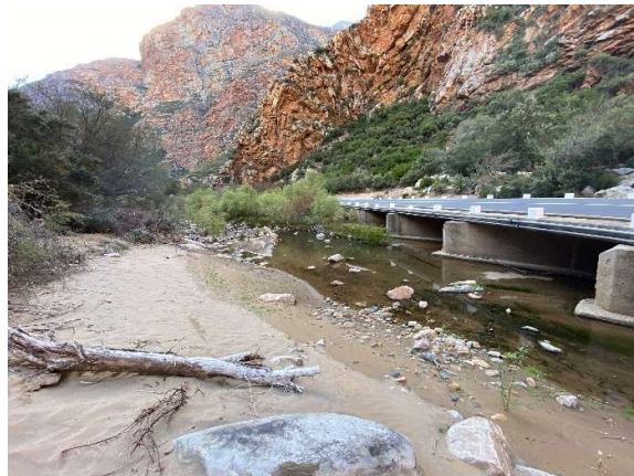
Potable water pipeline downstream of causeway 16 still in good condition.
