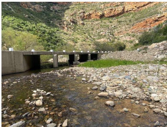
Downstream of causeway No 13 B2692A with cleared watercourse flow path and repair works evident.
