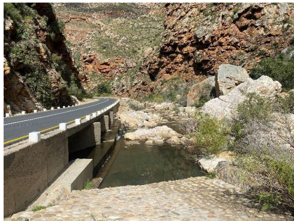
Stone-pitched side drains downstream of causeway 12.
