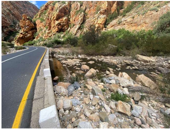
Visual downstream of causeway 9 with vegetation cleared.
