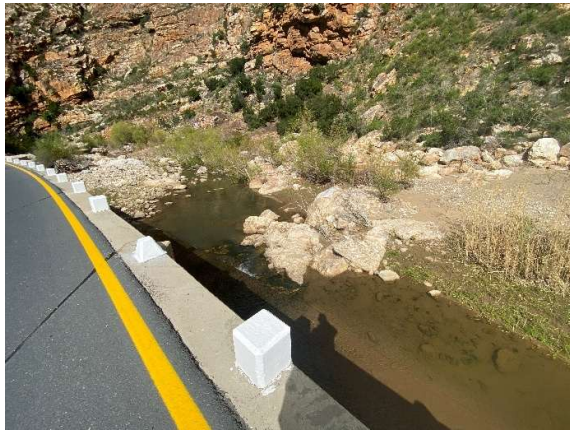
Upstream of causeway 10 where vegetation debris has been cleared.
