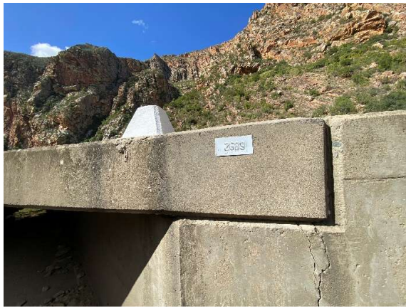
Newly installed structure number plates.
