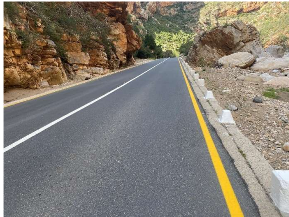
Visual of the road surface across causeway 14.
