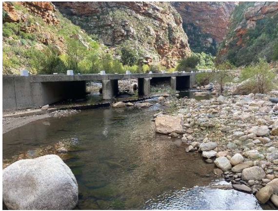
Downstream of Causeway No 11 with cleared watercourse flow path.
