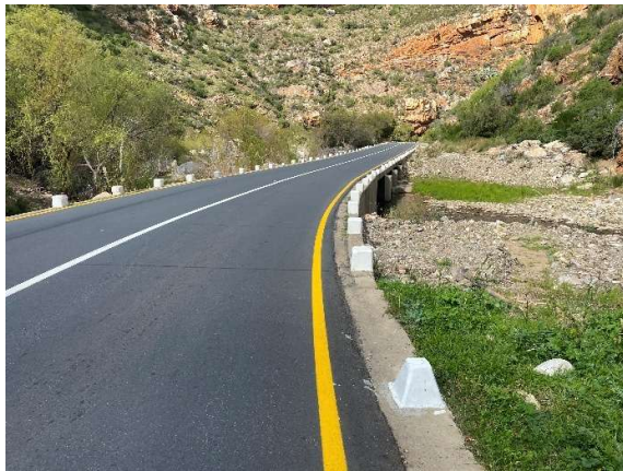
Downstream of causeway No 13 B2692A with cleared watercourse flow path and repair works evident.
