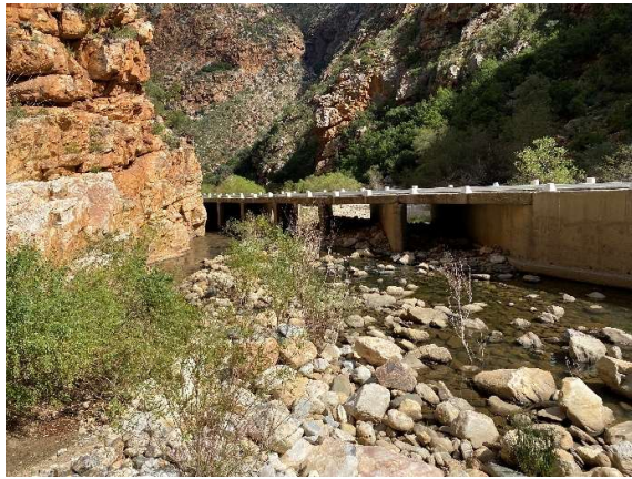
Maintenance of Causeway No 8 B2690 with cleared watercourse flow path.
