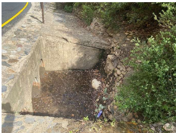
Cleared pipe culvert adjacent the causeway.
