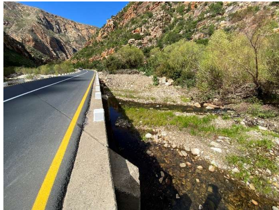
Repaired spalling and cracking with fibre polymer modified cementitious repair mortar.
