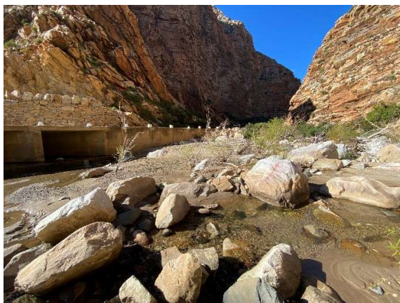
Downstream of causeway No 18 B2696 with cleared watercourse flow path.
