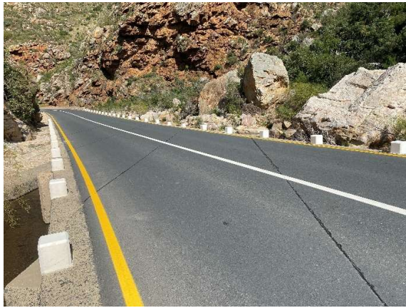
Repaired deck edge breaks and cell joint fillers upstream of causeway 12.
