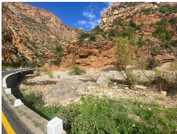
Downstream of causeway No 5 B2698A with cleared watercourse flow path.
