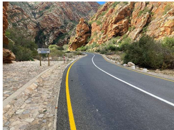
Newly installed stone-pitched side drains at causeway 9.
