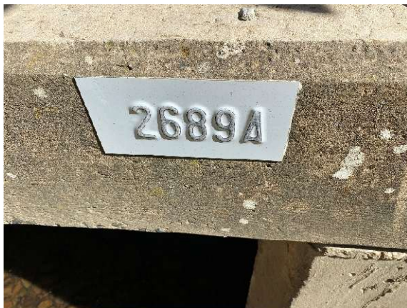
Newly installed structure number plates.
