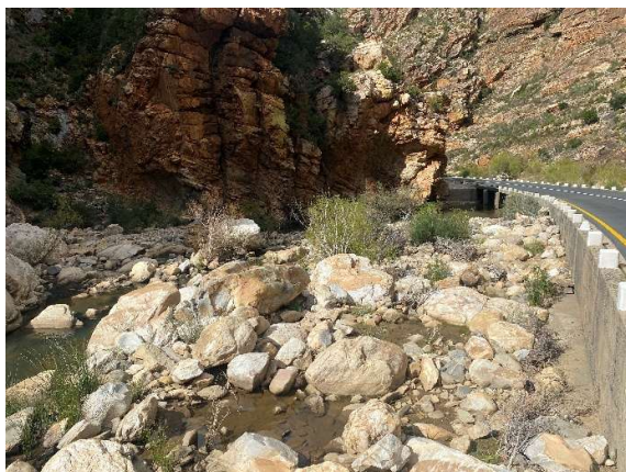
Upstream of the bridge deck at causeway 10 vegetation cleared and damages repaired.
