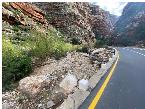
Cleared vegetation downstream of causeway.
