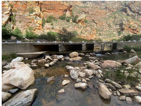
Maintenance of Causeway No 9 with cleared watercourse flow path.
