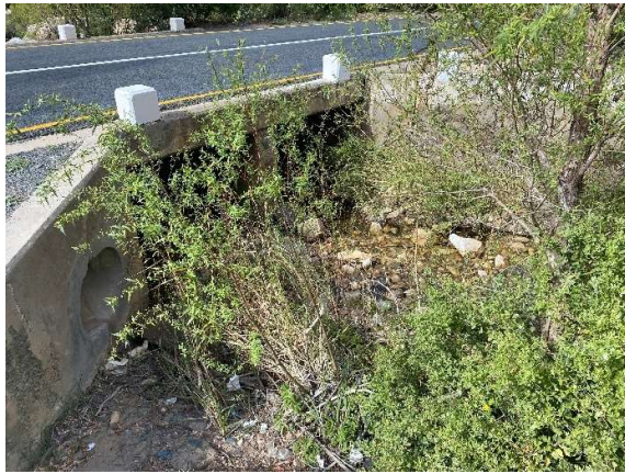
Cleared and revegetated culvert along causeway 15.
