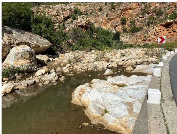
Repaired deck edge breaks upstream of causeway 8.
