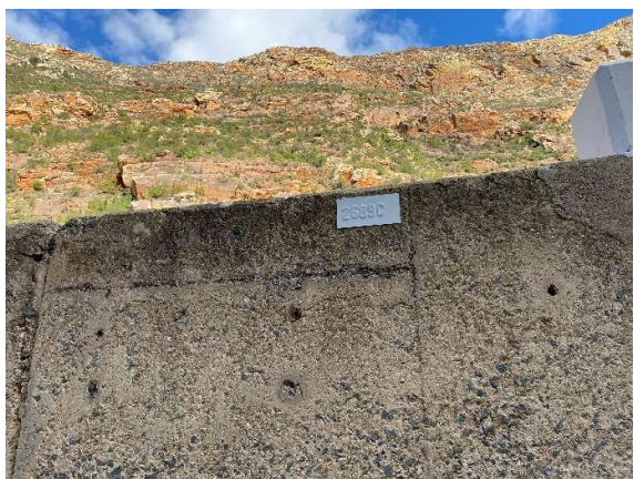
Newly installed structure number plate.
