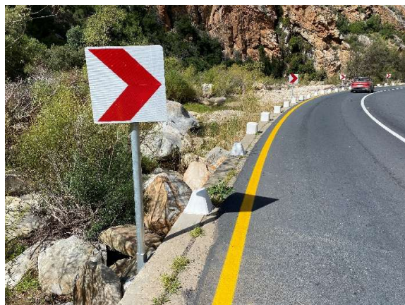
Repaired traffic notice boards.
