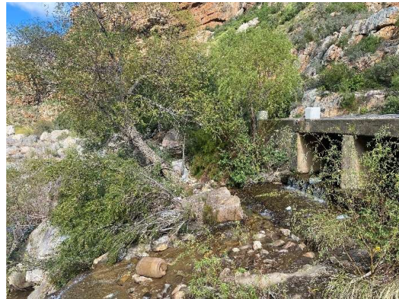
Cleared and revegetated culvert along causeway 15.
