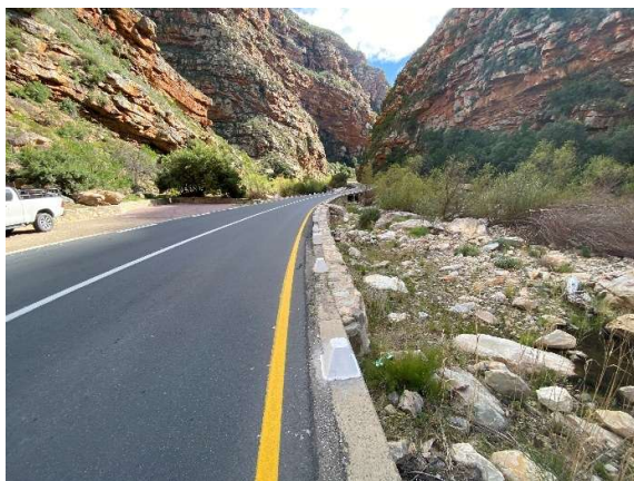
Repaired side of the road where material was displaced.
