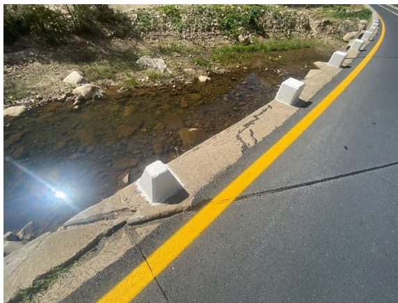
Vegetation debris cleared upstream of causeway 6.
