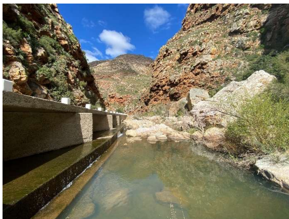
Downstream of Causeway No 12 B2692 with cleared watercourse flow path.
