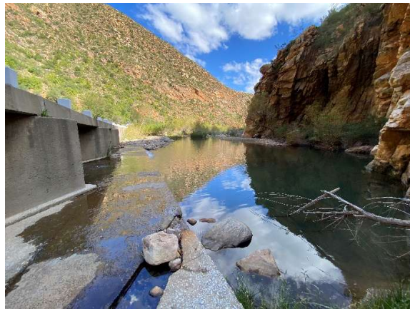
Downstream of causeway No 4 B2689 with a cleared watercourse flow path.
