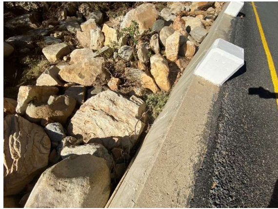
Repaired bridge edge breaks with stormwater and erosion control measures upstream of causeway 8.
