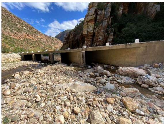
Visual upstream of the of the causeway with vegetation and sedimentation removed.
