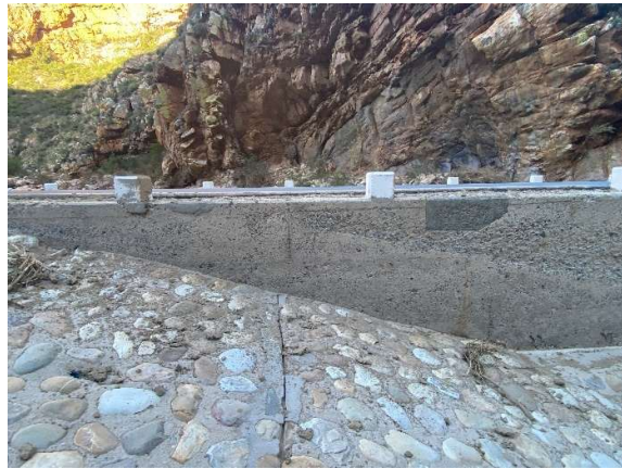
Repaired and strengthened deck edge breaks.
