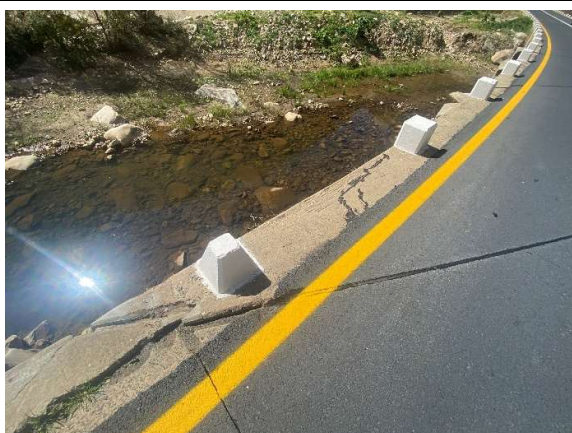
Repaired cell joint fillers and mortar works downstream of causeway 6.
