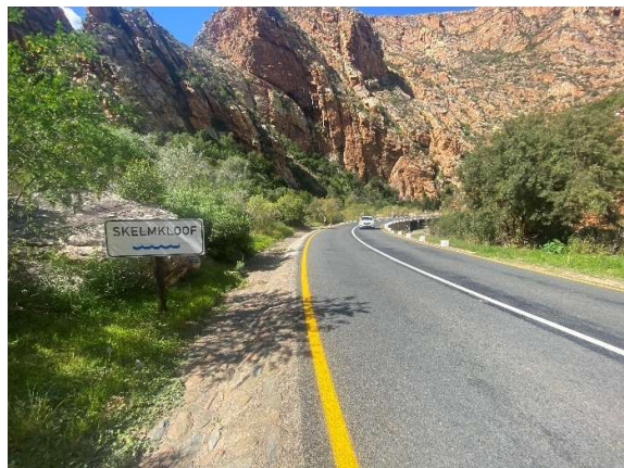
Indication of the skelmkloof causeway and stone-pitched side drains.
