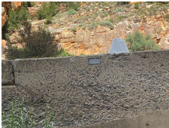
Newly installed structure number plate downstream of causeway 9.
