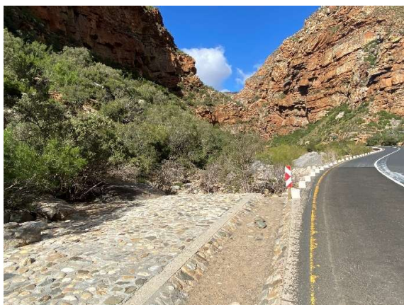
Stone-pitched side drains downstream of causeway 15.
