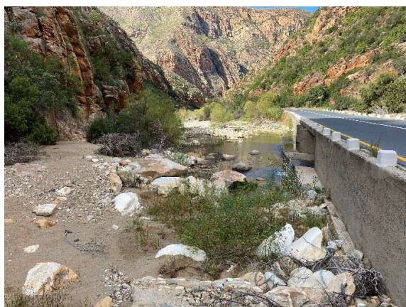
Downstream of Causeway No 7 B2698C with cleared watercourse flow path.
