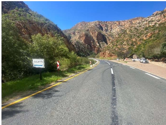
Visual of the bridge deck at causeway 6 as seen towards De Rust.
