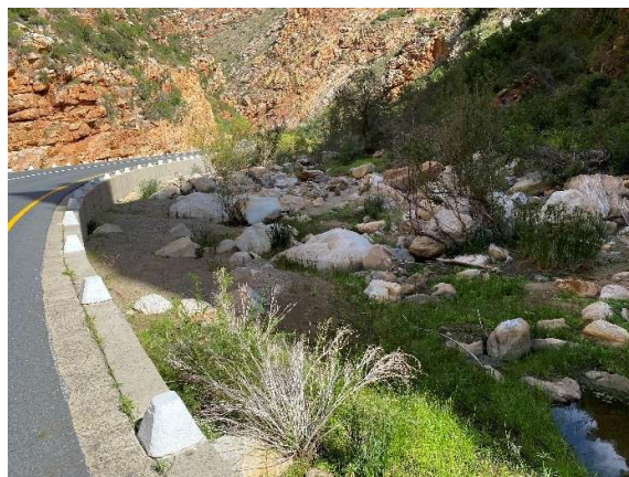
Damages of bollards repaired after the initial audit findings.
