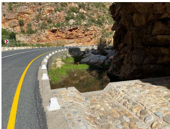
Newly installed stone-pitched side drains downstream of causeway 8.
